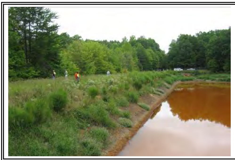
Upstream face of chemical washdown pond.
