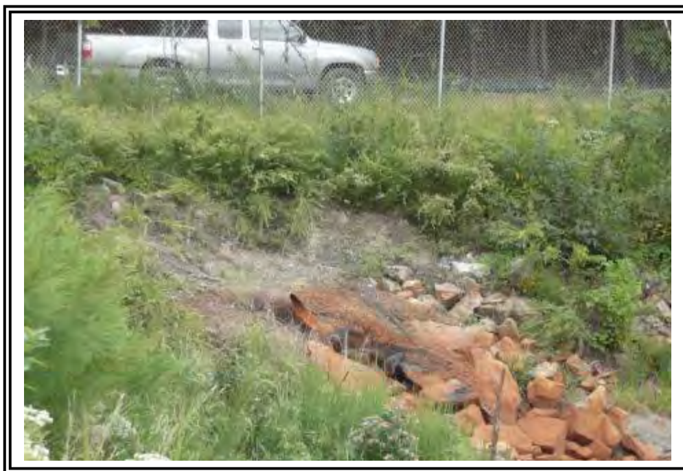
Chemical washdown pond inlet.
