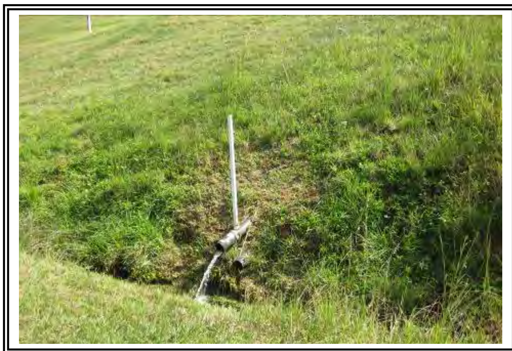
Horizontal drains from rip rap repair.
