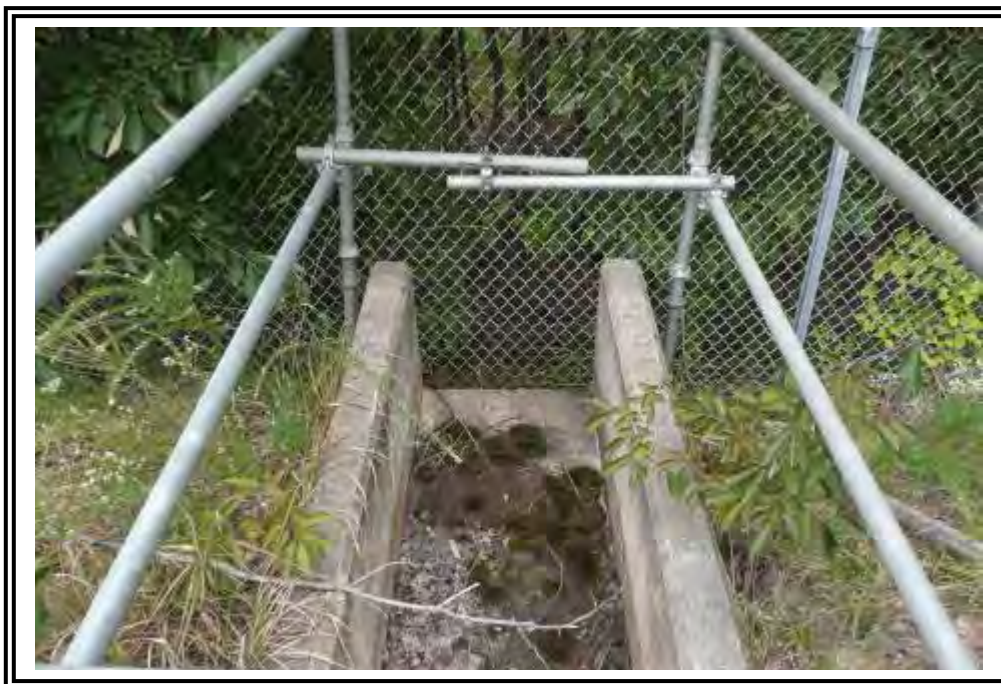
Chemical washdown pond overflow structure.
