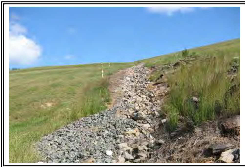
East (right groin) downstream. Drainage ditch.
