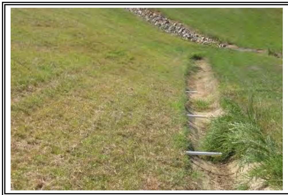
Horizontal drains at EL 720 bench, west side.
