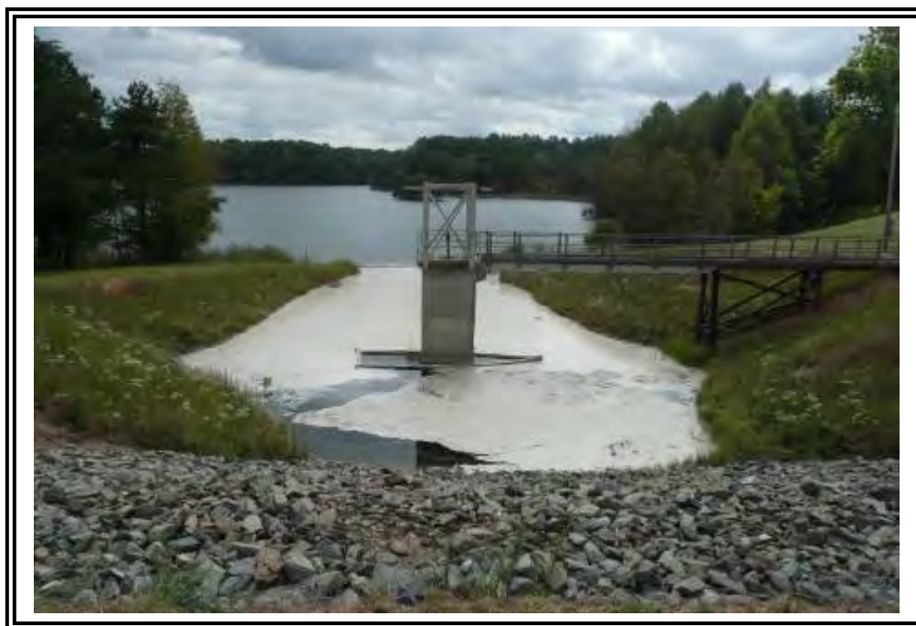
Ash tower outlet structure.
