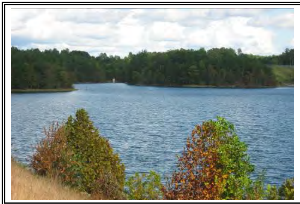
View of old outlet structure.
