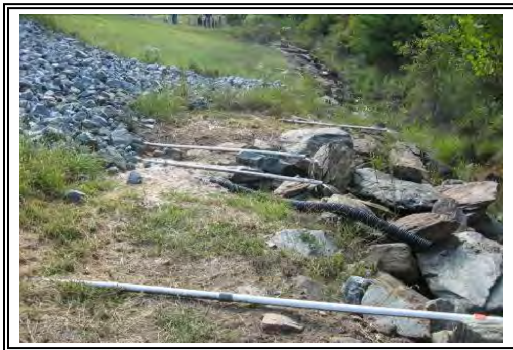
Horizontal drains from rip rap repair.
