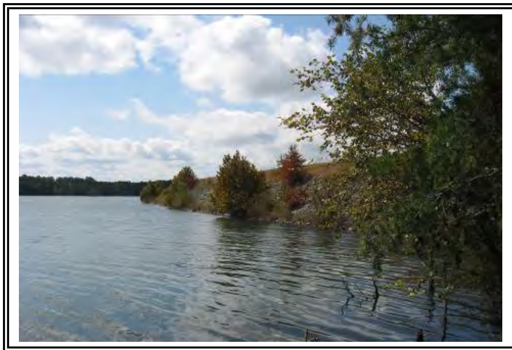
Upstream face, east side.
