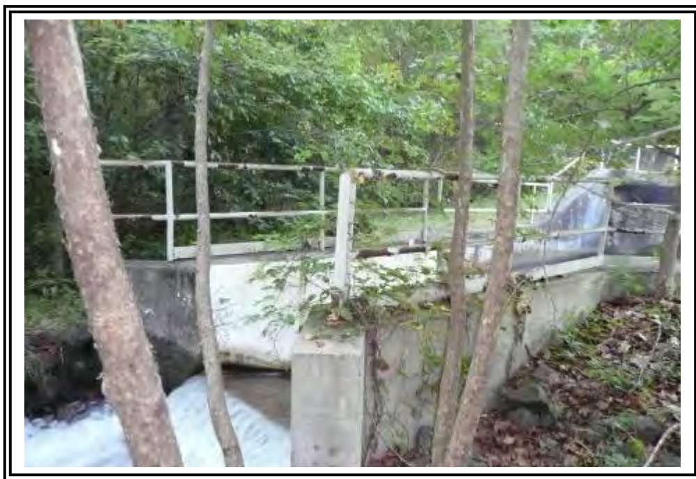
Downstream view of outlet flume.
