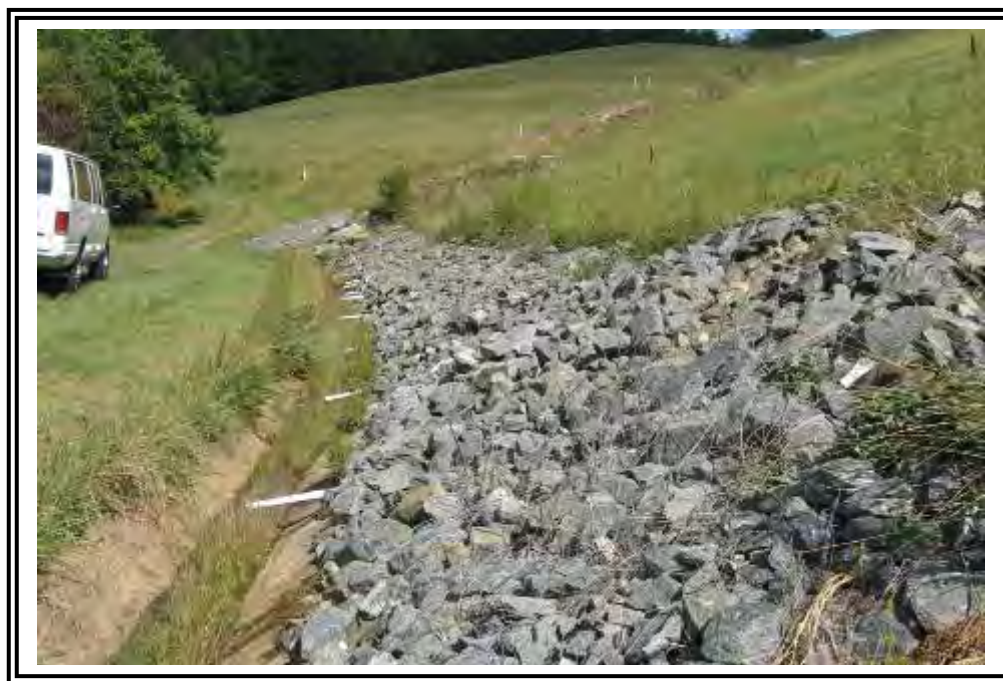
Rip rap repair with horizontal drains at EL 670 bench.
