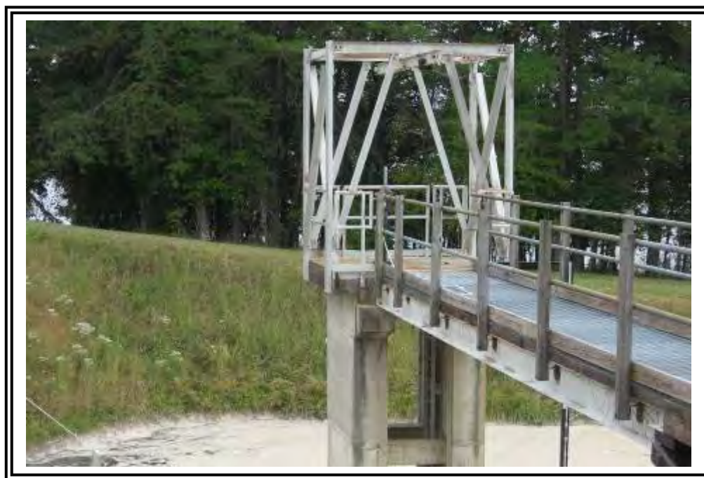
Ash tower outlet structure.
