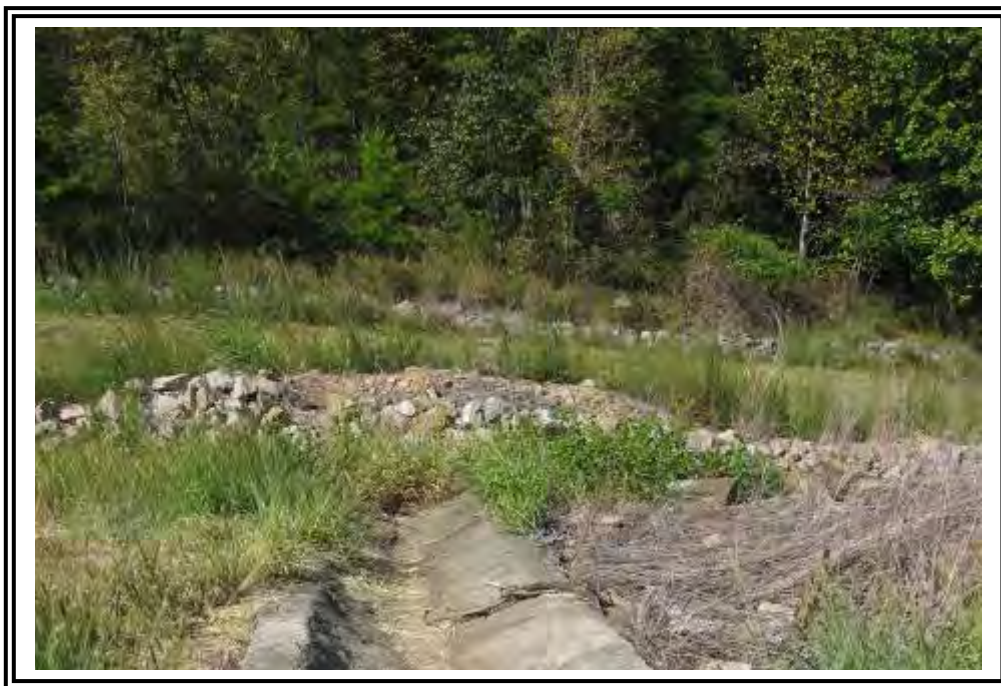
Precast drainage structures west (left) groin.
