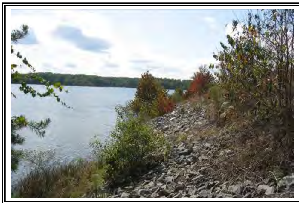
Upstream face, east side.
