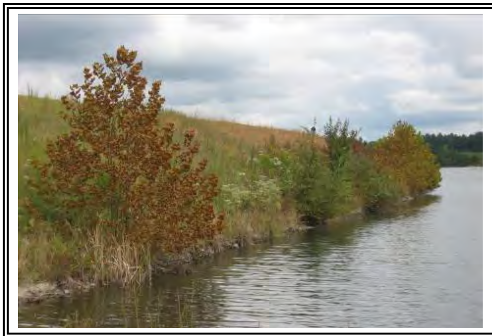
Upstream face of ash dike, west side.
