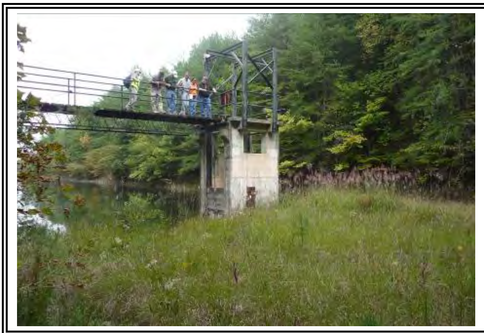
Abandoned ash tower outfall structure.
