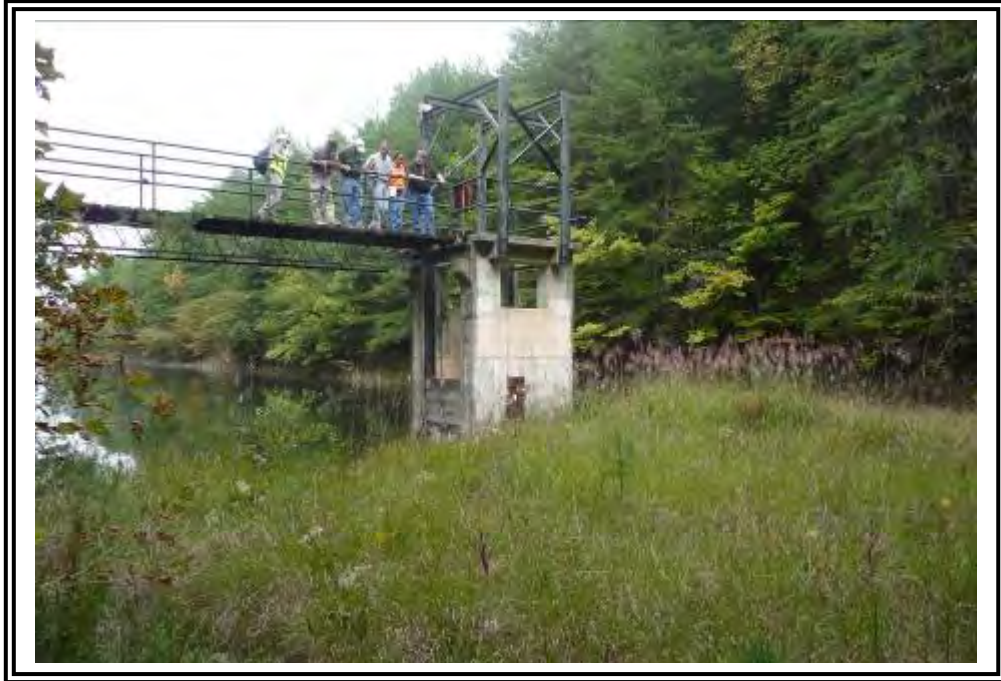
Abandoned ash tower outfall structure.
