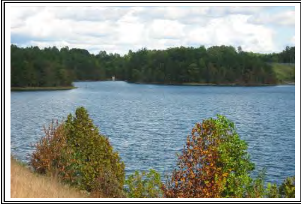
View of old outlet structure.
