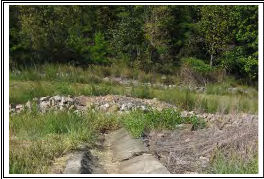
Precast drainage structures west (left) groin.
