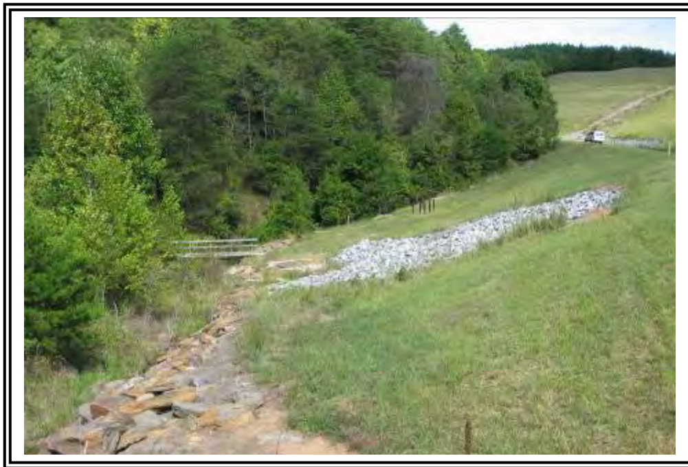
Drain swale and rip rap repair. Bridge to Parshall flume.
