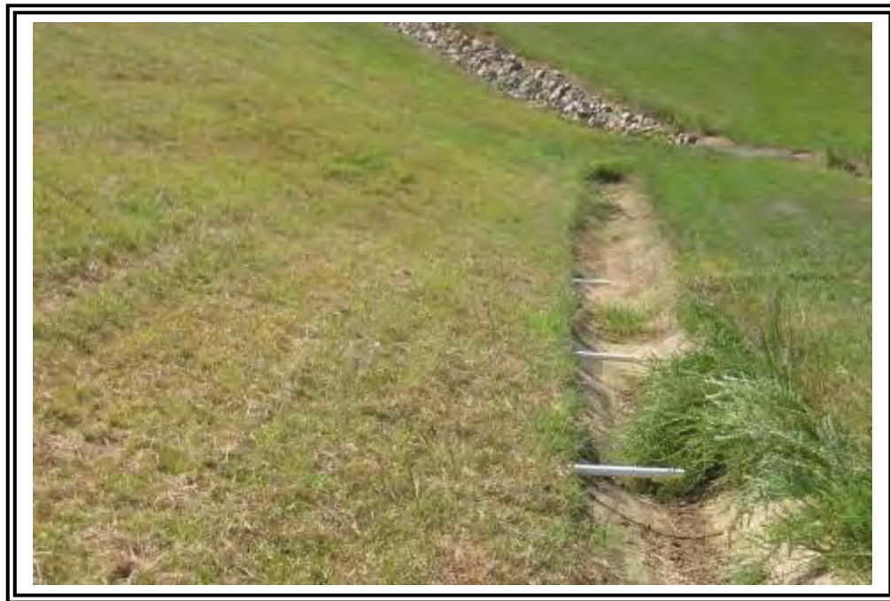
Horizontal drains at EL 720 bench, west side.
