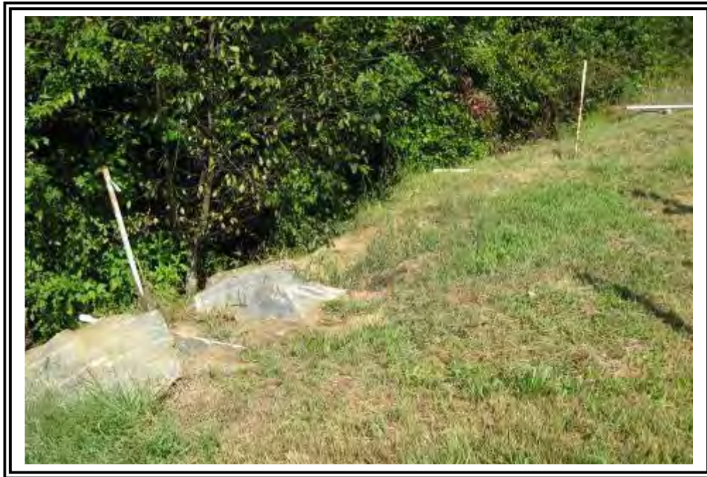
Slope instability noted in prior inspection report.
