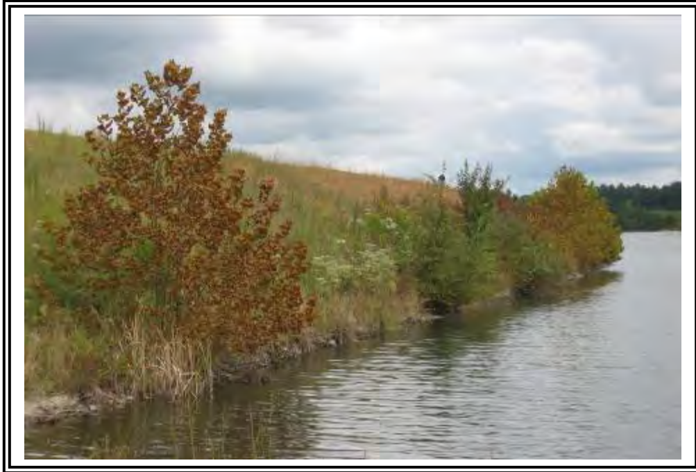
Upstream face of ash dike, west side.
