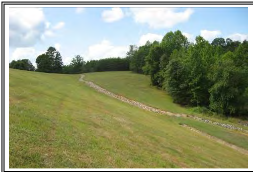
Downstream face of ash dike and west groin.
