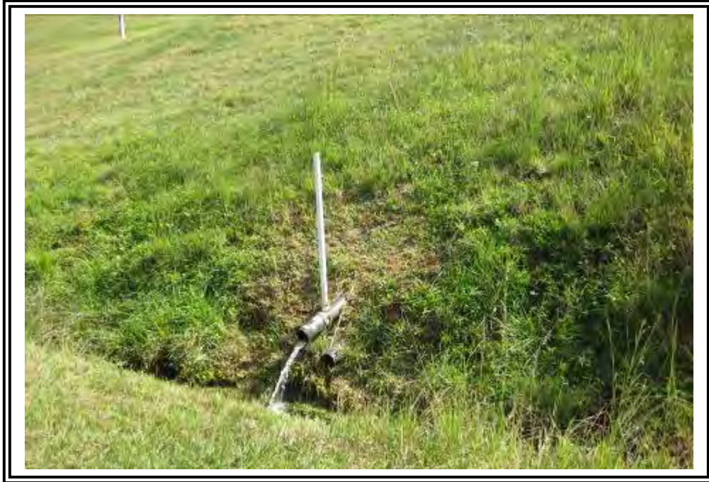
Horizontal drains from rip rap repair.
