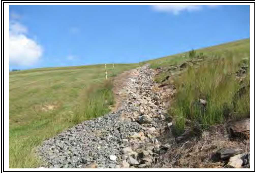
East (right groin) downstream. Drainage ditch.
