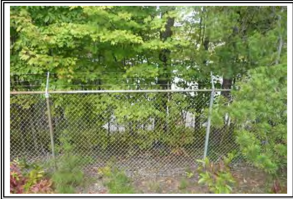
Downstream face of chemical washdown pond.
