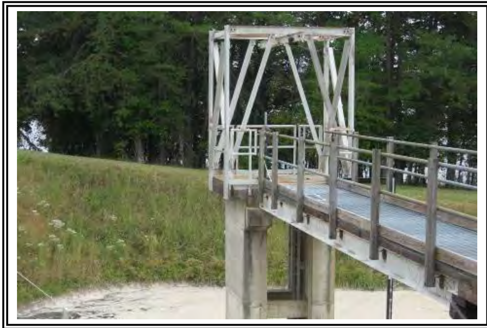
Ash tower outlet structure.
