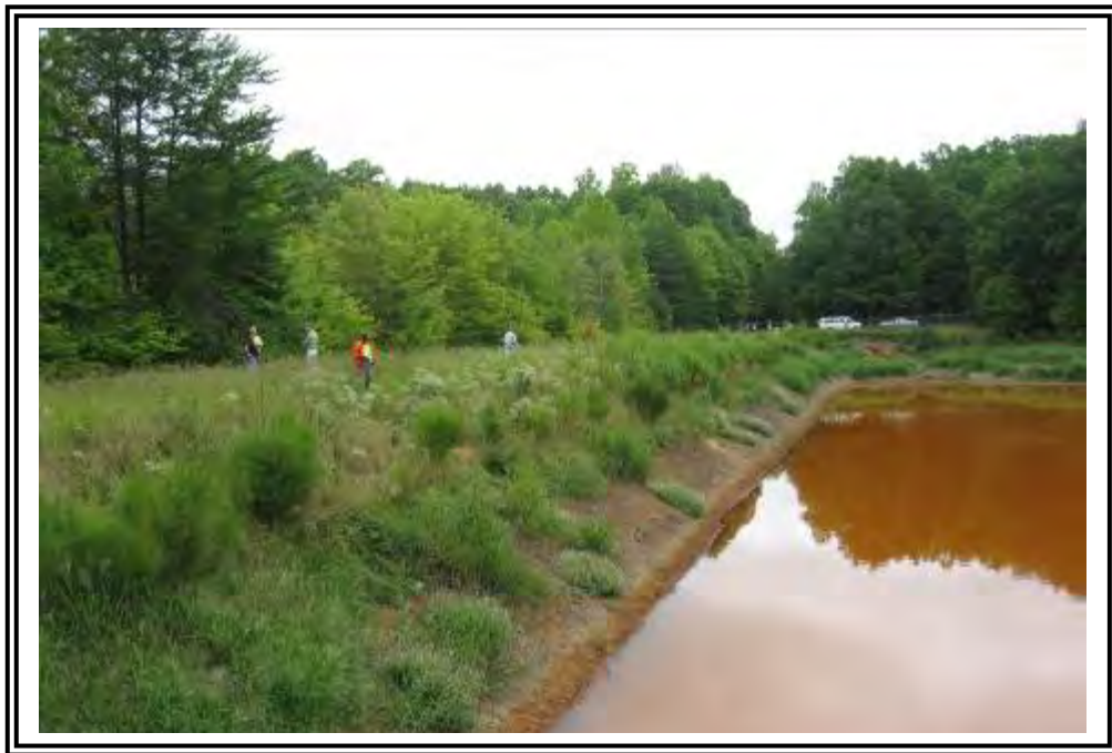
Upstream face of chemical washdown pond.
