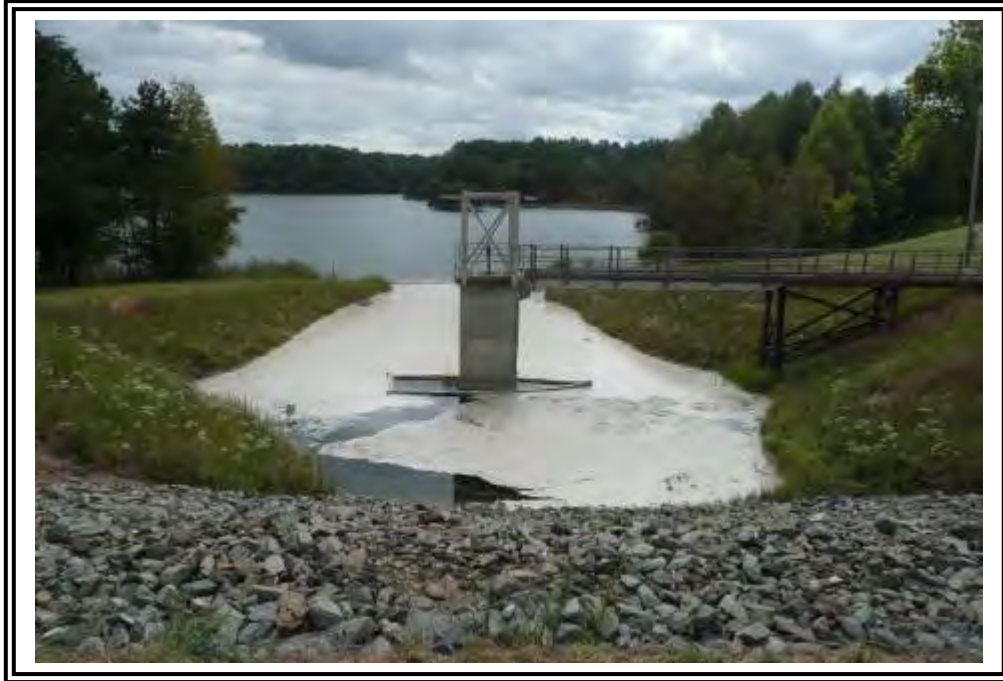
Ash tower outlet structure.
