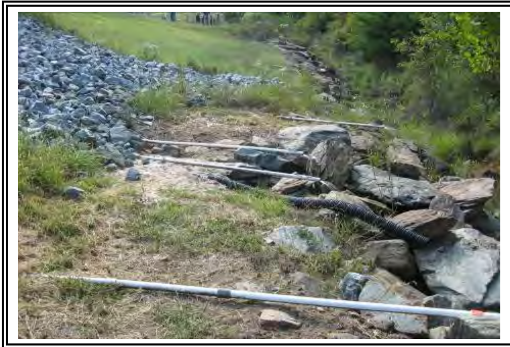
Horizontal drains from rip rap repair.
