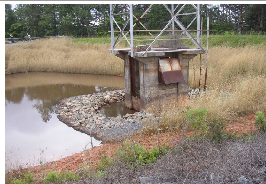
#55 Drop Inlet for Retained Ash Basin
