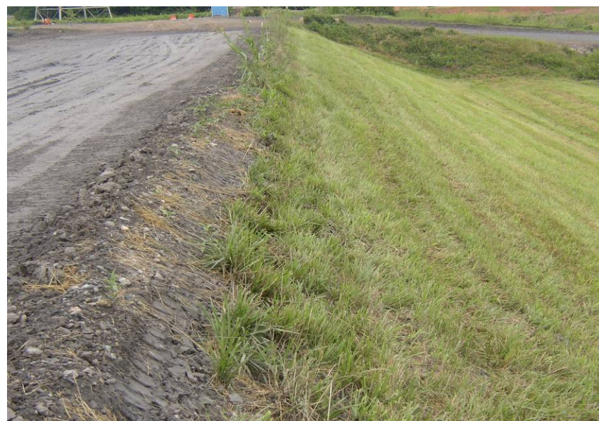
#62 Crest of Western Portion of North Dike
