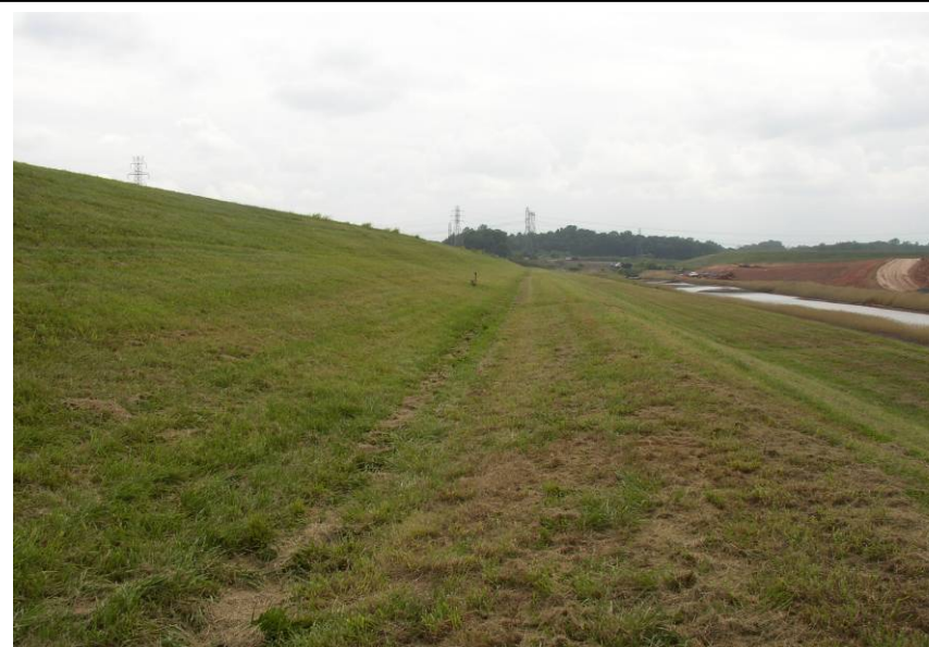
#44 Upper Berm of North Dike - 15 Feet Wide @ Elev. 630
