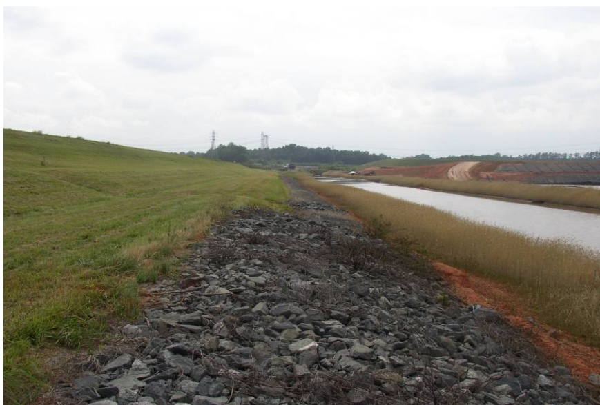
#45 Downstream Toe of North Dike
