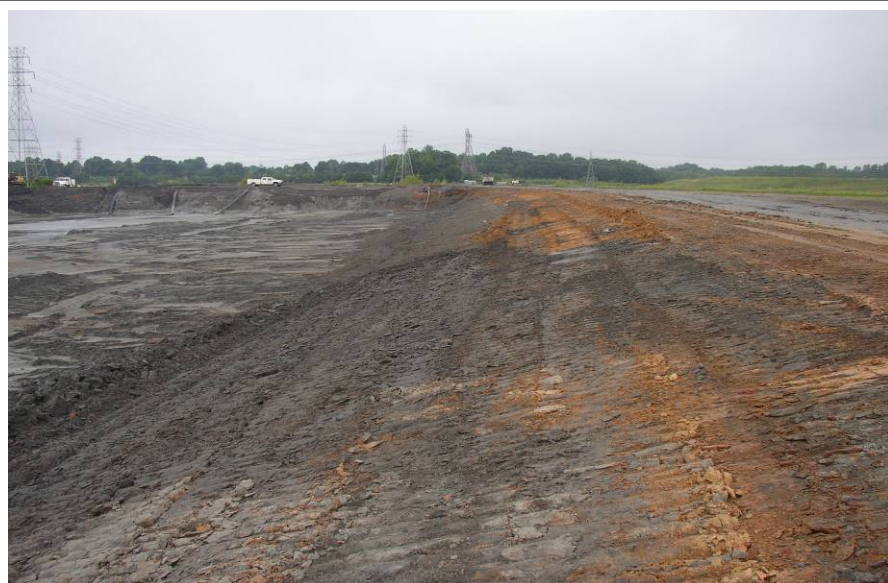
#58 Upstream Slope of Cell 3. Ash Excavated to Depth of About 20 Feet. No Water Impoundment
