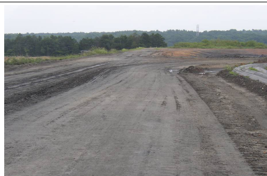
#51 Widened Crest in Cell 3 to Create Haul Road. Width Increased from 15 to about 45 Feet.
