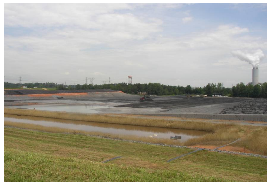
#18 New Ash Landfill Construction
