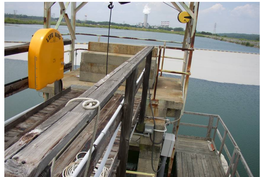
#29 Drop Inlet Structure - Note Concrete Stop Logs and Crane
