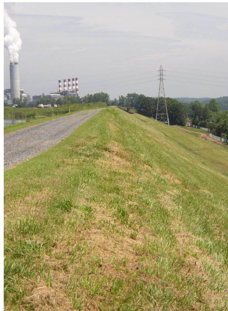
#6 Crest & Downstream Slope of East Dike
