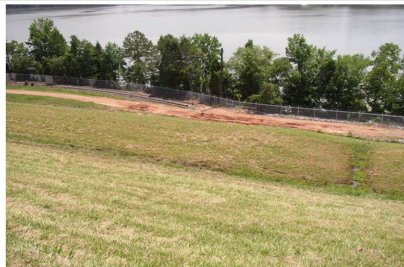
#13 Eroded Area of Downstream Toe Road from Operations due to Installation of Chain Link Fencing and Mowing
