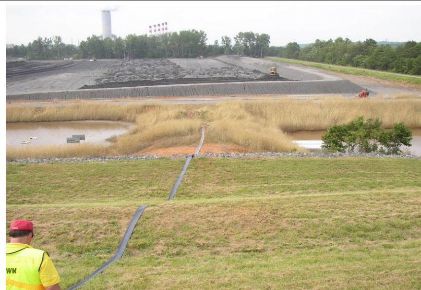
#43 Stabilizing Berm from Crest
