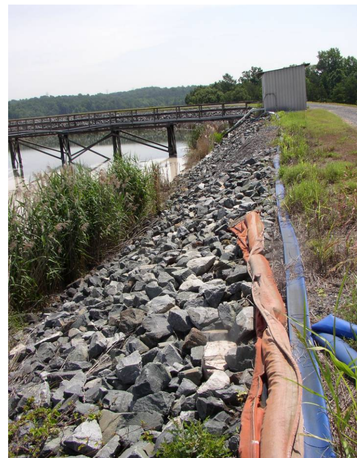
#3 Upstream Slope & Bridge to Drop Inlet Structure
