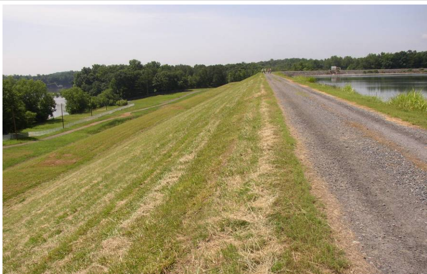
#11 Maximum Section Portion of East Dike – Note Wet Area at Toe and Local Berm Erosion
