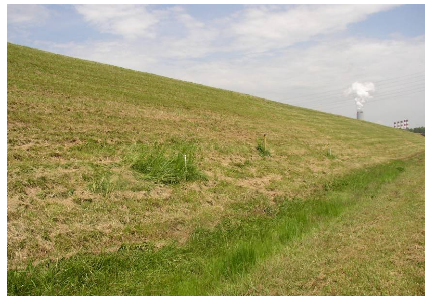
#26 Piezometers and Observation Wells Along Toe Stability Berm at South End of East Dike. (Note Standing Water at Toe)
