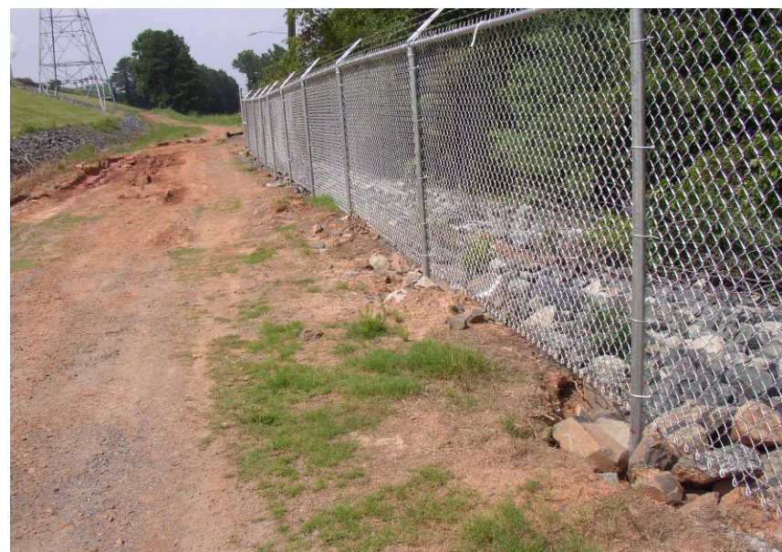
#39 Local Erosion / Rutting of Downstream Toe Road. Near Central Portion of East Dike
