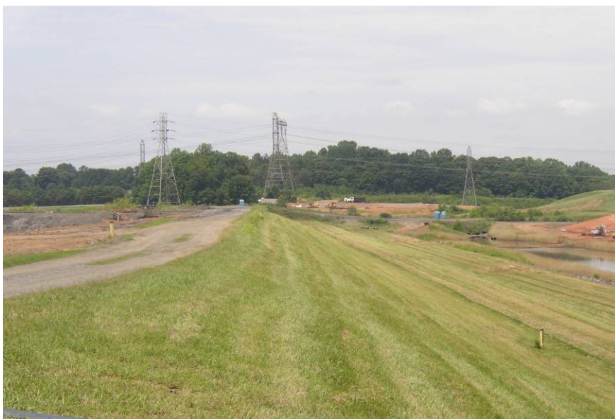
#20 Overview of Central Portion of North Dike
