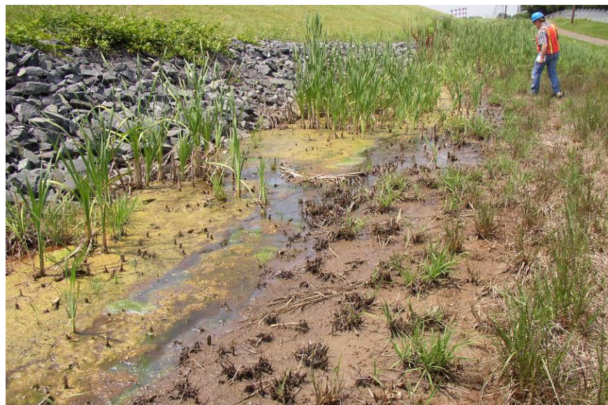
#36 Local Minor Seepage & Standing Drainage Flow at Downstream Toe of South End at East Dike
