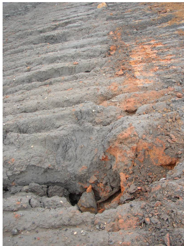
#59 Erosion in Ashfill in Upstream Excavated Slope of Cell 3
