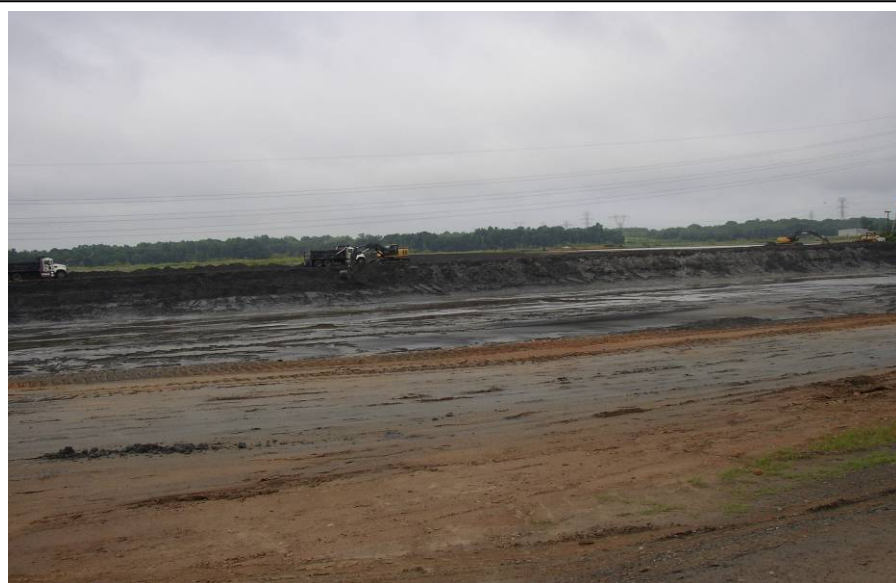
#57 Cell 3 Excavated to About 20-Foot Depth. No Water Impounded Due to Dewatering by Pumping.
