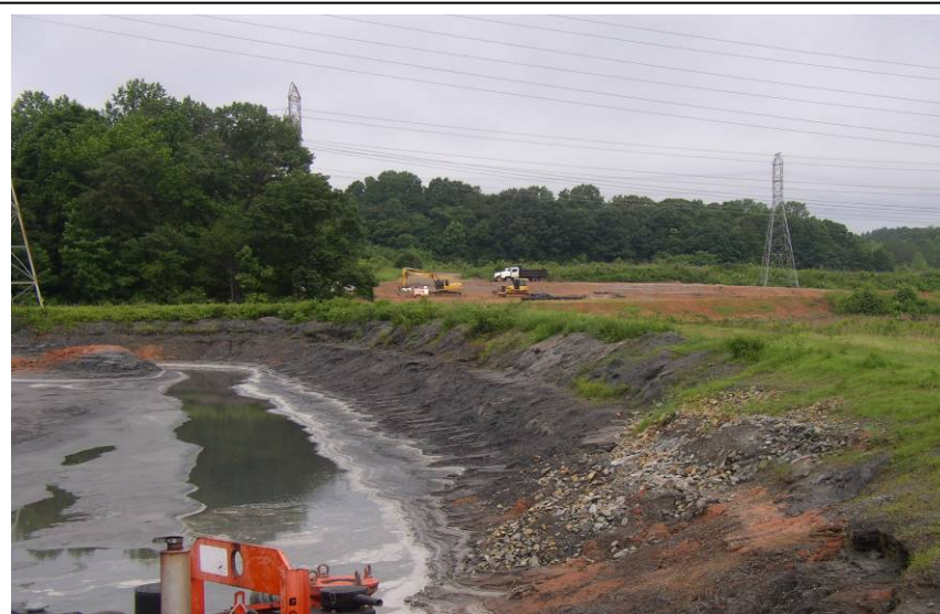
#63 Western Bend in North Dike at Cell 1 - Note Erosion in Upstream Slope of Ashfill
