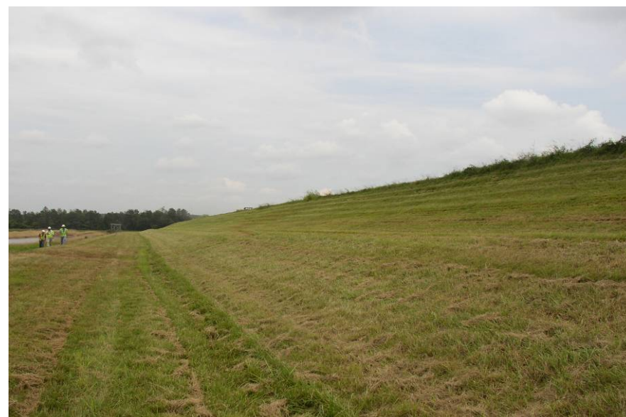
#47 Lower Berm of North Dike – 25-Foot-Wide Berm @ Elev. 625
