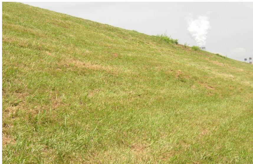
#27 Note Minor Bulging of Lower Portions – Upper Slope Above Stability Berm of East Dike
