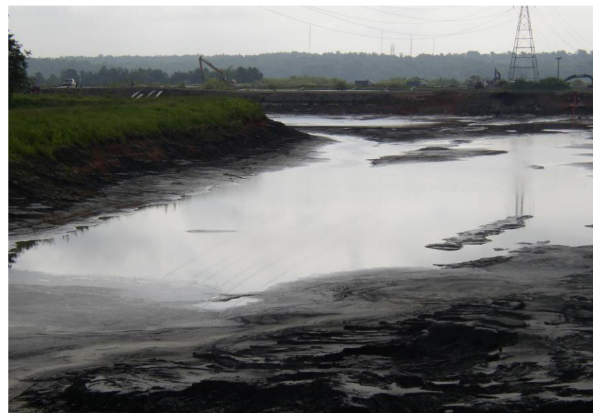
#74 Excavated Ash & Pool Elev. 635 in Cell 1
