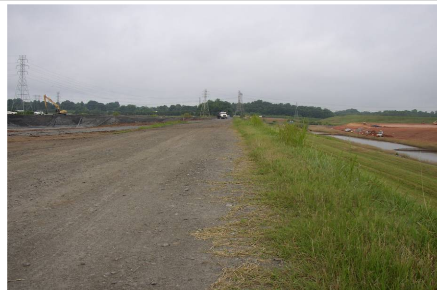
#56 Widened Upstream Crest (to 45 Feet) to Create Haul Road
