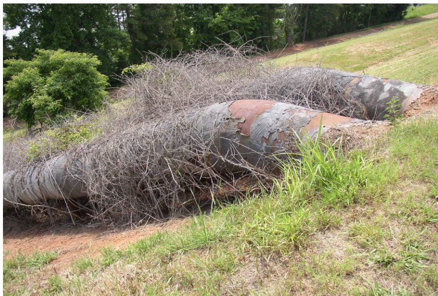
#16 Wastewater Sump Discharge Pipes @ Cell 3
