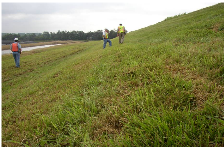
#53 Downstream Slope of North Dike (Central Area)
