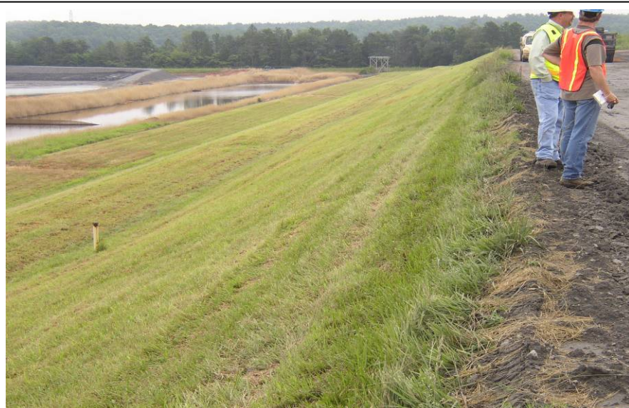
#61 Overview of Central Portion of North Dike
