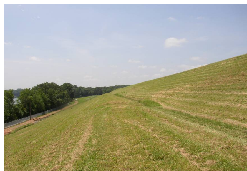
#22 Stability Berm and Downstream Slope of East Dike
