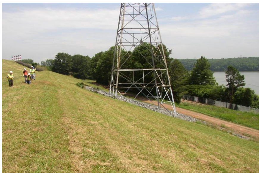
#23 Northern End of East Dike - Note Stability Berm Extends Over Transmission Tower
