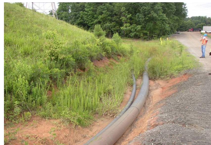
#75 Cut Into Downstream Toe of North Dike For Pipe Installation
