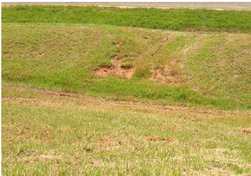
#4 Local Erosion on Top of Downstream Stability Berm – Southern Portion of East Dike
