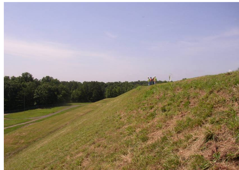
#10 Southern Downstream Slope of East Dike - Note Local Scarps in Upper Slope
