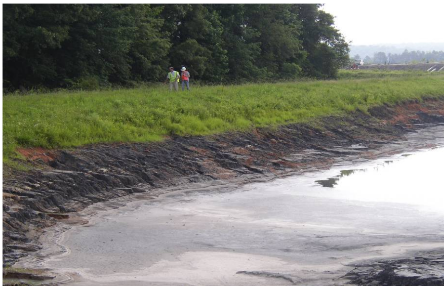
#73 Cell 1 Partially Excavated Ash on Upstream Side of Dike – Note Surface Erosion on Dike Slope
