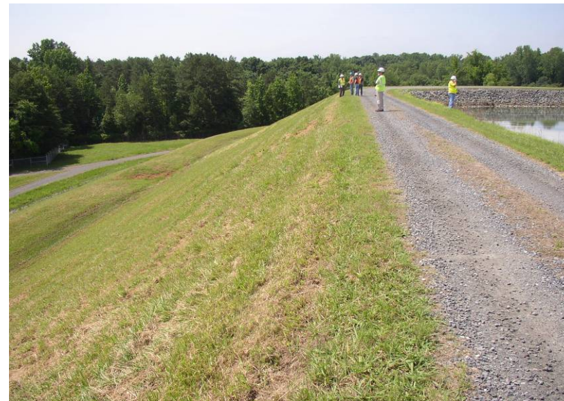
#9 Southern Portion of Crest & Downstream Slope of East Dike – Note Pooled Water on Berm
