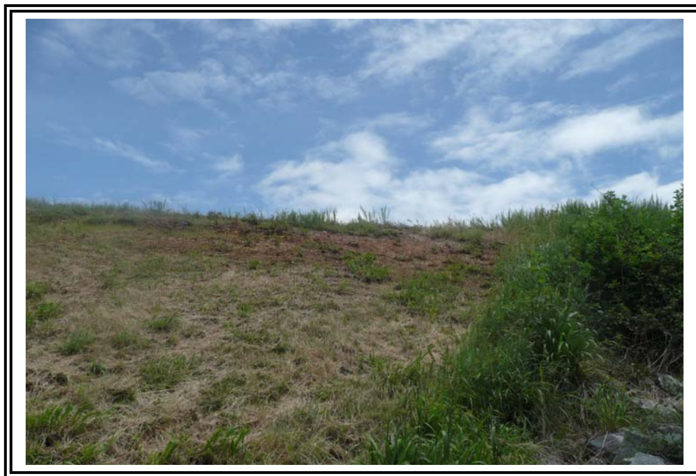
Close-up of slope at left (south) abutment with sparse vegetation.
