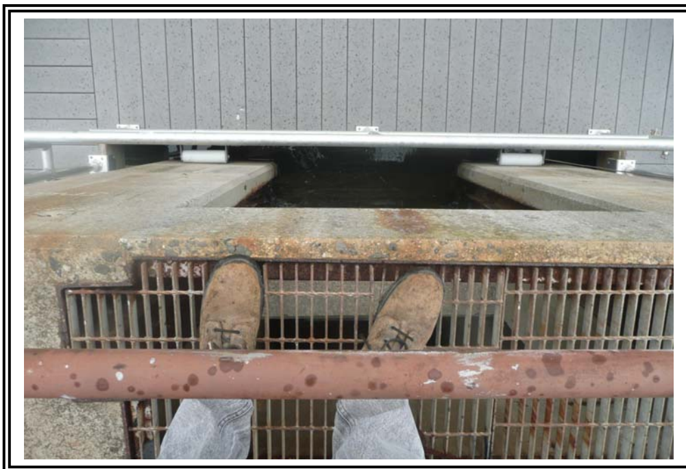
Open weir in primary cell outlet tower.
