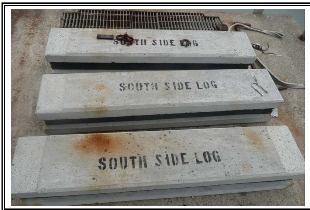
Concrete stop logs used to regulate water level in the primary pond.
