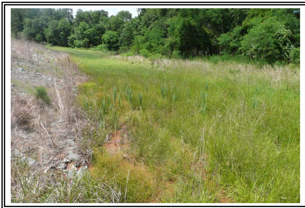
Reeds growing in area of seepage at the toe.
