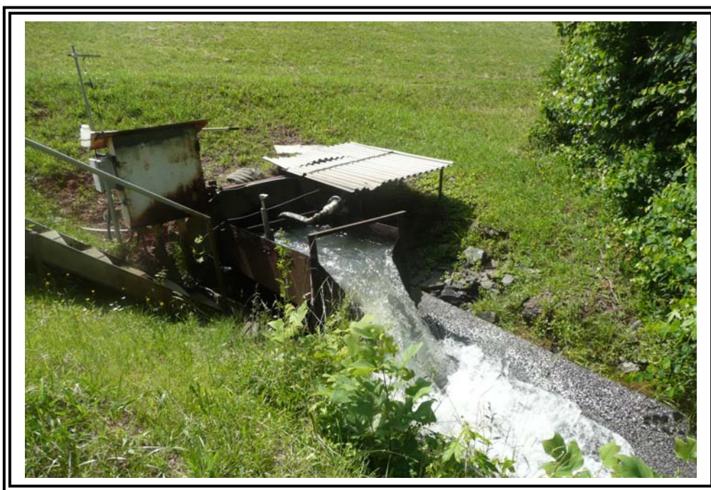
Outlet structure at toe of secondary dike, looking upstream.
