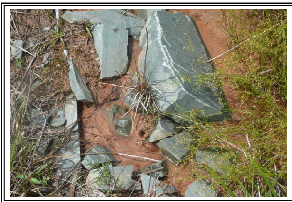
Seepage at the toe of the secondary dike about 300 feet from piezometer row. Water is clear.
