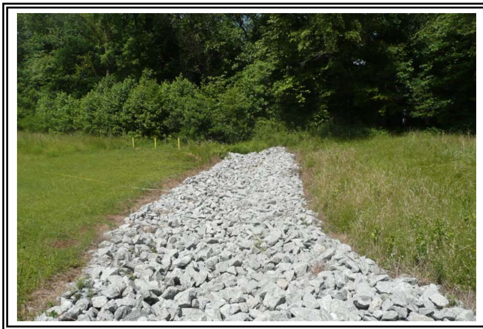
Rip rap placed in a wet area at the toe of the secondary dike. Based on field observations it appears the wet area was the result of surface drainage from the bench swale discharge and shallow groundwater levels in this area.
