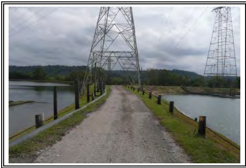
Transmission tower and Dupont unloading line on Interior Dike.
