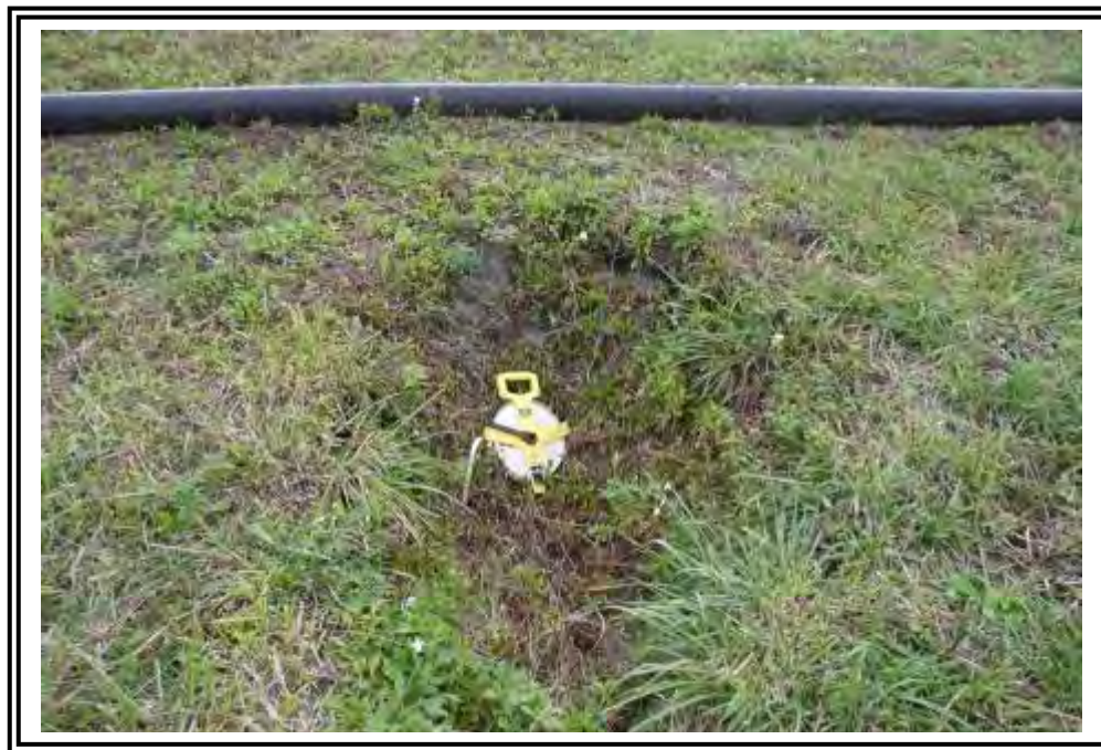
Erosion feature, Interior Dike Ash Pond B.
