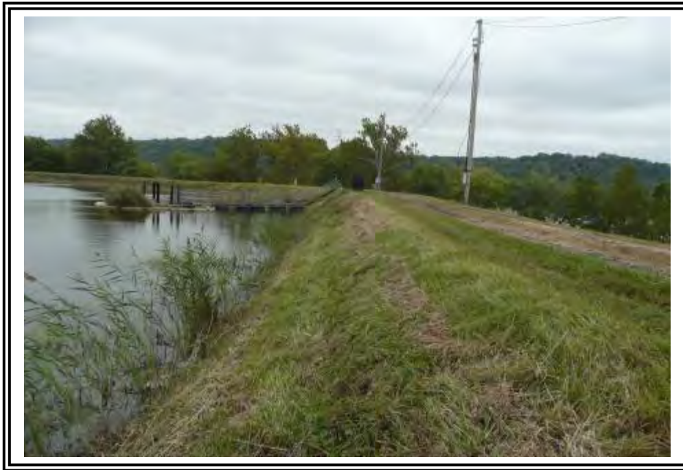
Ash Pond A crest and overflow structure, southwest corner.
