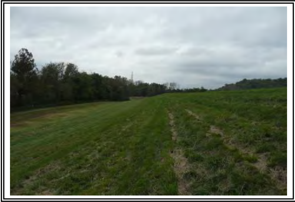
Downstream face of West Dike of Ash Pond B.
