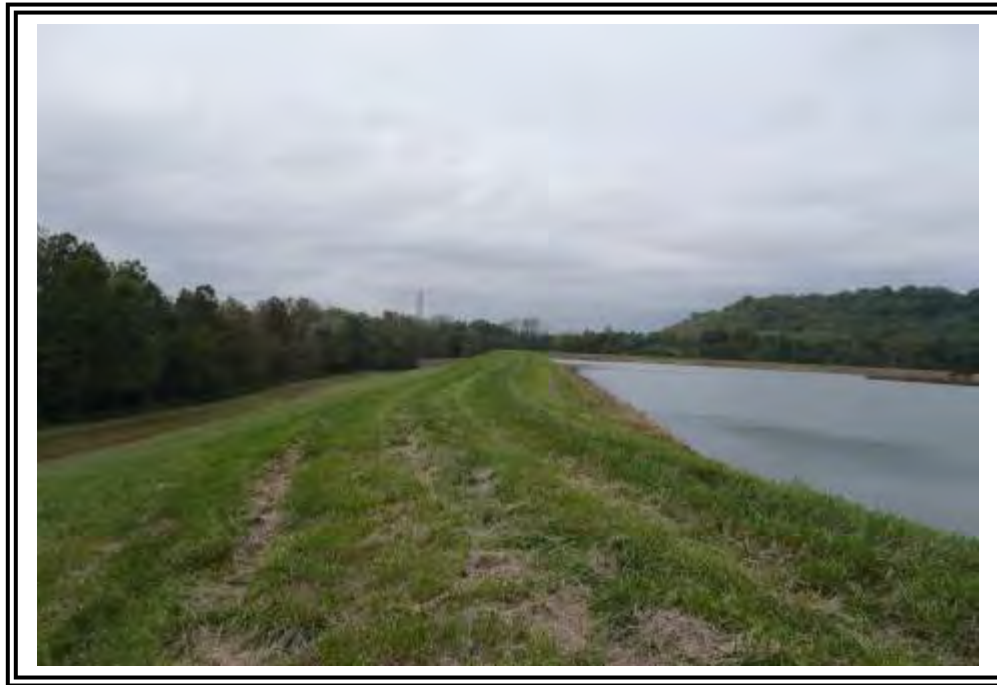
West Dike of Ash Pond B.
