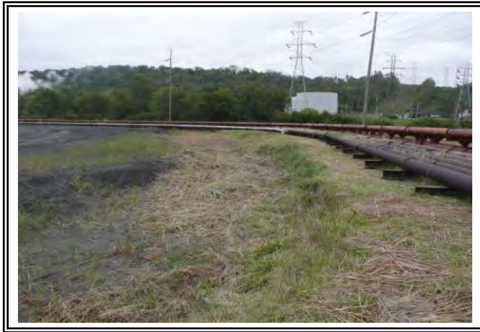
Ash Pond A northeast corner.
