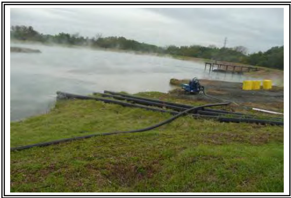
View of discharge pipes.
