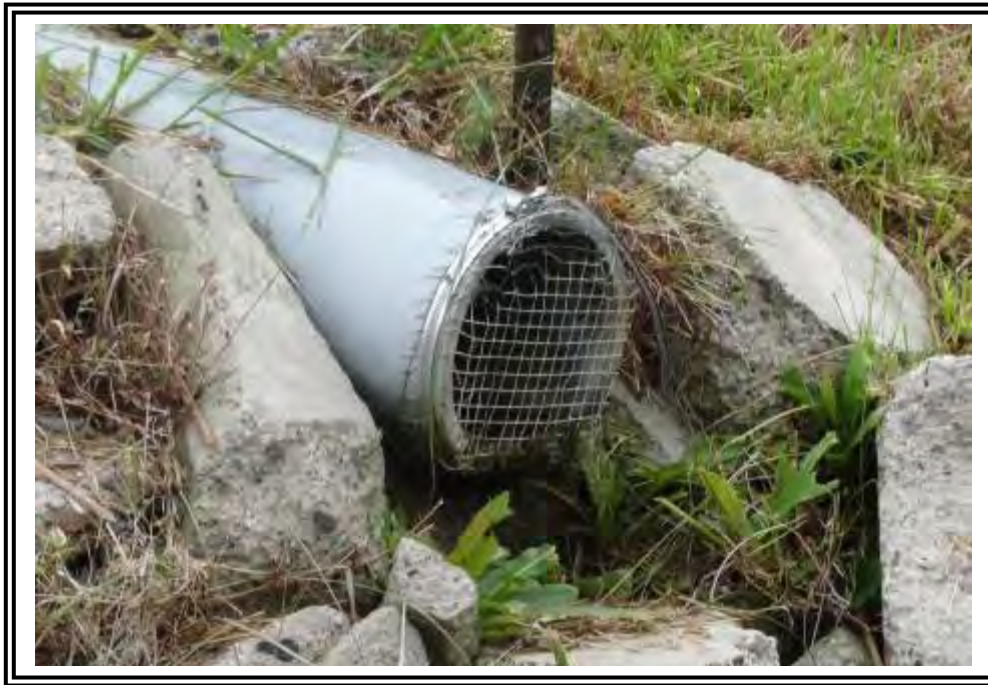
Ash Pond B typical toe drain outlet.
