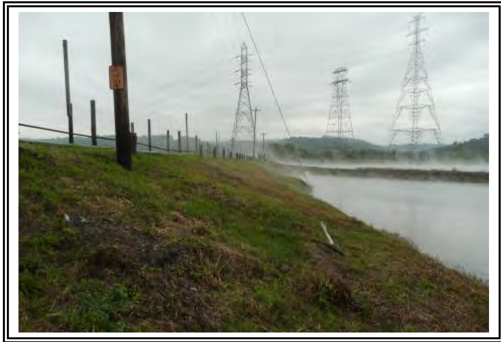
Interior Dike western side slope of Ash Pond B.
