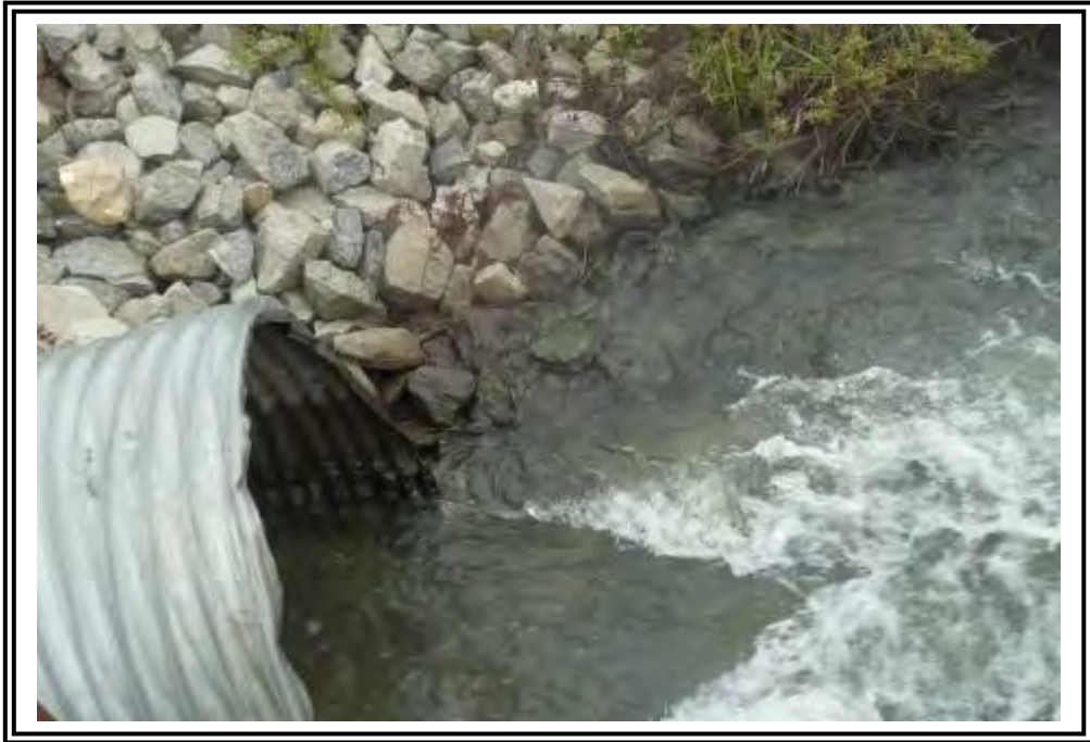
Culvert on northern side of interior groin in Ash Dike B.
