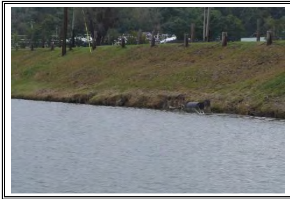
Culvert through embankment from Ash Pond A.
