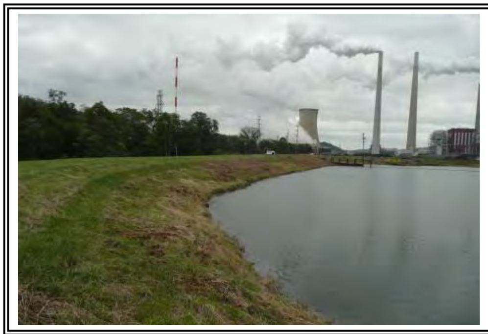
Ash Pond B, North Dike, northwest corner, looking east.
