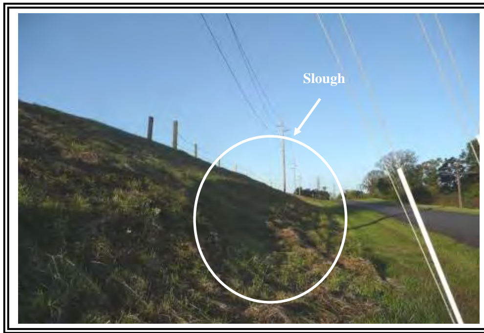
Ash Pond A slope slough, north slope.
