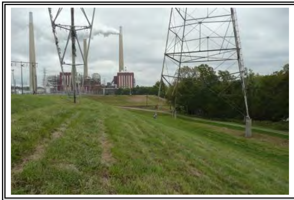
Tower foundations, looking east, South Dike Ash Pond B.
