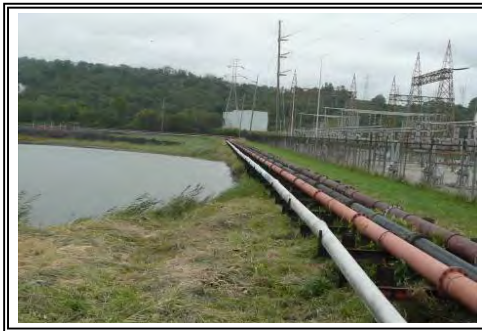
Ash Pond A East side, Ash pipes and coal pile run off pipes.
