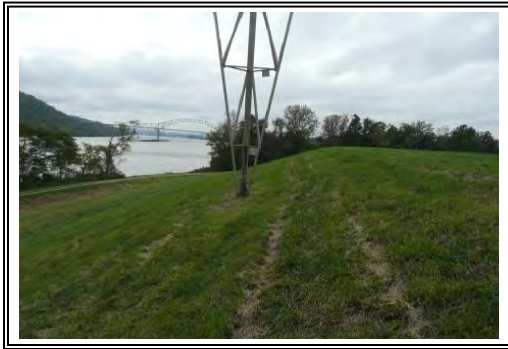
Downstream slope and transmission tower foundation.
