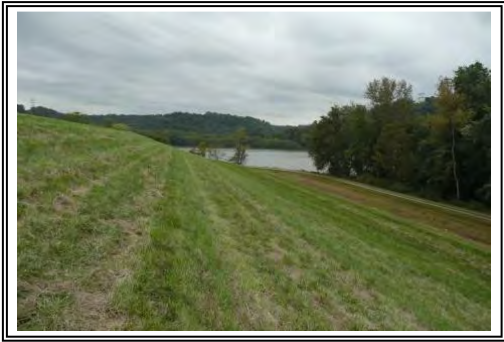
Downstream face of West Dike of Ash Pond B, looking south.
