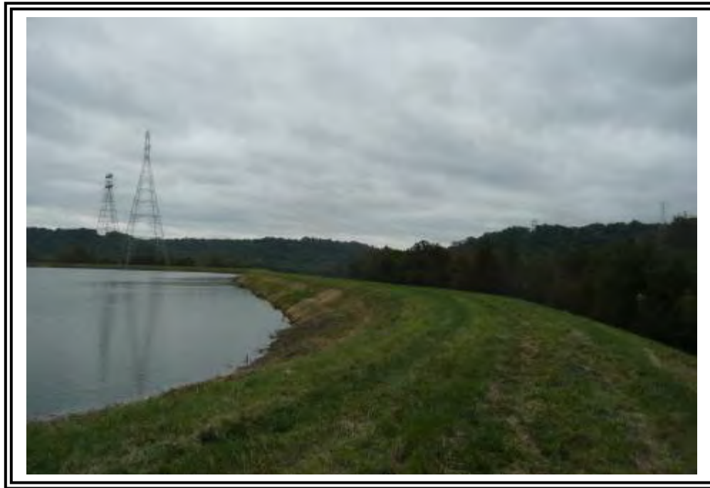
Ash Pond B, West Dike northwest corner, looking south.
