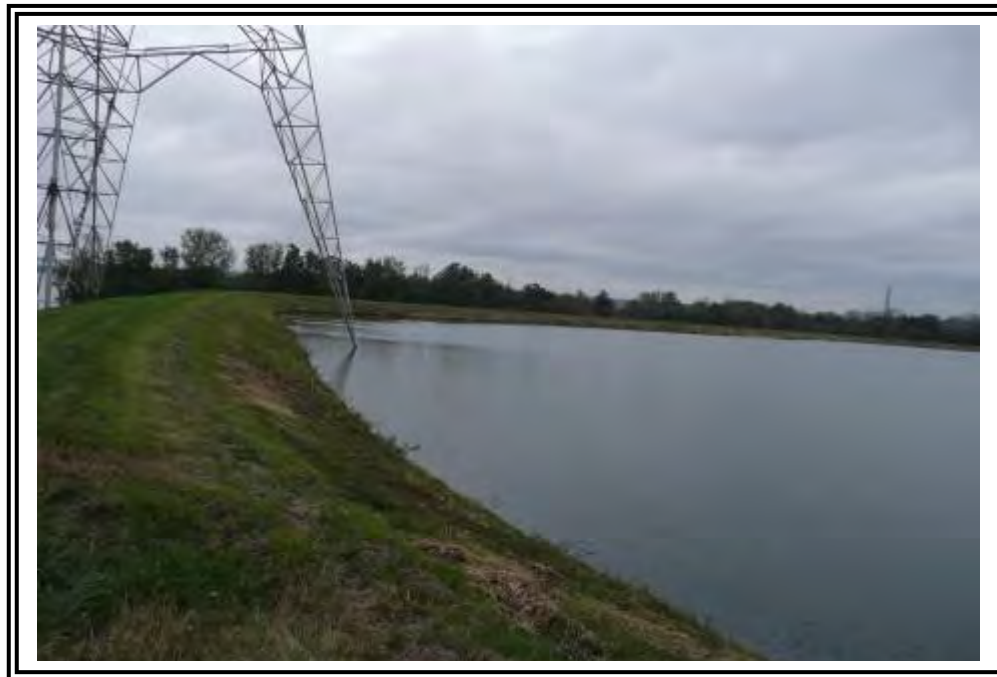
Tower foundation at crest of embankment Ash Pond B.
