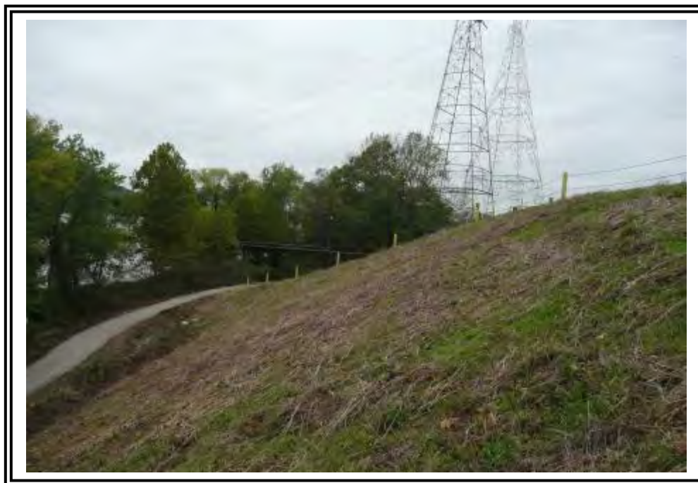
Ash Pond A, South Dike.
