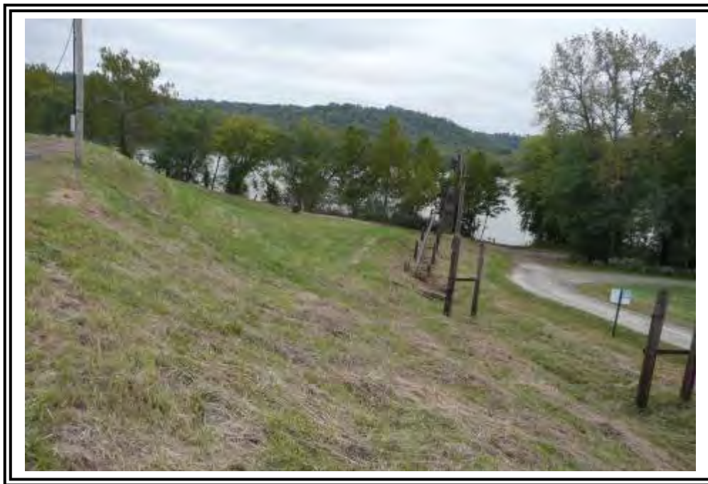
Ash Pond A, downstream face and Dupont loading rack.
