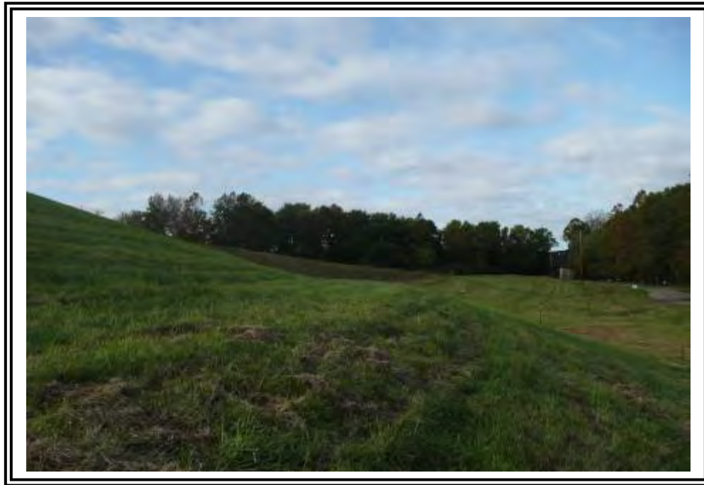
Ash Pond B northwest corner of exterior berm looking west.
