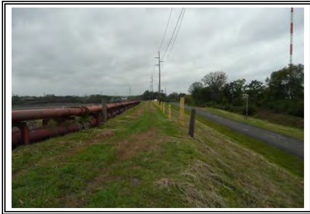
Ash Pond A North Dike, exterior slope.
