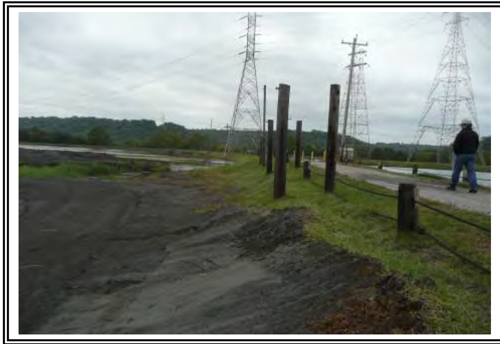
View of Ash Pond A from Interior Dike.
