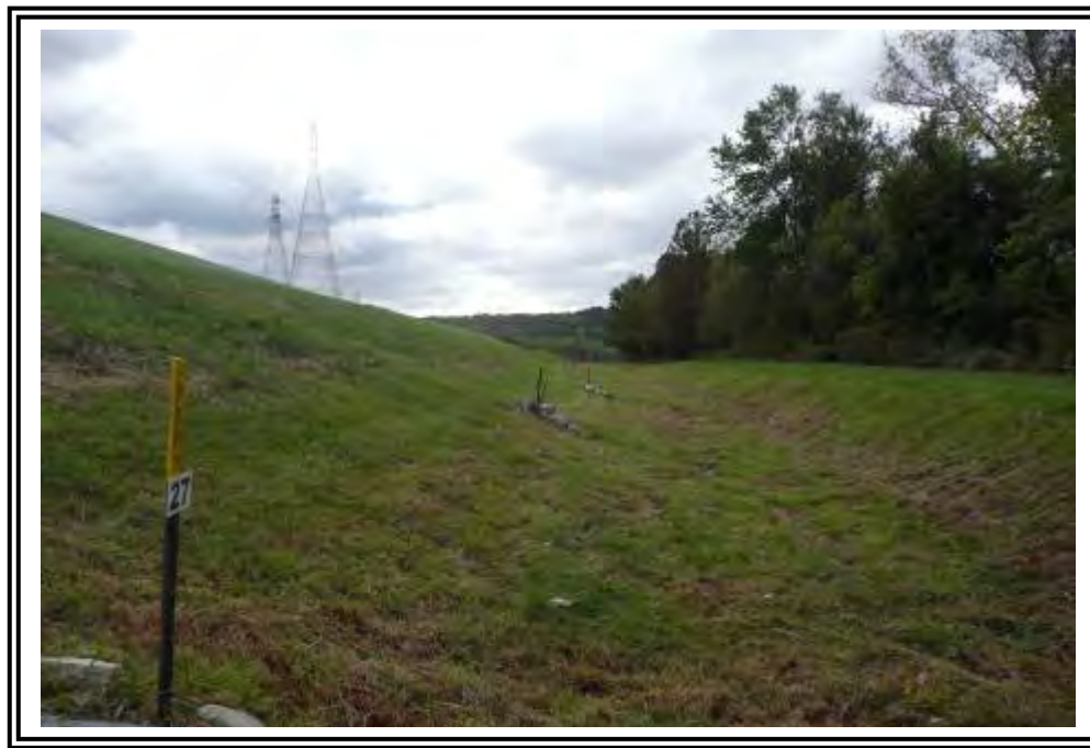
Ash Pond B toe drains, West Dike.
