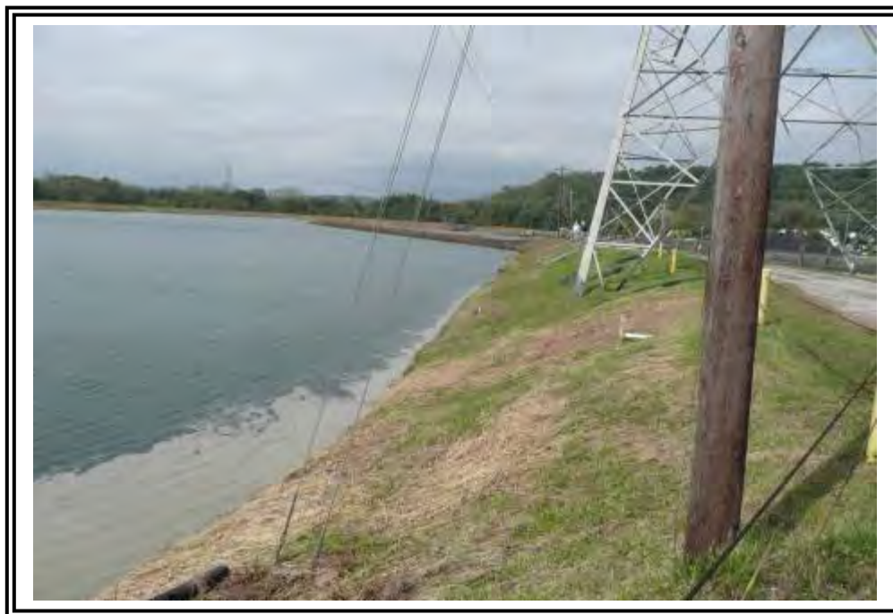
Interior Dike side slope of Ash Pond B.
