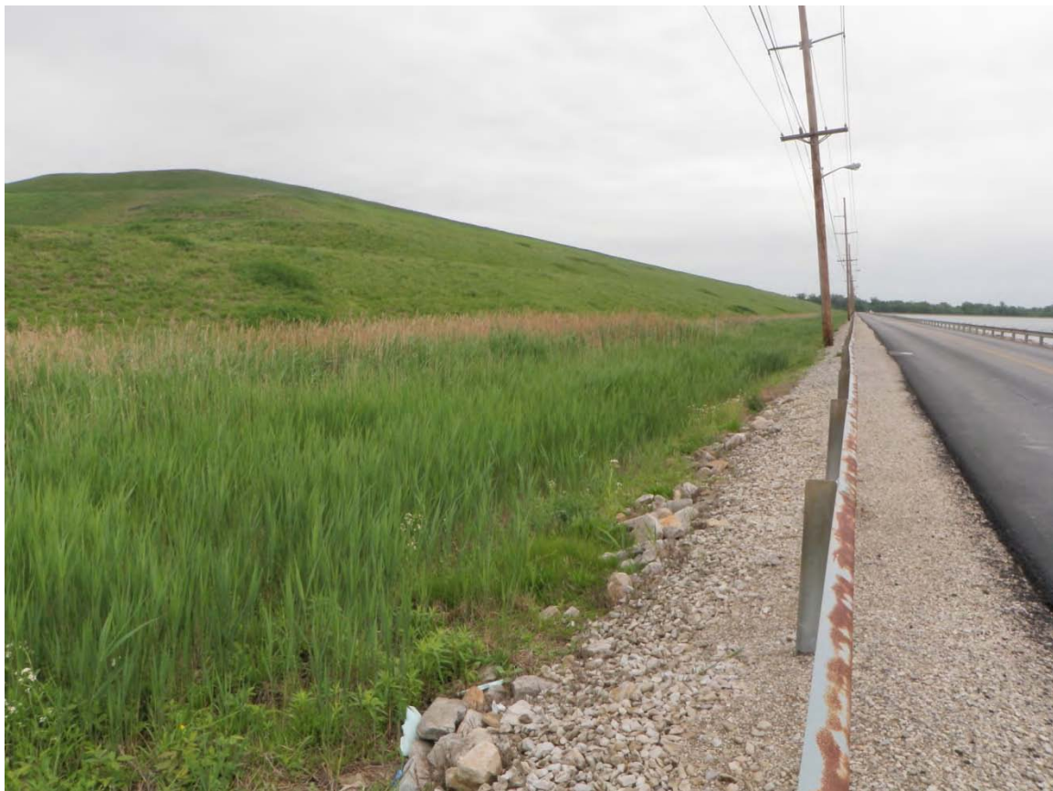
Photo 45: North Ash Pond – Southeast dike upstream slope, crest and road, looking southeast from crest.
