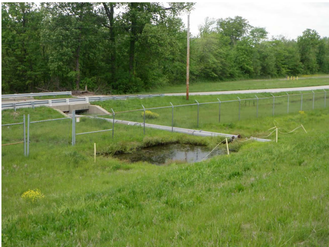
Photo 30: East Ash Pond #2 - EAP #2 downstream slope, abandoned discharge lines and drainage sump, looking northwest.
