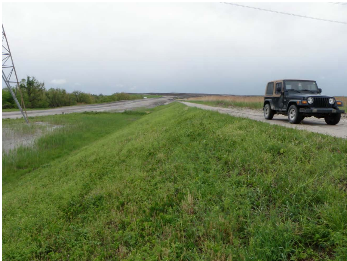
Photo 35: North Ash Pond – North dike downstream slope, looking southeast at northeast dike.
