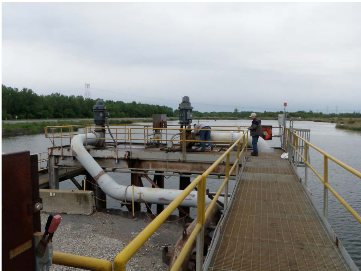
Photo 41: North Settling Basin – Pump intake structure that discharges to cooling pond, looking northeast.
