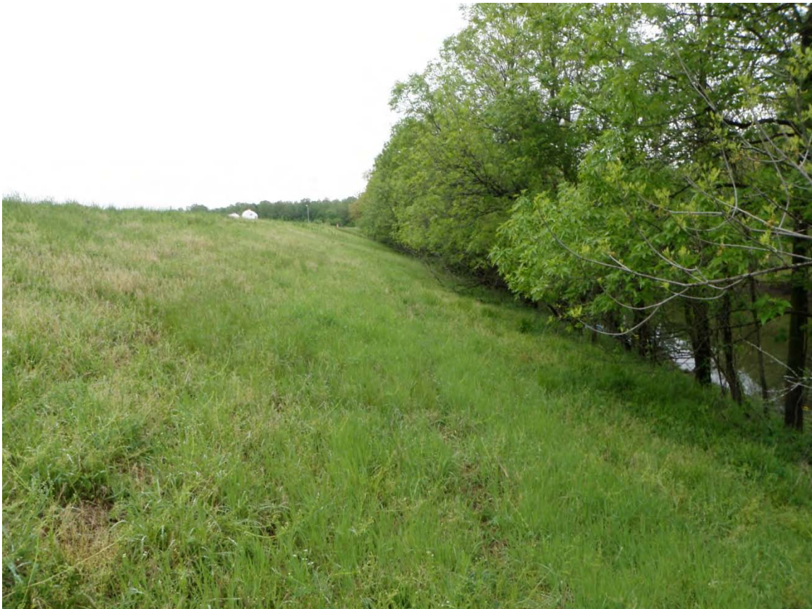
Photo 38: North Ash Pond – North dike downstream slope, looking west, notice large trees in wetland at toe of slope.
