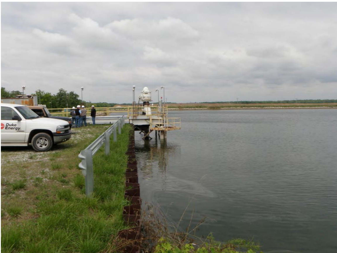
Photo 2: East Settling Basin - Pump intake that discharges to the Cooling Pond, looking north.
