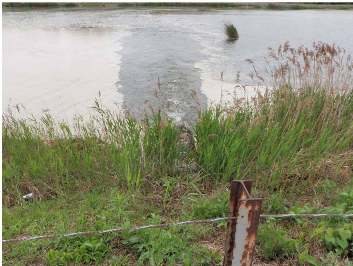
Photo 43: North Settling Basin – Discharge into settling basin, looking northwest from interior dike between NAP and NSB.
