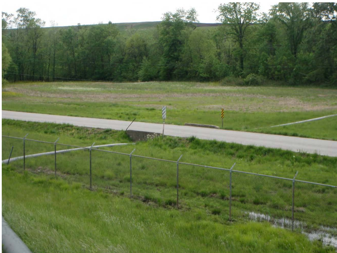
Photo 26: East Ash Pond #2 – CCW discharge line crossing under county road, looking southwest from west dike.
