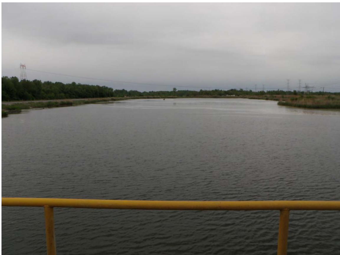
Photo 42: North Settling Basin – Reservoir area looking northeast from pump intake structure.
