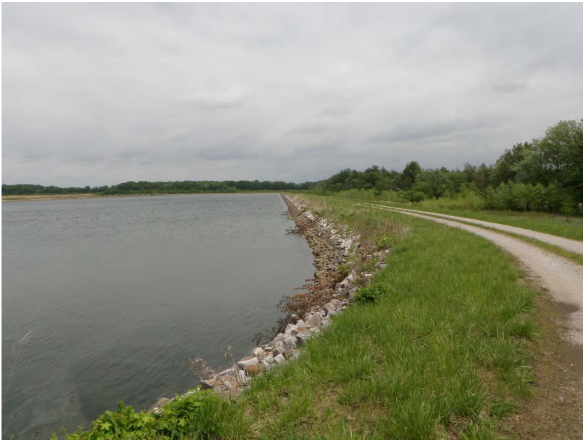
Photo 1: East Settling Basin - South dike upstream slope, looking east from south west corner.
