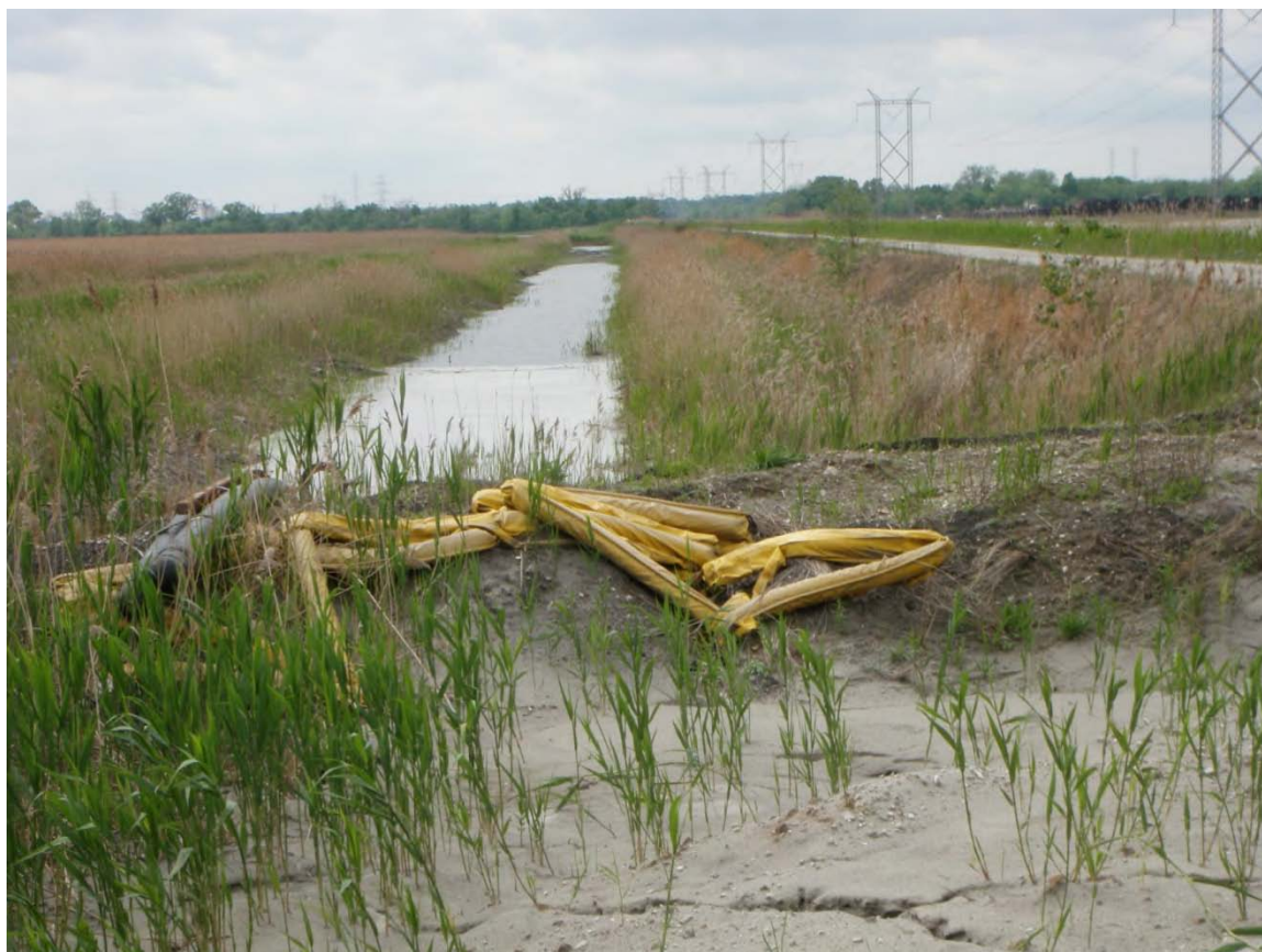
Photo 15: East Ash Pond #1 – Drainage swell on north side of EAP #1 that discharges to EAP #2, looking west.
