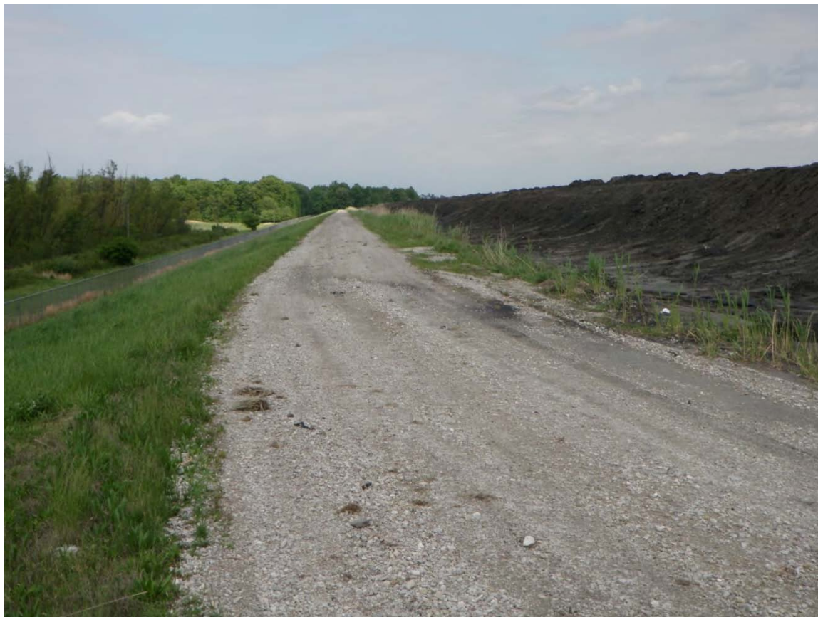
Photo 23: East Ash Pond #3 – North dike crest and capping material, looking east from northwest corner of EAP #3.
