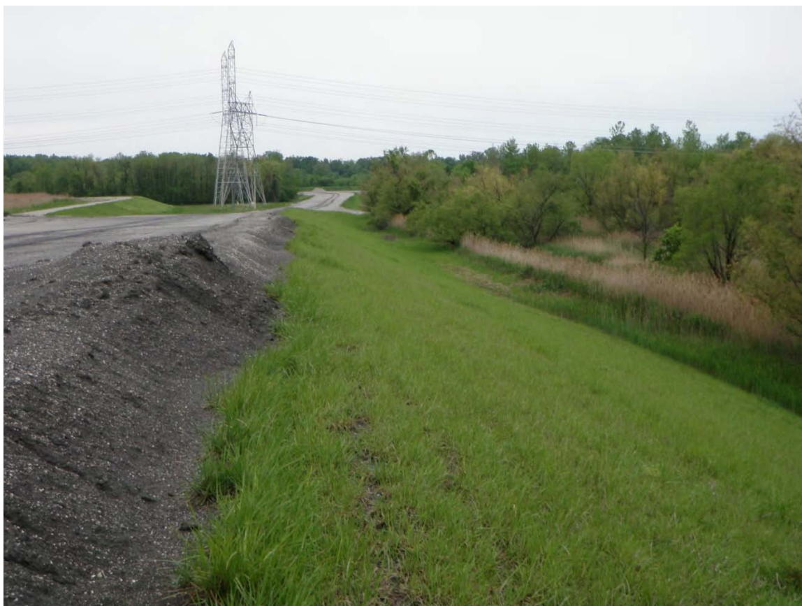
Photo 33: North Ash Pond – Downstream slope and crest of northeast dike, looking northwest.
