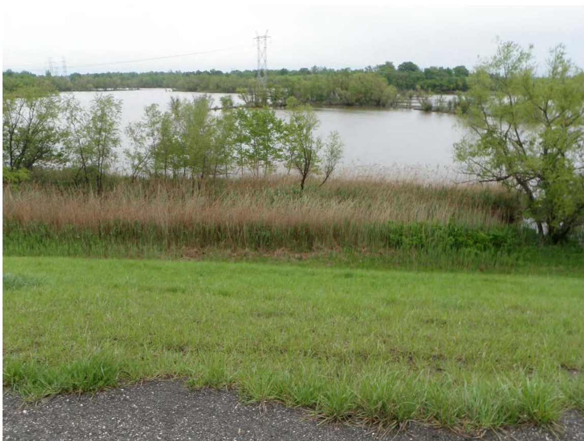
Photo 34: North Ash Pond – Downstream slope of northeast dike looking northeast at wetlands area from crest.
