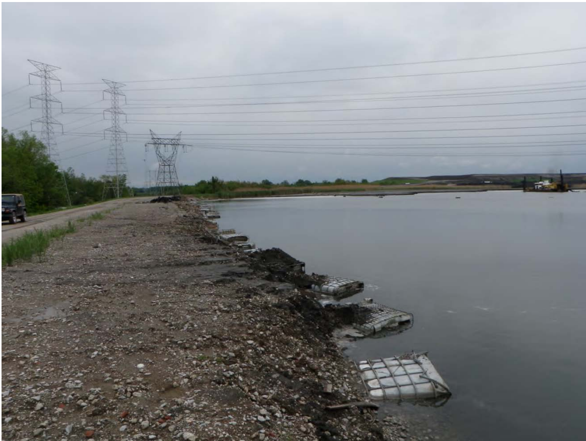
Photo 37: North Ash Pond – North Ash Pond reservoir area, looking east, notice upstream slope extended into reservoir.
