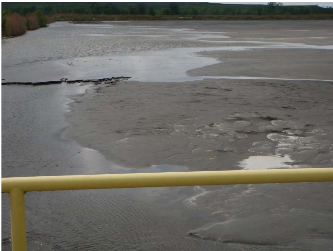
Photo 11: East Ash Pond #1 – EAP #1 reservoir area, approximately 95% full of CCW, looking west.
