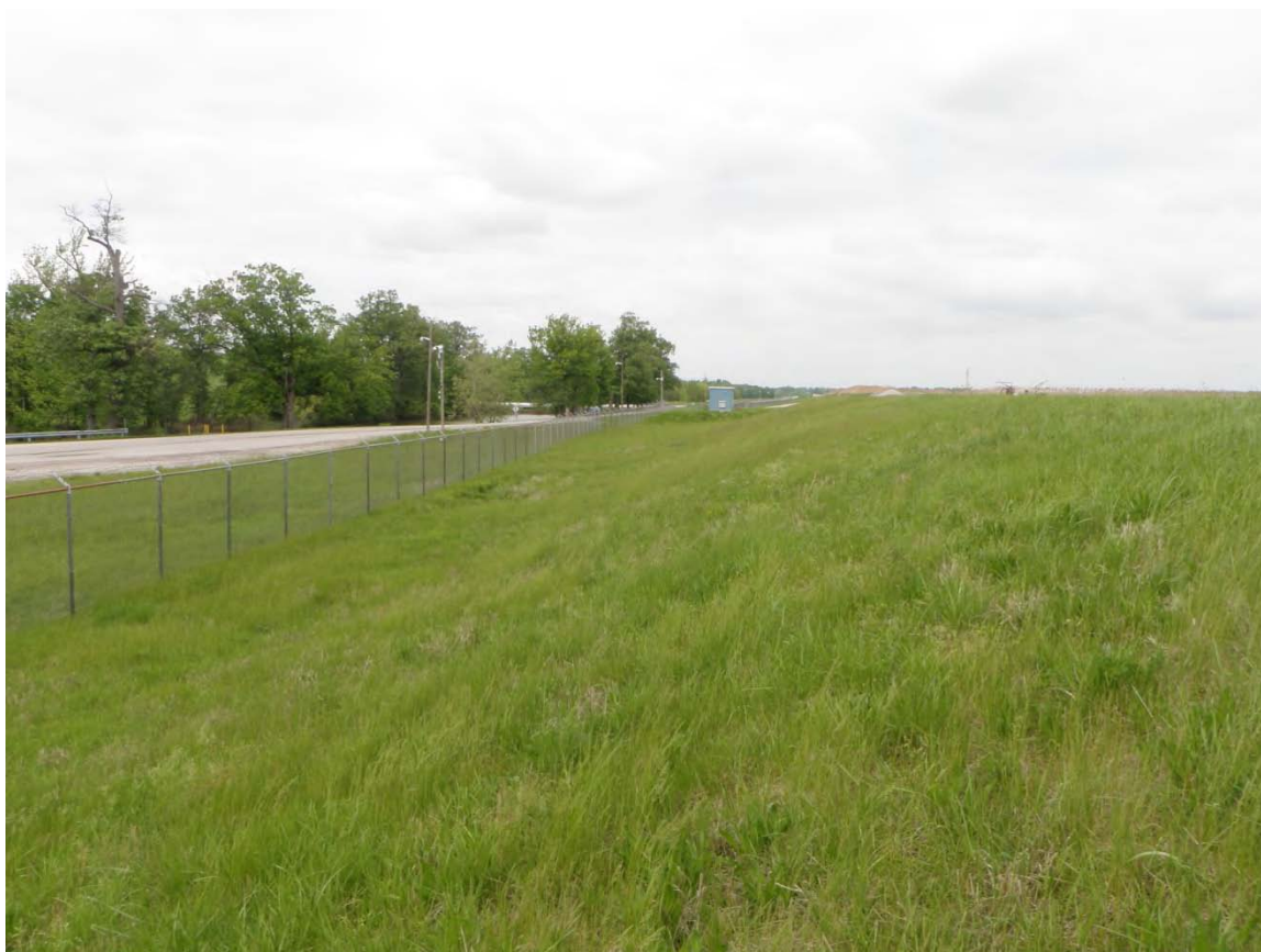
Photo 4: East Settling Basin – West dike downstream slope, looking north.
