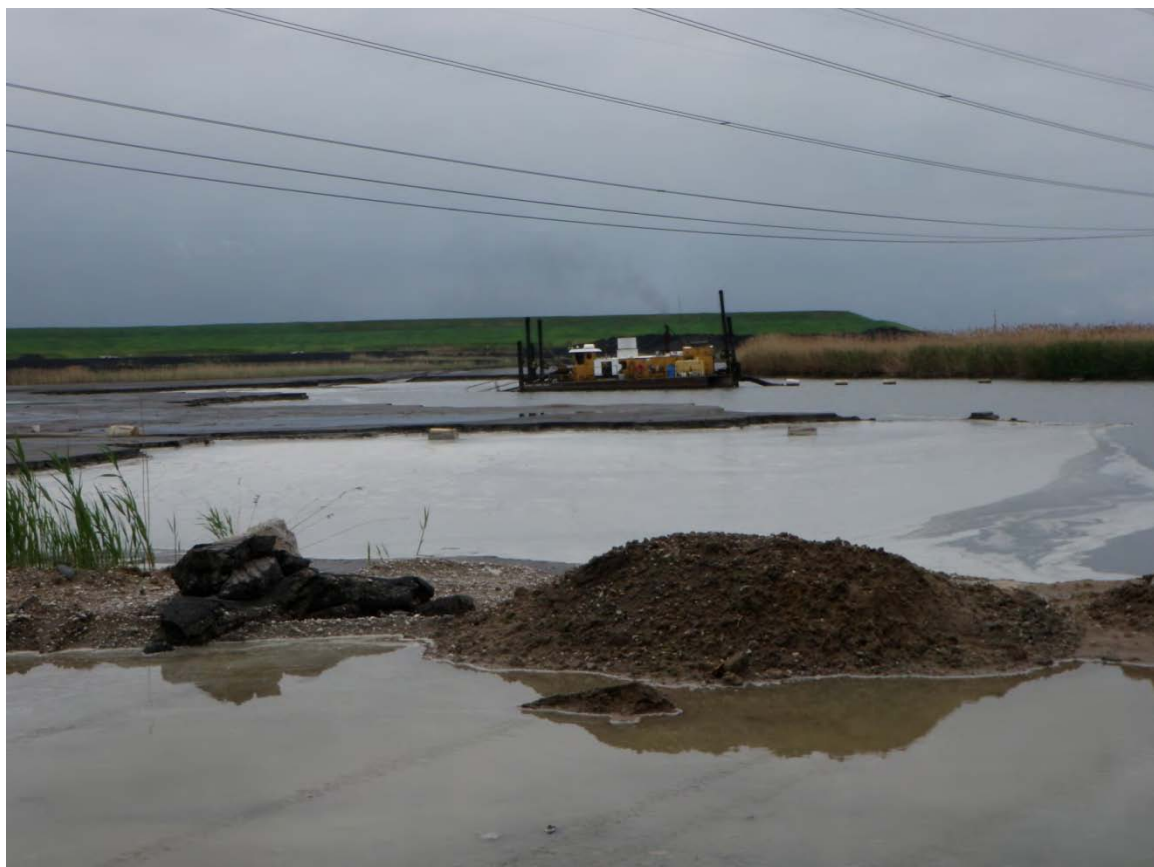
Photo 36: North Ash Pond – North Ash Pond reservoir area and dredging equipment, looking southeast from north dike.
