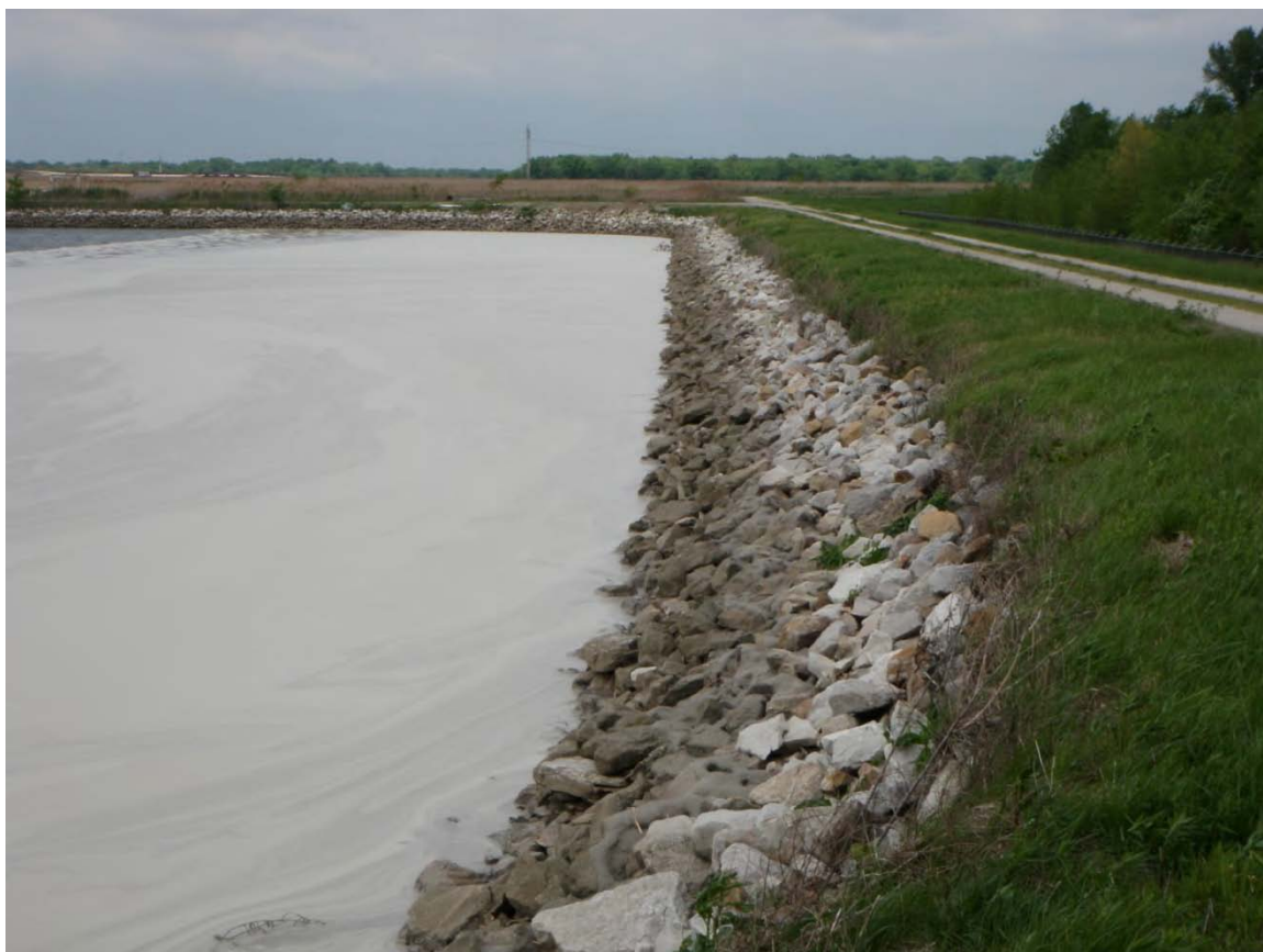
Photo 8: East Settling Basin – East Dike upstream slope, looking north.
