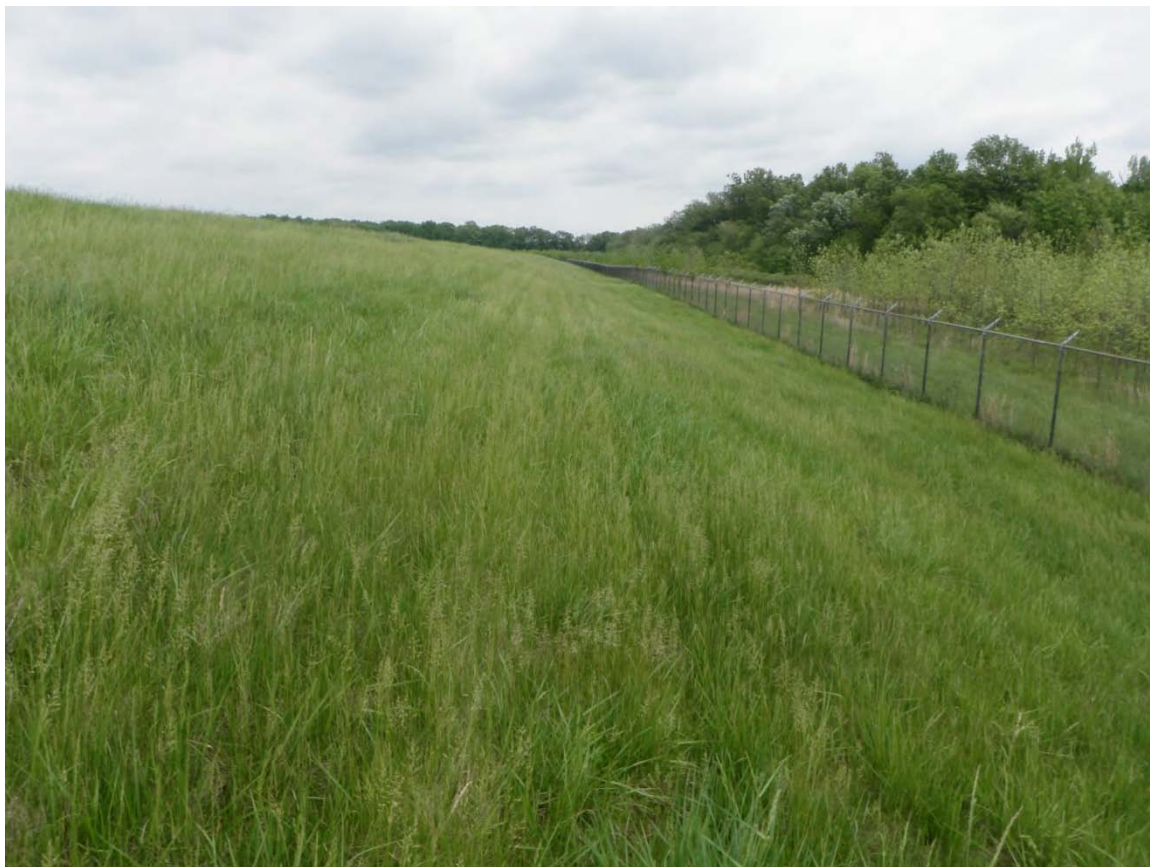
Photo 7: East Settling Basin – South Dike downstream slope, looking west.
