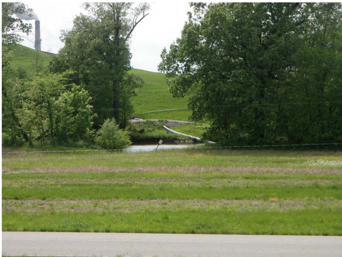
Photo 25: East Ash Pond #2 – CCW discharge line crossing Coon Creek, downstream of west dike, looking west.
