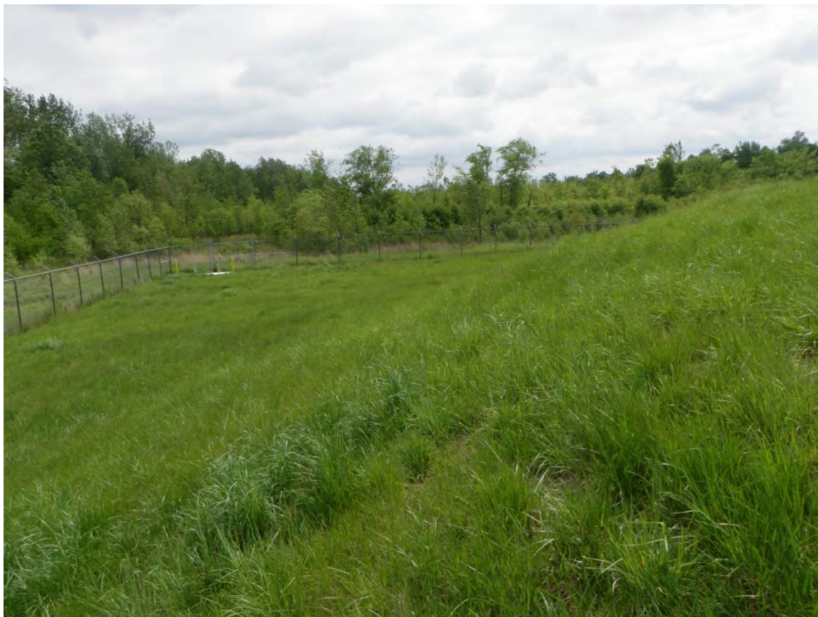
Photo 9: East Settling Basin – East and south dike downstream corner, looking south.
