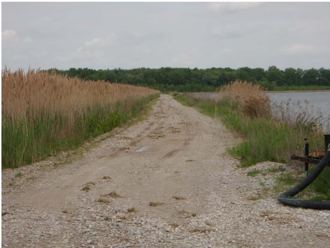
Photo 29: East Settling Basin – Interior dike crest between East Settling Basin and EAP #2, looking east.
