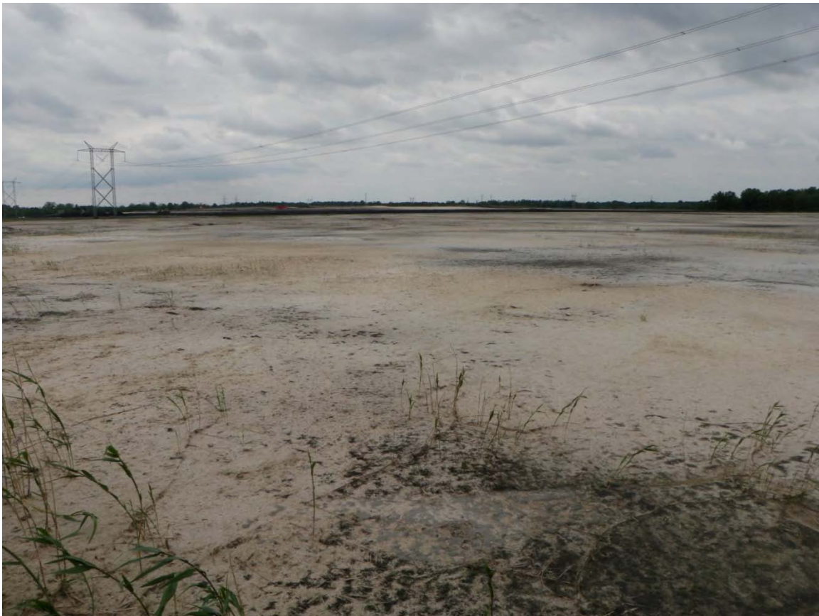
Photo 17: East Ash Pond #3 – EAP #3 reservoir area, about 95% full, in close out phase, looking northwest.
