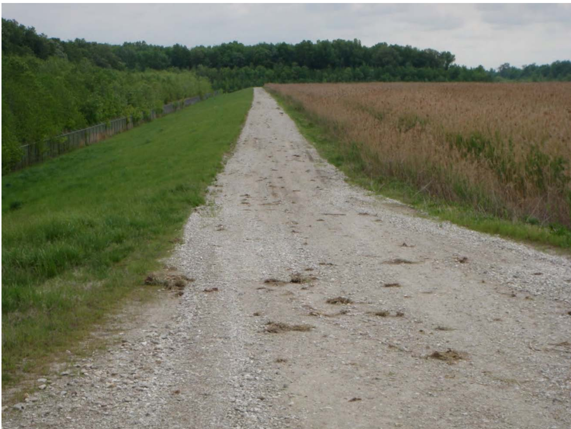
Photo 14: East Ash Pond #1 – East Dike crest and road, looking south from NE corner.
