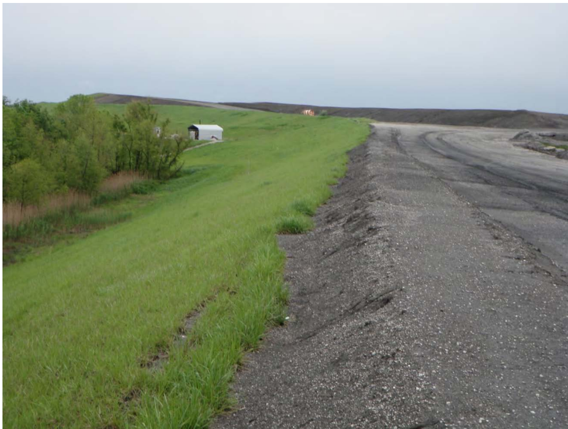
Photo 31: North Ash Pond – Downstream slope and crest of northeast dike, looking southeast.
