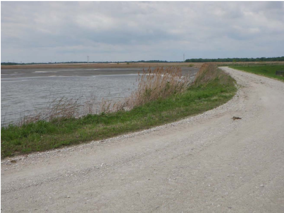
Photo 13: East Ash Pond #1 – East Dike crest, road, and reservoir area, looking north from SE corner.
