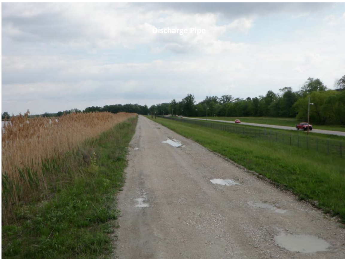
Photo 28: East Ash Pond #2 – EAP #2 west dike crest, looking south.
