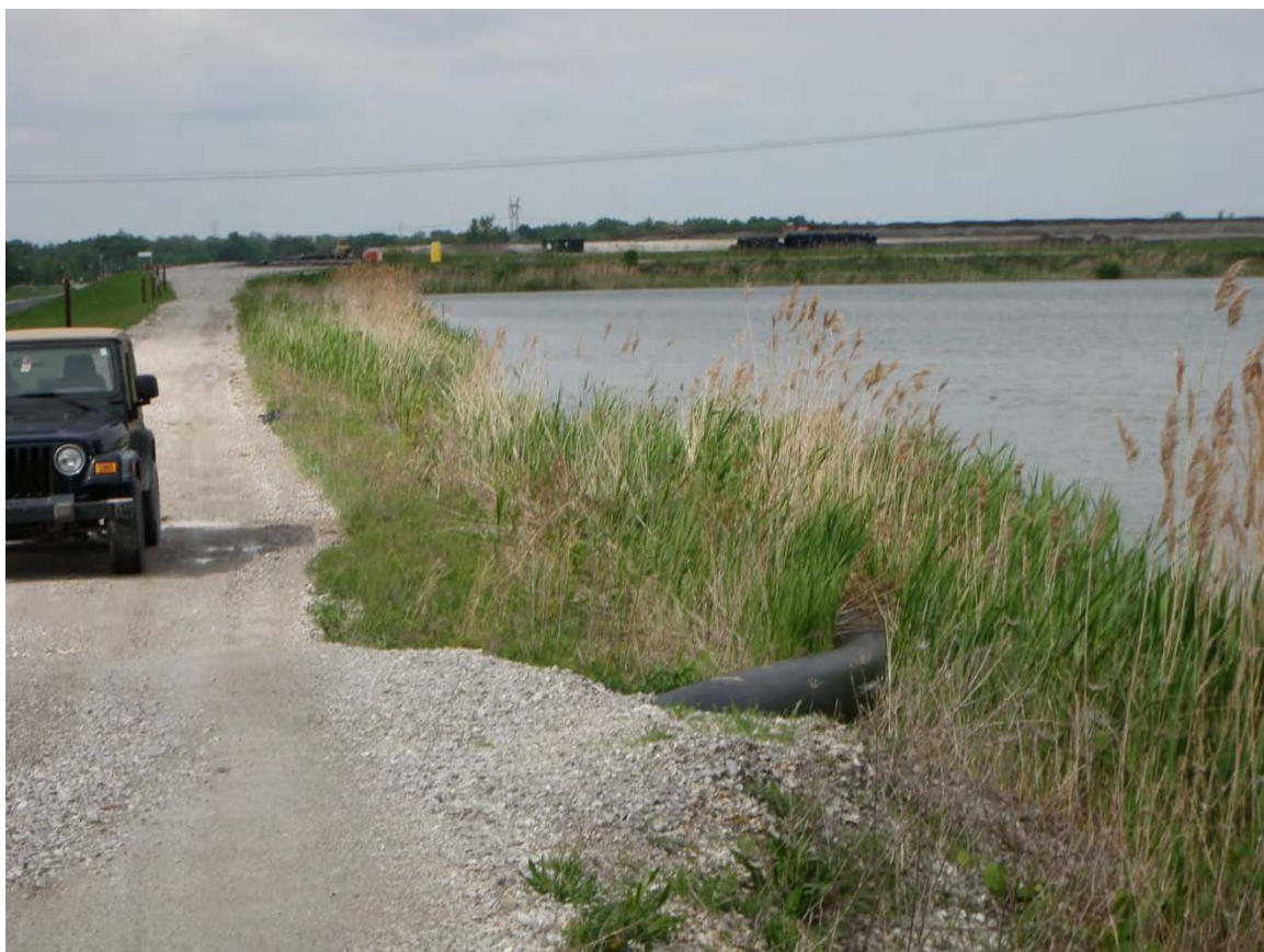
Photo 27: East Ash Pond #2 – CCW discharge line crossing west dike dam crest, looking north.
