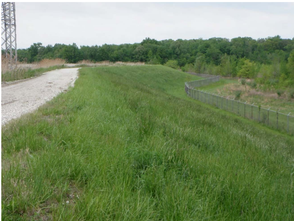
Photo 20: East Ash Pond #3 – East dike downstream slope, looking north from the corner of EAP #1 and EAP #3 interior dike.
