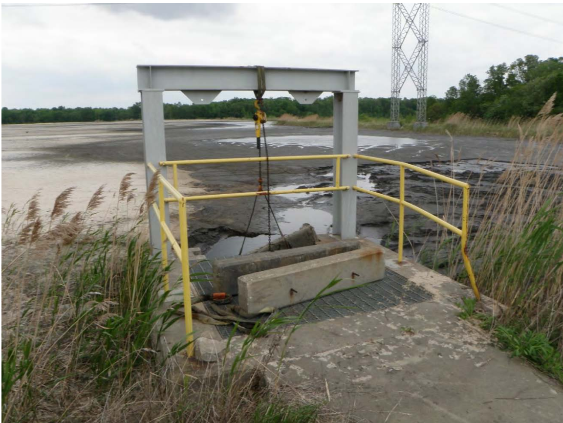
Photo 18: East Ash Pond #3 – EAP #3 Intake structure, looking north from interior dike between EAP #1 and EAP #3.
