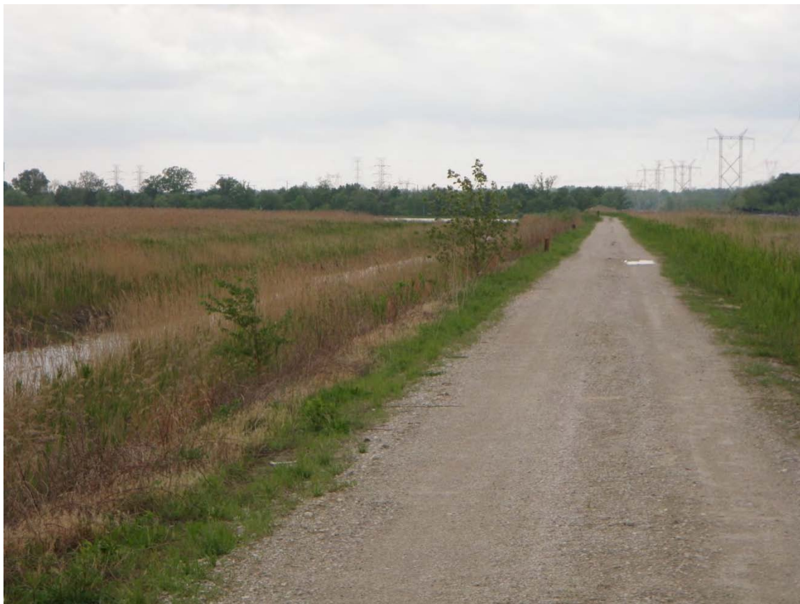
Photo 19: East Ash Pond #3 – Interior dike between EAP #1 and EAP #3, looking west, notice trees along dike.
