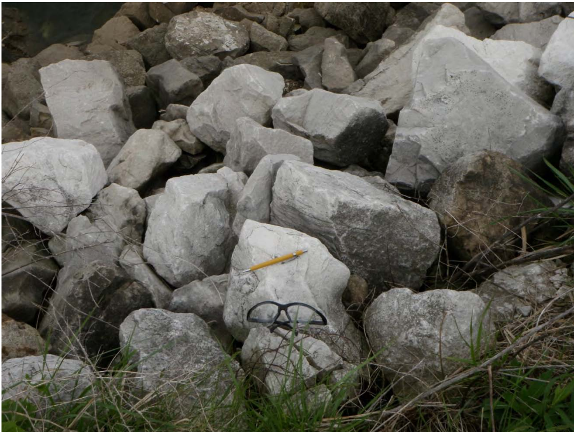
Photo 5: East Settling Basin – South dike upstream slope protection detail.
