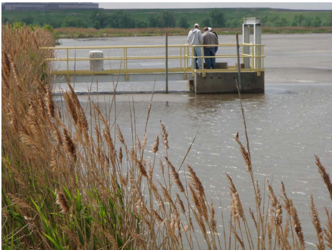
Photo 10: East Ash Pond #1 – Intake structure near southeast corner of EAP #1 that discharges to Settling Basin, looking west.
