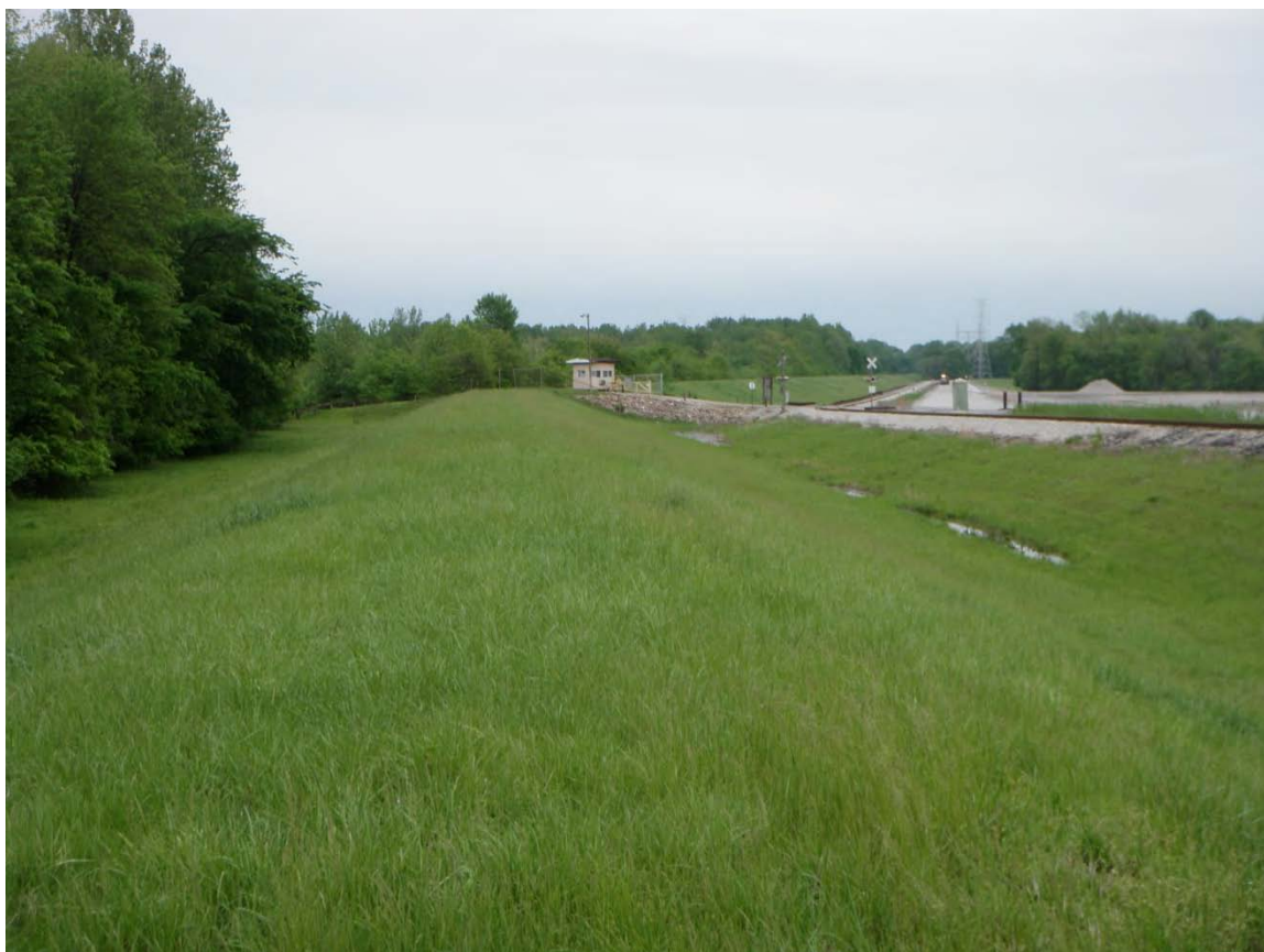
Photo 40: North Settling Basin – USACE Levee, looking northeast from levee crest.
