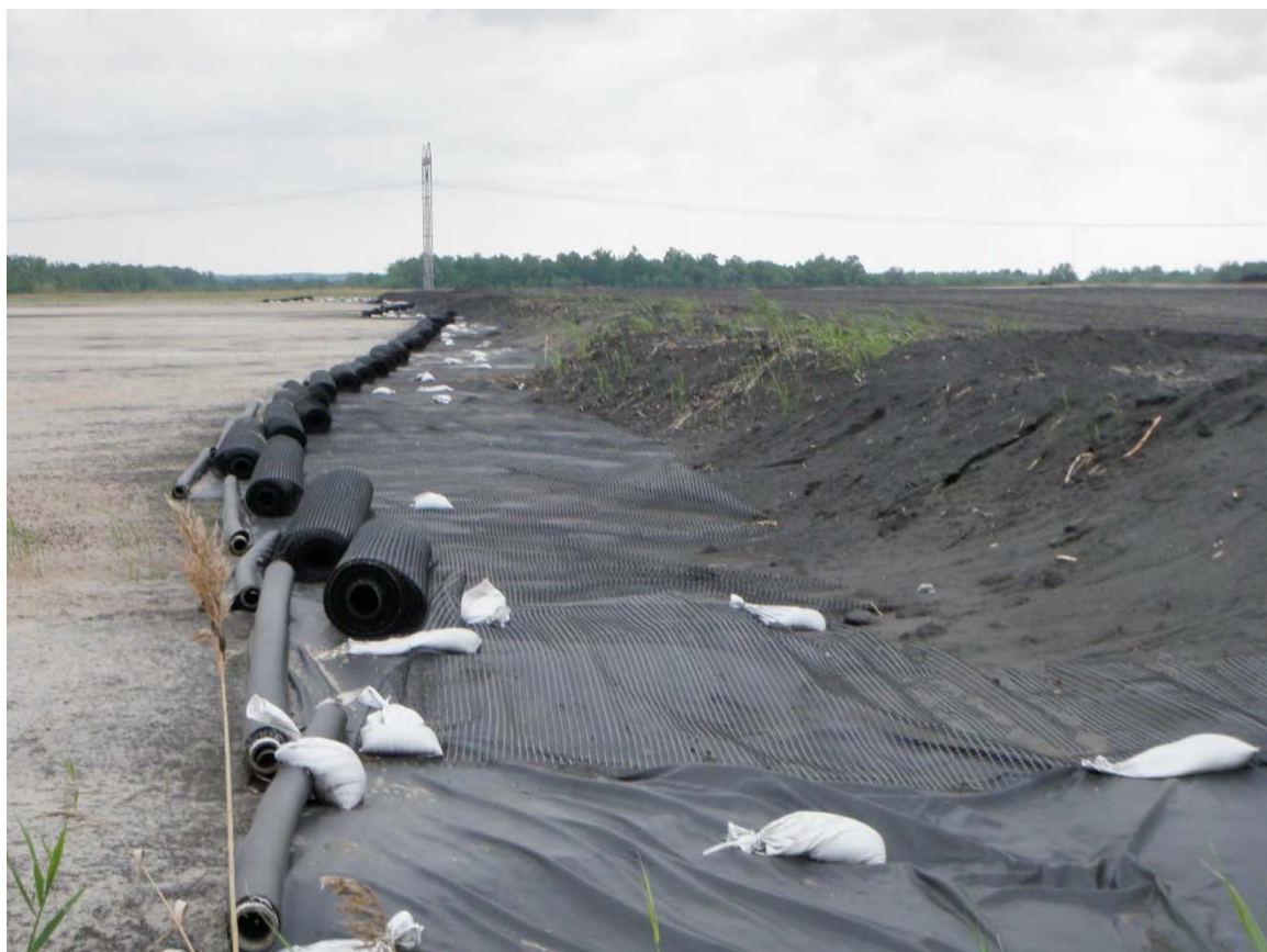
Photo 22: East Ash Pond #3 – EAP #3 capping construction, notice geofabric and geogrid, looking south from north dike.
