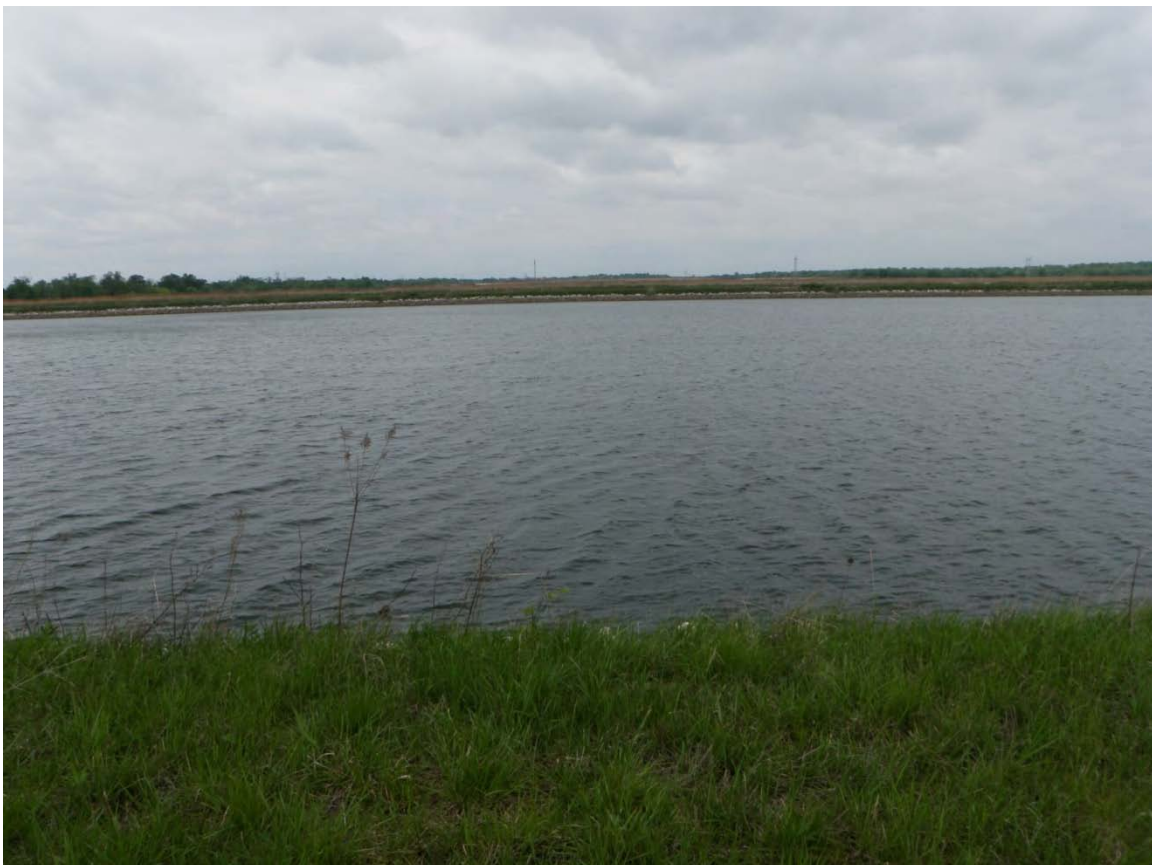
Photo 6: East Settling Basin – Reservoir area from south dike, looking north.
