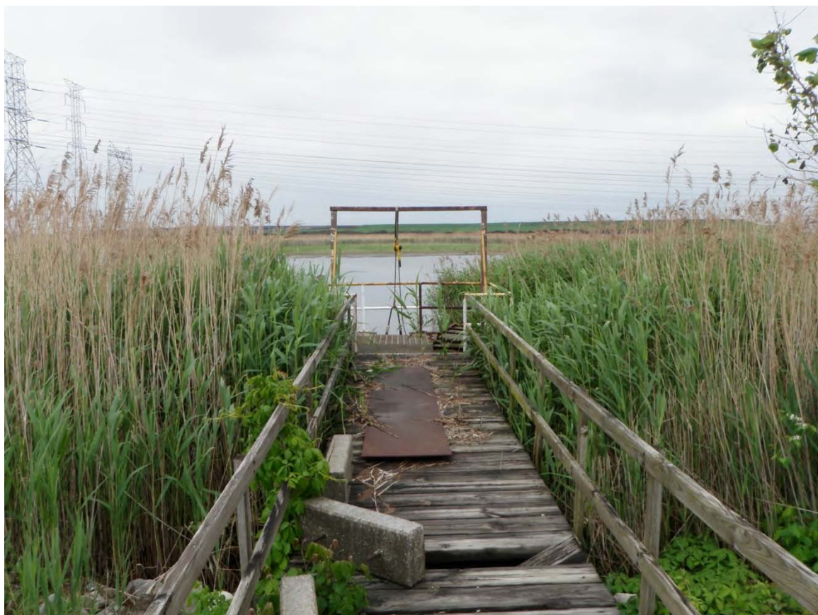
Photo 44: North Ash Pond – Intake structure in NAP that discharges into NSB, looking southeast from interior dike.
