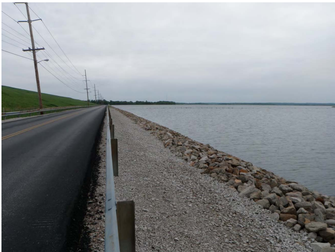
Photo 46: North Ash Pond – Southeast dike downstream, crest and cooling pond reservoir area, looking southeast.
