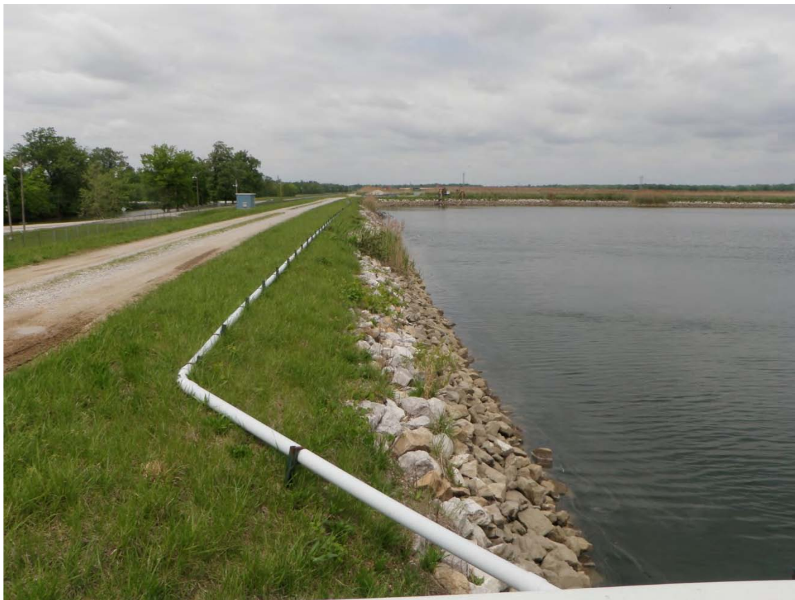
Photo 3: East Settling Basin – West dike upstream slope, looking north.
