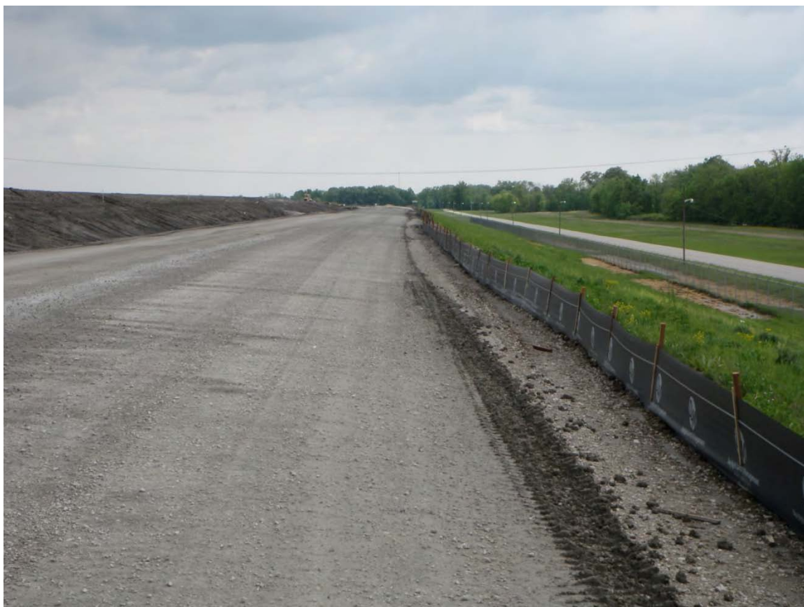
Photo 24: East Ash Pond #3 – West dike crest and road, looking south, notice county road to the west.\
