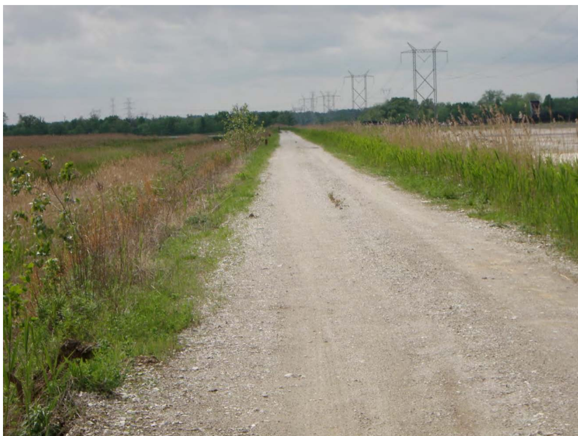
Photo 16: East Ash Pond #3 – Interior dike crest and road between EAP #1 and EAP #3, looking west.
