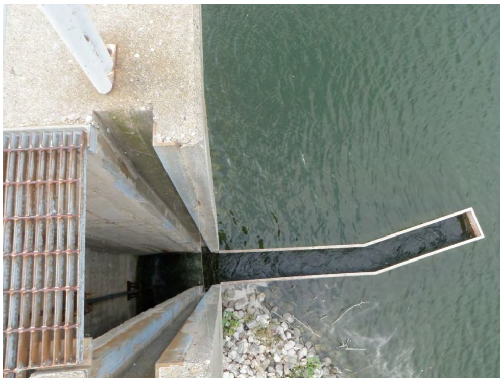
Photo 25: Primary Ash Settling Pond – Intake structure, concrete weir #2
