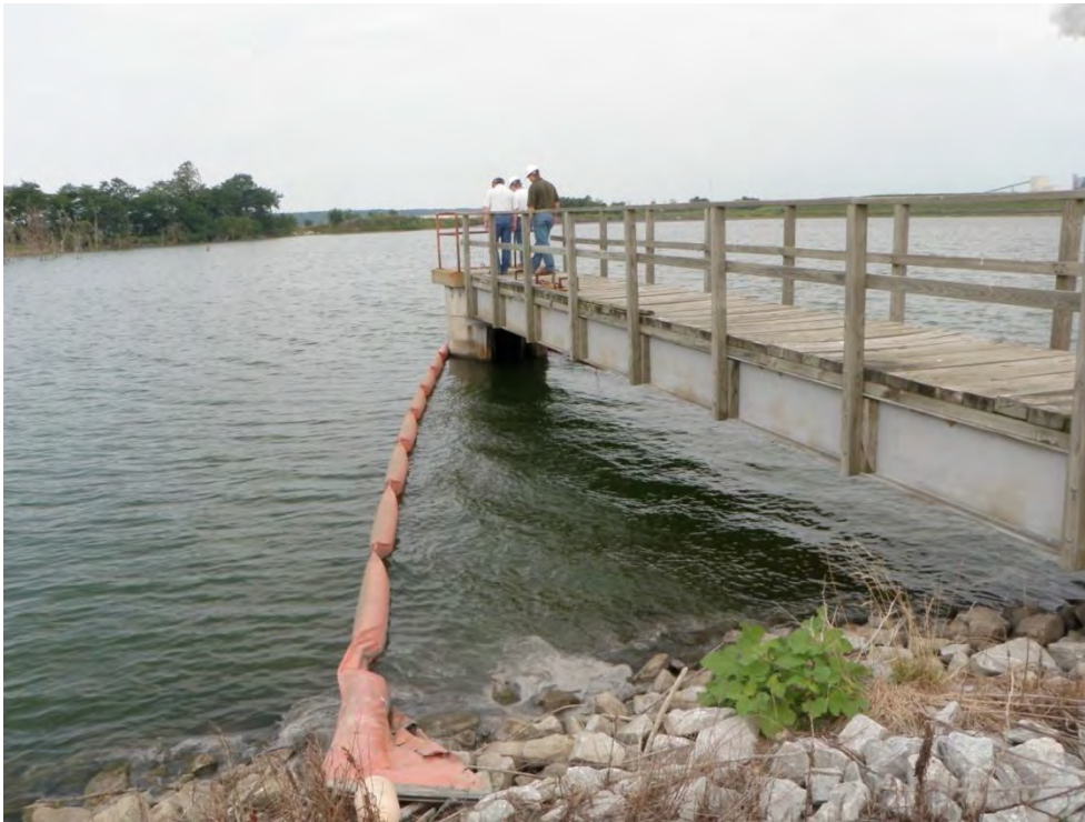
Photo 19: Ash Disposal Area #1 – Intake structure, weir #5, east dike, looking west
