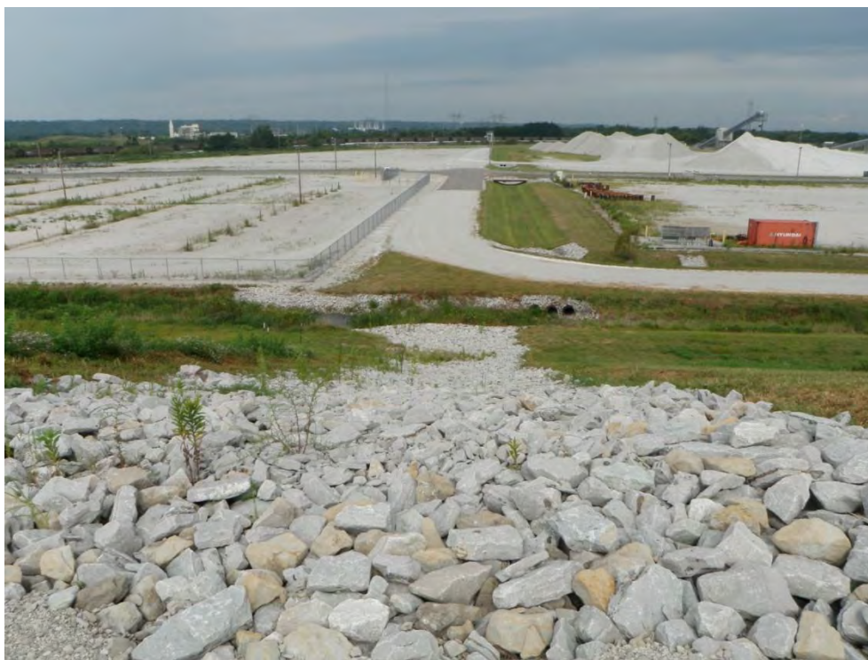
Photo 4: Lined Ash Disposal Pond – Cell #1 – Emergency spillway, west dike, looking west
