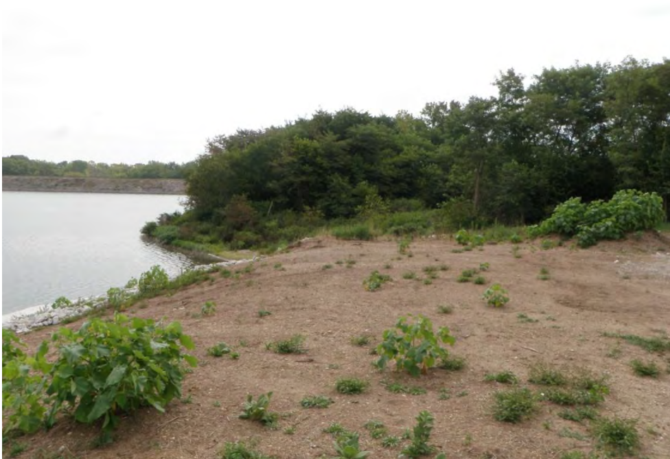
Photo 18: Primary Ash Settling Pond – South embankment upstream slope, looking east
