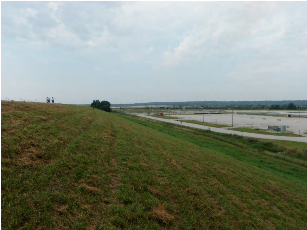
Photo 2: Lined Ash Disposal Pond – Cell #1 – West dike downstream slope, looking southwest
