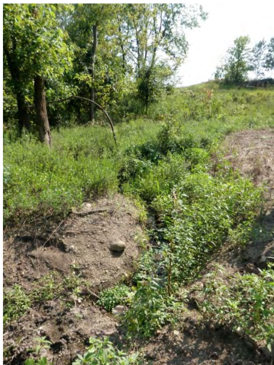
Photo 47: Ash Disposal Area #1 – Downstream of northeast dike downstream toe, note seeps / natural springs, looking southeast
