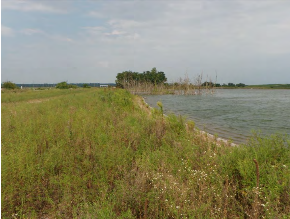
Photo 15: Ash Disposal Area #1 – South embankment upstream slope, looking west
