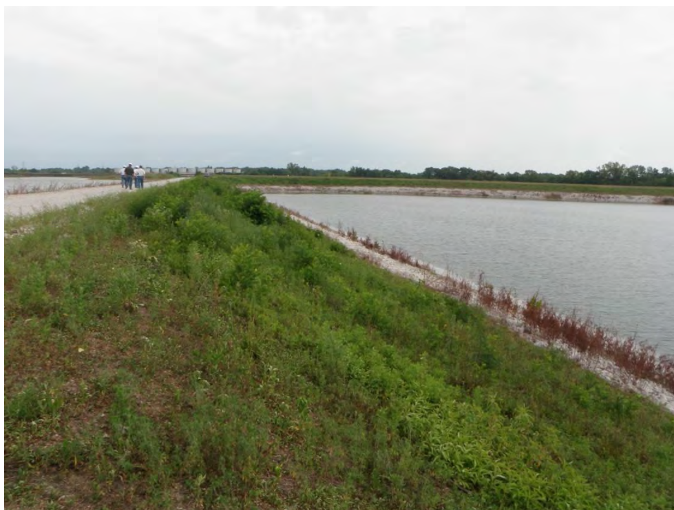
Photo 21: Primary Ash Settling Pond – West dike upstream slope (divider dike with Ash Disposal Area #1), looking north
