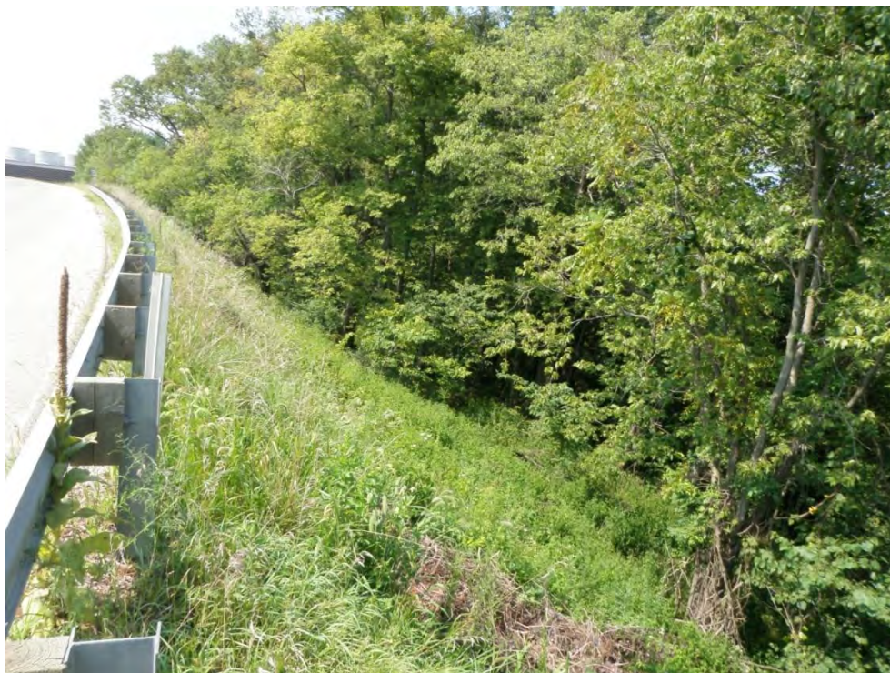
Photo 45: Ash Disposal Area #1 – Northeast corner downstream slope, looking northwest
