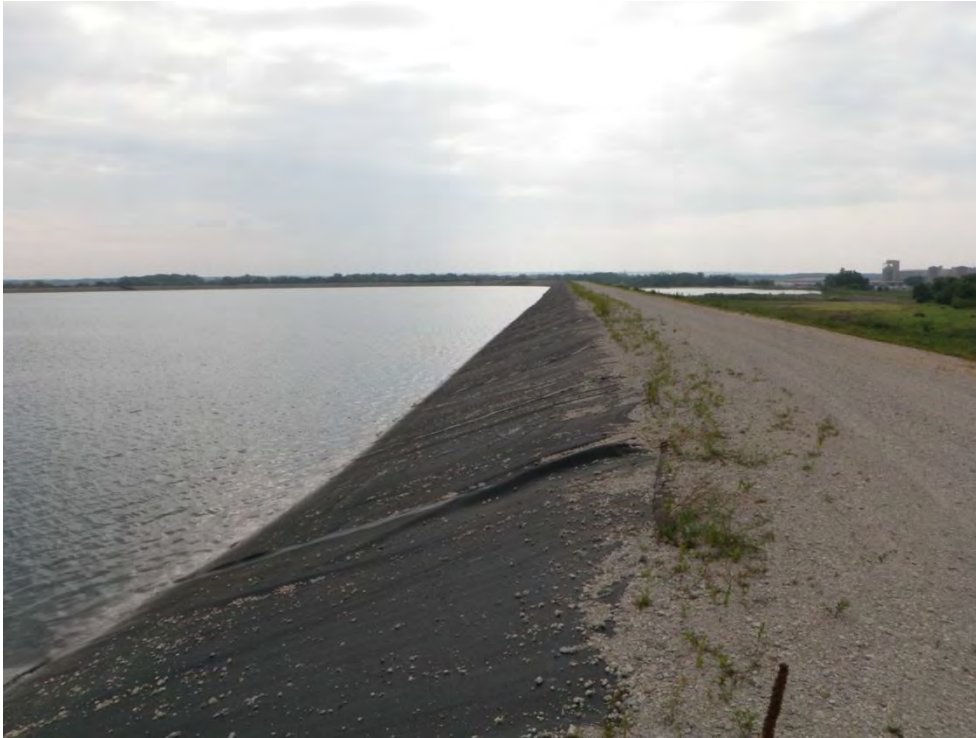
Photo 9: Lined Ash Disposal Pond – Cell #1 – South dike upstream slope, looking east
