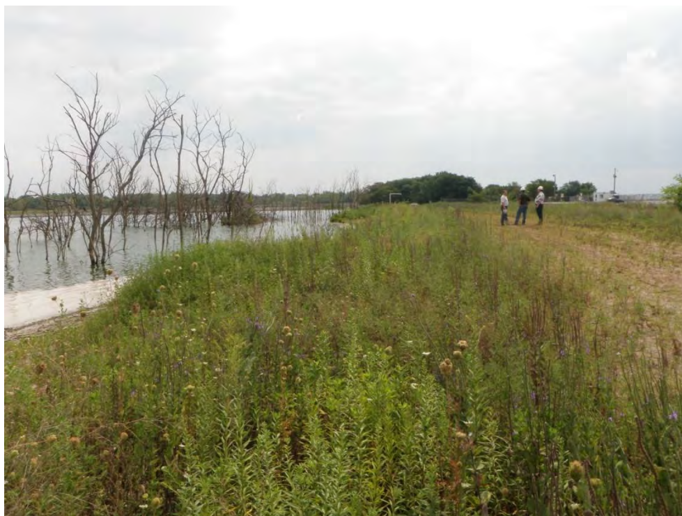
Photo 14: Ash Disposal Area #1 – South embankment upstream slope, looking east
