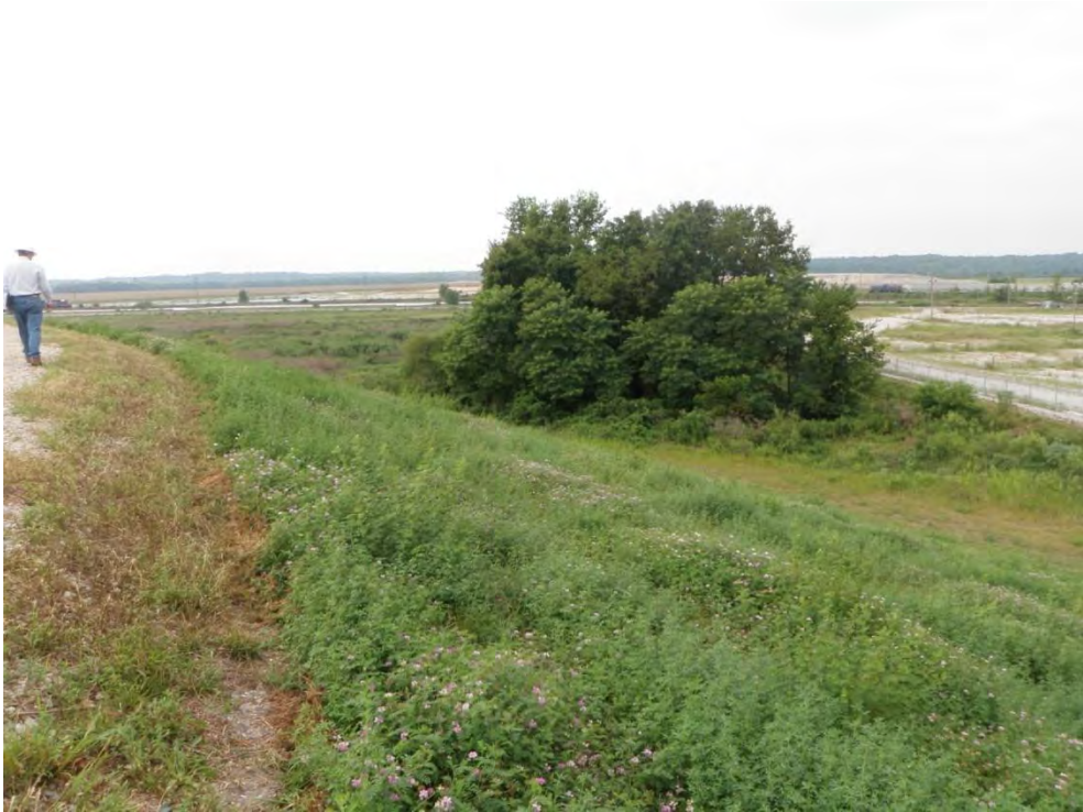
Photo 7: Lined Ash Disposal Pond – Cell #1 – West dike downstream slope, looking south
