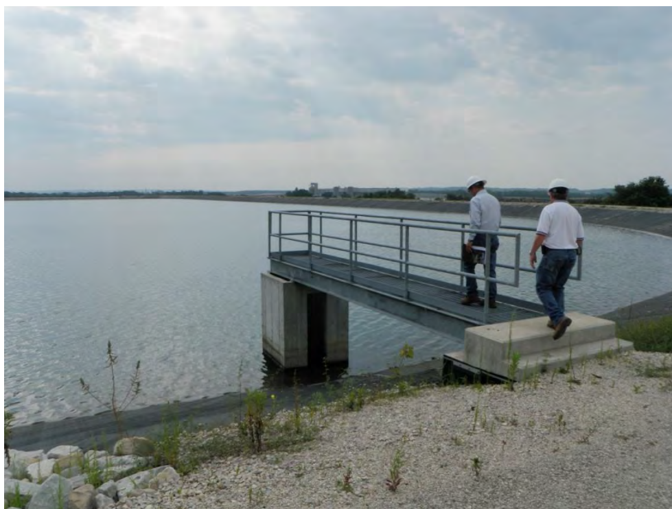
Photo 5: Lined Ash Disposal Pond – Cell #1 – Intake structure, west dike, looking southeast
