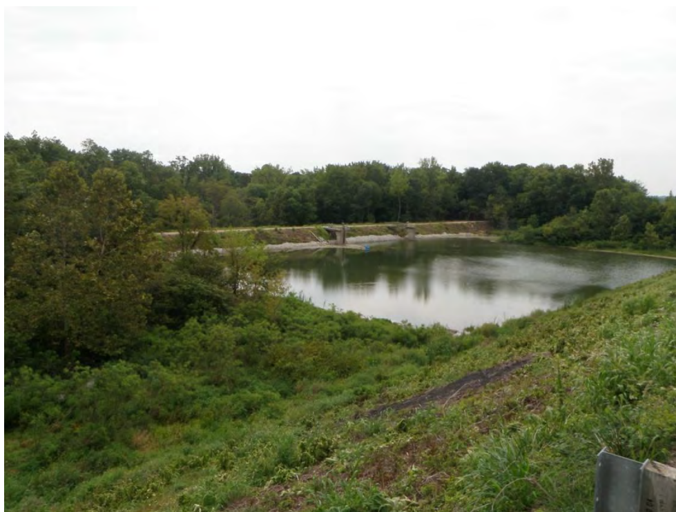
Photo 28: Secondary Ash Settling Pond – looking southeast
