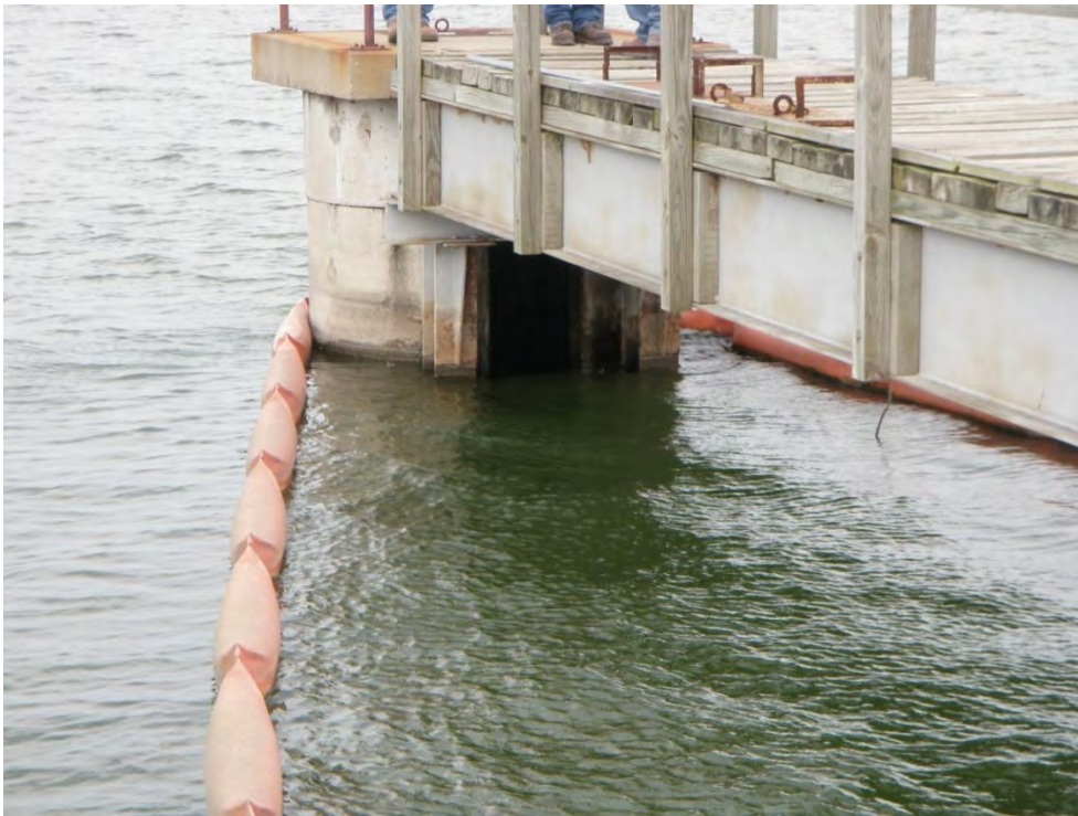
Photo 20: Ash Disposal Area #1 – Intake structure, concrete weir #5
