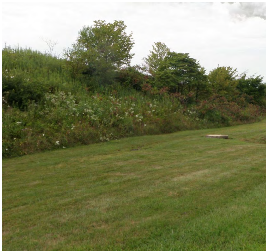
Photo 39: Original Ash Pond – North dike downstream slope, note trees, looking southwest
