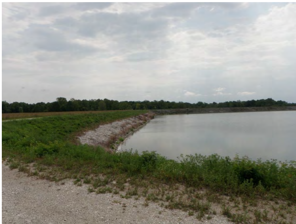
Photo 23: Primary Ash Settling Pond – North dike, upstream slope, looking east
