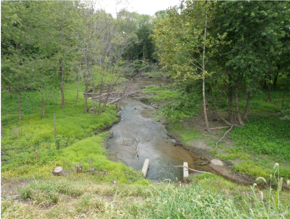
Photo 37: Secondary Ash Settling Basin – Outlet to Wabash River, looking east
