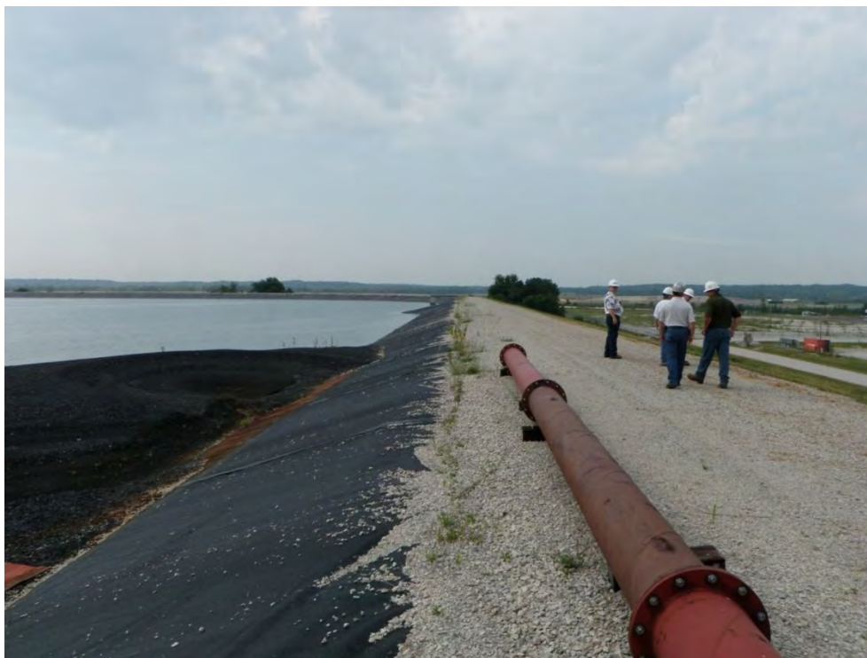
Photo 3: Lined Ash Disposal Pond – Cell #1 – West dike upstream slope, looking south
