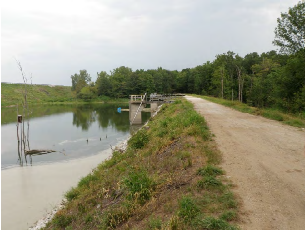
Photo 33: Secondary Ash Settling Pond – East dike upstream slope, looking north
