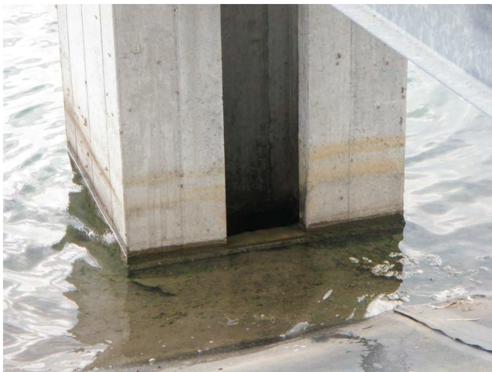
Photo 6: Lined Ash Disposal Pond – Cell #1 – Intake structure, fixed concrete weir
