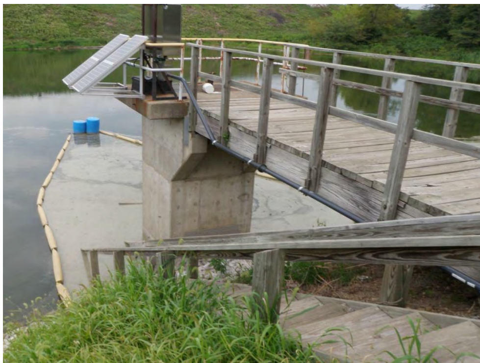
Photo 36: Secondary Ash Settling Basin – Intake structure, weir #4, looking west
