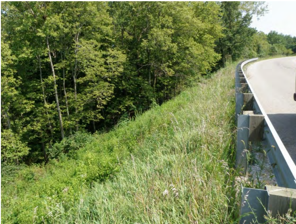
Photo 44: Ash Disposal Area #1 – Northeast dike downstream slope, looking southeast
