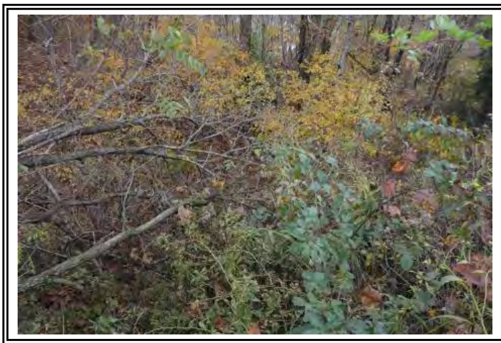
Dense to very dense vegetation on the downstream slope of Pond 7/7A east dike.
