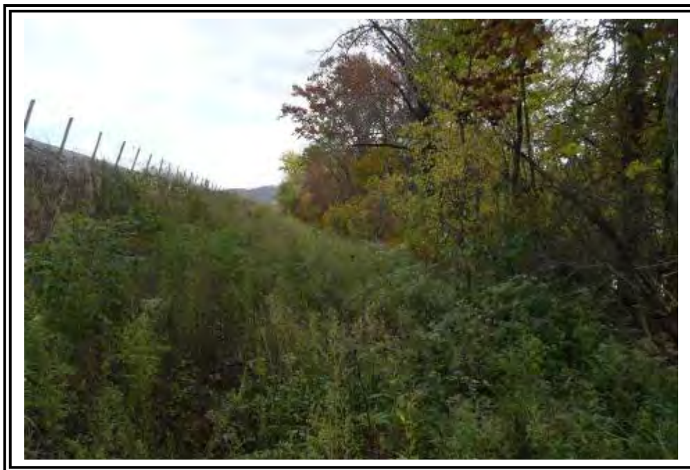
Looking east along the downstream slope of the Pond 7 south dike near the Ohio River bank. Note heavier woody vegetation and trees encroaching on dike toe.
