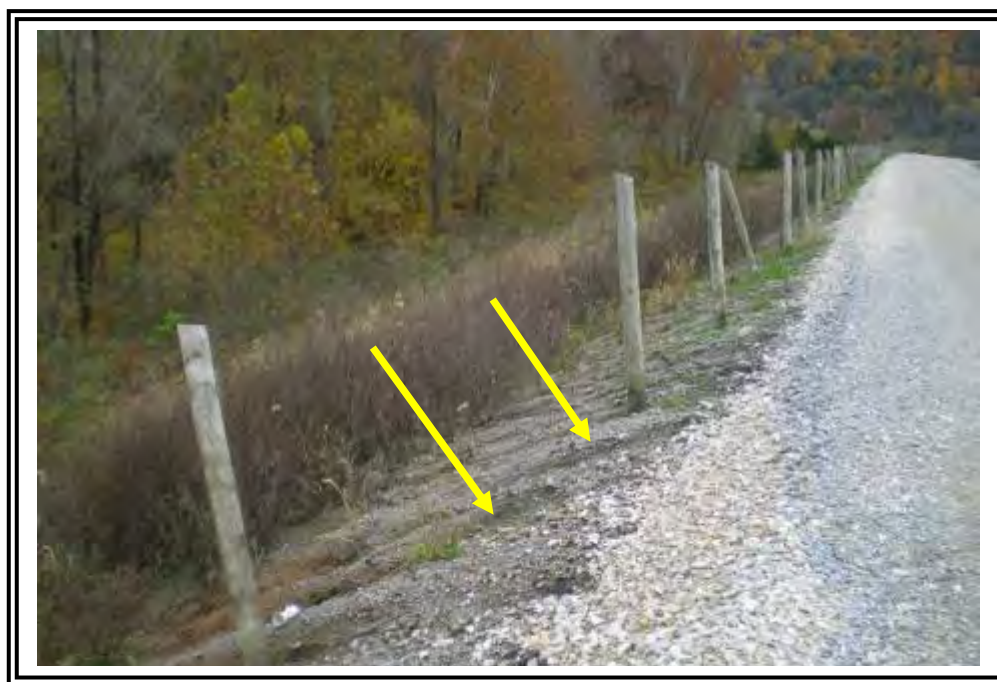
Looking south along the crest and downstream slope of the east dike. Note erosion rills near crest (arrow).
