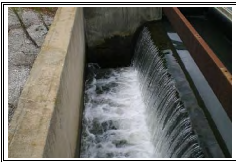
Close-up of outfall structure at Pond 7A
