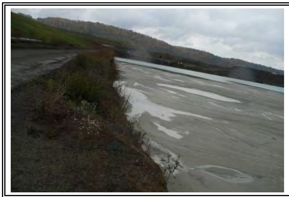
Looking north along the Pond 7 west dike upstream slope. Note ash delta in pond surface.
