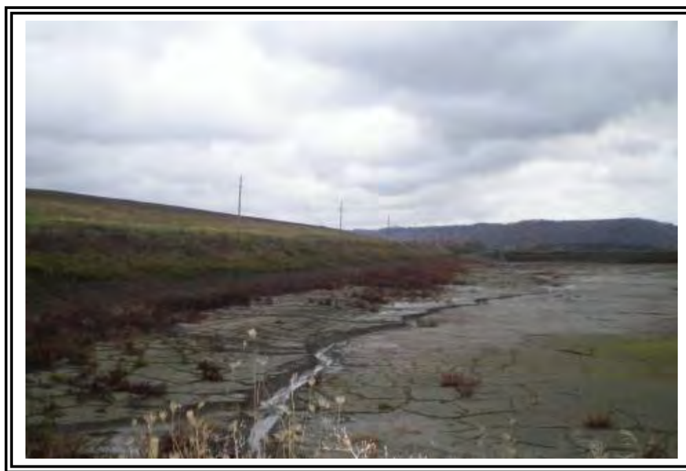
Looking east at upstream slope of the north dike of the pond. There is some beaching just above the ash line on the upstream slope.
