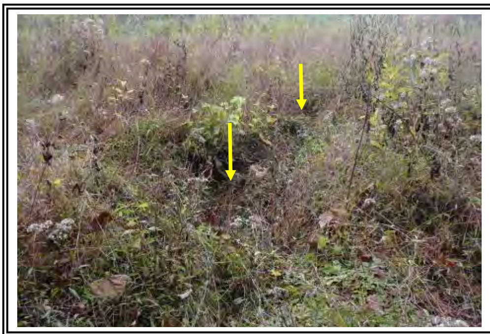
Vegetated erosion rill toward the center of the east dike of Pond 6 approximately 1.0 to 2.0 feet deep.
