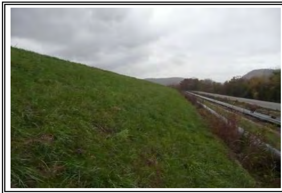
Looking east along the downstream slope of the south dike. Inactive sluice pipe in bench is visible at dike toe.
