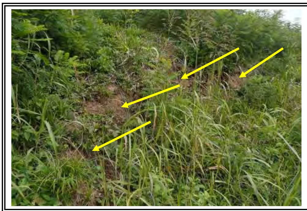
Partially vegetated scarp in heavily vegetated, steeper slope on south side of the pond. Approximately 52 feet long. (See arrows)
