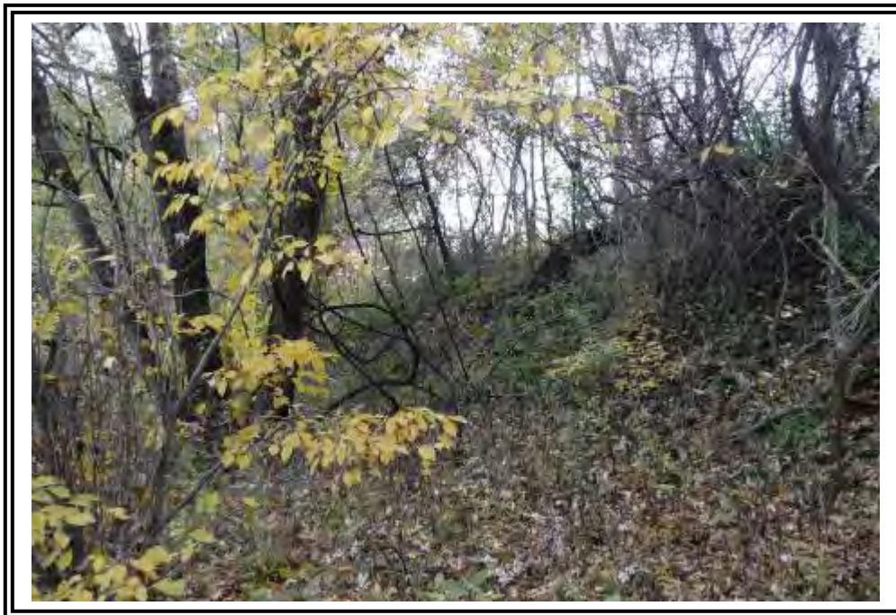
Another view of larger trees at the toe of the downstream slope of Pond 7 near the Ohio River bank.
