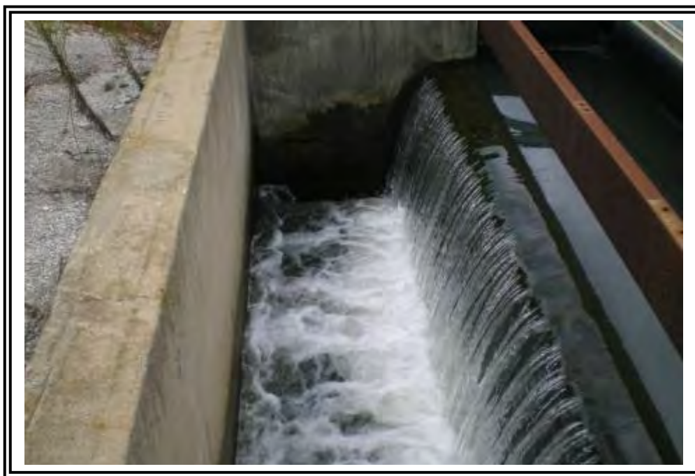
Pond 6 outfall structure at the northeast corner of the pond.
