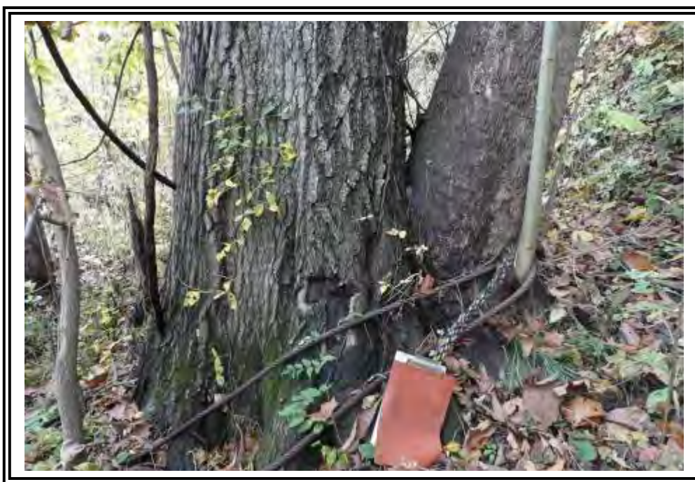
A close up of a large tree on the downstream slope of Pond 7 south dike near the Ohio River bank.
