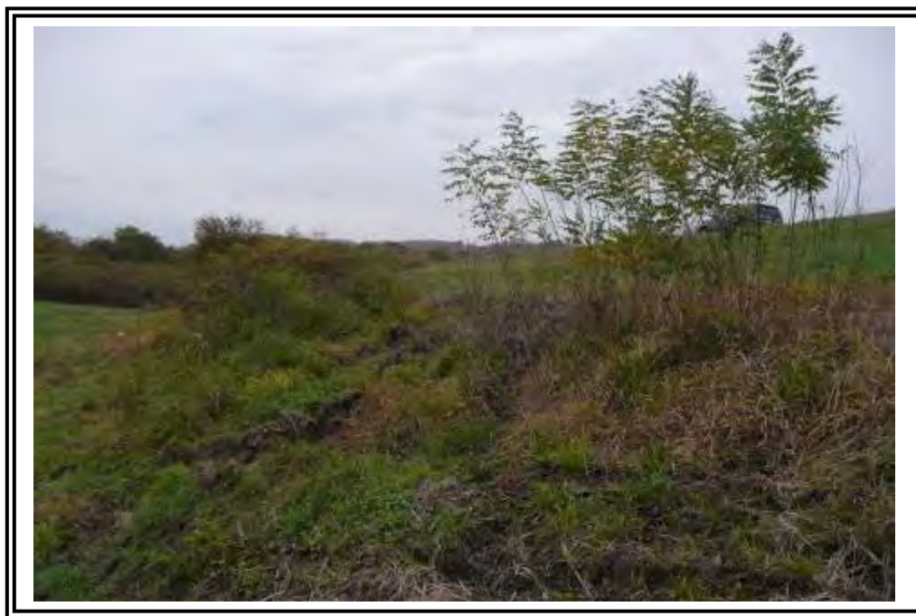
Seep softened and deformed area with denser vegetation on the downstream slope at the southwest end of the pond.
