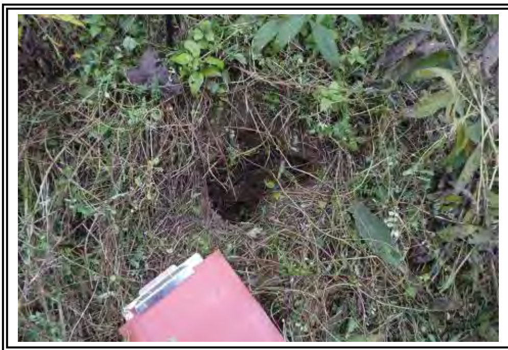
Close up of a potentially abandoned rodent hole in the downstream slope of Pond 7/7A east dike.
