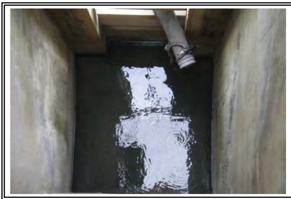
Close up of inside the outfall structure.
