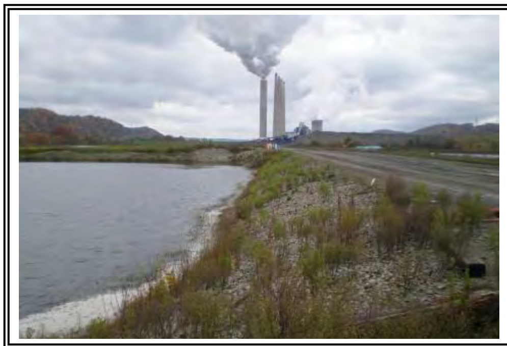
Looking west along the Pond 7/7A north dike upstream slope impounding Pond 7A. Note gravel slope surface and freeboard at this location of the dike.
