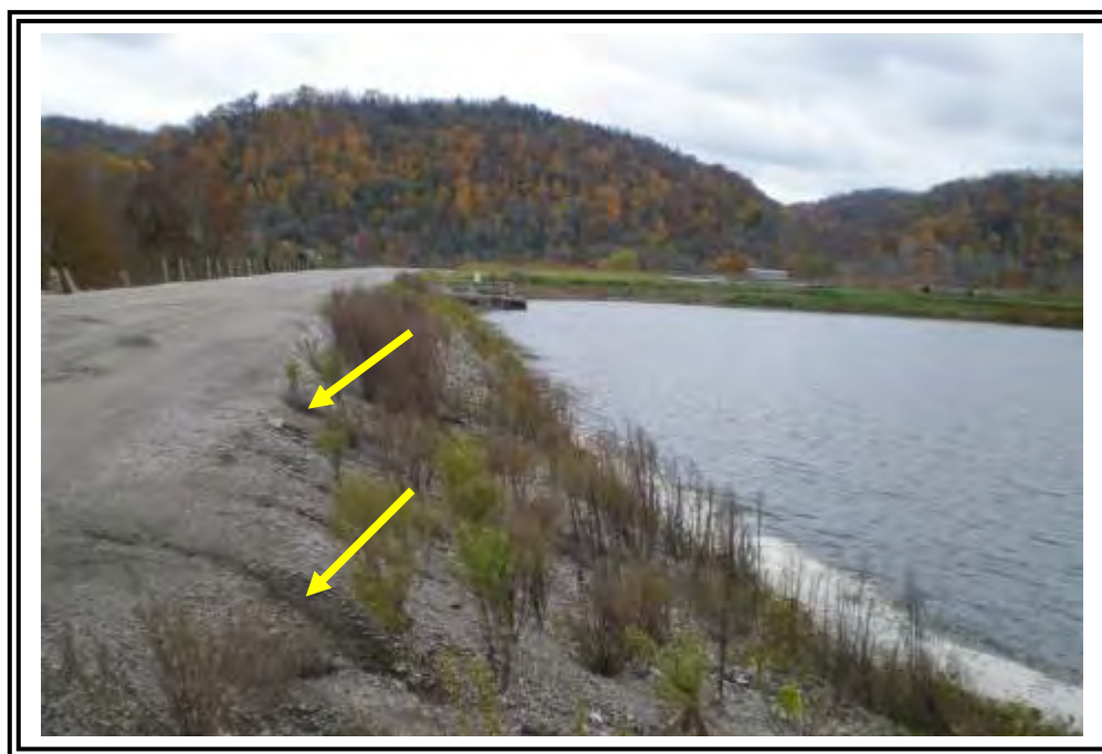
Looking south along the crest and upstream slope of the Pond 7A east dike. Note the erosion rills at the crest (arrows).
