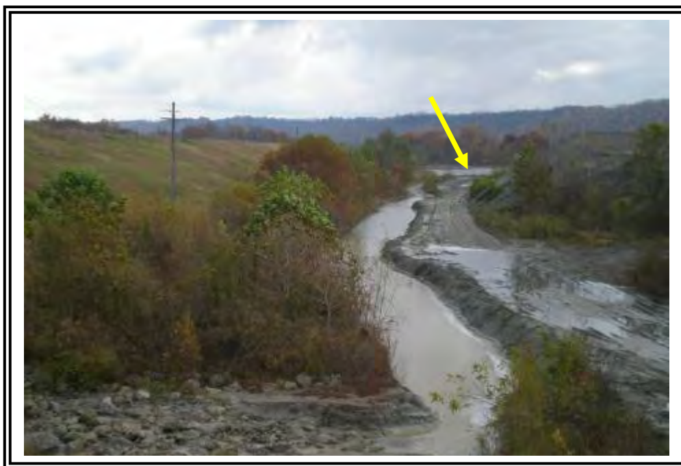
Looking east at the discharge channel that conveys effluent from Pond 10 and Pond 3A into Pond 6. Open water in Pond 6 is in distant background (see arrow).
