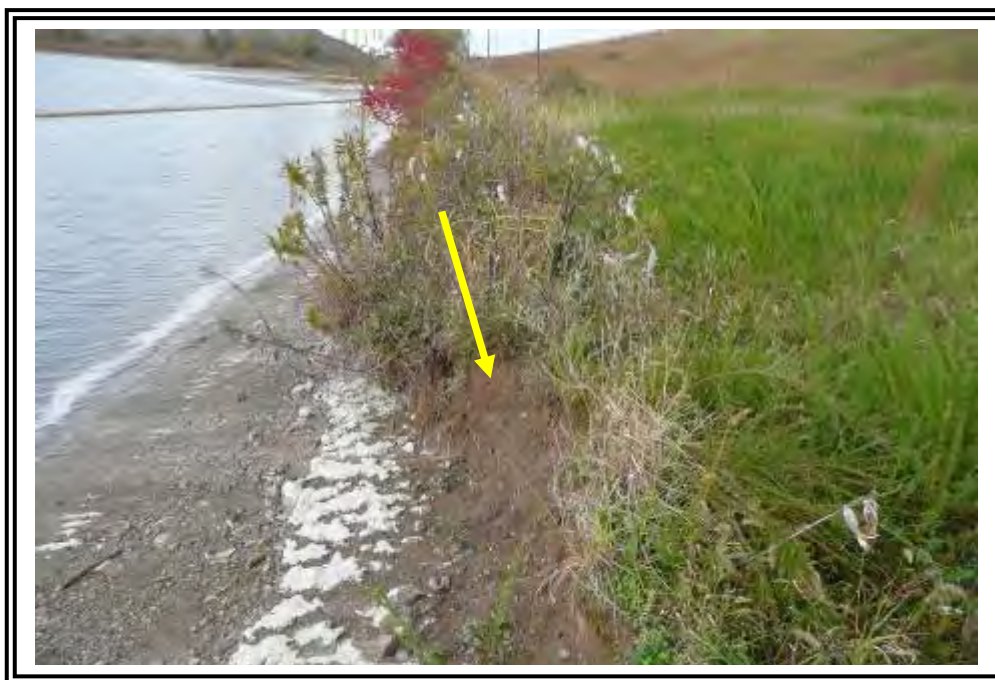
Looking west at beaching erosion (arrow) on north wall of Pond 6. Recent high water level is evident from deposited ash in picture.
