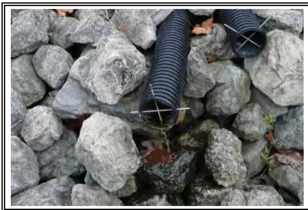
Close up of the drainage pipes that empty into the riprap drainage swale.
