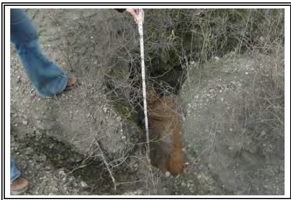
Close up of deep erosion rill in the Pond 6 side of the separator dike.
