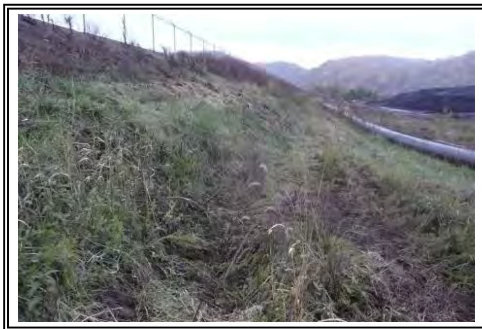
Looking south along the downstream slope at over-steepened area of the west dike of pond. Note sluice pipe near dike toe.
