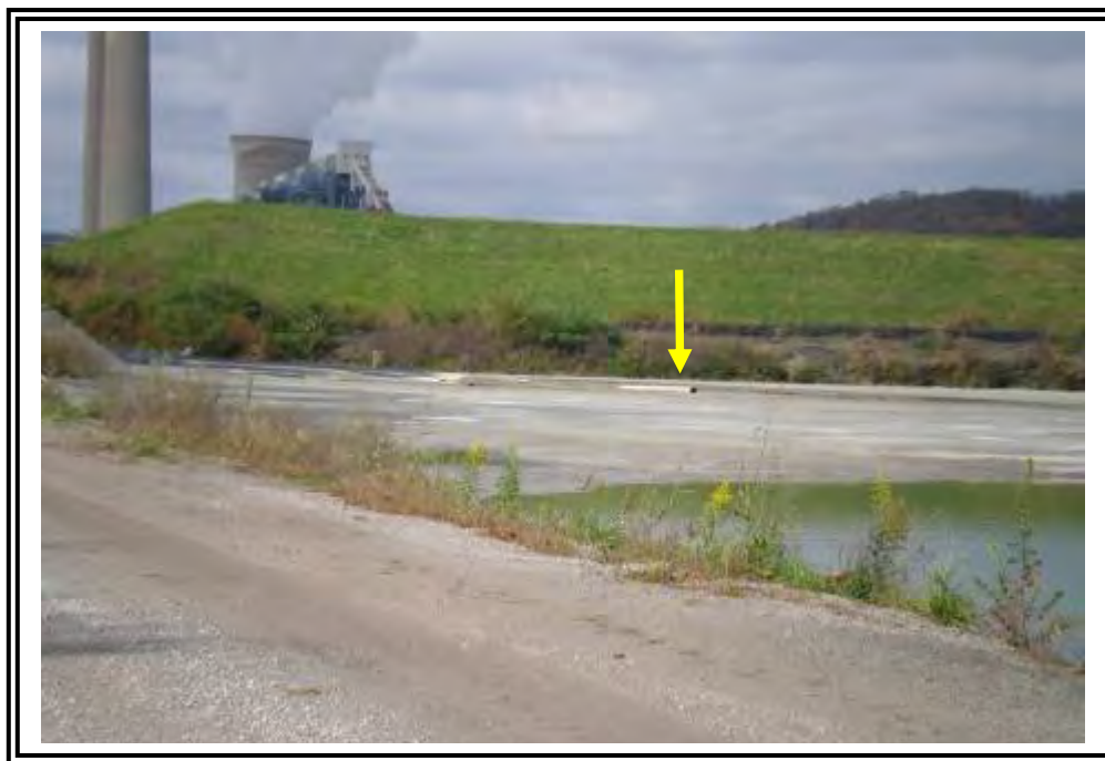
Looking at the northwest corner of Pond 7 showing ash delta and sluice lines (arrow). Pond 3A's east dike is in the background.
