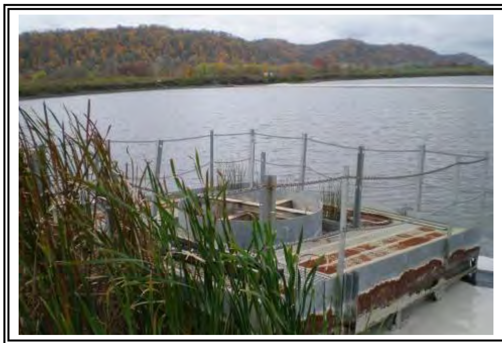
Close up of the old outfall structure.
