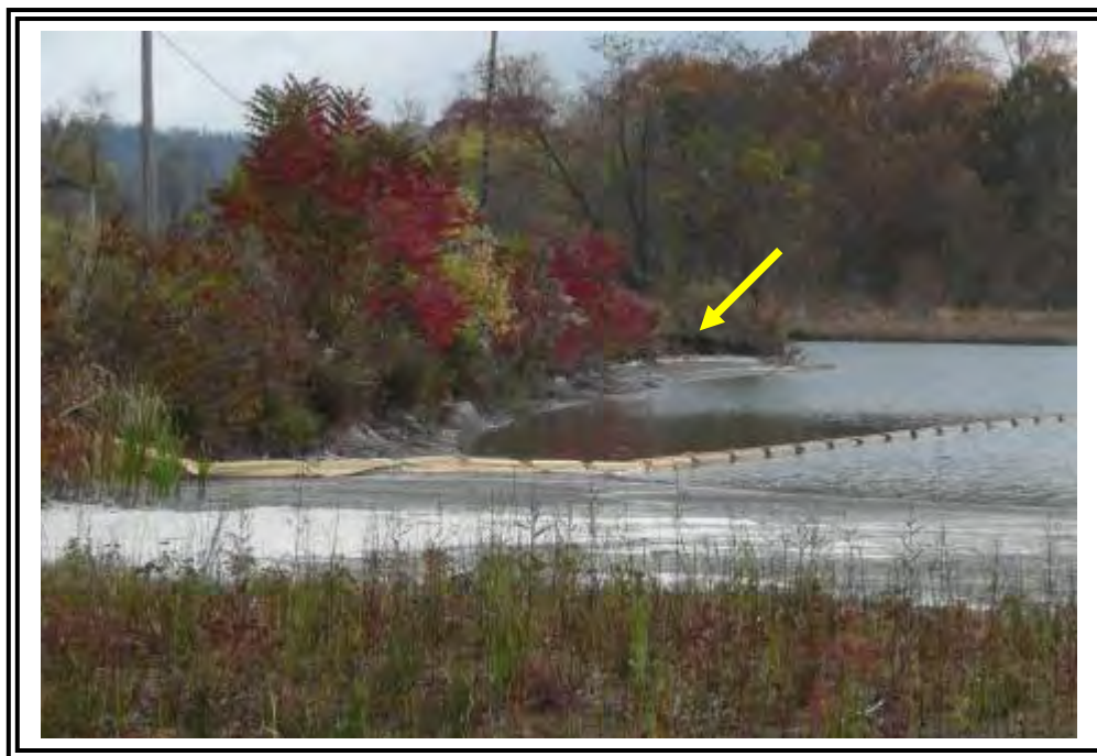
Vegetation on north dike of Pond 6 and beaching erosion (arrow), looking east.
