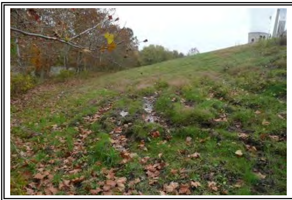
Looking east along the downstream slope of the northern dike. Notice the taller grass and rutting with standing seep water.
