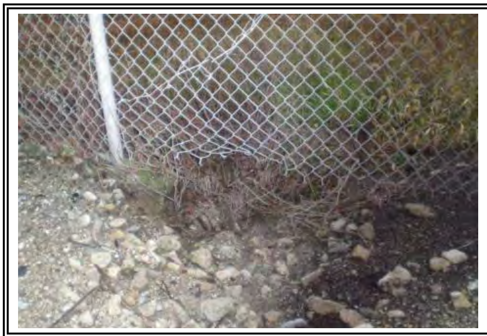
Close up of erosion at edge of crest under the fence on the west dike of pond.
