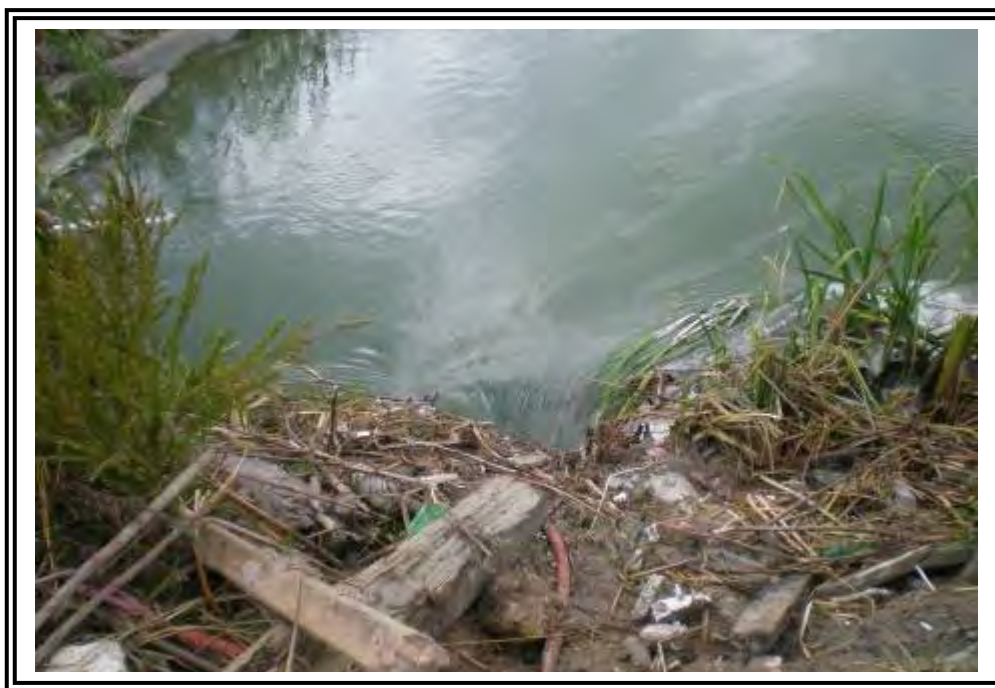
Submerged outlet structure for Pond 7 to Pond 6. Note absence of inlet protection.
