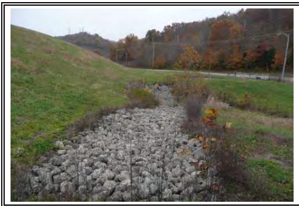
Looking northwest along the riprap drainage swale at the north tip of the pond
