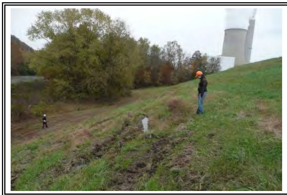
Looking east at the downstream slope of the northern dike near the middle of the pond where some seepage, subsequent softening, and slope deformation due to rutting has occurred.
