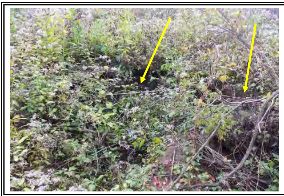
Deep, heavily vegetated erosion gullies on downstream east dike slope of Pond 6. These were 3.5 to 4 feet deep located near the north end of the dike.
