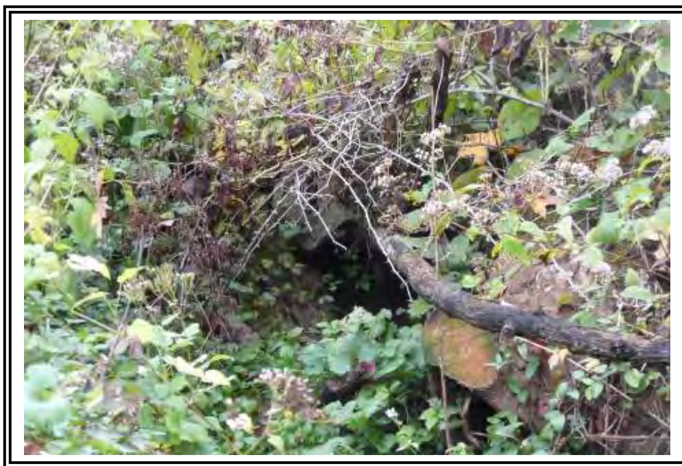
Close up of a possible rodent burrow or animal cave in the dense vegetation on the downstream slope of Pond 6 east dike.
