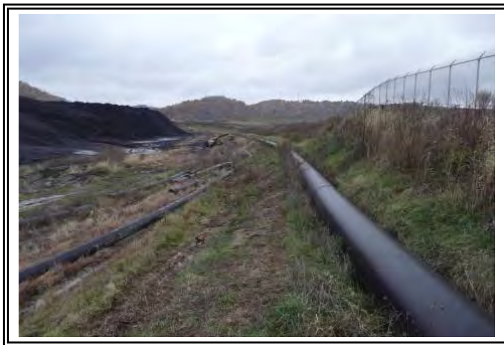
Looking north along the downstream slope of the west dike from the south end. Note sluice pipe on slope.
