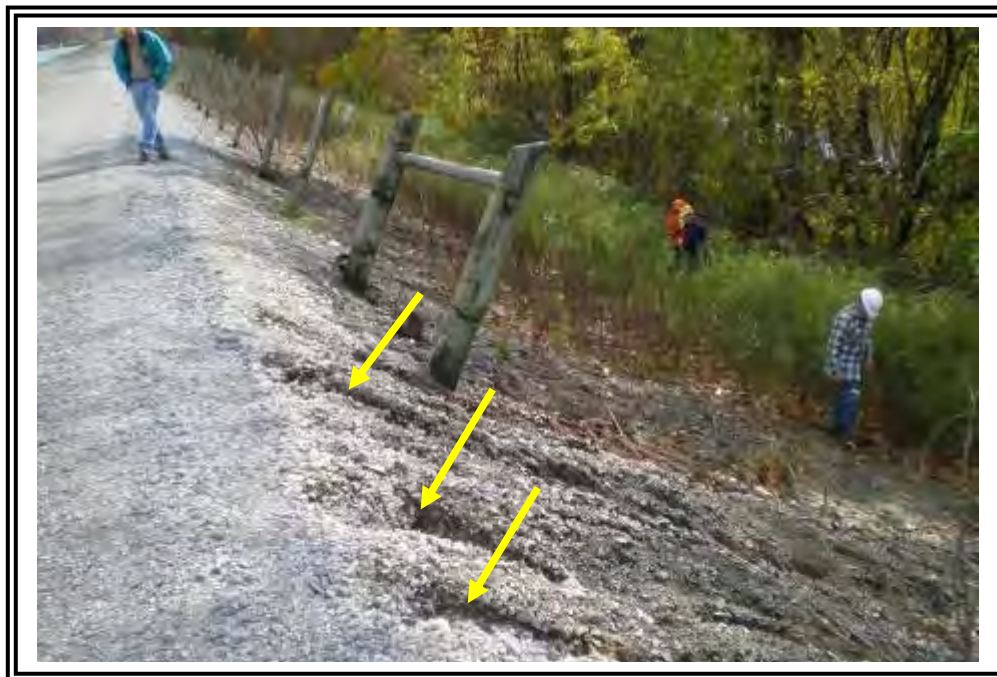
Looking east along the crest and downstream slope of Pond 7 south dike. Note erosion rills in slope (arrows)
