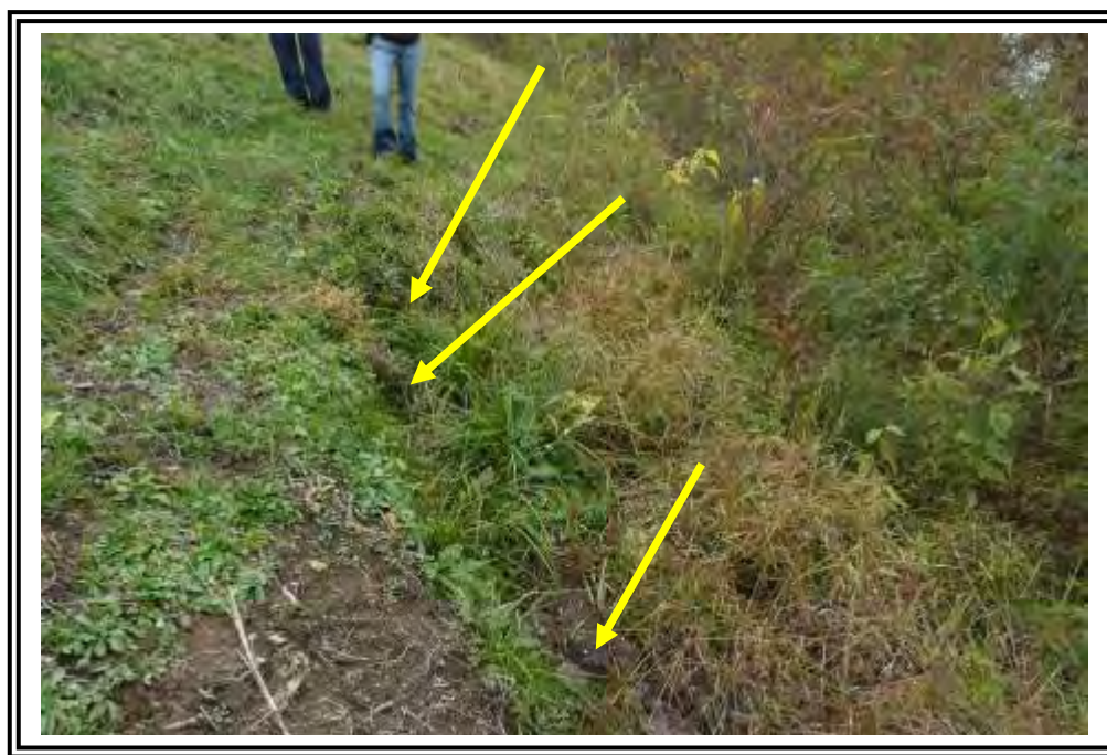
Vegetated scarp with standing water on west side of the pond. Approximately 30 feet long. (See arrows)
