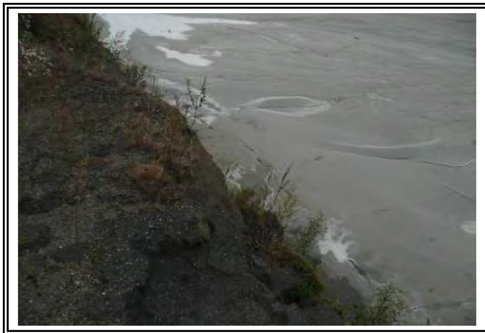
Close-up of steep upstream slope and looser material on western dike of Pond 7.
