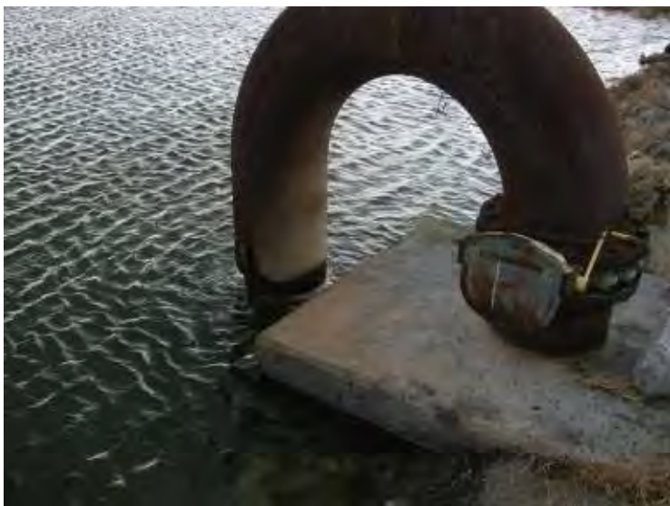
Photo 37: Ash Cell No. 1 – Metal inlet pipe (15-inch diameter) & submerged Splash pad, looking west.
