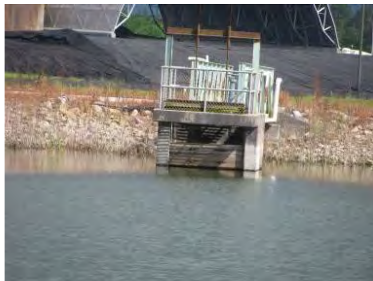
Photo 30: Ash Cell No. 2 – Northwest embankment, outlet structure with stop logs southeast divider embankment interior slope, looking southeast.
