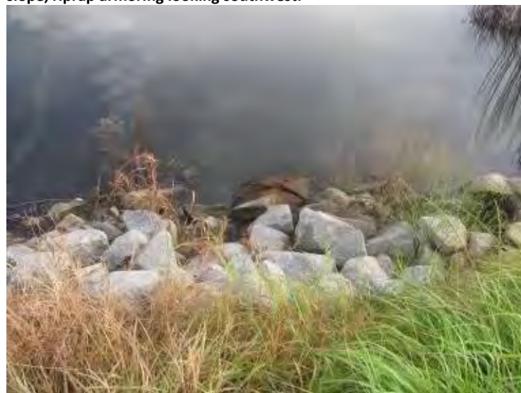
Photo 48: Coal Stockpile Runoff Collection Pond – south embankment interior slope, rusted corrugated inlet metal pipe looking north.
