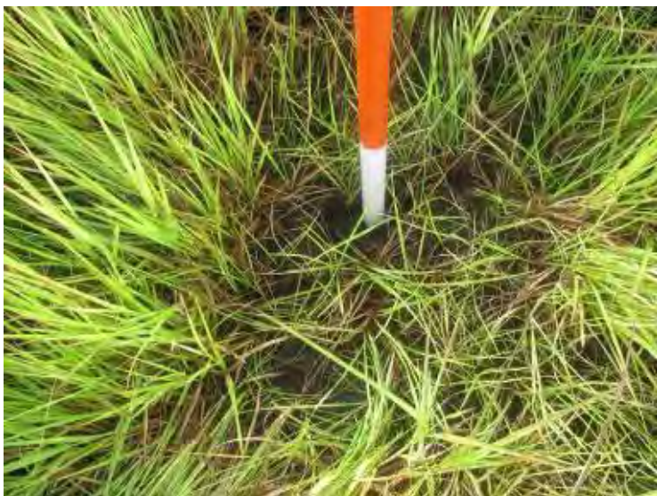
Photo 85: Ash Cell No. 2 – Northwest embankment exterior slope, saturated area along toe of slope, looking southeast.
