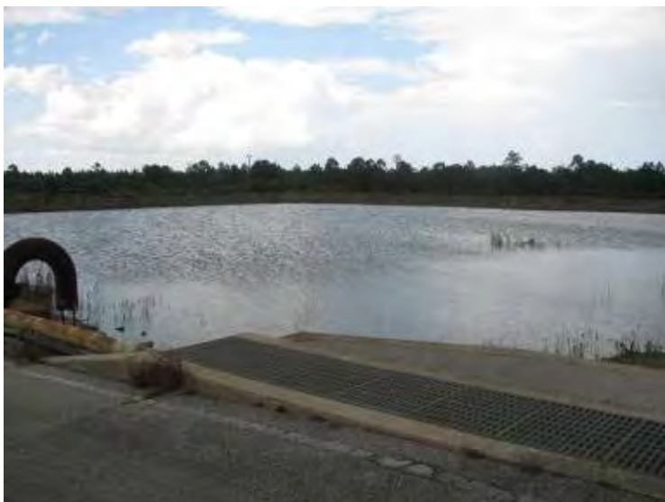
Photo 41: Ash Cell No. 2 – General view of pond looking north. Note concrete U-shaped channel and metal grate to protect sluice ash pipelines.
