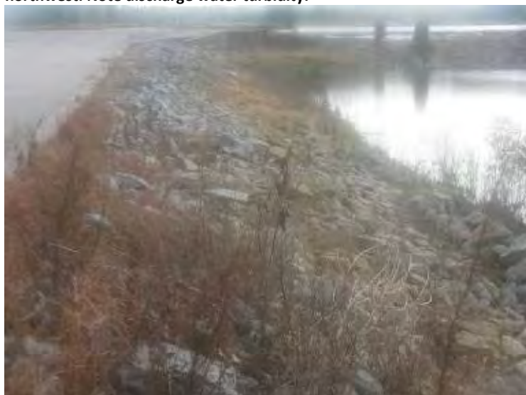
Photo 47: Ash Cell No. 2 – Northwest divider embankment interior slope, rip-rap slope treatment looking southwest.
