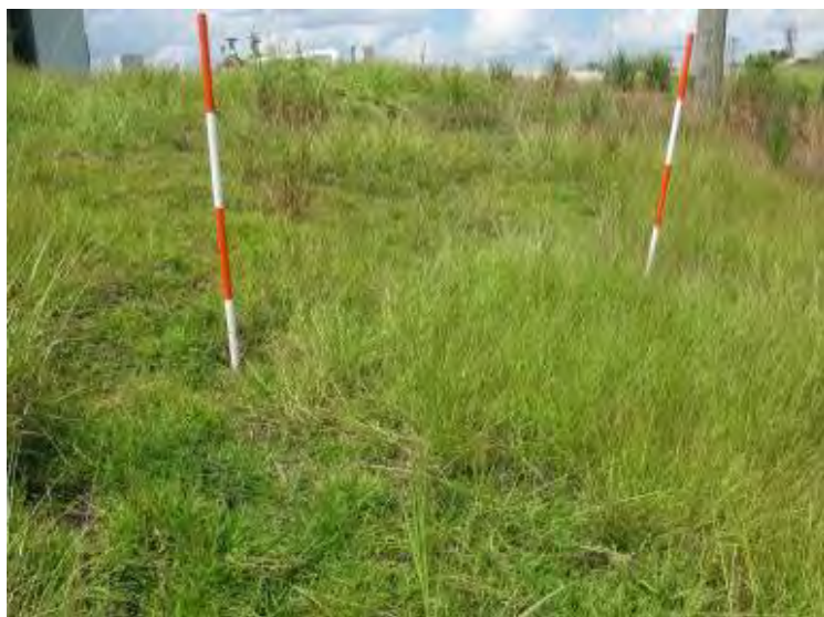
Photo 5: Pump Back Cell No. 1 – Southeast embankment exterior slope, minor surficial erosion rills looking northeast.
