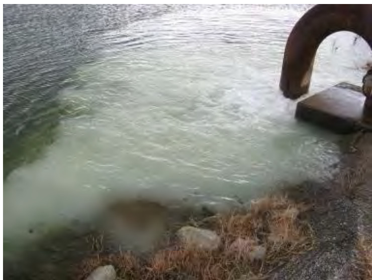
Photo 45: Ash Cell No. 1 – Inlet metal pipe (15-inch diameter), looking northwest. Note discharge water turbidity.
