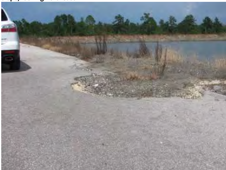
Photo 27: Ash Cell No. 2 – Northwest embankment interior slope, erosion along top of slope looking southeast. Note pavement distress.
