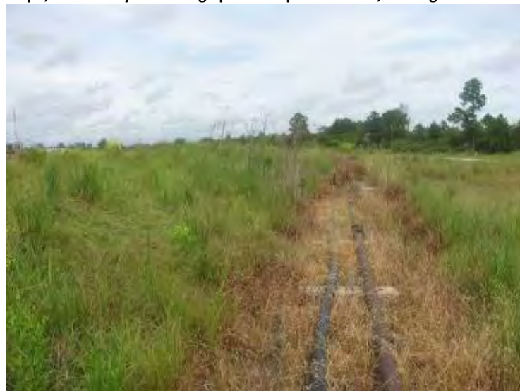
Photo 96: Lime Sludge Pond No. 2 – Northeast embankment exterior slope, looking northwest. Note lime sludge pipes on ground.
