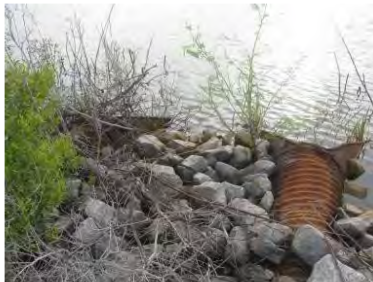
Photo 62: Coal Stockpile Runoff Collection Pond – West embankment interior slope, upstream side of 24-inch diameter metal outlet pipes, looking east. Pipes are partially crushed and blocked. No flow was observed.
