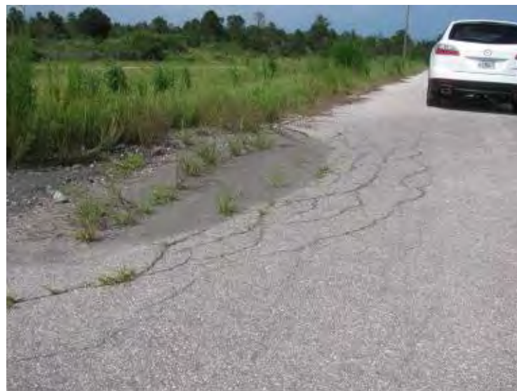
Photo 26: Ash Cell No. 2 – Northwest embankment exterior slope, erosion along top of slope, looking north. Note pavement distress.
