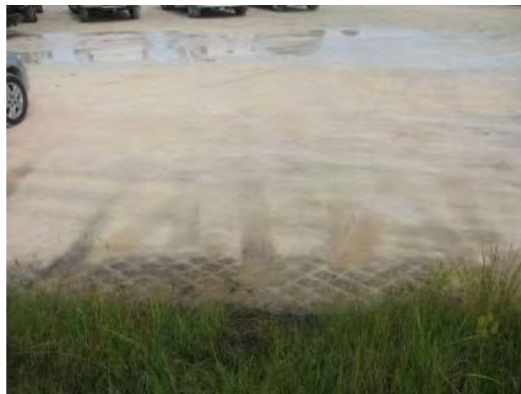
Photo 82: Ash Cell No. 1 – Northwest embankment exterior slope, ponded water and saturation along toe of slope, looking northwest.
