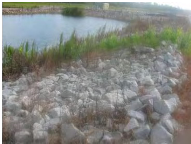
Photo 46: Pump Back Cell No. 2 – Northwest divider embankment interior slope, riprap armoring looking southwest.
