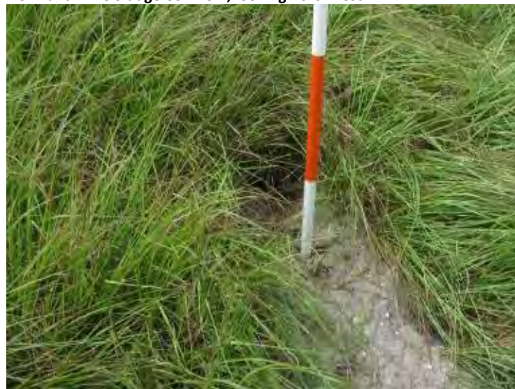
Photo 16: Lime Sludge Cell No. 2 – Animal burrow, southeast embankment exterior slope, looking northwest.
