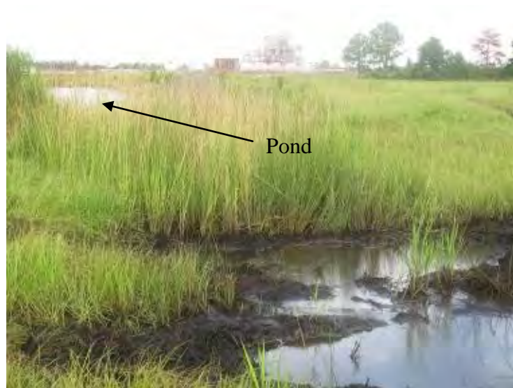
Photo 54: Coal Stockpile Runoff Collection Pond – Runoff swale at toe of north embankment, looking west.
