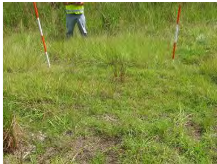
Photo 6: Pump Back Cell No. 1 – Southeast embankment exterior slope, minor erosion rills looking southeast.
