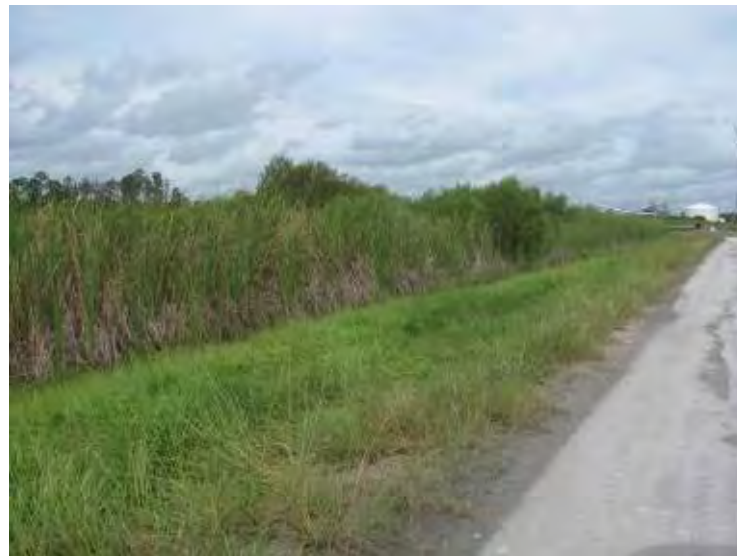
Photo 98: Stormwater Pond – Northeast embankment interior slope, looking west. Note areas of dense vegetation (i.e. – cattails).
