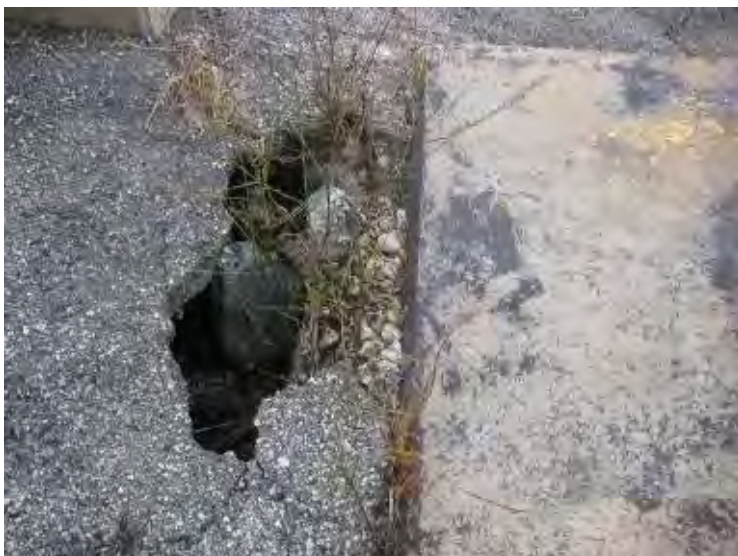
Photo 35: Ash Cell No. 2 – Erosion of slope pavement behind inlet pipe shown in previous photo.
