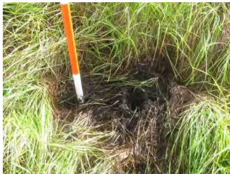
Photo 78: Ash Cell No. 1 – Southwest embankment exterior slope, saturated area along exterior toe of slope (typical), looking northeast.
