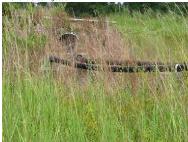
Photo 12: Pump Back Cell No. 2 – Southeast embankment exterior slope, 24-inch dia. corrugated culvert pipe below access road between Pump Back Cell No. 2 and Lime Sludge Cell No. 2, looking northeast. Note lime sludge pipes.
