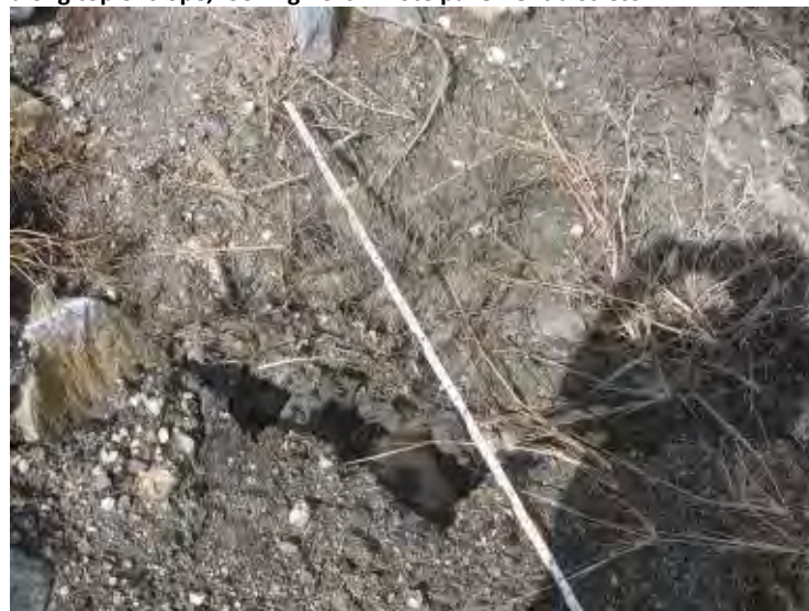
Photo 28: Ash Cell No. 2 – Northwest embankment interior slope, erosion rill looking southeast. (typical of several)
