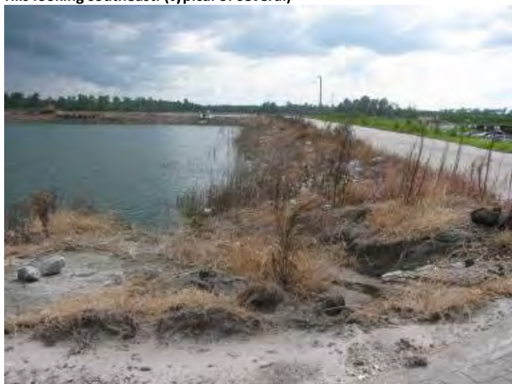
Photo 31: Ash Cell No. 2 – Northwest embankment interior slope, erosion along edge of crest looking south.
