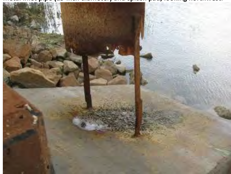
Photo 36: Ash Cell No. 2 – Close up of splash pad looking north. Note rusted end of inlet pipe and eroded concrete.
