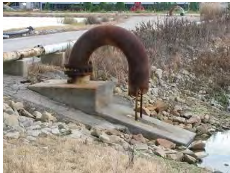
Photo 34: Ash Cell No. 2 – Southwest divider embankment interior slope, metal inlet pipe (15-inch diameter) and splash pad, looking northwest.
