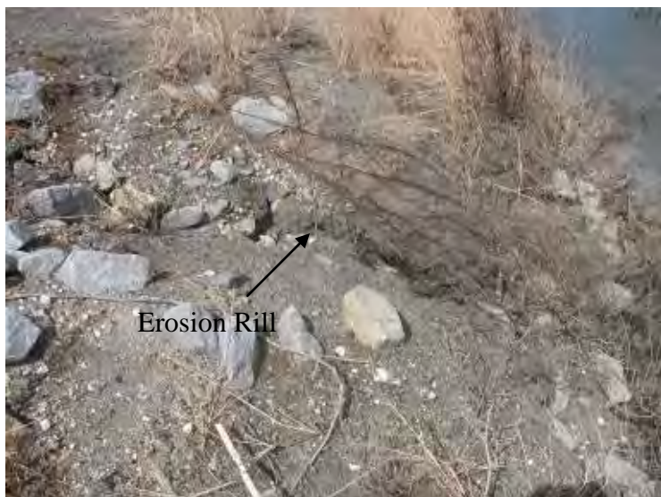
Photo 29: Ash Cell No. 2 – Northwest embankment interior slope, erosion rills looking southeast. (typical of several)
