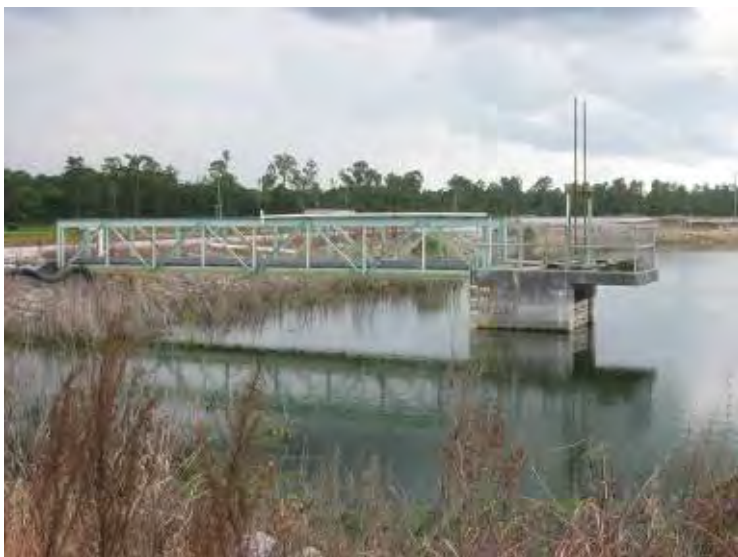
Photo 33: Ash Cell No. 2 – Outlet structure/stop logs looking southwest.
