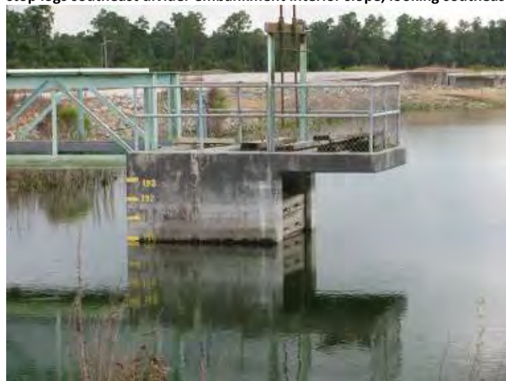
Photo 32: Ash Cell No. 2 – Outlet structure/stop logs and staff gage, looking southwest.
