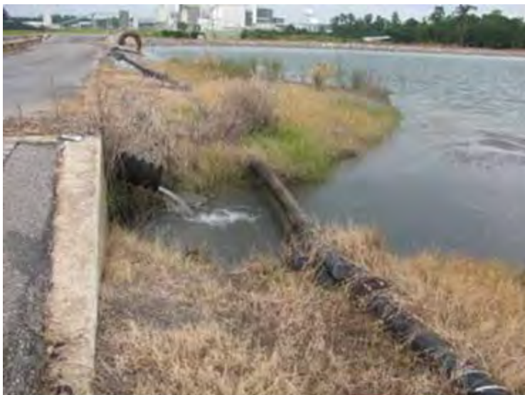
Photo 43: Ash Cell No. 1 – Inlet pipe and northeast divider embankment Interior slope, looking southeast. Note abandoned HDPE pipe.
