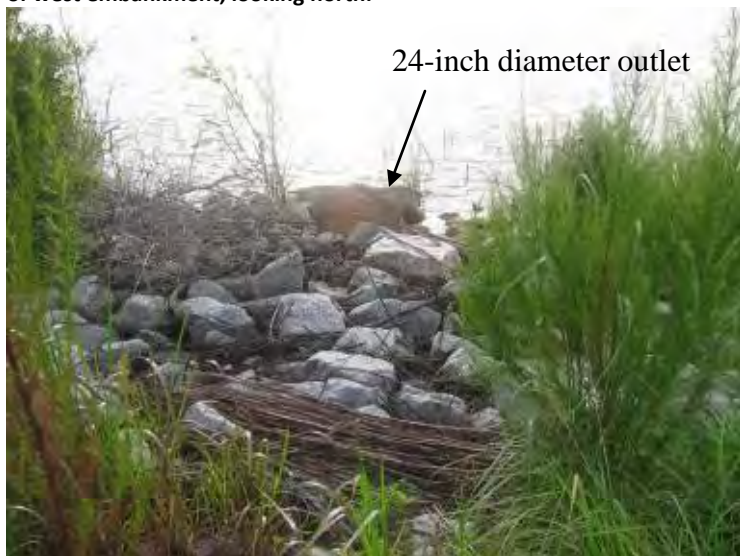
Photo 59: Coal Stockpile Collection Pond – West embankment interior slope upstream side of 24-inch diameter metal outlet pipe, looking east. Pipes are partially crushed and blocked. No flow was observed.
