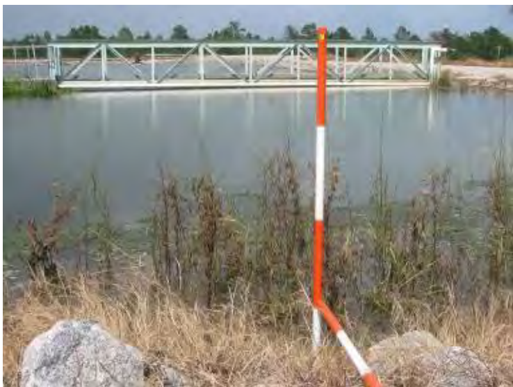
Photo 21: Ash Cell No. 1 – Southwest embankment interior slope, view of pond surface showing 1-foot of freeboard looking northeast.
