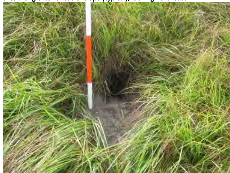
Photo 80: Ash Cell No. 1 – Animal burrow, northwest embankment exterior slope, looking southeast.
