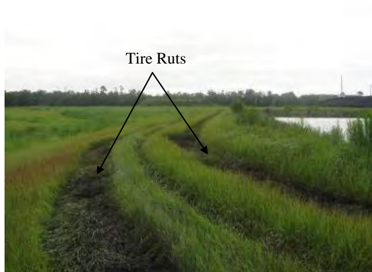
Photo 64: Coal Stockpile Runoff Collection Pond – Crest of north embankment, looking east. Note tire ruts.
