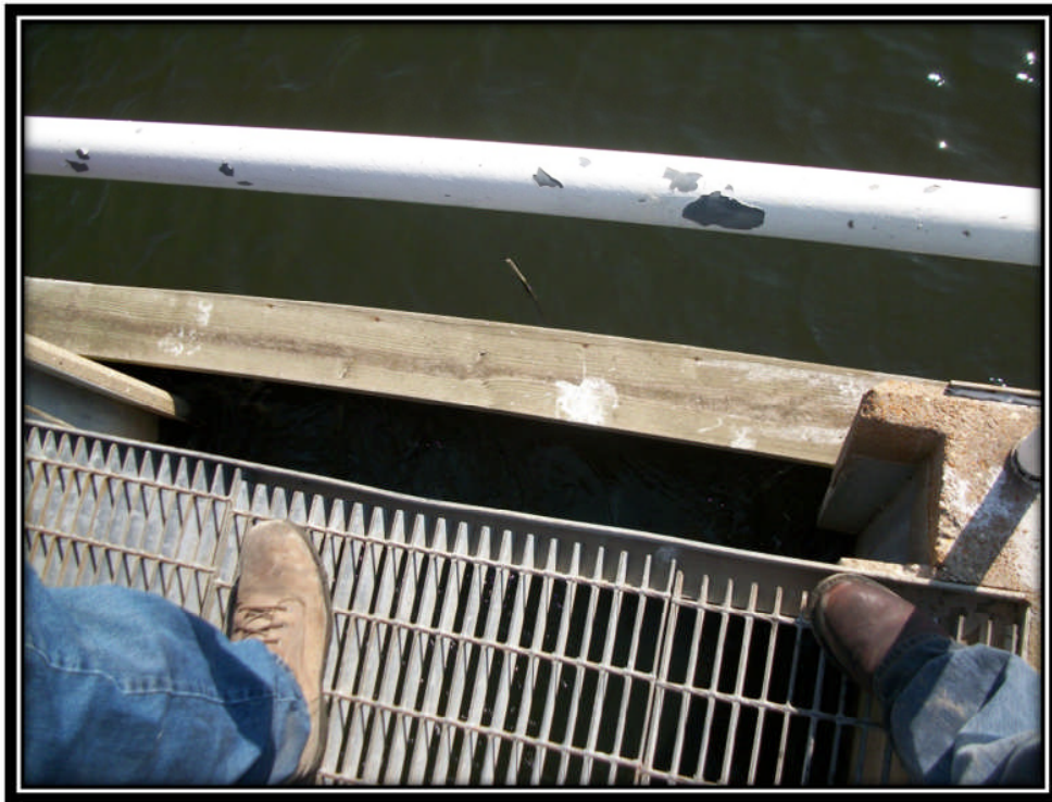
Photo 21 – Clarification Pond Outlet Structure Intake
