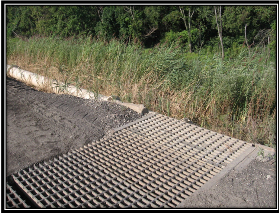
Photo 9 – Grate on Crest Providing Roadway Access Over Sluice Pipe Inlet into Dallman Ash Pond
