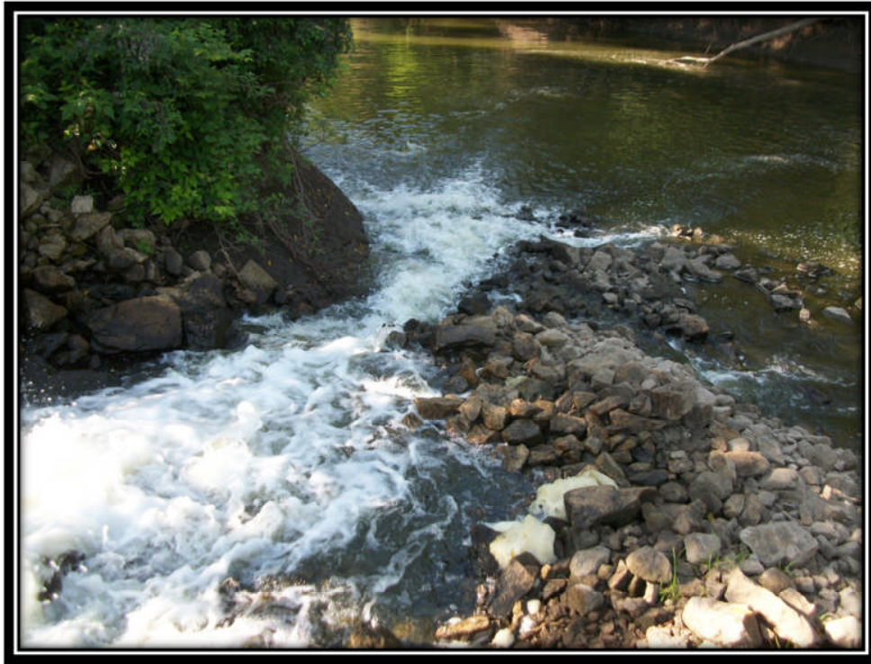
Photo 19 – Channel from Clarification Pond Outlet Piping (Note Riprapped Channel)
