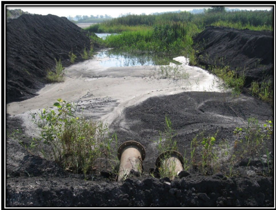
Photo 10 – Alternate Sluice Pipes (Not Active during Inspection, Note Cut in Embankment)
