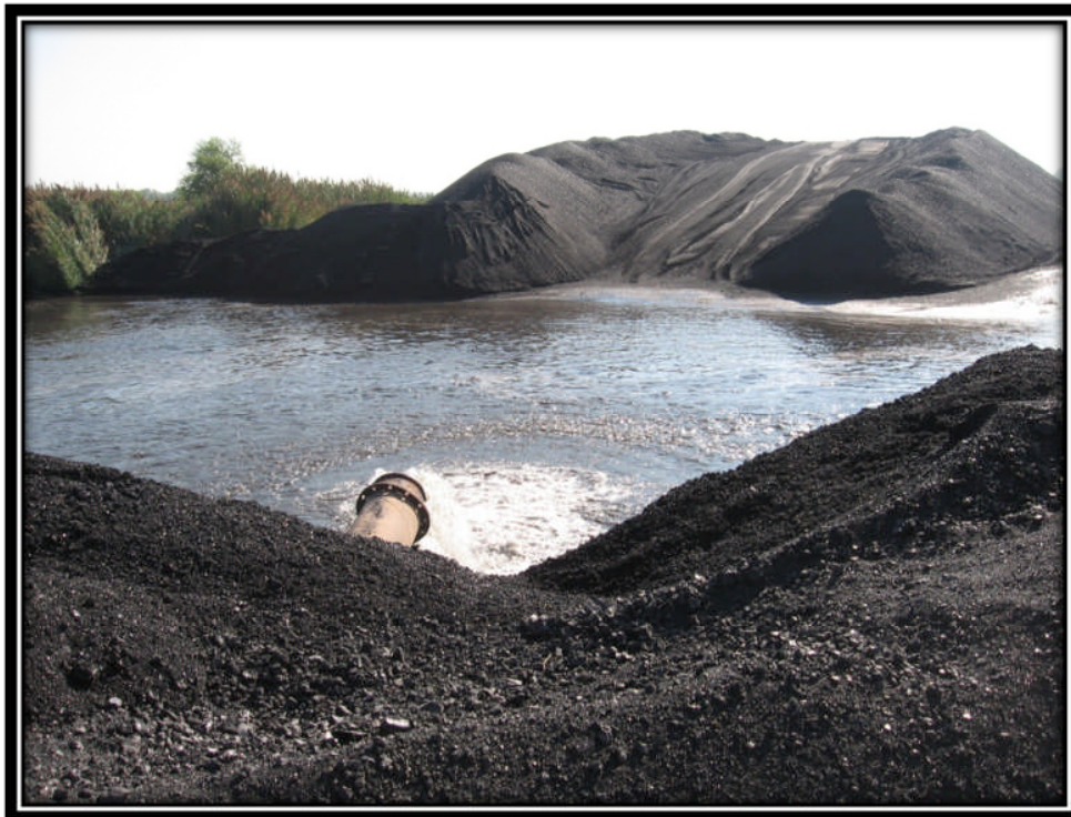
Photo 12 – Boiler Slag Sluice Pipe into Dallman Ash Pond (Note Backfilled Embankment)
