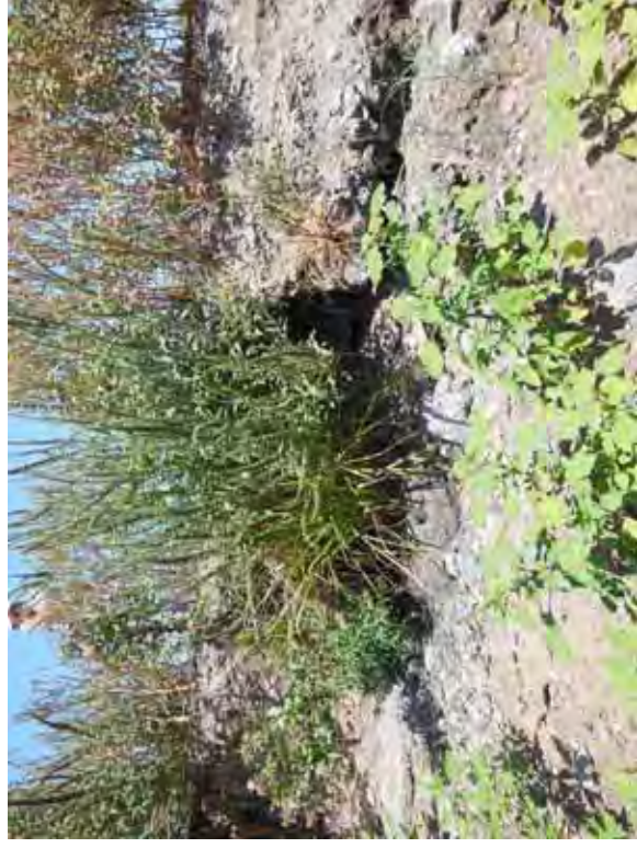
Photo 25: NP/SP - Vegetation and ash material on common embankment south slope.
