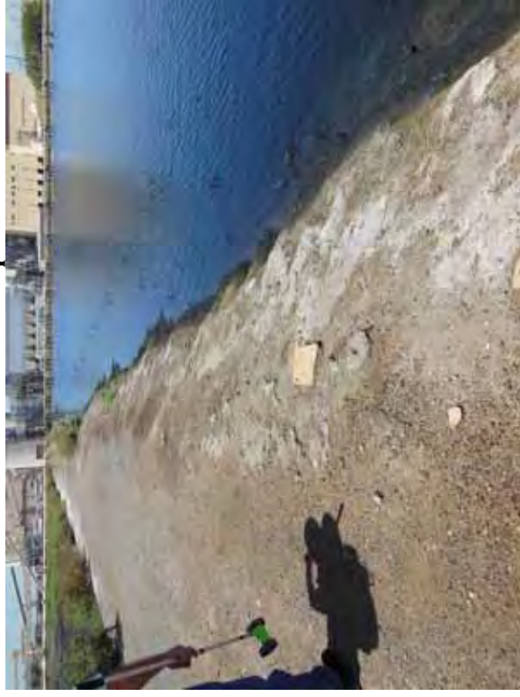
Photo 25: NP/SP - Vegetation and ash material on common embankment south slope.
