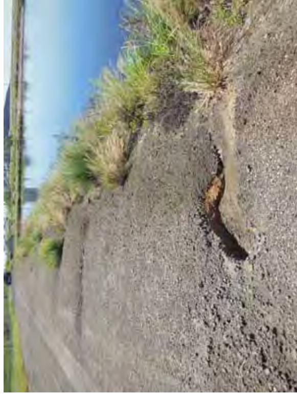
Photo 17: NP - East embankment interior slope, looking south. Note erosion rills in ash material.
