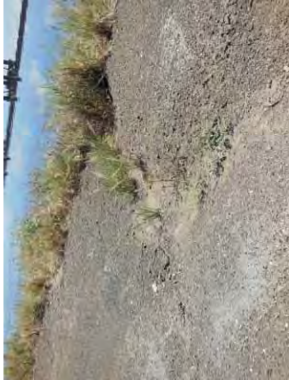
Photo 38: NP - Erosion rill in ash material at west embankment interior slope.
