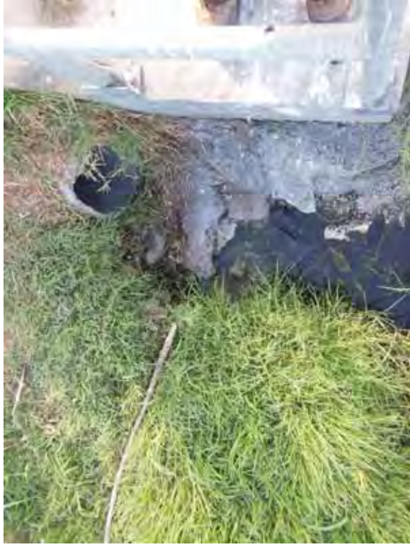
Photo 89: SP – 12-inch-diameter piping at outfall 103B.
