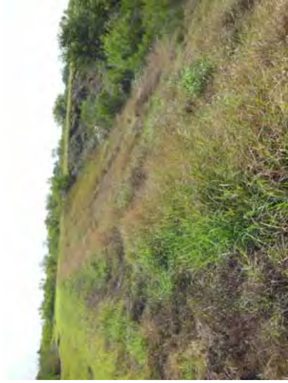
Photo 121: South embankment exterior slope, looking east.
