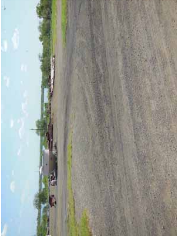
Photo 17: NP - East embankment interior slope, looking south. Note erosion rills in ash material.
