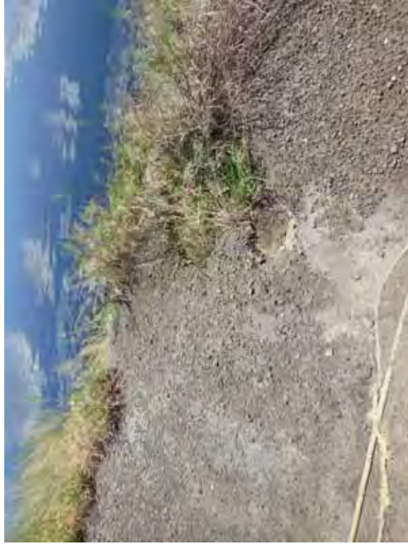
Photo 41: NP - West embankment exterior slope, looking north. Note area of loose soil/ash material.
