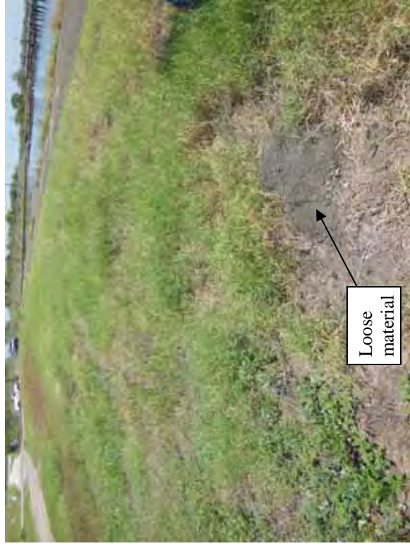
Photo 41: NP - West embankment exterior slope, looking north. Note area of loose soil/ash material.
