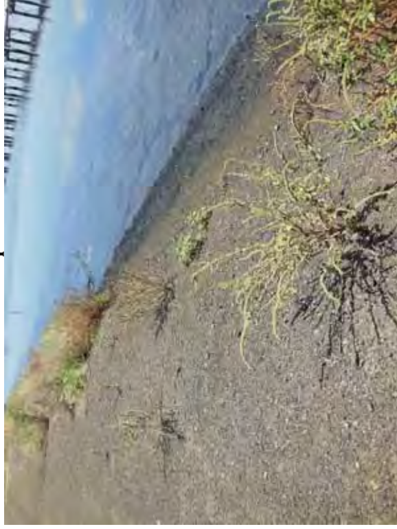
Photo 38: NP - Erosion rill in ash material at west embankment interior slope.
