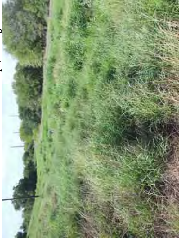
Photo 109: West embankment exterior slope, looking southwest.
