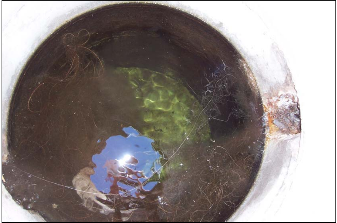
Photo 15: View inside left toe drain manhole. Note standing water and roots within manhole. Toe drain collection pipe flowing at right.
