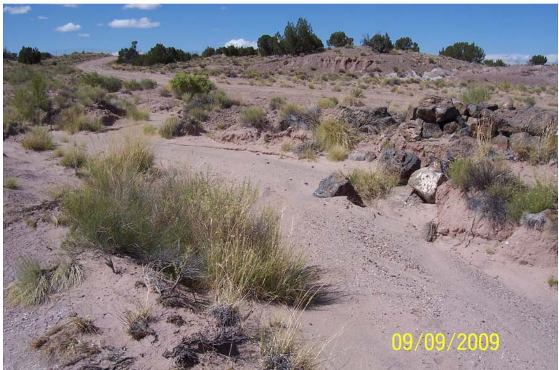
Photo 26: View of erosion channel along left upstream abutment groin. Note undercutting and displacement of riprap slope at right.
