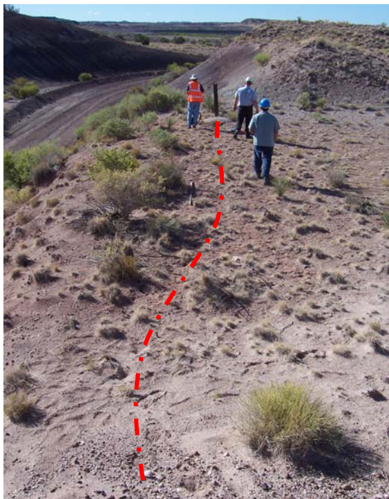
Photo 38: Overview of top of slope area where surface crack was observed. Approximate alignment of surface crack shown with dashed line.
