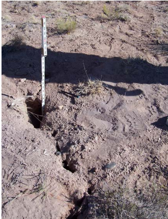
Photo 37: Detail view of surface crack near top of left slope of emergency spillway channel. Note ruler inserted approximately 30 inches into crack.
