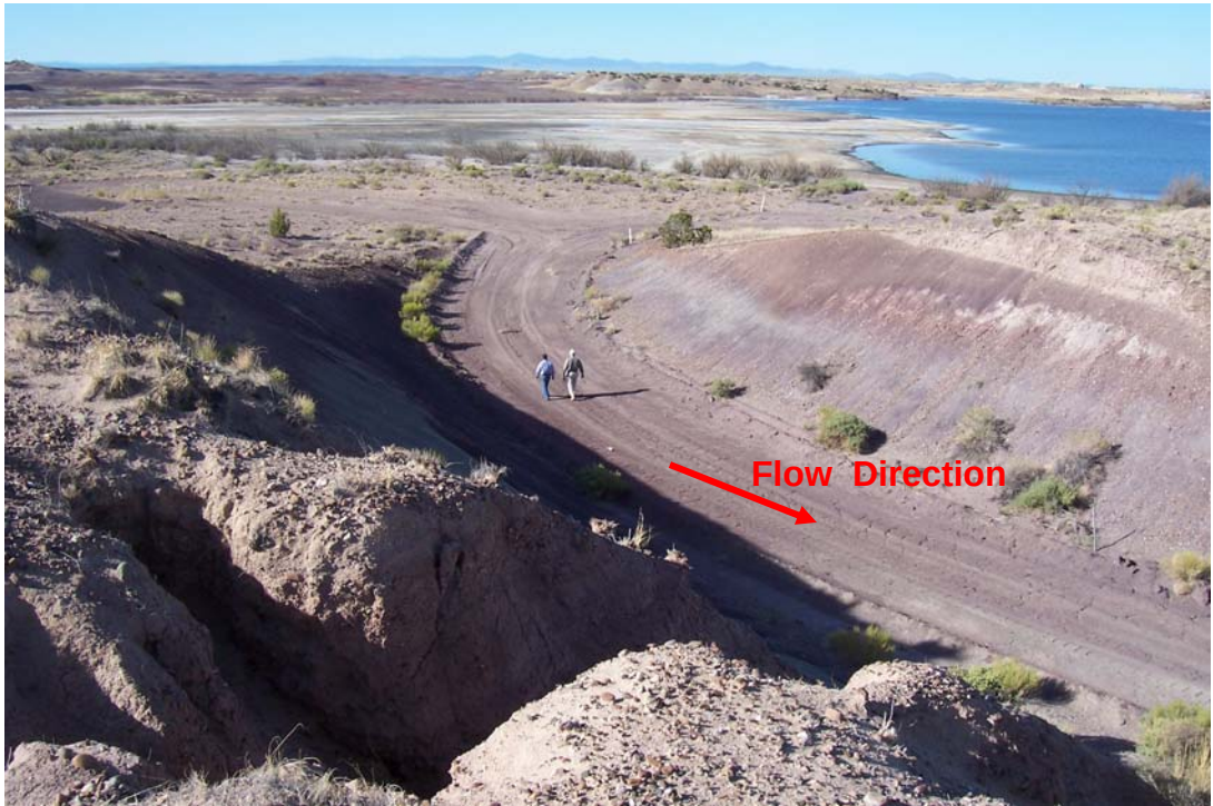
Photo 29: View of emergency spillway approach channel and pond from top of right channel slope. Note slope erosion in foreground.
