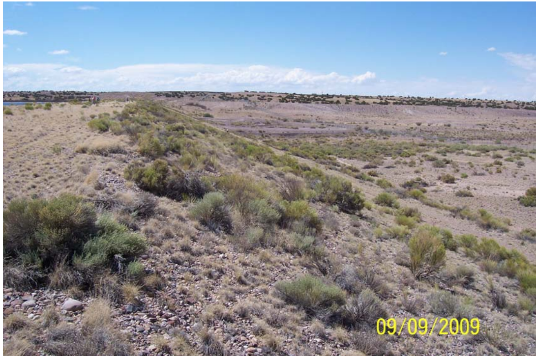
Photo 5: View along downstream slope of dam from right side of dam. Note gravel surface, and grass and brush vegetative cover.
