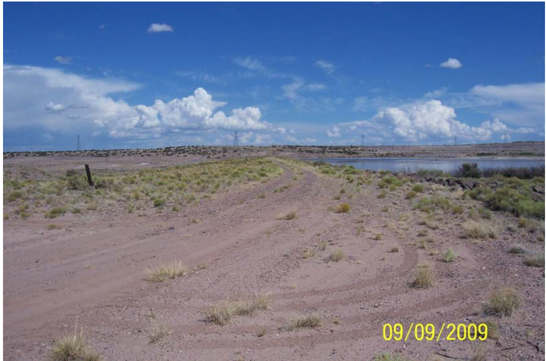
Photo 25: View along top of dam from left abutment. Note minor rutting from vehicle traffic.
