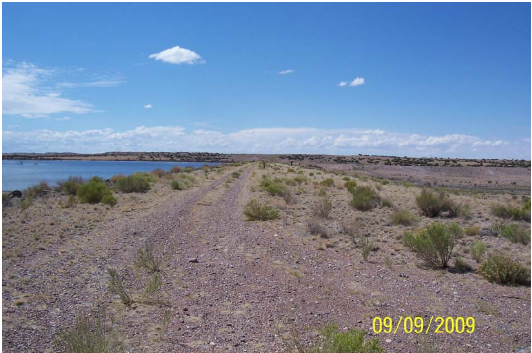
Photo 4: View along top of dam from right abutment area. Note grass and brush vegetative cover and minor rutting from vehicular traffic.
