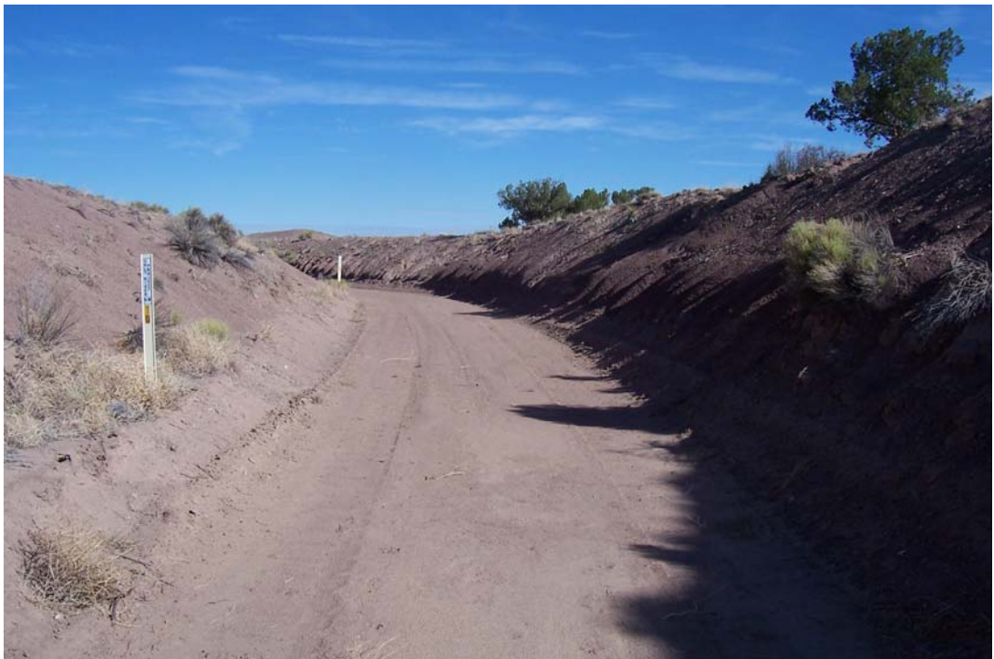
Photo 32: View within emergency spillway channel, looking downstream towards discharge area. Note recent grading of spillway channel bottom.
