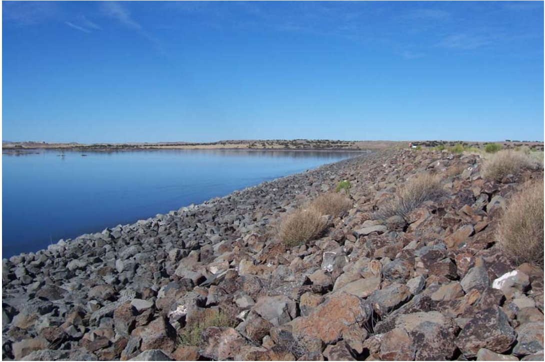
Photo 3: View along upstream riprap slope from right side of dam. Note upstream berm and lower portion of upstream slope submerged by Pond.
