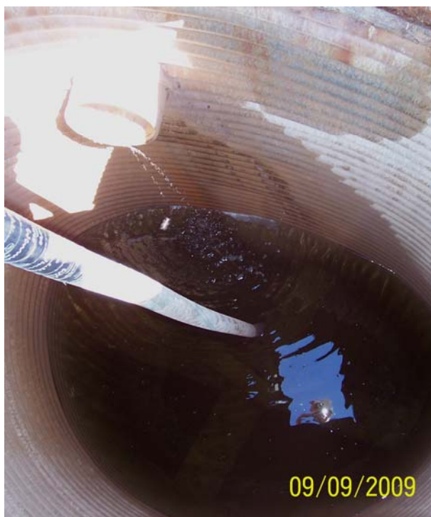
Photo 18: View inside left toe drain sump. Note seepage discharge from inlet pipe, and hanging pipe for pumping collected seepage back to Pond.
