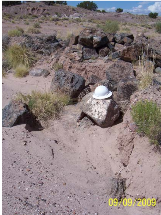
Photo 27: View of undercutting and displacement of riprap at left abutment contact. Hard hat shown for scale.
