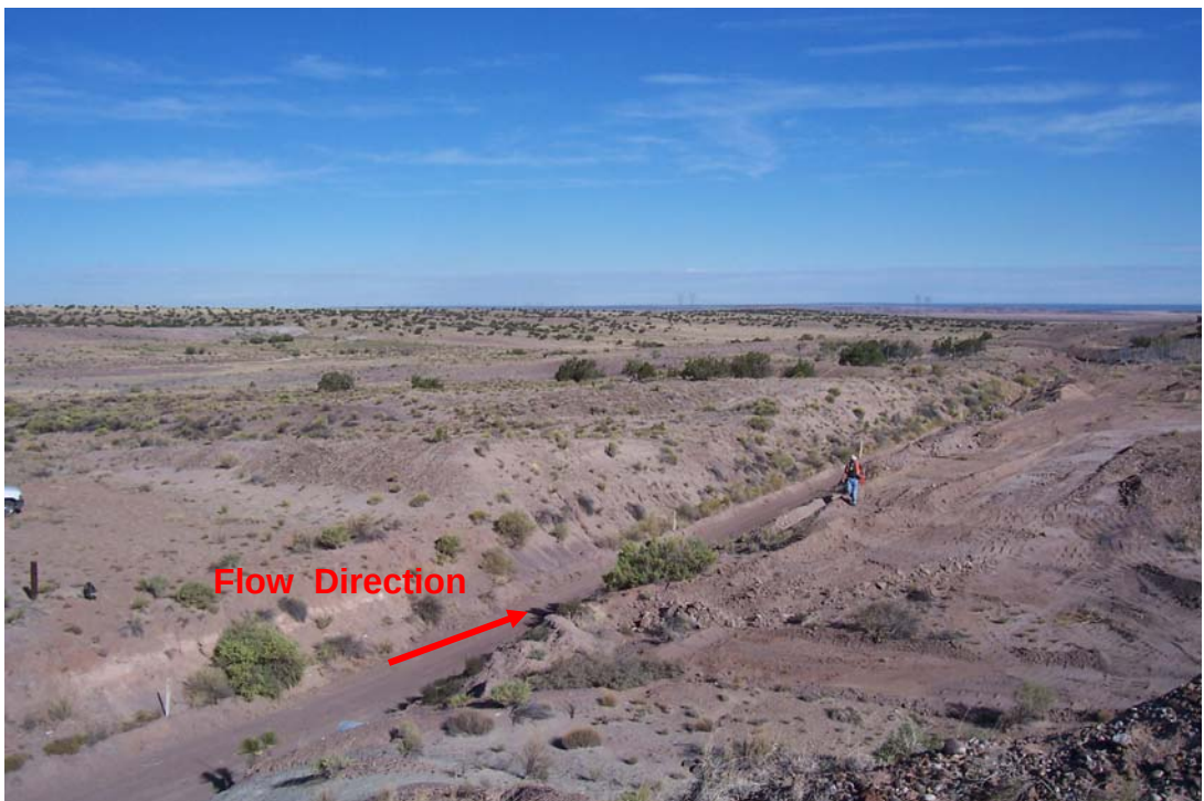
Photo 30: Overview of emergency spillway channel from top of right channel slope. Channel invert in foreground, discharge area in background.
