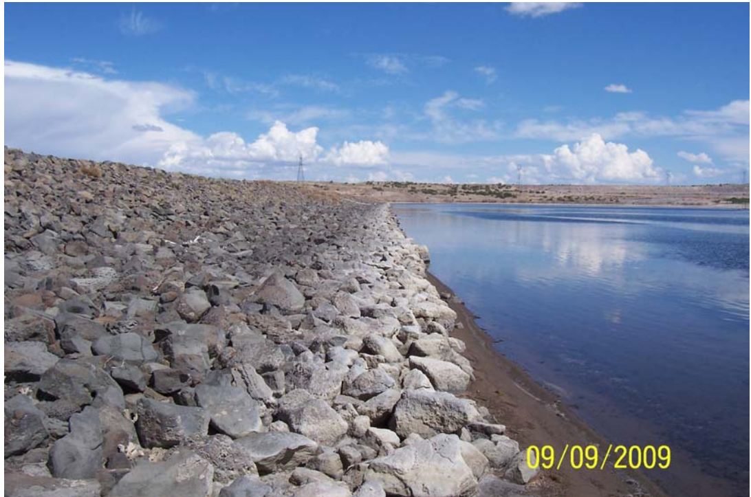
Photo 23: View along upstream slope of dam from left side. Note upstream berm partially visible above water line.
