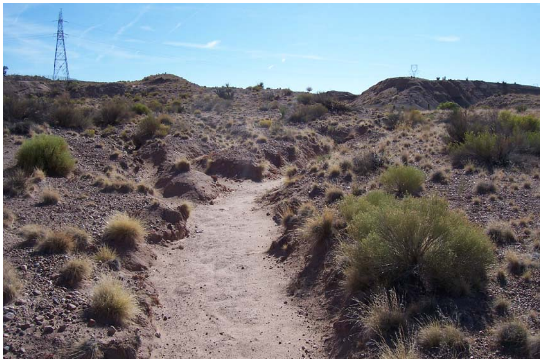
Photo 28: View of erosion channel along right downstream abutment contact.
