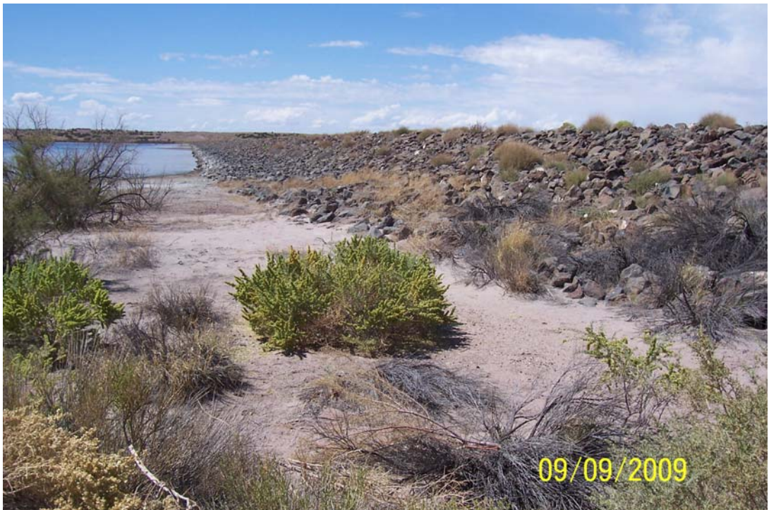
Photo 2: Overview of upstream slope of dam from right abutment contact. Note moderate brush growth on riprap slope.
