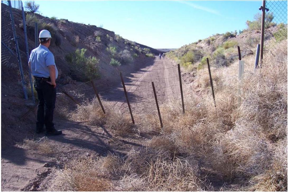
Photo 31: View within emergency spillway channel looking upstream from break-away cattle gate. Note accumulation of tumbleweeds.
