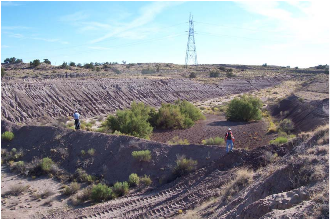
Photo 34: View of excavated area at right abutment, with earthen berm constructed to prevent stormwater runoff from eroding spillway slopes.
