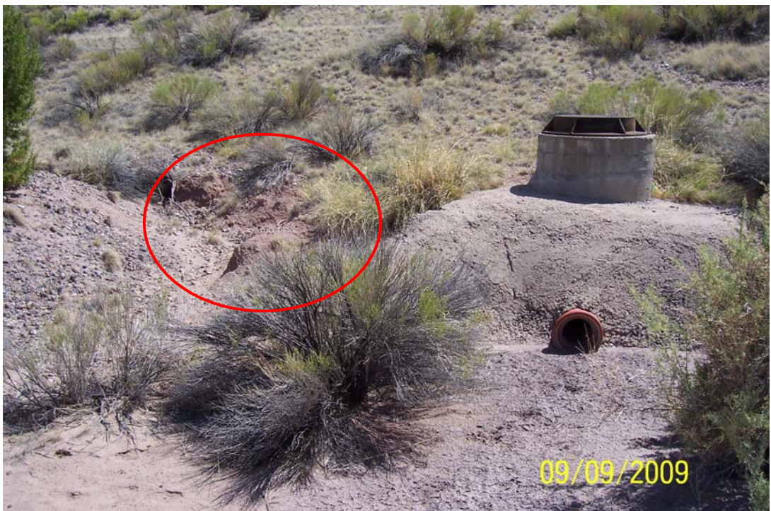
Photo 10: View of right toe drain manhole from downstream dry channel. Note minor erosion adjacent to concrete cover (circled).
