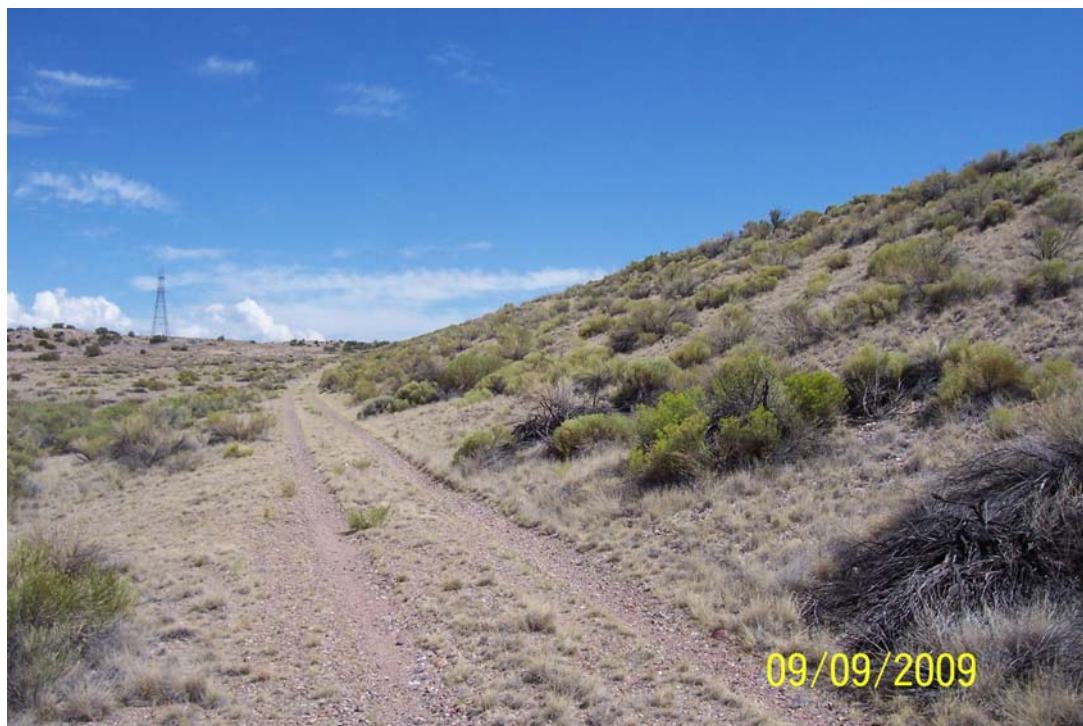
Photo 7: View along downstream slope of dam looking towards right abutment, taken from access road along downstream toe. Note minor rutting of access road.
