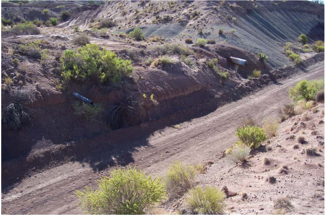
Photo 35: View of emergency spillway near channel control section. Note eroded channel slope. Surface crack observed at top of left slope (see following photos).
