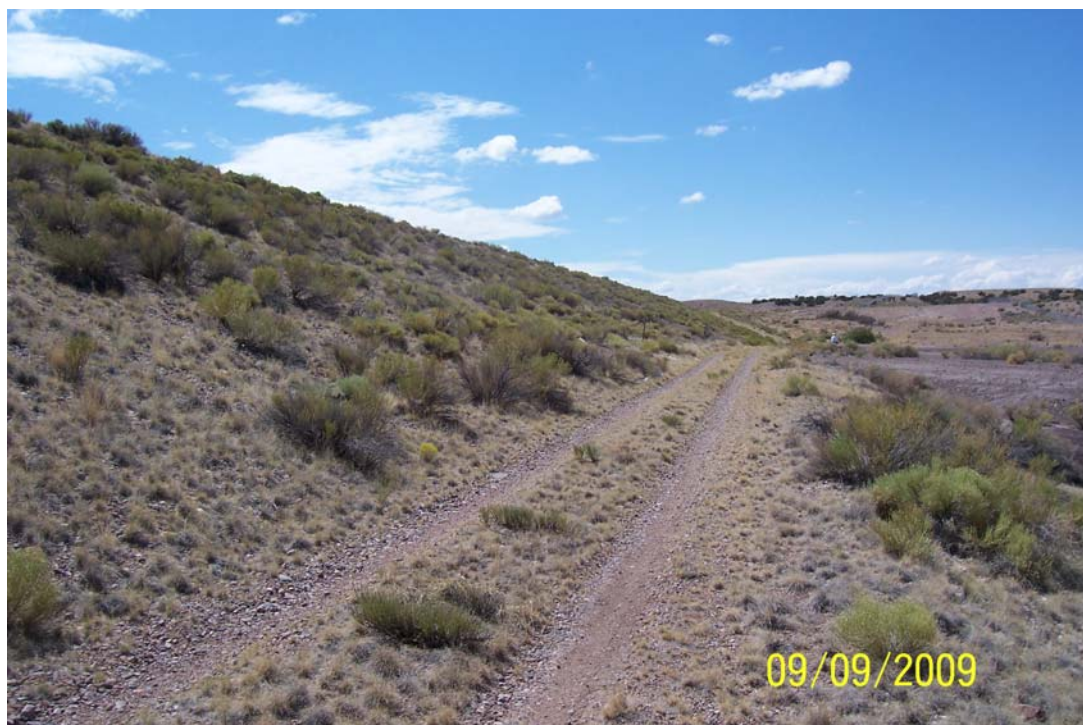
Photo 8: View along downstream slope of dam looking towards left abutment, taken from access road along downstream toe. Note minor rutting of access road
