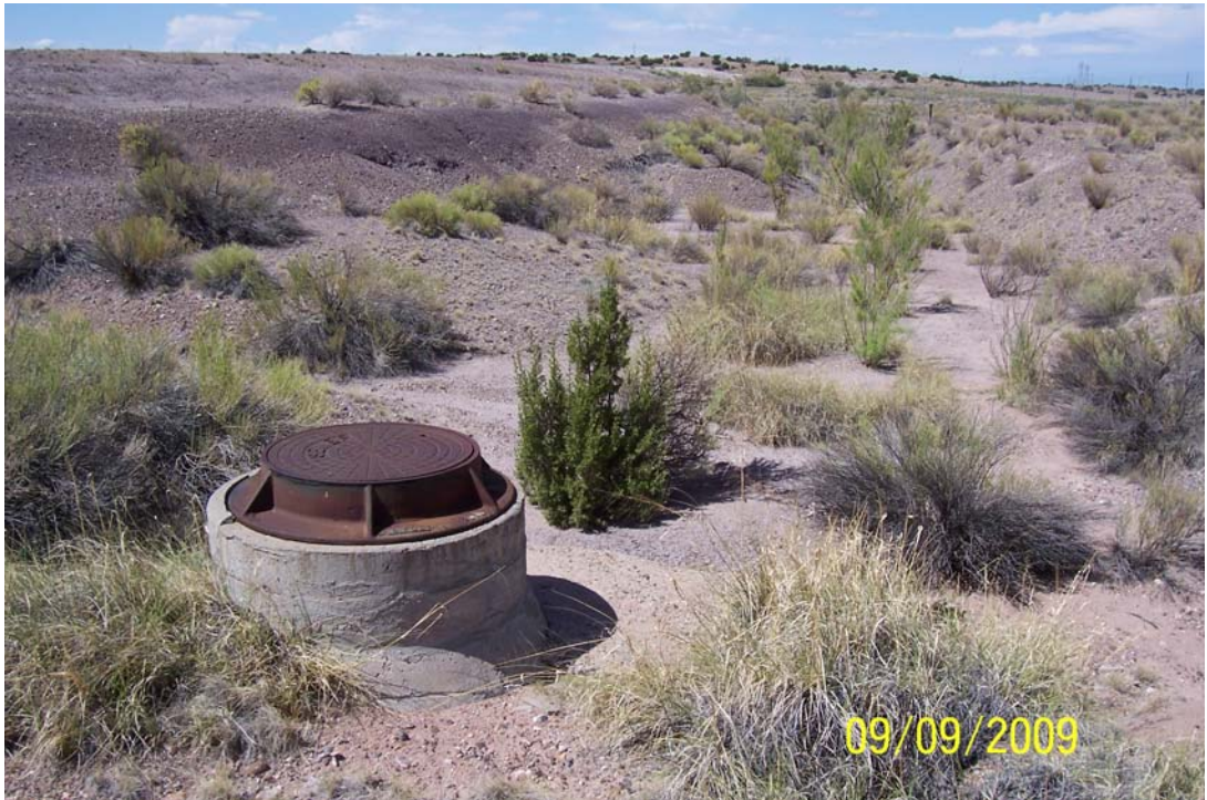
Photo 9: View of right toe drain manhole at downstream toe of dam. Note dry discharge channel surrounded by secondary containment berms
