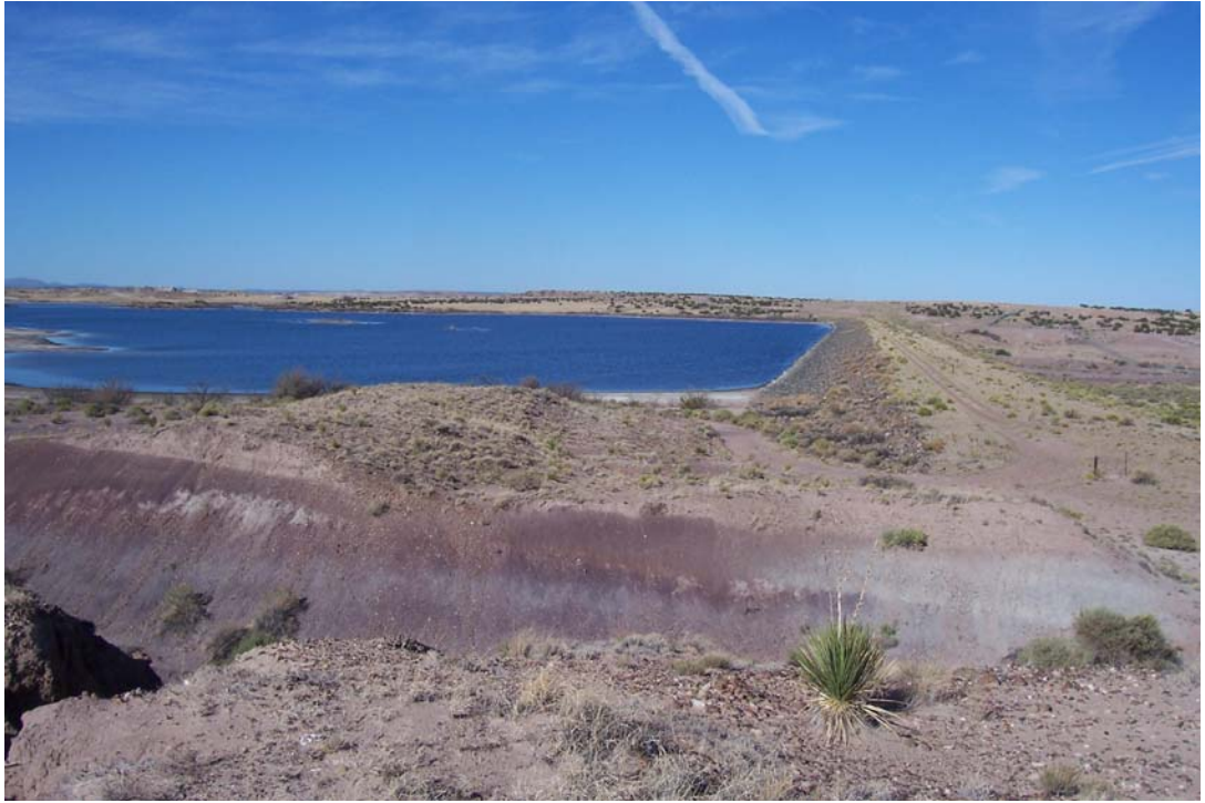
Photo 1: Overview of Evaporation Pond and Dam from right abutment. Note emergency spillway cut in foreground.
