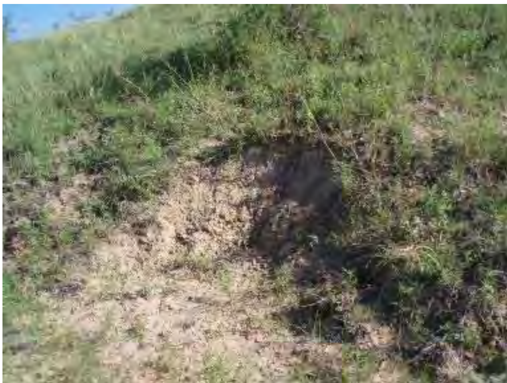
Photo No. 34: Secondary Pond - North embankment exterior slope, looking at 8'Lx4'Wx2'D erosion rill.
