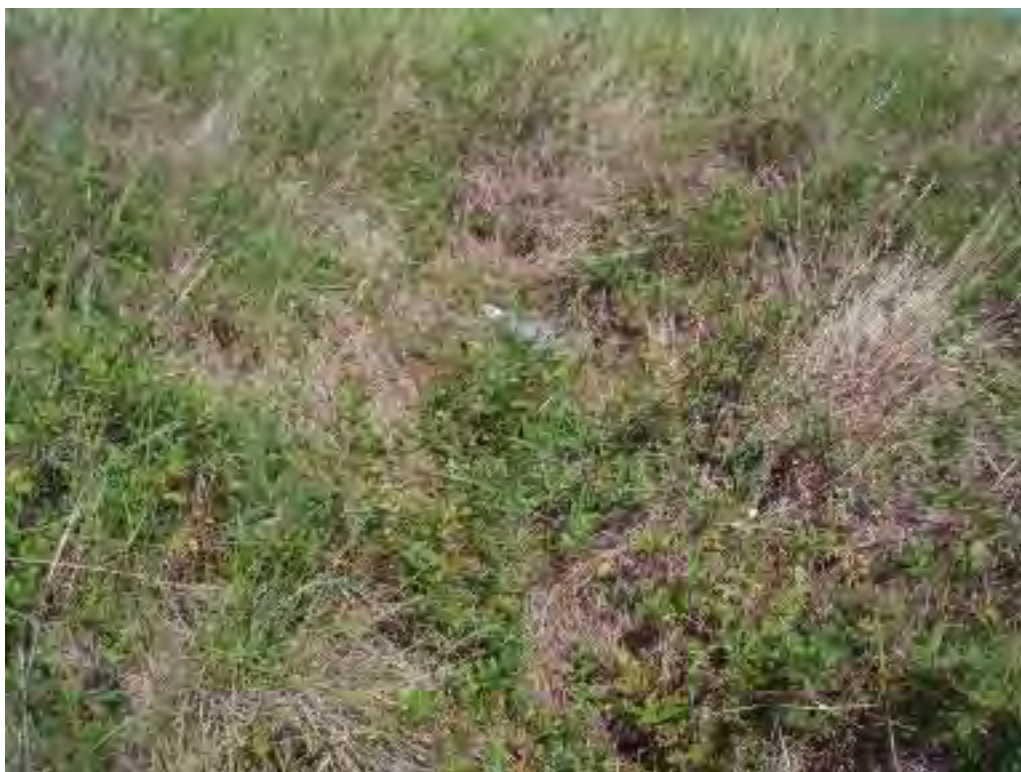
Photo No. 106: Primary Ash Pond - East embankment exterior slope, looking at 4'Wx4'Lx2'D depression. Note apparent dried seepage areas in the vicinity.
