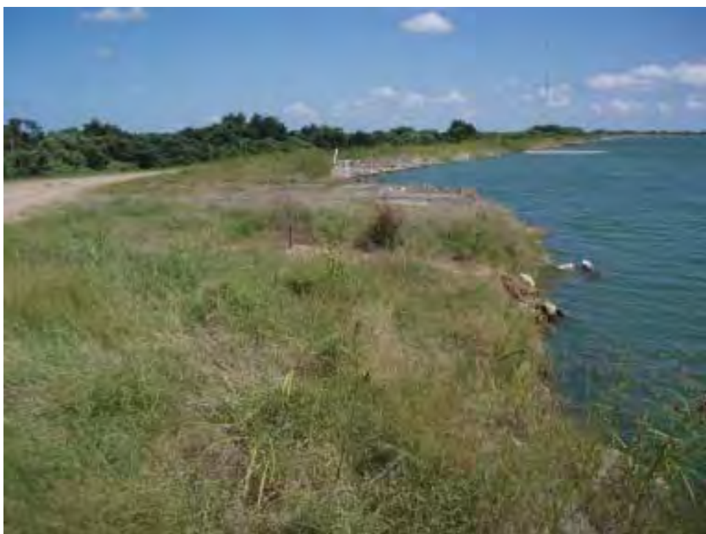
Photo No. 12: Primary Ash Pond - East interior slope, looking southeast. Note areas where Boral trucks have dumped excess material on the interior slope.
