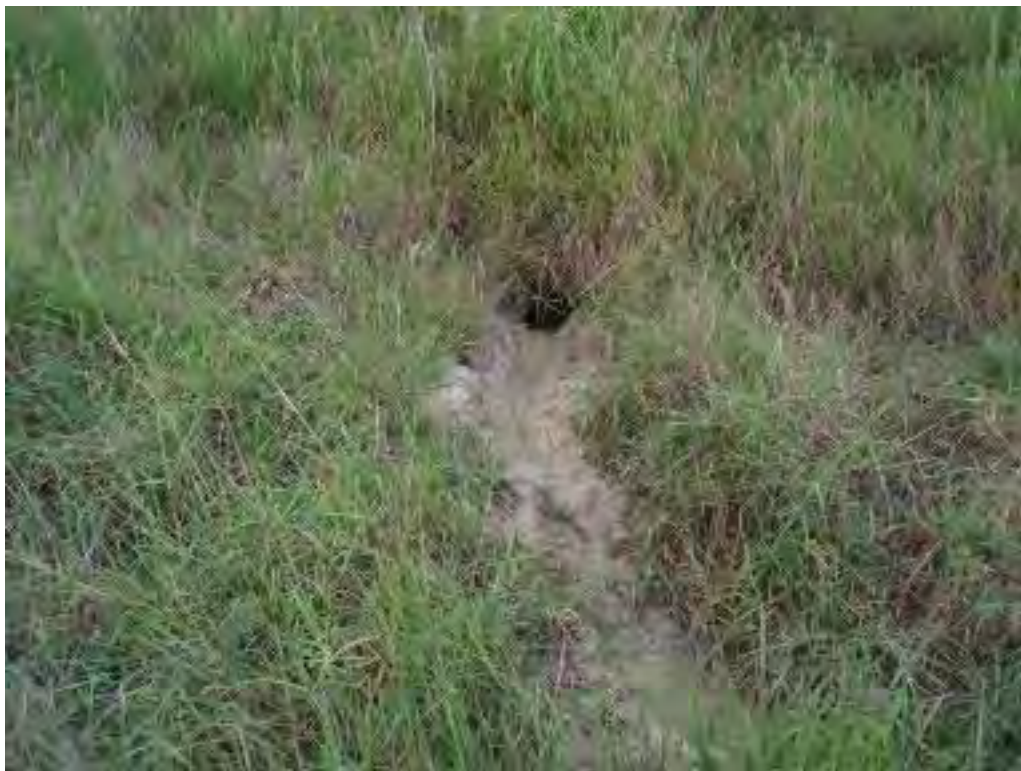
Photo No. 97: Primary Ash Pond – Southeast embankment exterior slope, looking at 8-inch-diameter rodent burrow hole and seep.
