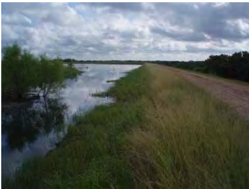
Photo No. 94: Primary Ash Pond - Southeast embankment interior slope, looking northeast.
