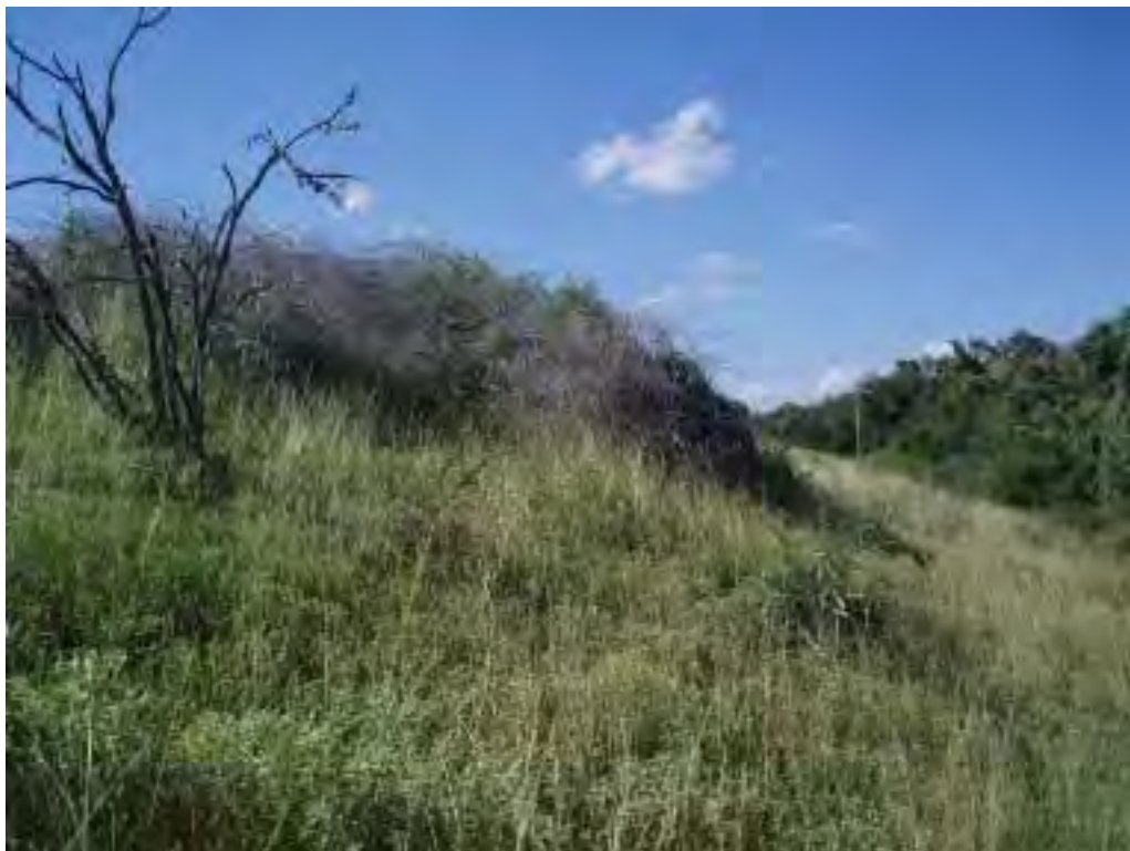
Photo No. 29: Secondary Pond - East embankment exterior slope, looking north at thick brush and dead trees.
