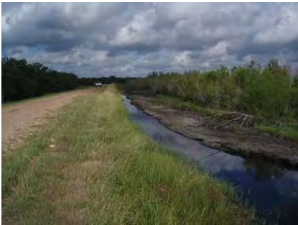
Photo No. 93: Primary Ash Pond - South embankment interior slope, looking west.
