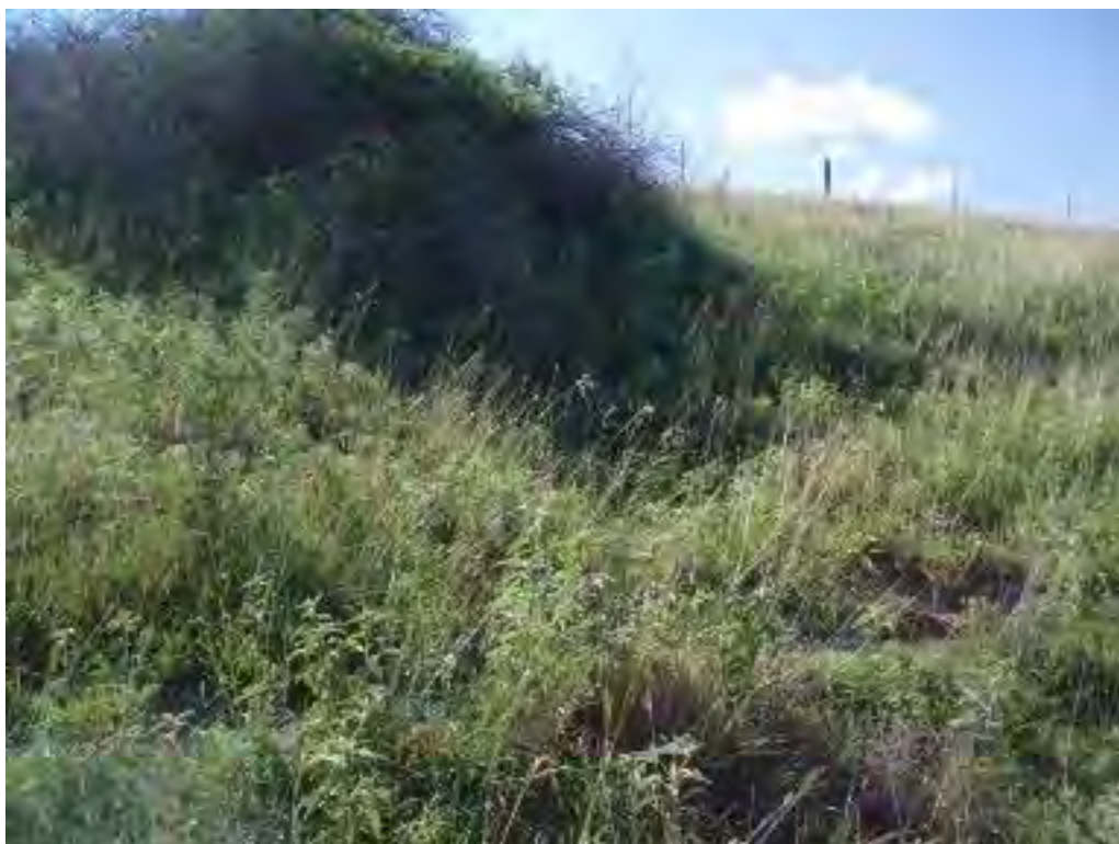
Photo No. 30: Secondary Pond - East embankment exterior slope, looking at 8'Lx8'Wx2'D depression.
