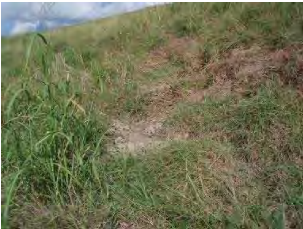
Photo No. 98: Primary Ash Pond – Southeast embankment exterior slope, looking at 8'Lx2'W seep near toe.
