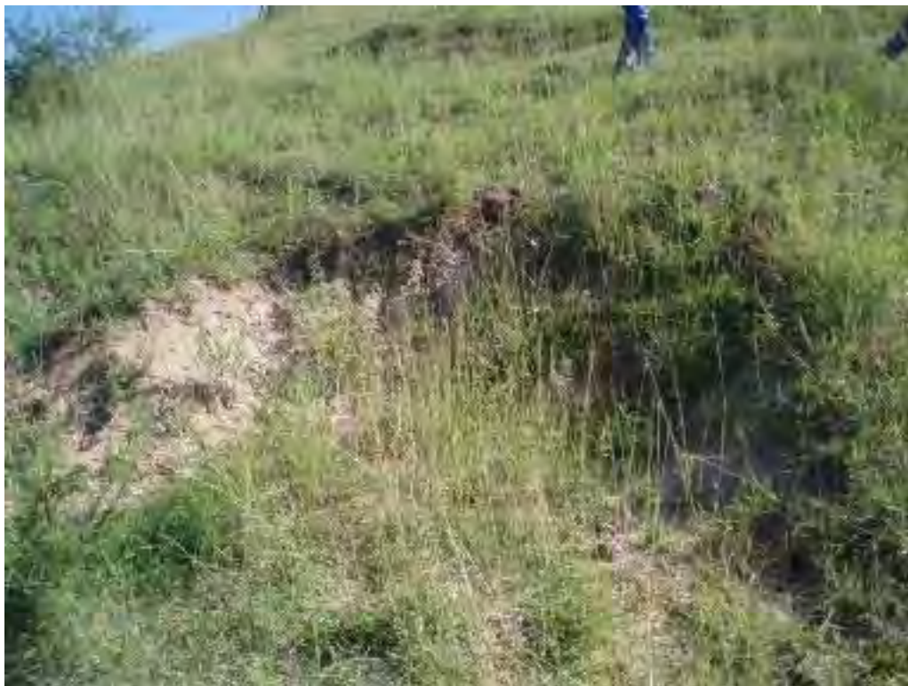
Photo No. 33: Secondary Pond - North embankment exterior slope, looking at 10'Lx4'Wx3'D erosion rill. Note the brush in background.
