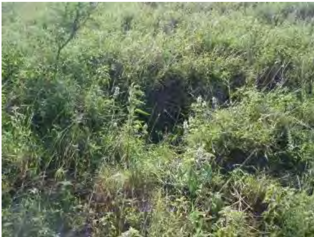
Photo No. 31: Secondary Pond - East embankment exterior slope, looking at 6'Lx4'Wx3'D depression.
