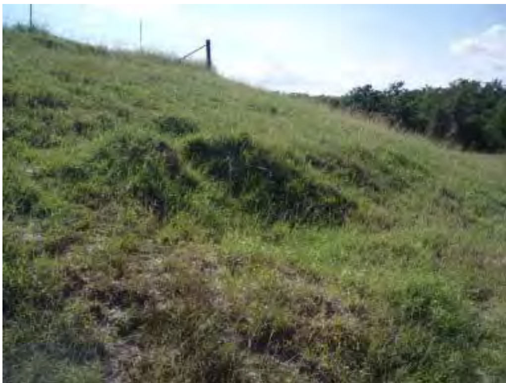
Photo No. 32: Secondary Pond - North embankment exterior slope, looking at 8'Lx8'Wx3'D depression.
