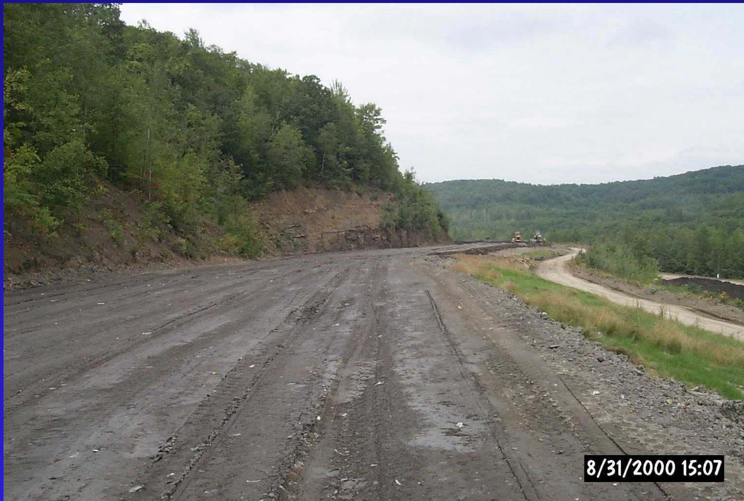
Material in place after spreading and roller compacting
