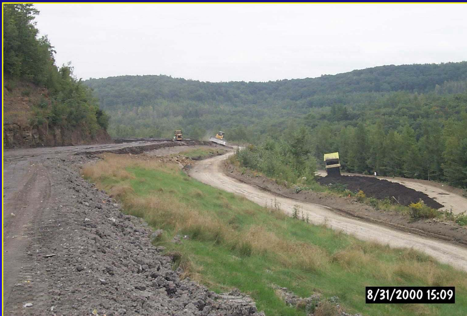
Mixed product is allowed to air dry for 2-3 days before it is spread and compacted as shown on lower bench (right side)
