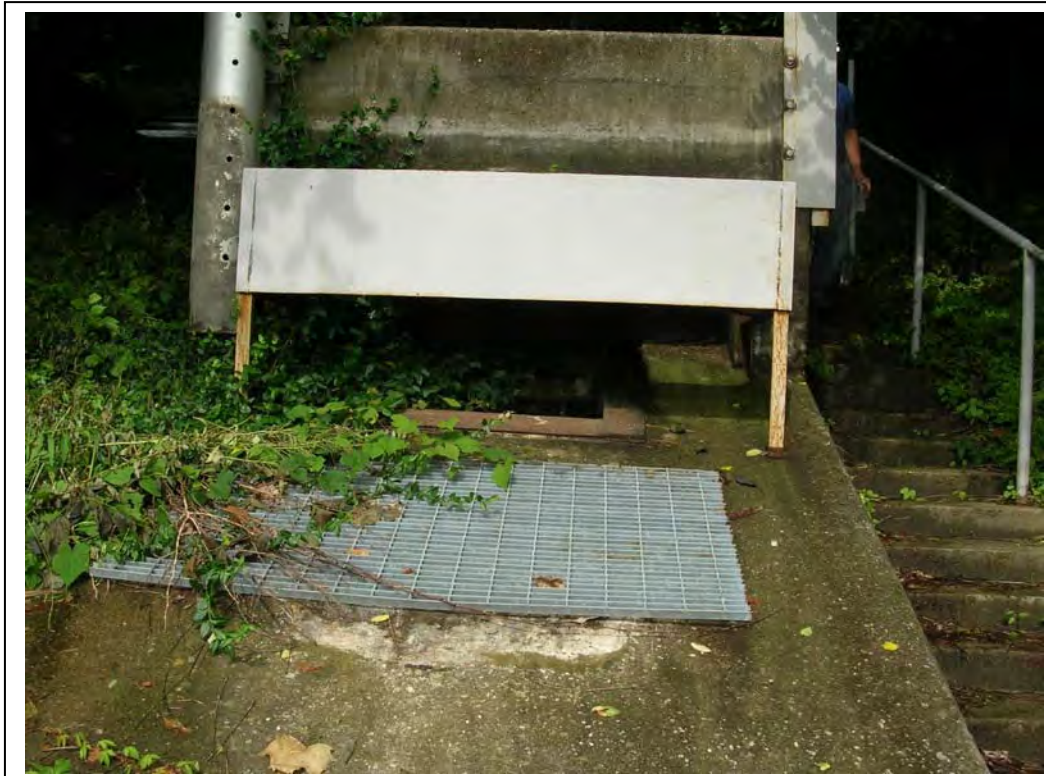
#21 – Minor Vegetative Growth Blocking Portion of Upper Intake (Vegetation Subsequently Removed)
