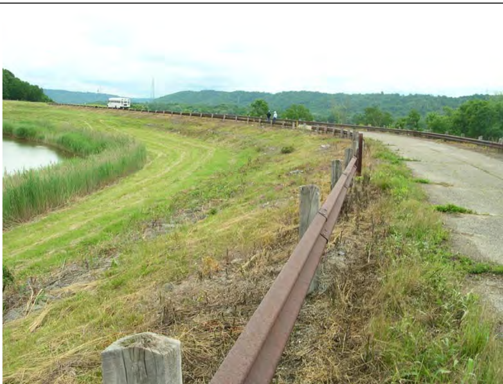
#2 – Upstream Face and Roadway at Crest with Wetland Growth at Pond Level
