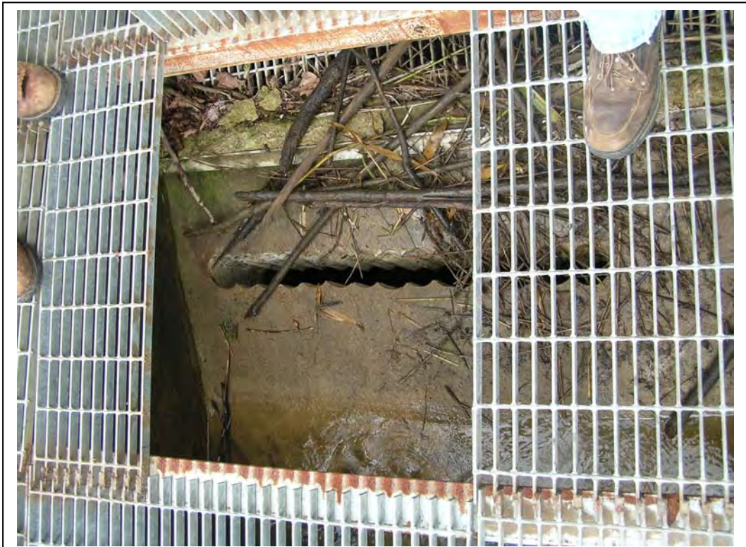
#19 – Mid-level Intake with Minor Woody Debris; Note Concrete Cores Creating Modified Intakes
