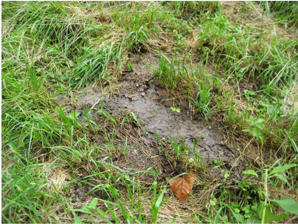
#11 – Soil Erosion Due to Surface Runoff at Toe Near Outlet Pipe Headwall
