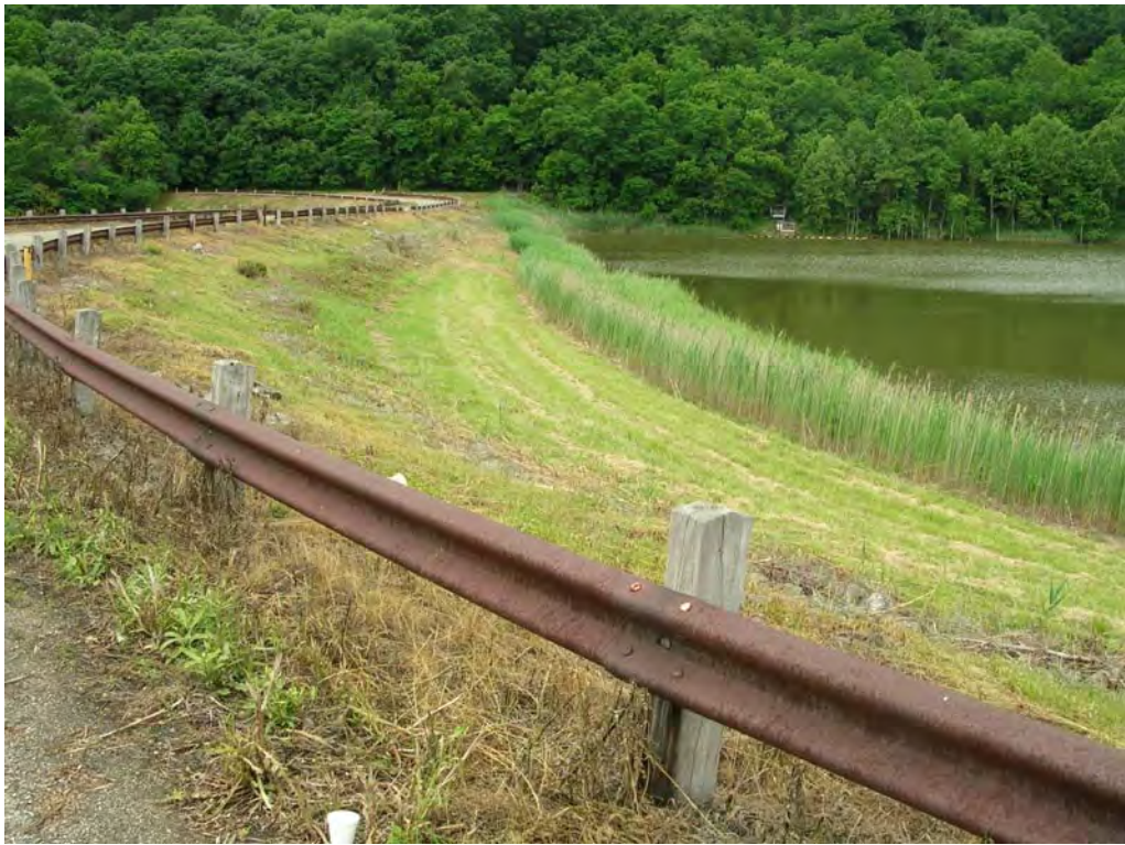
#3 – Central Portion of Upstream Face of Embankment Looking Toward Right Abutment
