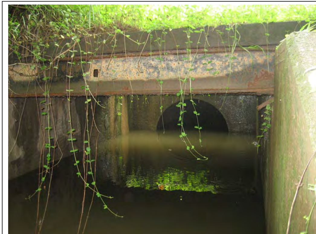
#22 – Outlet Headwall and Training Walls for 72-inch Discharge Pipe
