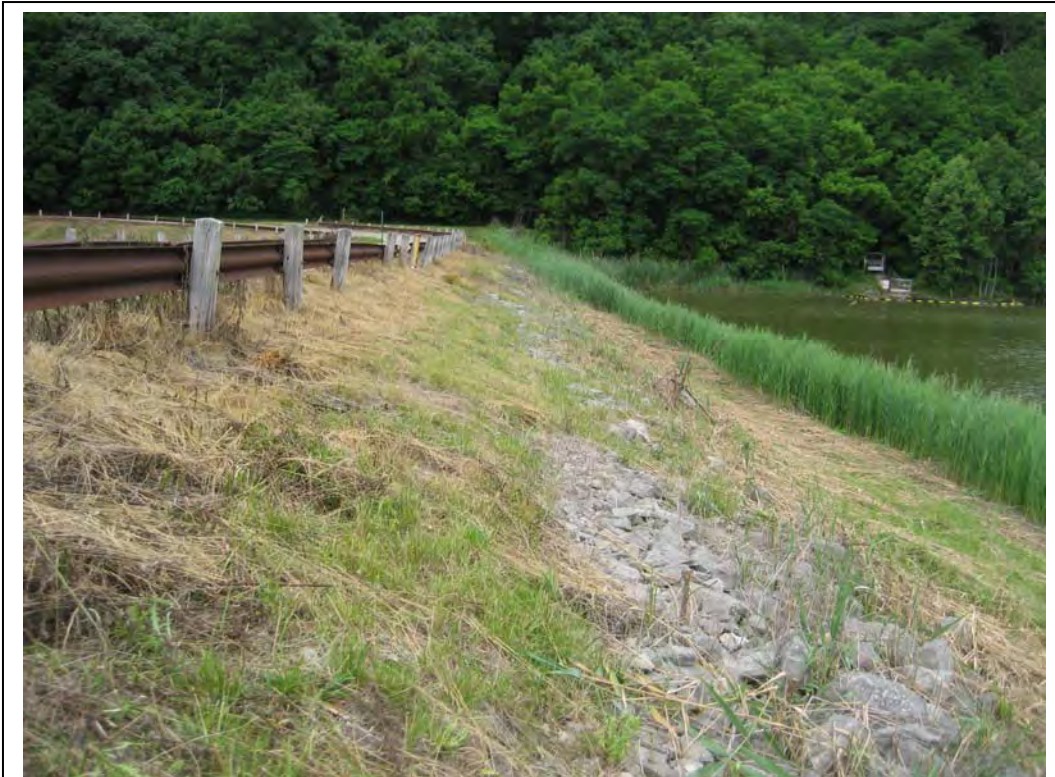
#5 – Upstream Slope; Note Riprap Protection
