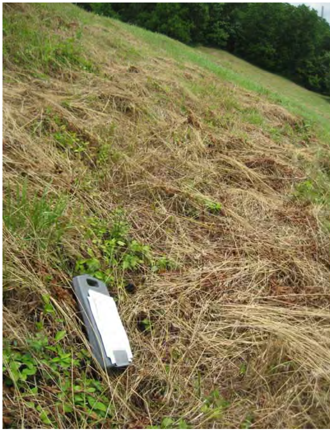
#17 – Typical Slope Scarp on Downstream Face on Saddle Dike
