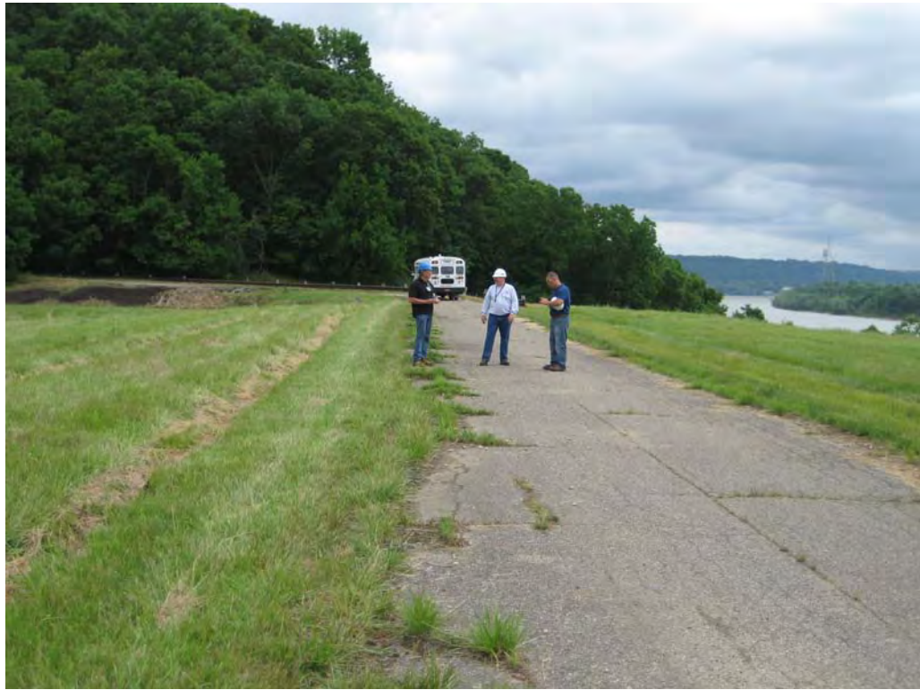
#7 – Paved Crest and Stability Berm (to left) Looking Toward Left Abutment
