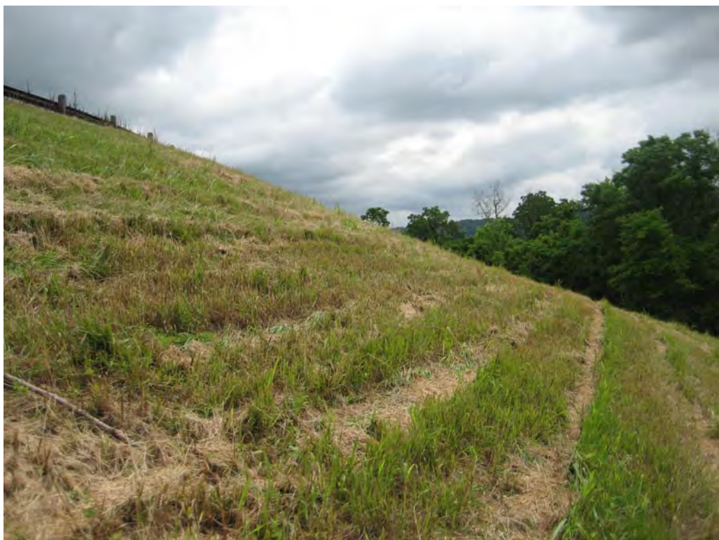
#12 – Typical Condition of Downstream Slope
