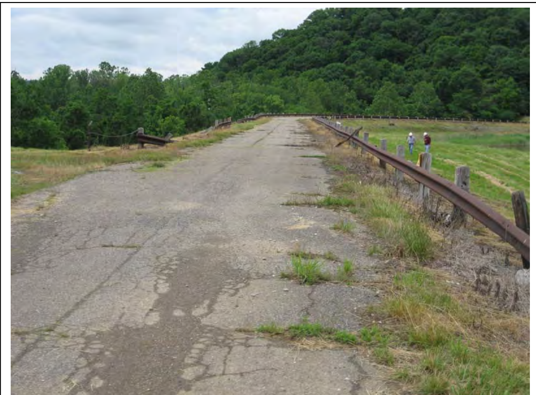
#6 – Paved Crest Looking Toward Right Abutment
