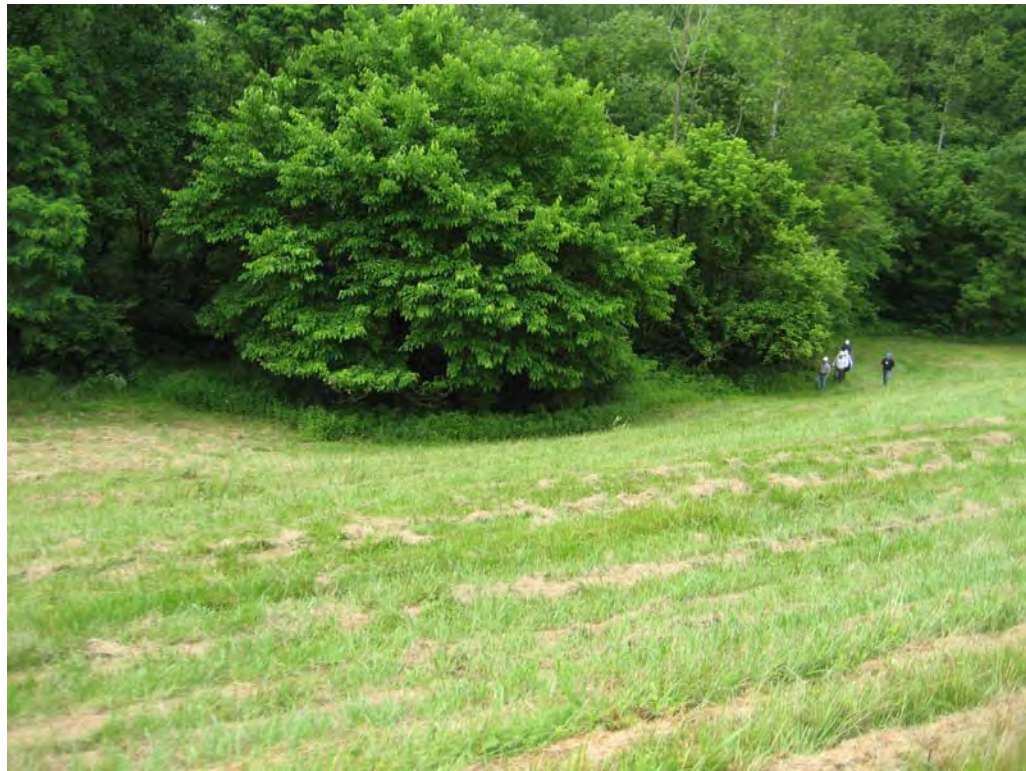
#13 – Downstream Face and Tree Growth Just Beyond Toe
