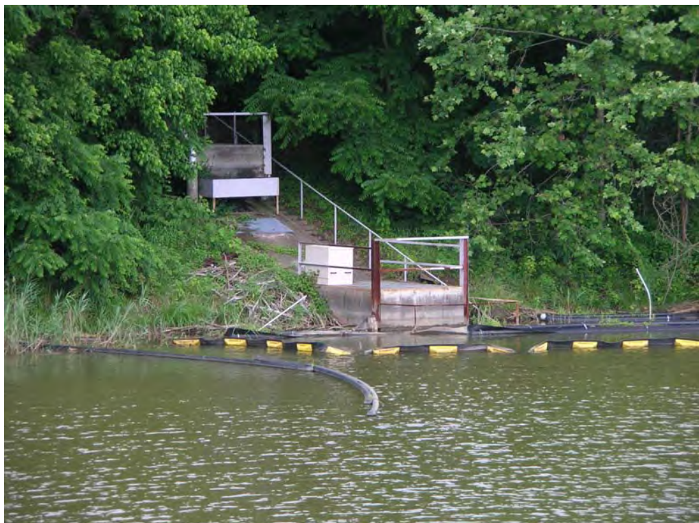
#18 – Sloped Decant Spillway Structure and Oil Skimmer
