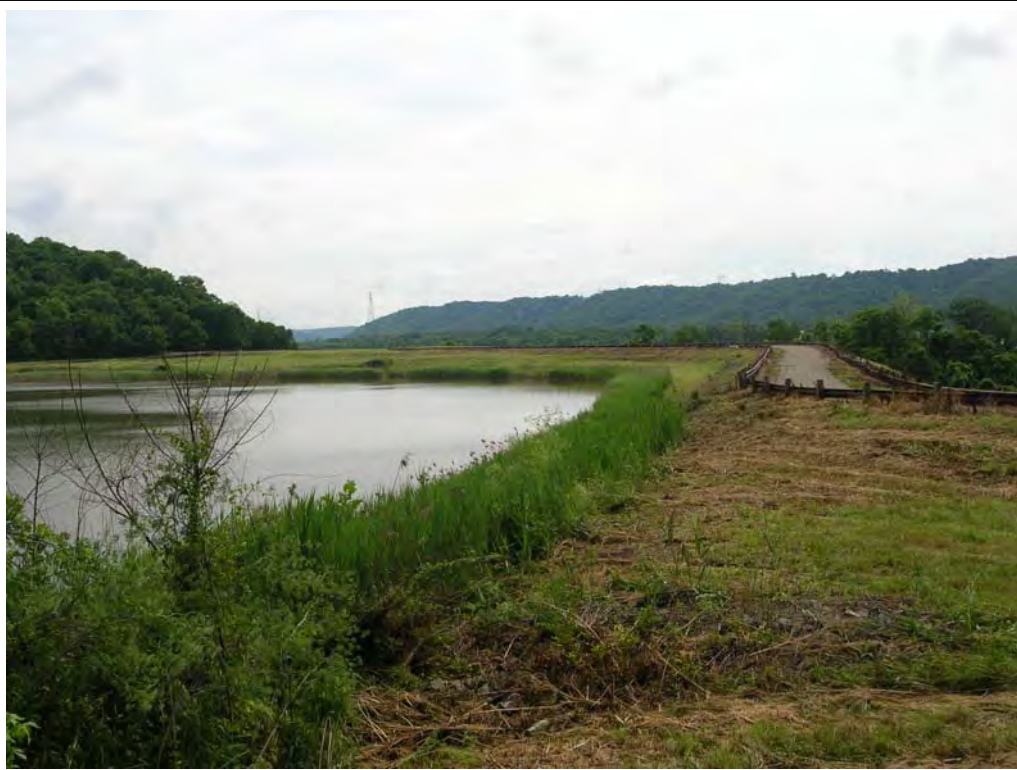
#1 – Pond and Upstream Face of Embankment as Viewed from Beyond Right Abutment
