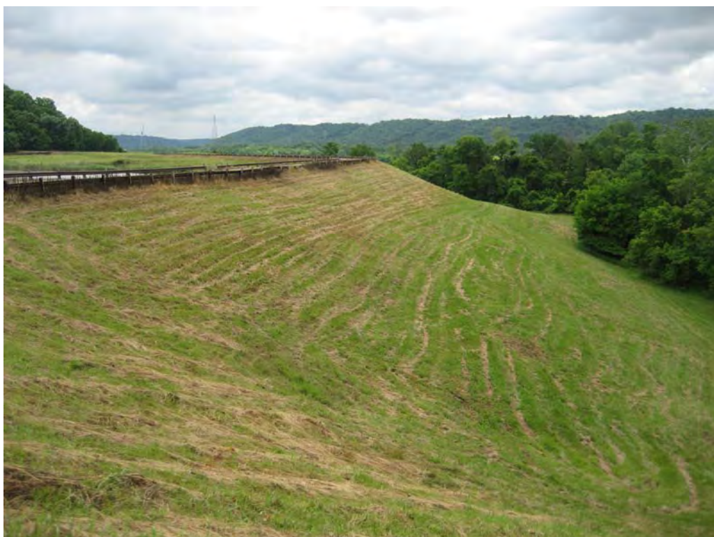
#8 – Downstream Slope Near Right Abutment Looking East
