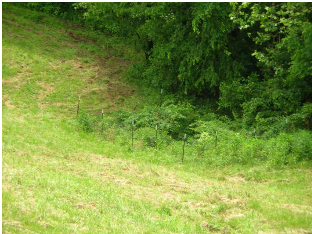
#14 – Looking Downgradient at Toe at 72" Pipe Outfall Location; Note Heavy Growth
