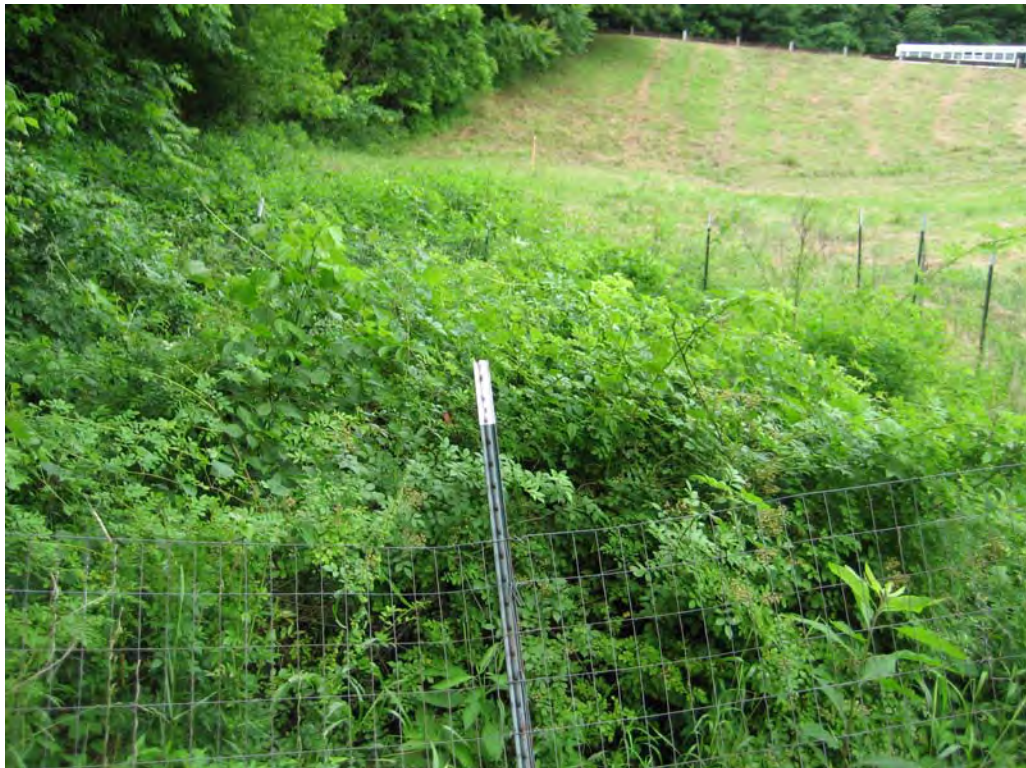
#10 – Downstream Slope Looking Up Toward Crest Near Right Groin. Overgrowth of Vegetation Near Outfall in Foreground of Picture.
