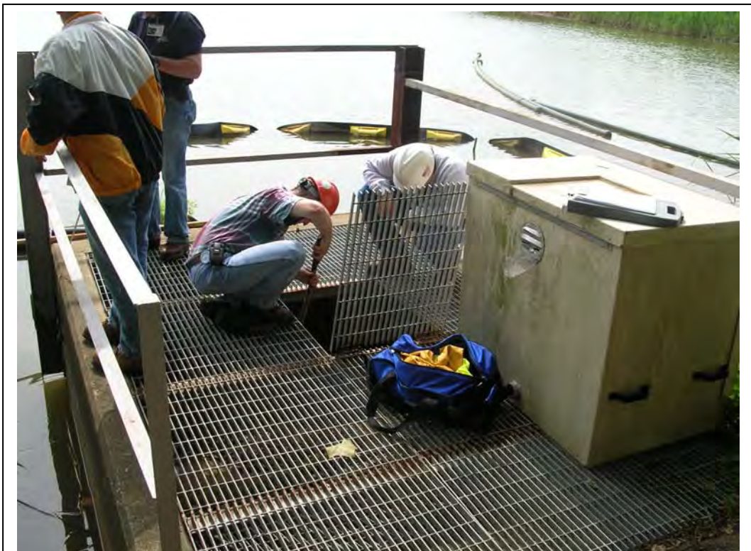
#20 – Spillway Intake Looking Toward Pond
