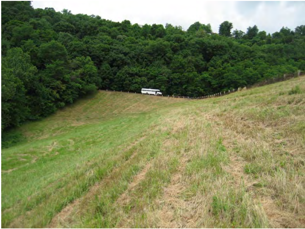
#9 – Downstream Slope Looking Toward Right Abutment; Outlet Pipe Outfall Just Beyond Left of Frame.
