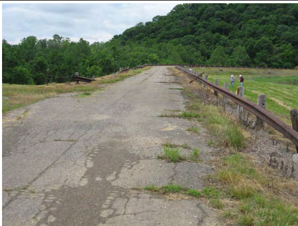
#6 – Paved Crest Looking Toward Right Abutment
