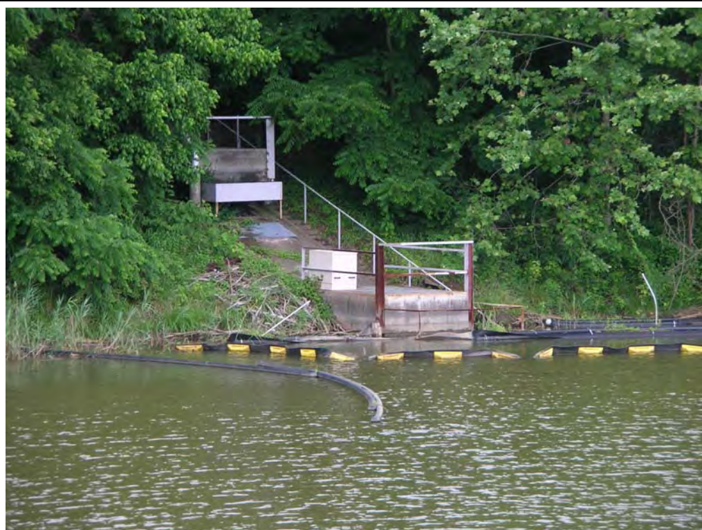
#18 – Sloped Decant Spillway Structure and Debris Boom
