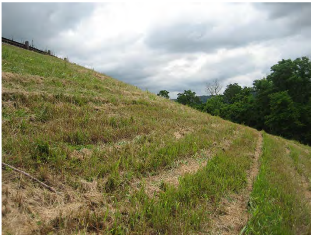
#12 – Typical Condition of Downstream Slope
