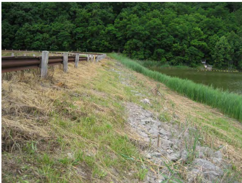
#5 – Upstream Slope; Note Riprap Protection
