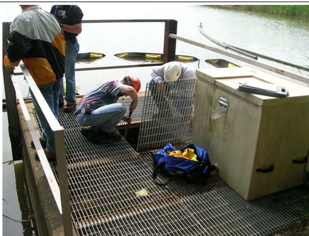
#20 – Spillway Intake Looking Toward Pond
