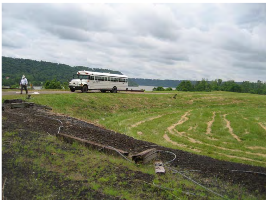
# 4 – Stability Berm on Upstream Face Near Left Abutment
