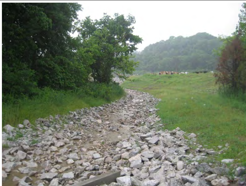
#2 - Relocated Runoff Drain Entering Pond
