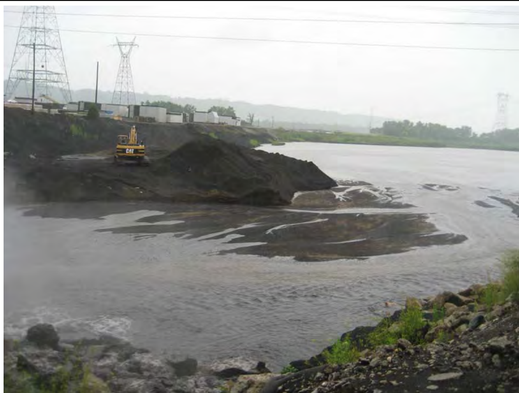
#1 - Overview of Bottom Ash Pond taken from head water area looking southwest
