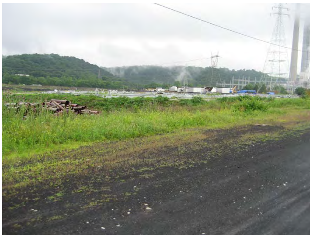
#15 - Crest and Upstream Face at Left Abutment
