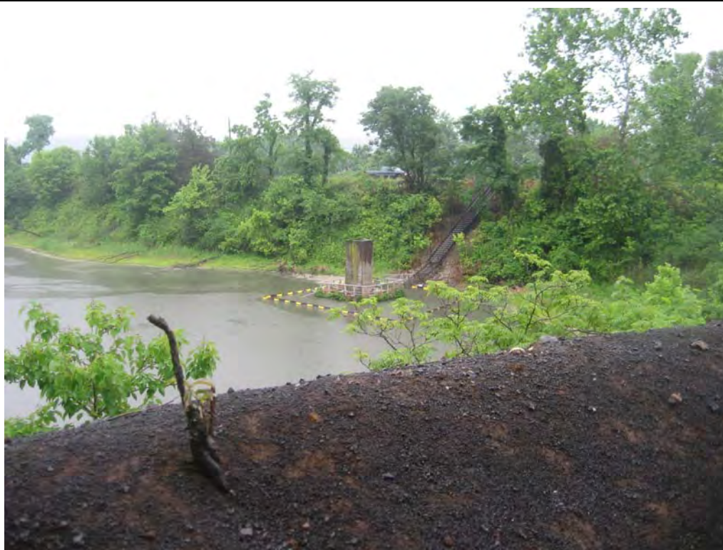
# 4 - Decant Spillway and Portion of Upstream Face of Dam Embankment; (note dense tree growth)
