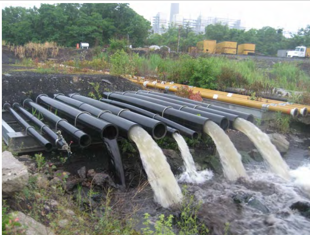
#3 - Boiler Room Sumps and Sluice Discharge Lines Into Pond
