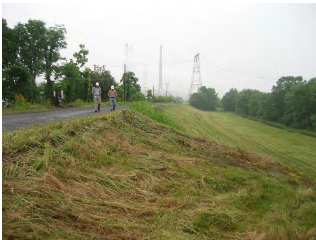
#6 - Upper Slope and Berm of Downstream Face Taken Near Right Abutment
