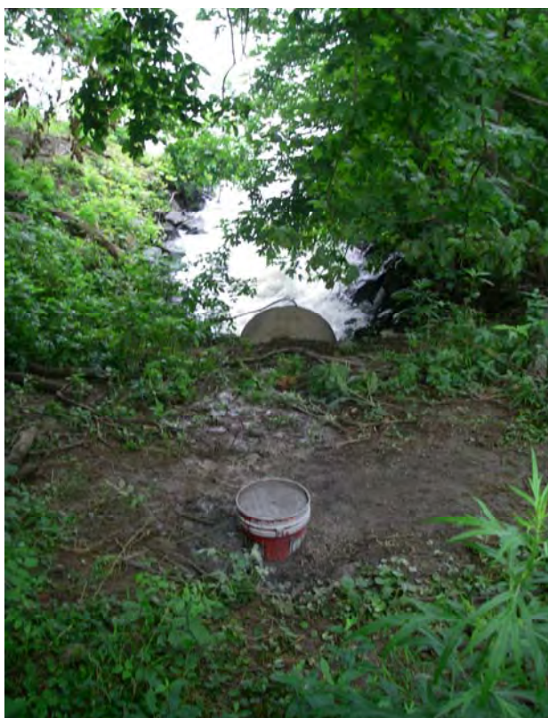
#8 - Repaired Sinkhole & RCP Outlet to Ohio River
