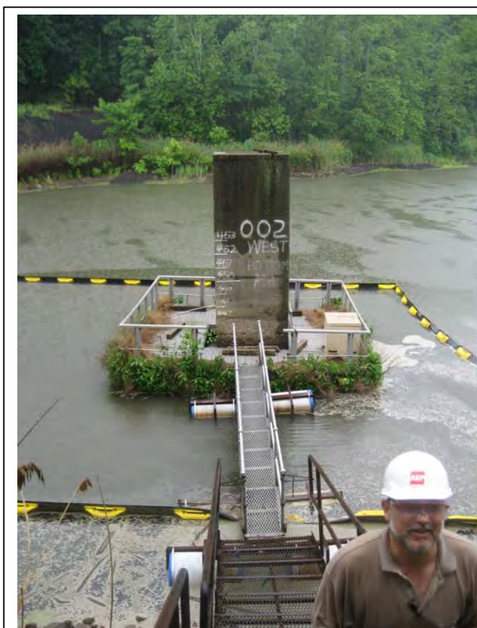
#9 - Decant Spillway in Floating Catwalk/Spillway and debris boom
