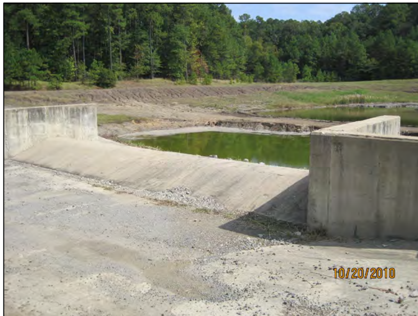
67 LANDFILL RUNOFF POND-LOOKING EAST AT EMERGENCY SPILLWAY
