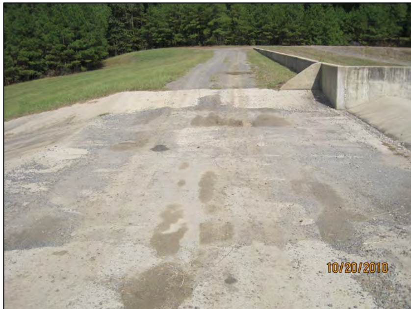
66 LANDFILL RUNOFF POND-LOOKING NORTHEAST ACROSS EMERGENCY SPILLWAY
