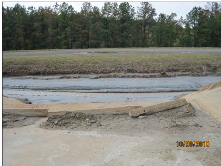
42 AUXILIARY SURGE POND-DISCHARGE SPILLWAY
