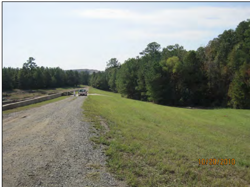
62 LANDFILL RUNOFF POND-LOOKING SOUTHWEST ALONG DOWNSTREAM EMBANKMENT
