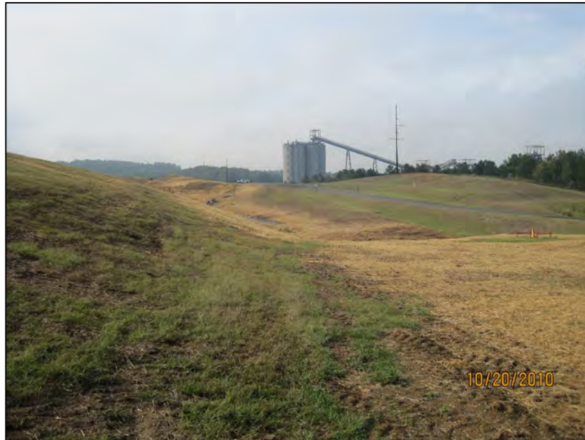
ASH POND 2-LOOKING SOUTHWEST AT RESEEDING ALONG DOWNSTREAM EMBANKMENT FACE
