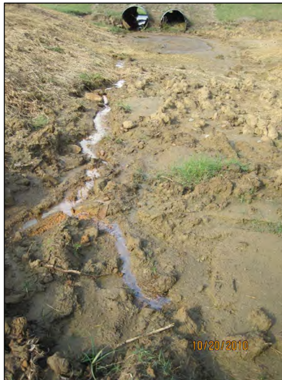
ASH POND 2-APPARENT SEEPAGE UPSTREAM OF STORMWATER CULVERTS, RIGHT (NORTH) CULVERT HALF FILLED WITH SEDIMENT
