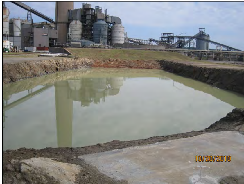
41 AUXILIARY SURGE POND-INFLUENT PIPE
