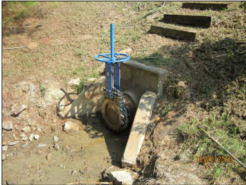
LANDFILL RUNOFF POND-VALVE CONTROL AT DISCHARGE
