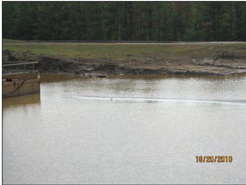
SURGE POND 1-MOSTLY SUBMERGED INFLUENT CULVERT
