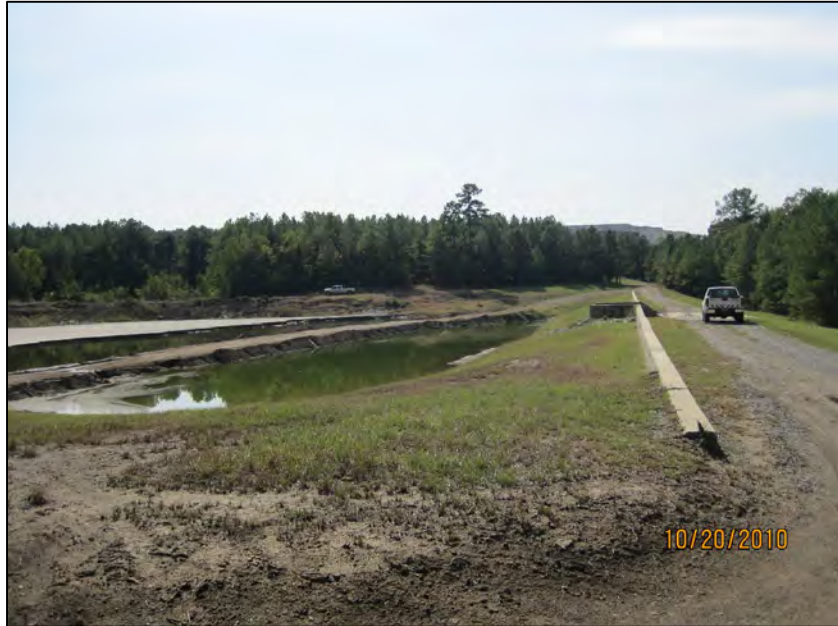
61 LANDFILL RUNOFF POND-LOOKING SOUTHWEST ALONG EMBANKMENT CREST
