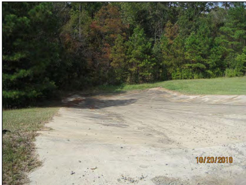
68 LANDFILL RUNOFF POND-DOWNSTREAM PORTION OF EMERGENCY SPILLWAY
