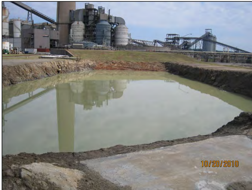
41 AUXILIARY SURGE POND-INFLUENT PIPE
