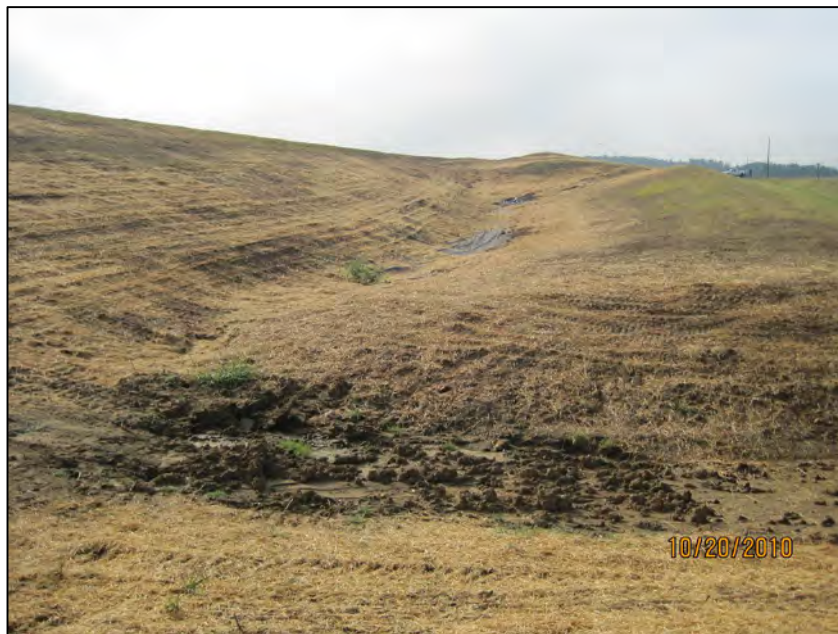
32 ASH POND 2-LOOKING SOUTH ALONG RESEED EMBANKMENT FACE
