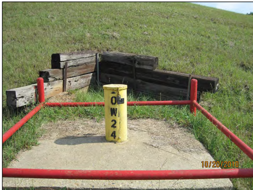
SURGE POND 2-MONITORING WELL 24 LOCATED AT SOUTHWEST CORNER
