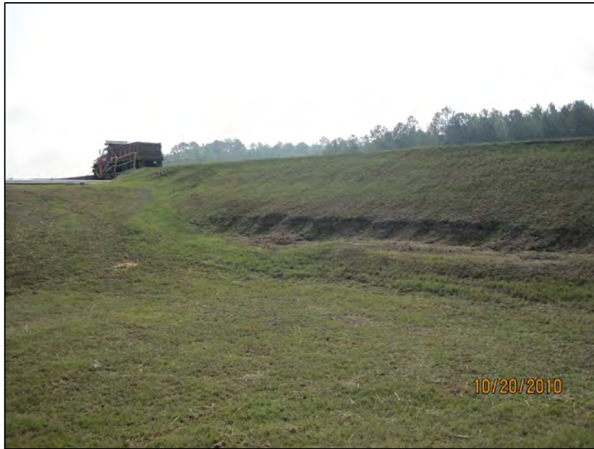
ASH POND 1-LOOKING SOUTHEAST AT EROSION ON SIDE OF ROADWAY LEADING TO ASH POND 1 EMBANKMENT CREST
