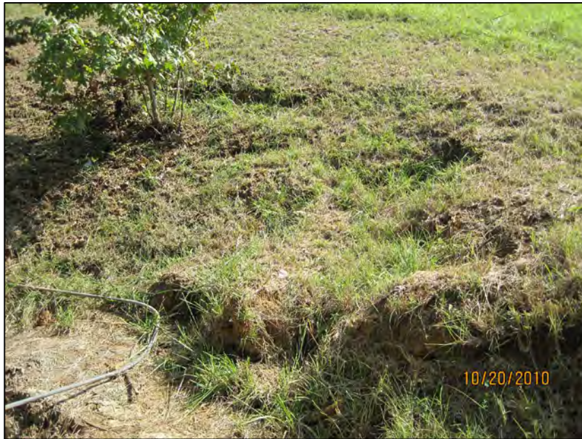
LANDFILL RUNOFF POND-SLUMP ADJACENT TO POND DISCHARGE VALVE
