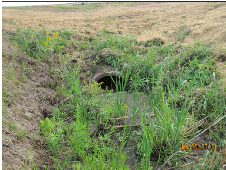
38 ASH POND 2-LOOKING UPSTREAM (EAST) AT ROADWAY EMBANKMENT STORM DRAIN
