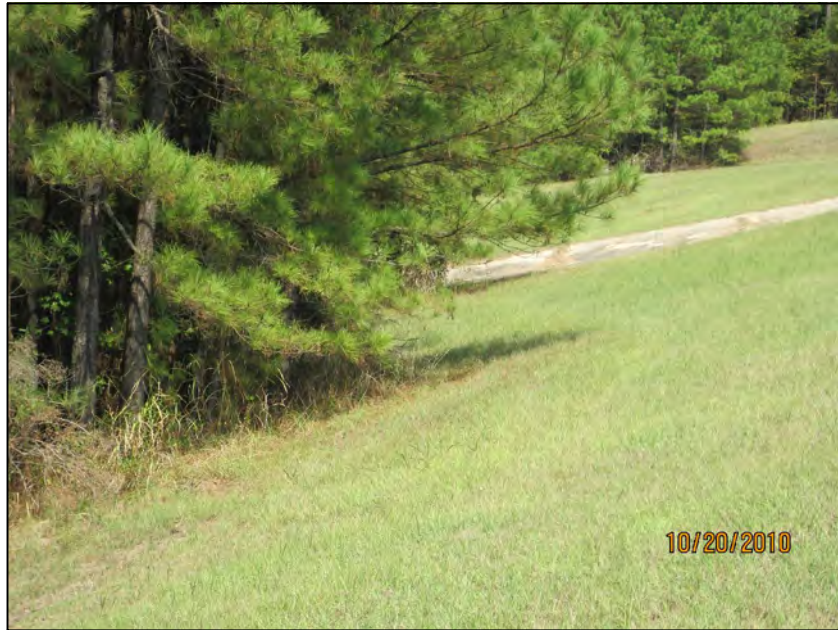
65 LANDFILL RUNOFF POND-TREES ON DOWNSTREAM TOE OF EMBANKMENT
