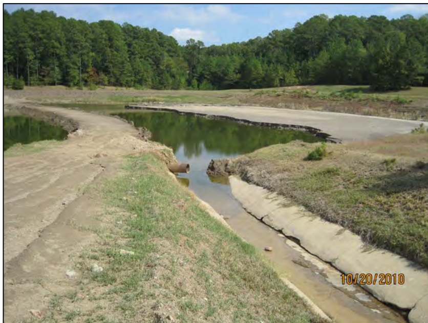
70 LANDFILL RUNOFF POND-LOOKING NORTHEAST AT POND INFLUENT CHANNEL
