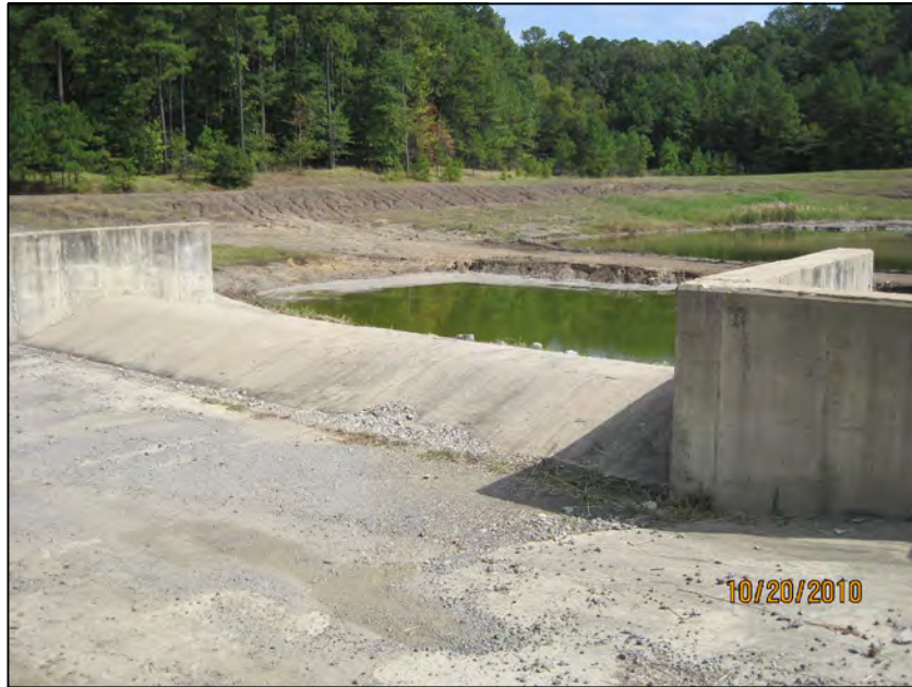
67 LANDFILL RUNOFF POND-LOOKING EAST AT EMERGENCY SPILLWAY
