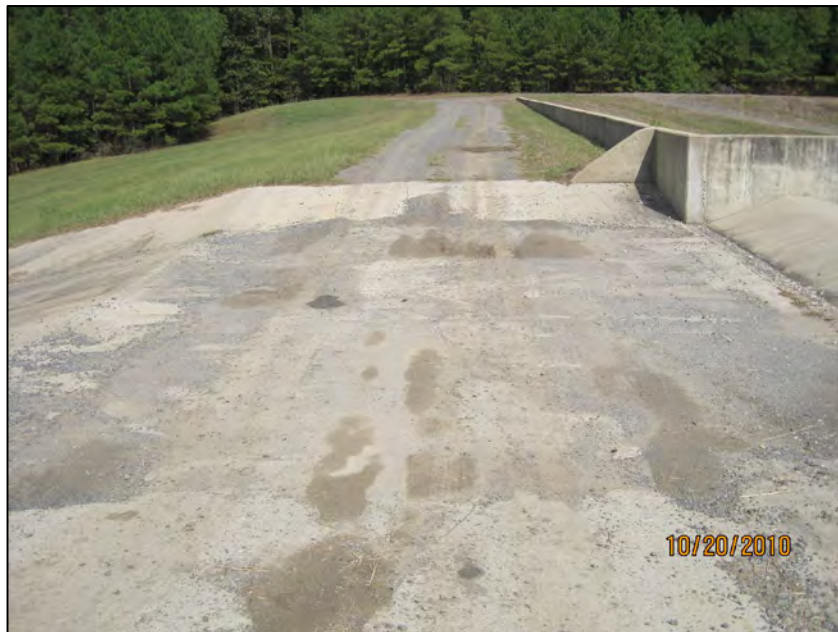
66 LANDFILL RUNOFF POND-LOOKING NORTHEAST ACROSS EMERGENCY SPILLWAY
