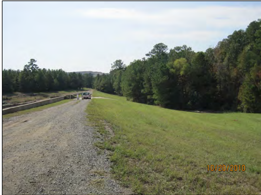
62 LANDFILL RUNOFF POND-LOOKING SOUTHWEST ALONG DOWNSTREAM EMBANKMENT
