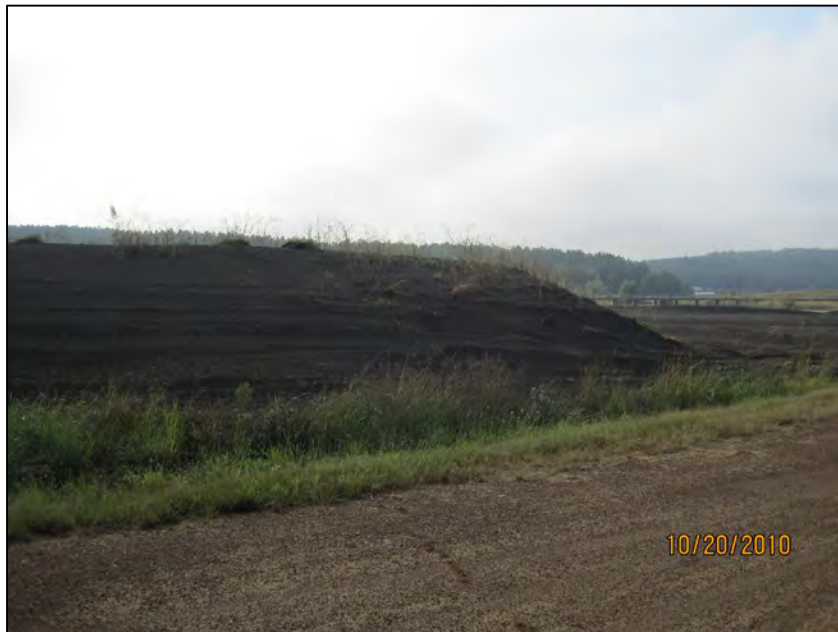
26 ASH POND 2-LOOKING SOUTH AT STACKED ASH
