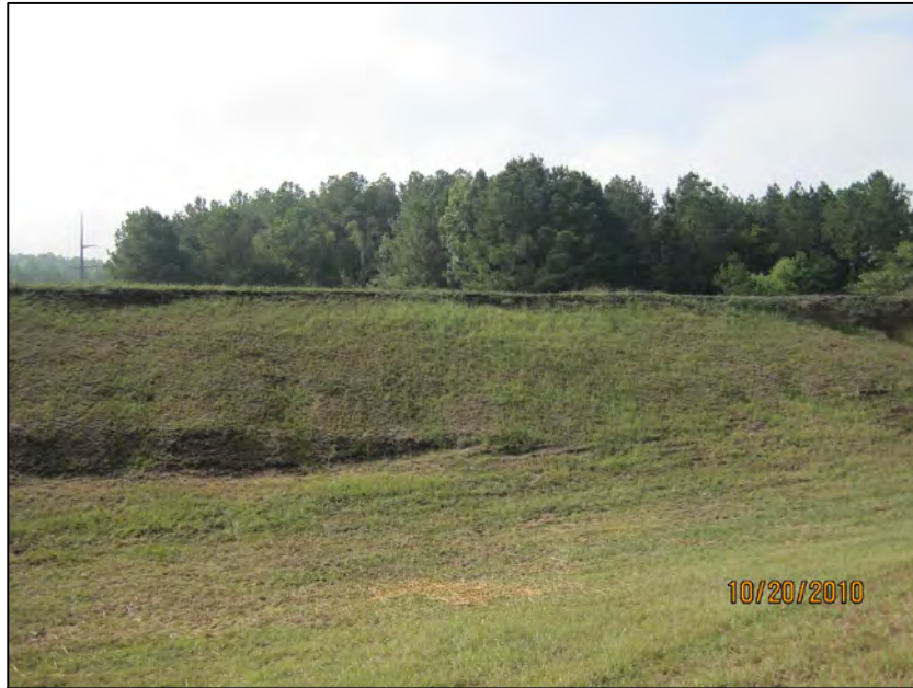
ASH POND 1-LOOKING SOUTHWEST AT EROSION ON SIDE OF ROADWAY LEADING TO ASH POND 1 EMBANKMENT CREST
