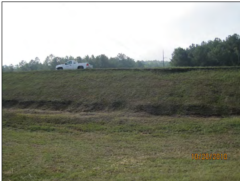
ASH POND 1-LOOKING SOUTH AT EROSION ON SIDE OF ROADWAY LEADING TO ASH POND 1 EMBANKMENT CREST
