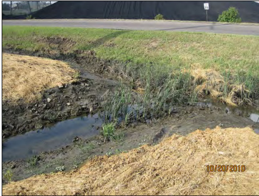
11 SECONDARY ASH POND-LOOKING SOUTHWEST AT LPDES OUTFALL 002 CHANNEL
