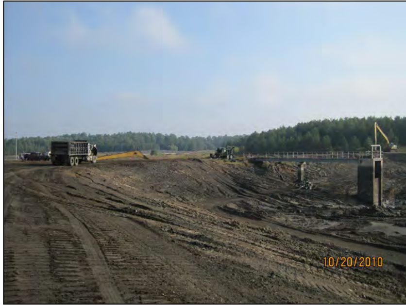
15 ASH POND 1-LOOKING NORTH FROM CREST
