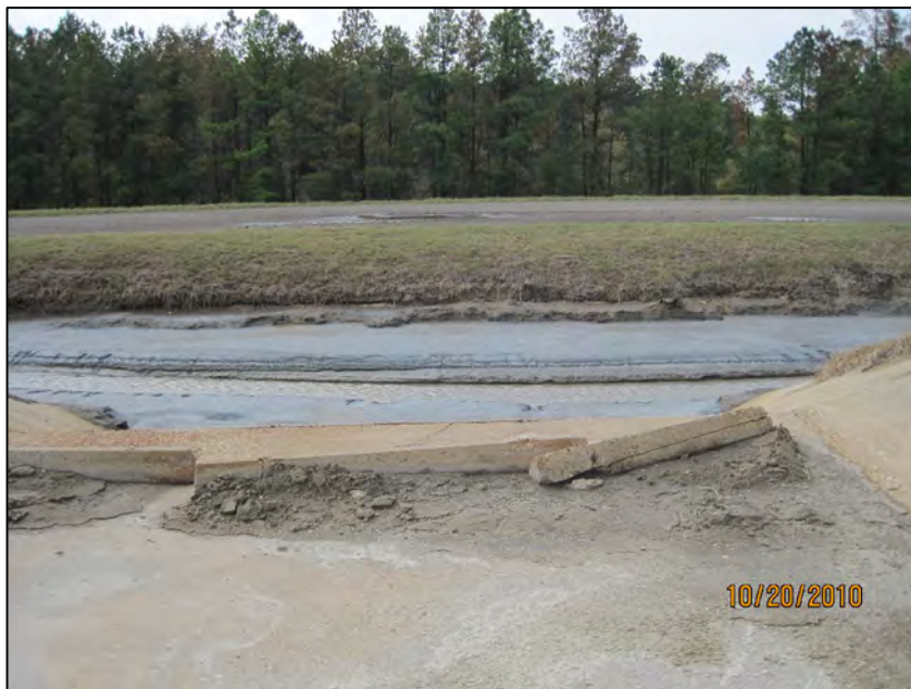
42 AUXILIARY SURGE POND-DISCHARGE SPILLWAY
