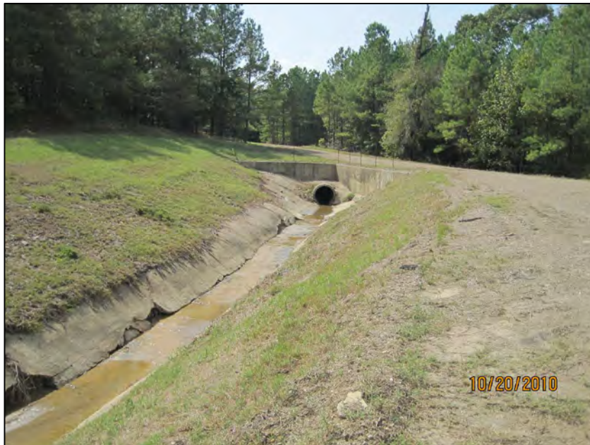
69 LANDFILL RUNOFF POND-LOOKING SOUTHWEST AT POND INFLUENT PIPE
