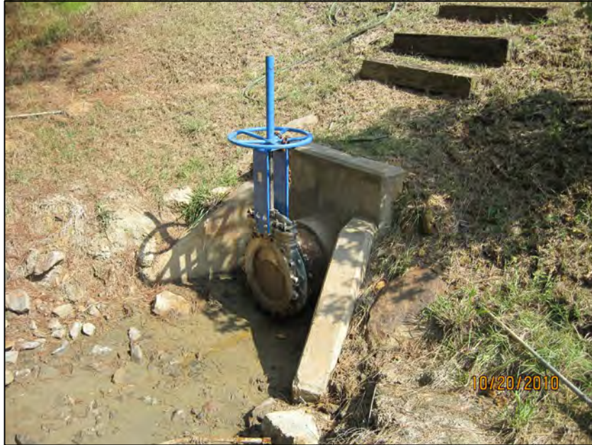
LANDFILL RUNOFF POND-VALVE CONTROL AT DISCHARGE
