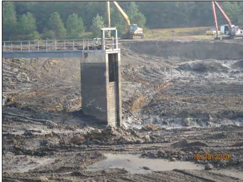
16 ASH POND 1-LOOKING NORTHEAST AT DISCHARGE STRUCTURE
