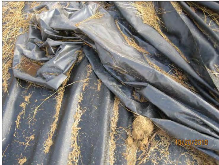
ASH POND 2-WOVEN AND PLASTIC FABRIC DRAINAGE SWALE PROTECTION
