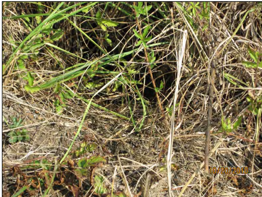
SURGE POND 1-ANIMAL BURROW LOCATED ON SOUTH FACE OF EMBANKMENT
