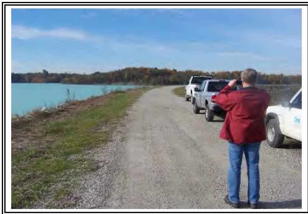
Dam crest, looking southwest.
