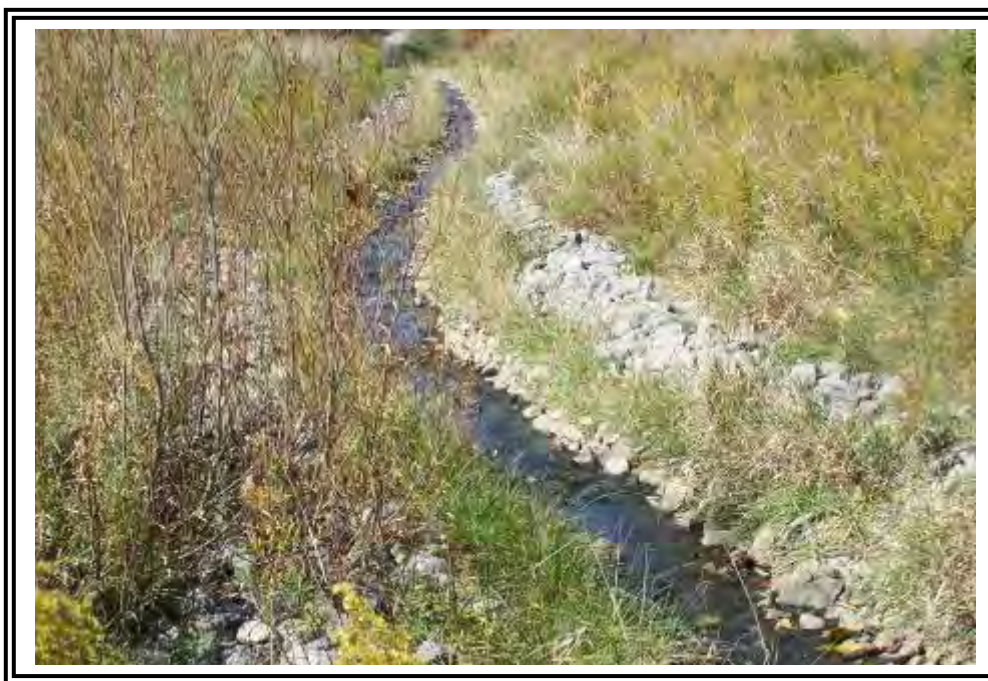
Channel downstream of the right abutment (RA) v-notch weir to stilling basin.
