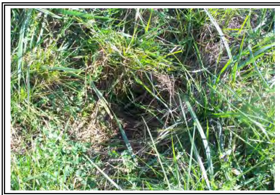
Small rodent hole on upstream slope of Little Blue Run Saddle Dam.
