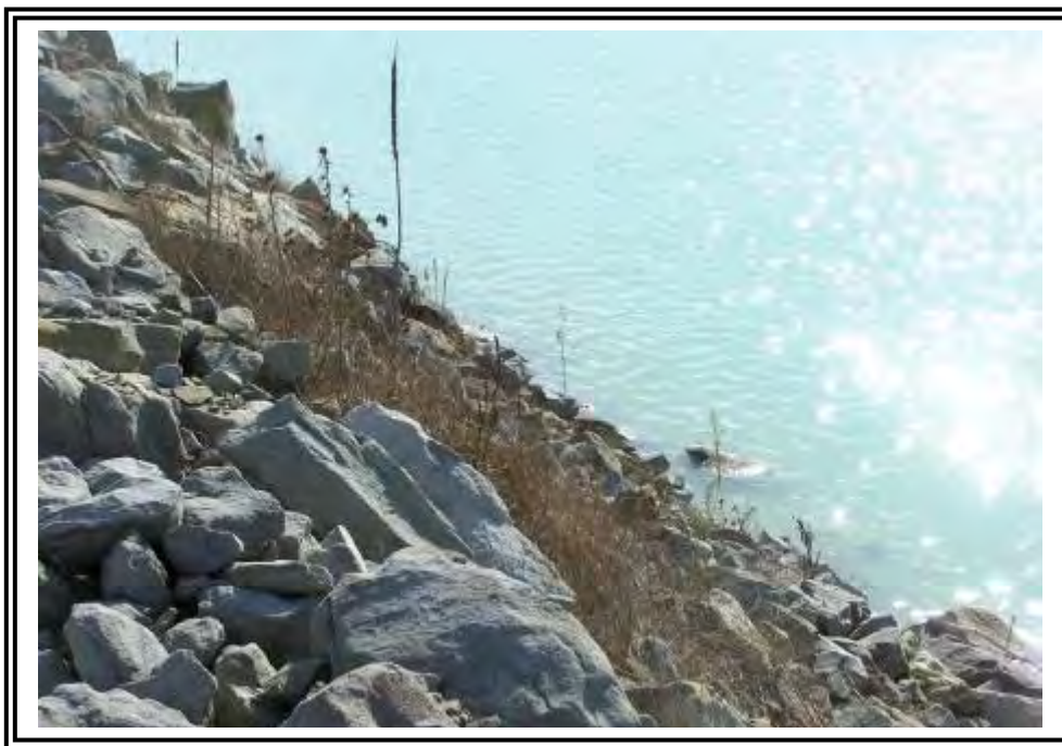
Upstream slope, looking southeast.
