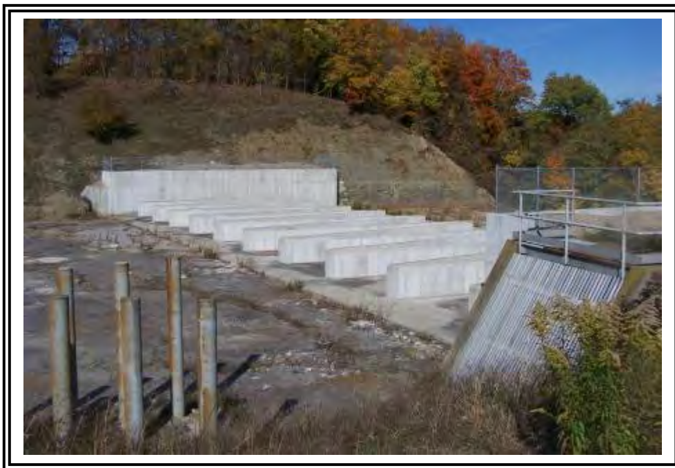
Concrete labyrinth (left-center) and Service Spillway inlet with trash rack and bollards (right).
