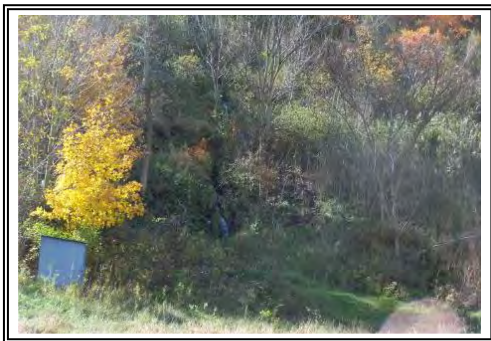
West abutment seepage.
