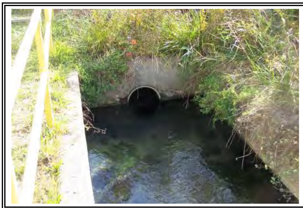
Toe drain (TD) collection pipe terminating in Parshall Flume.
