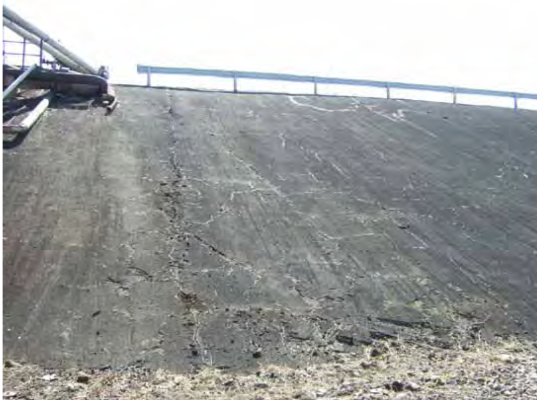
PHOTO 22: NORTH DOWNSTREAM SLOPE OF WEST HDS POND
