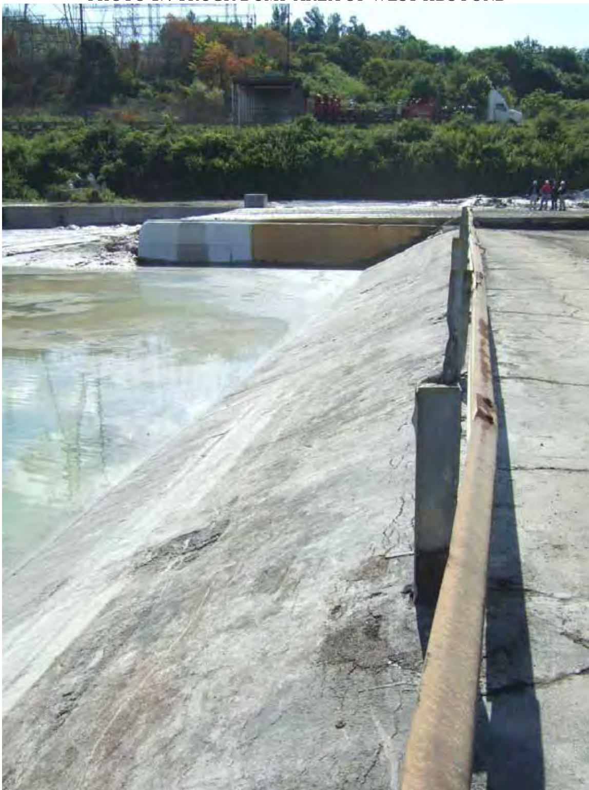
PHOTO 17: TRUCK DUMP AREA OF WEST HDS POND
