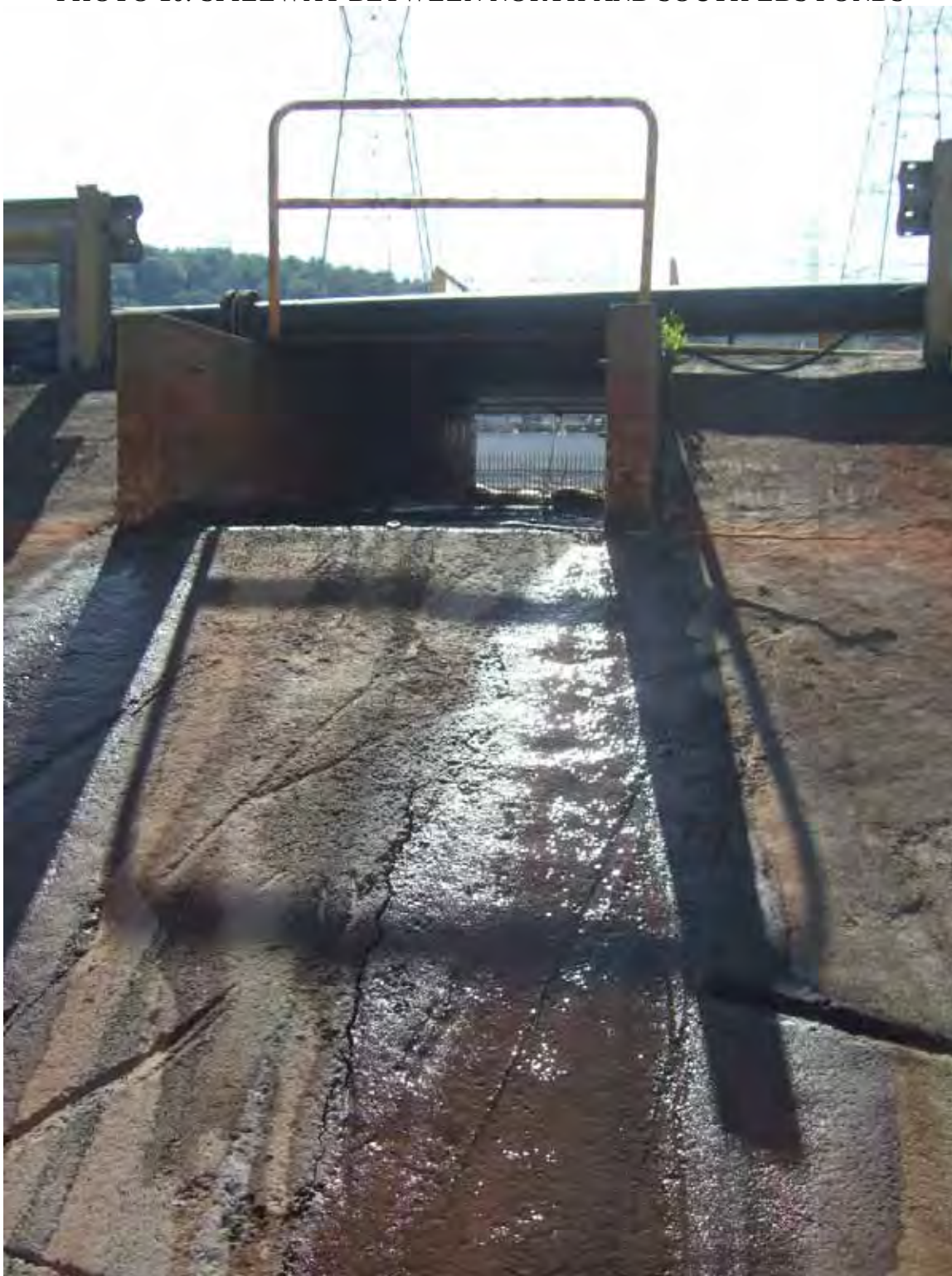
PHOTO 10: SPILLWAY BETWEEN NORTH AND SOUTH LDS PONDS
