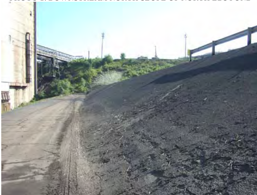
PHOTO 1: DOWNSTREAM NORTH SLOPE OF NORTH LDS POND
