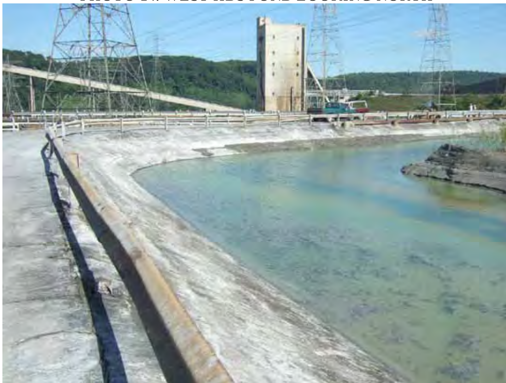
PHOTO 14: WEST HDS POND LOOKING NORTH
