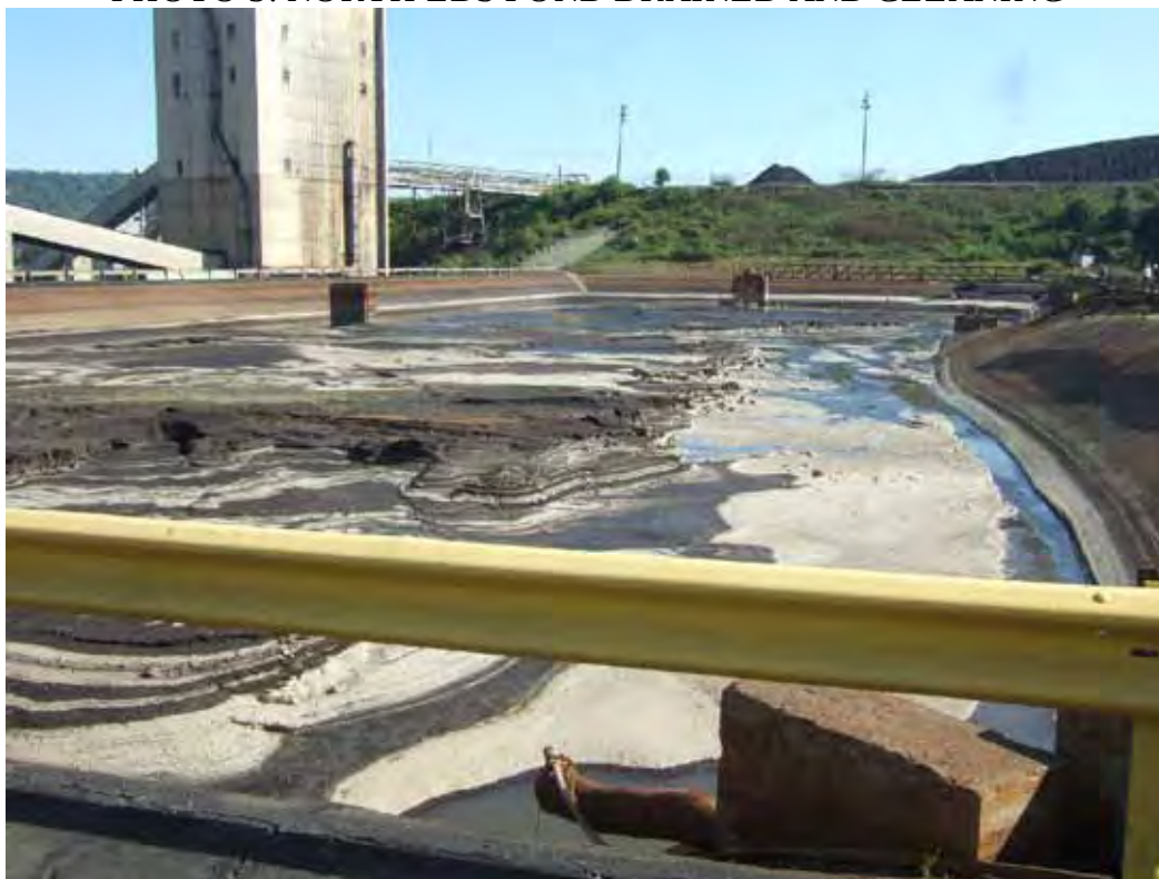
PHOTO 3: NORTH LDS POND DRAINED AND CLEANING
