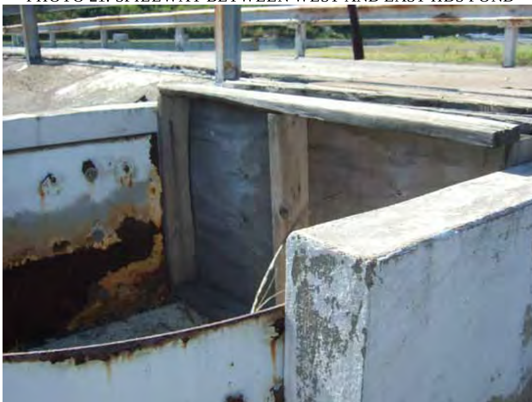
PHOTO 21: SPILLWAY BETWEEN WEST AND EAST HDS POND
