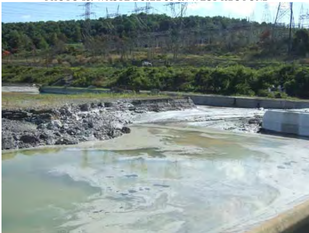
PHOTO 15: WASTE BUILDUP IN WEST HDS POND
