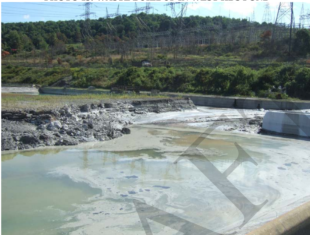
PHOTO 15: WASTE BUILDUP IN WEST HDS POND
