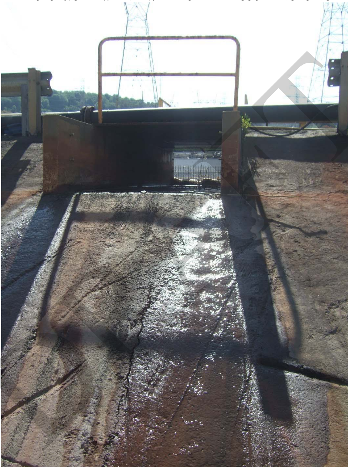
PHOTO 10: SPILLWAY BETWEEN NORTH AND SOUTH LDS PONDS
