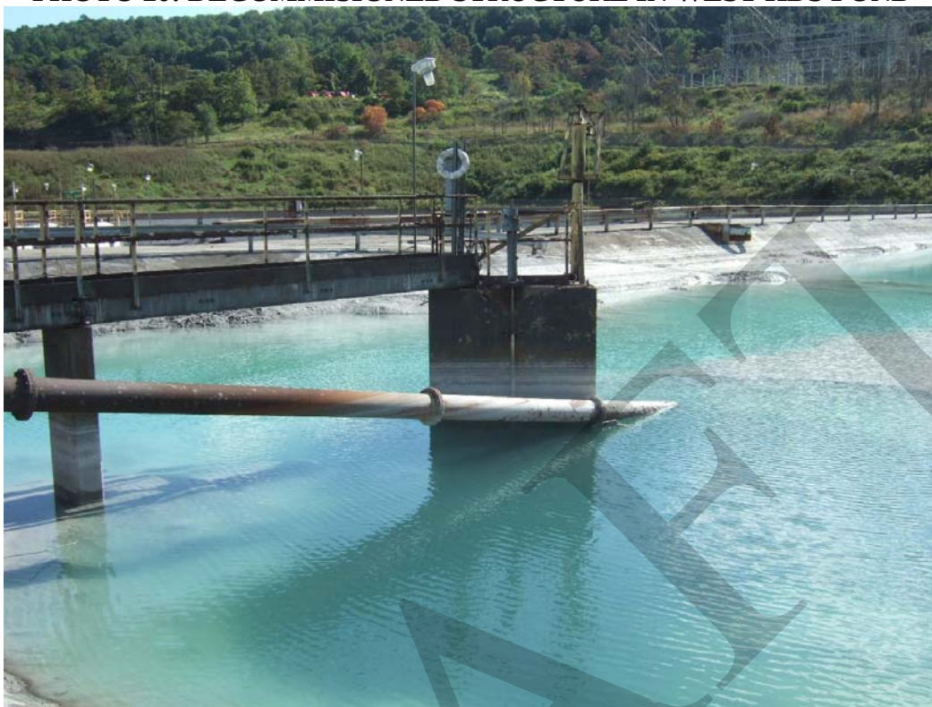
PHOTO 20: DECOMMISSIONED STRUCTURE IN WEST HDS POND
