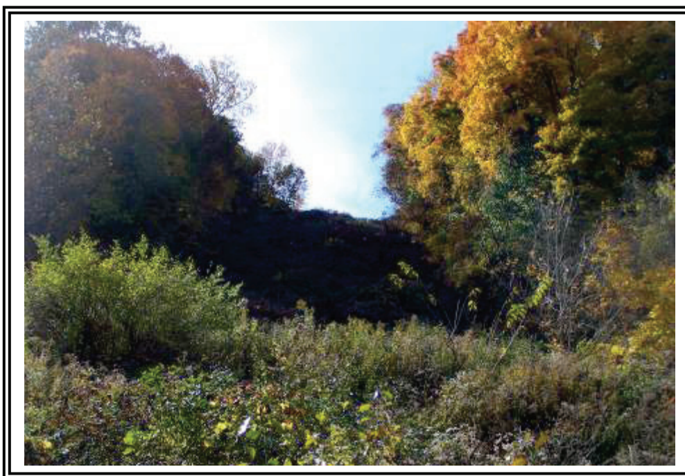
Emergency spillway channel over natural slope, looking upstream from the stilling basin.
