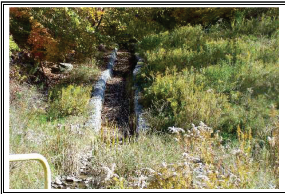
Gabion channel from secondary spillway.
