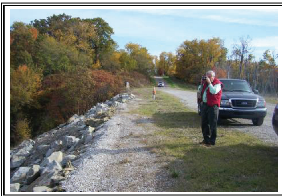
East abutment, looking east.
