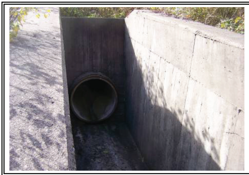
Terminus of service spillway at stilling basin.
