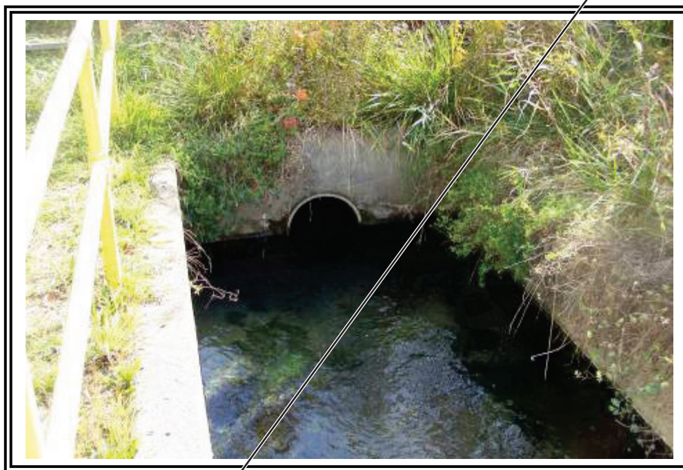
Toe drain collection pipe terminating in Parshall Flume.
