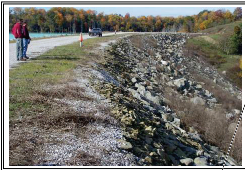
Crest elevation re-establishment made with darker stone and gravel.
