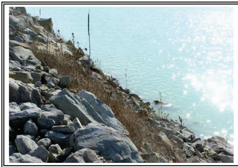
Upstream slope, looking southeast.
