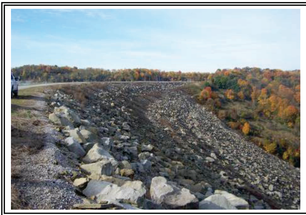
Downstream slope, looking west.
