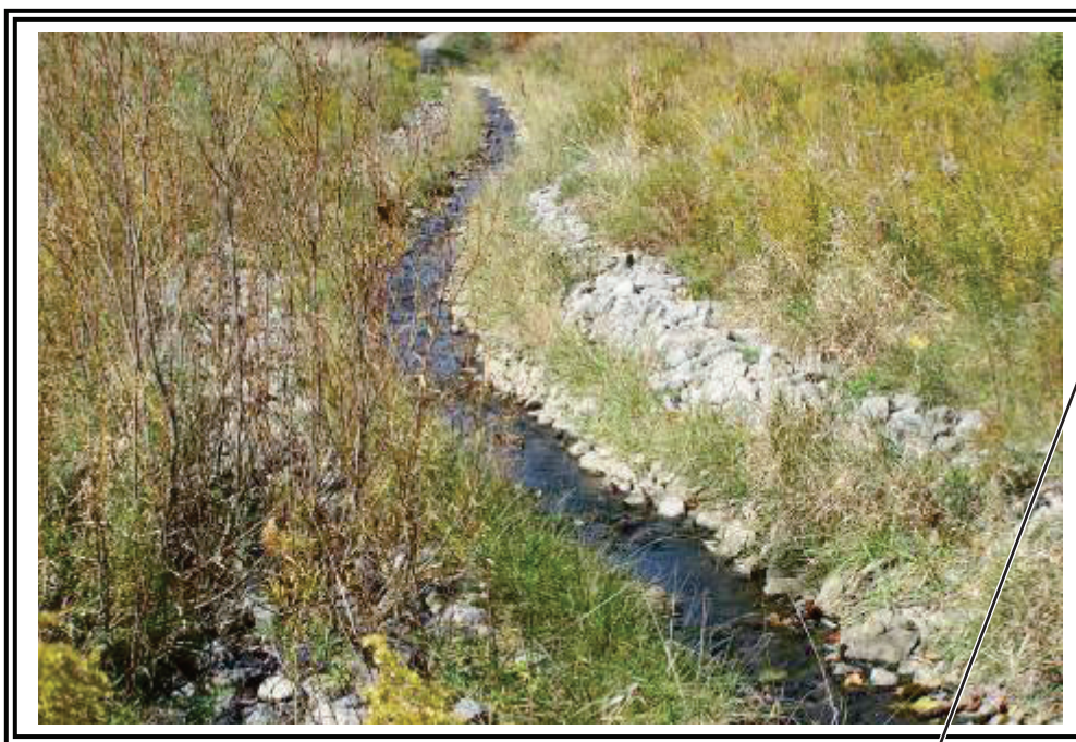
Channel downstream of east abutment v-notch to stilling basin.
