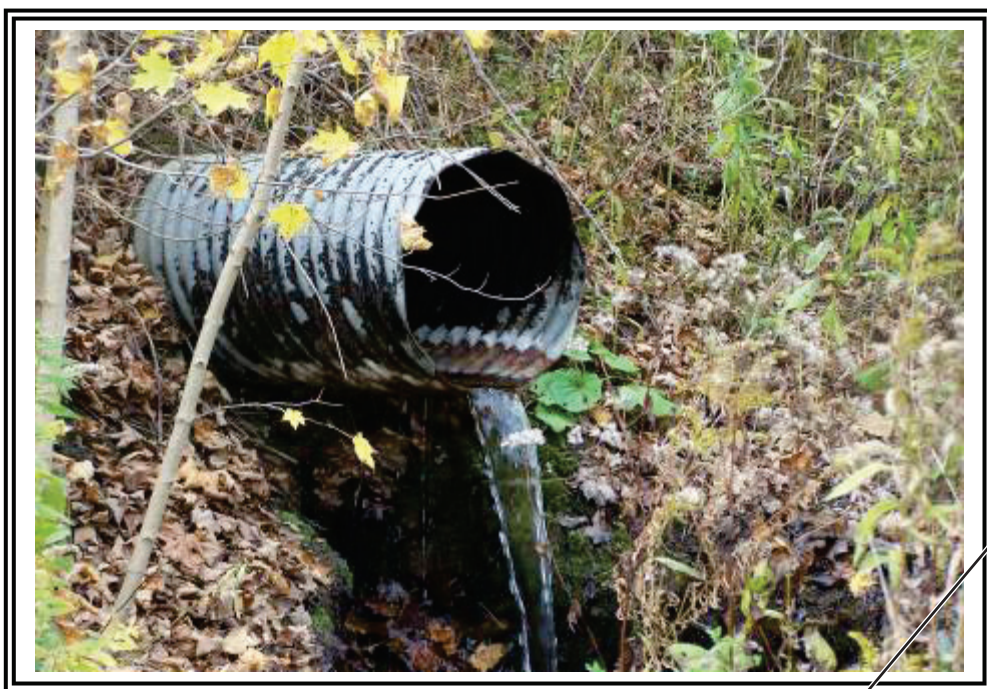
Lower left (west) abutment seepage. This natural seepage maintains flow in Little Blue Run per permit conditions.
