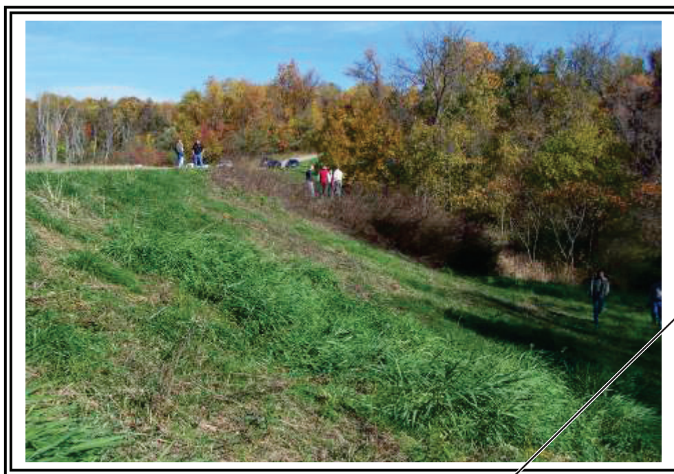
Downstream slope of Little Blue Run Saddle Dike , looking north. Vegetation near group of people on slope consists of material that the mower cannot traverse.
