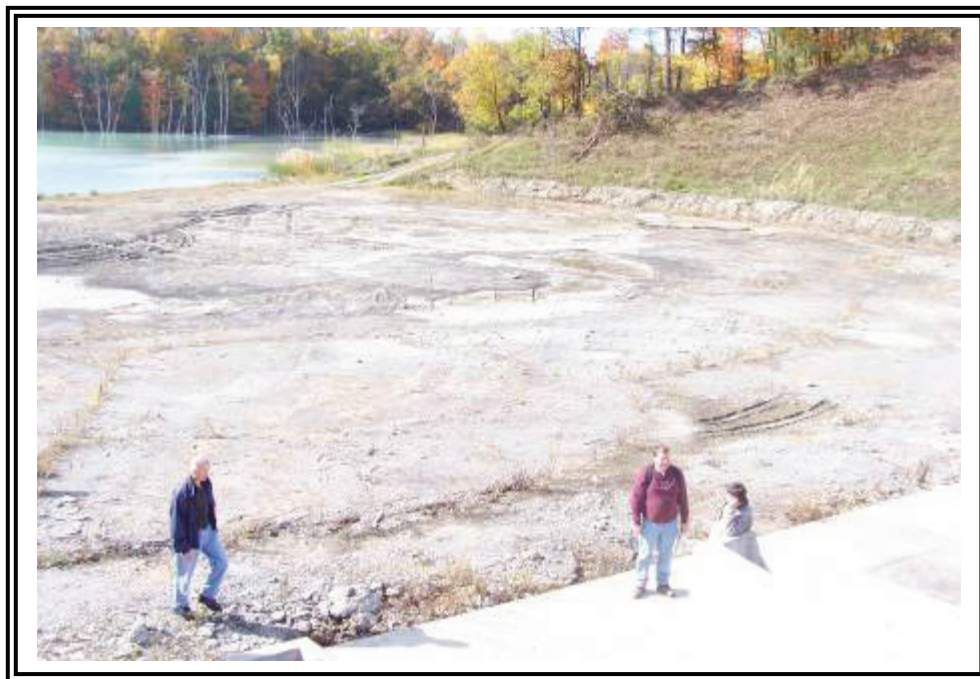
Approach to emergency spillway in bedrock.
