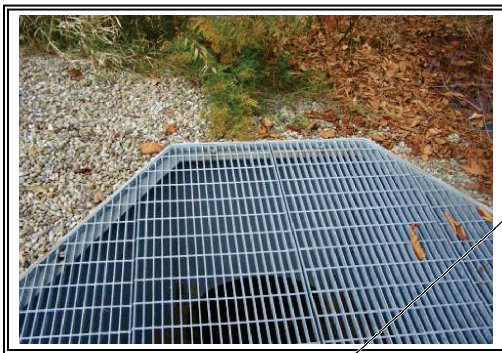
Outfall from stilling basin conveyed by buried pipe to the Ohio River.
