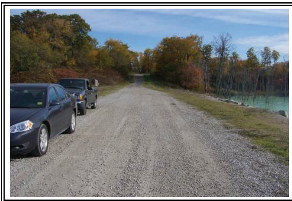
Crest and east abutment, looking east.
