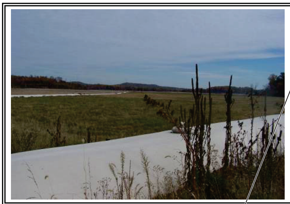
Geotubes and dry ash placement at south end of reservoir.
