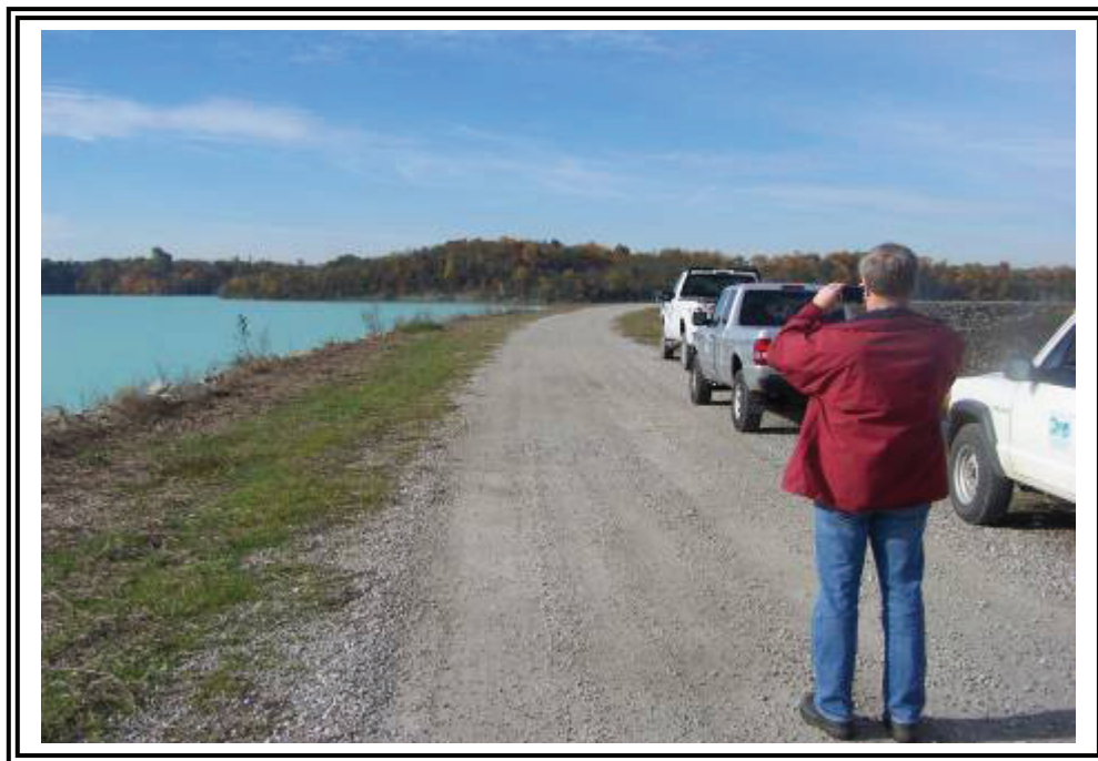
Dam crest, looking southwest.
