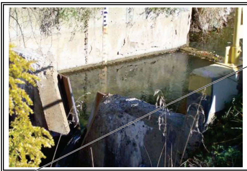
V-notch monitoring weir containing secondary spillway and east abutment seepage flow.
