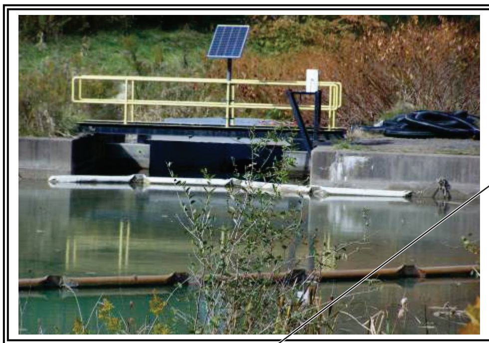
Stilling basin sediment control.
