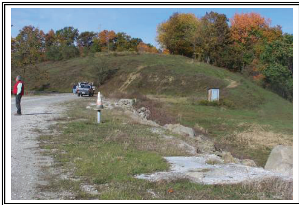
West abutment, looking west.
