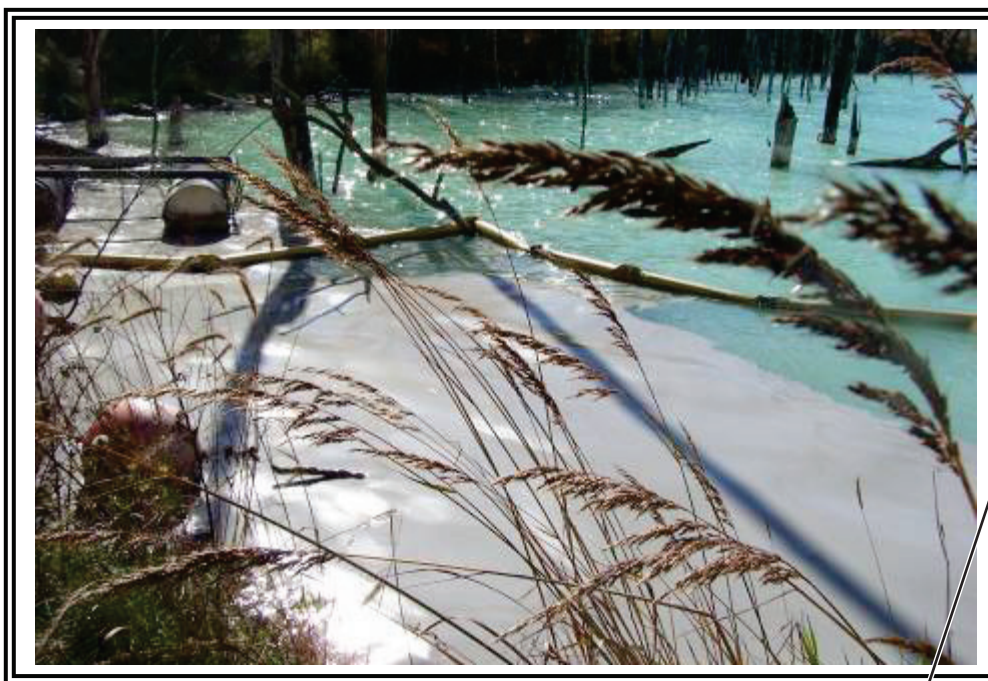
Area of secondary spillway intake. Pipe was submerged during our sit visit.
