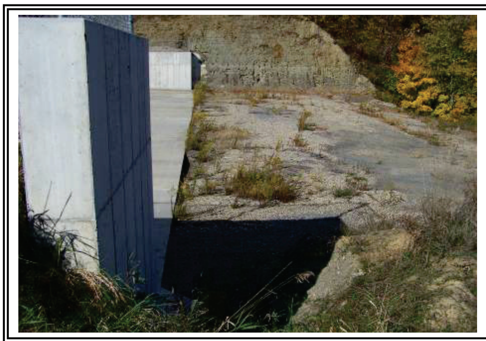
Downstream channel of emergency spillway.
