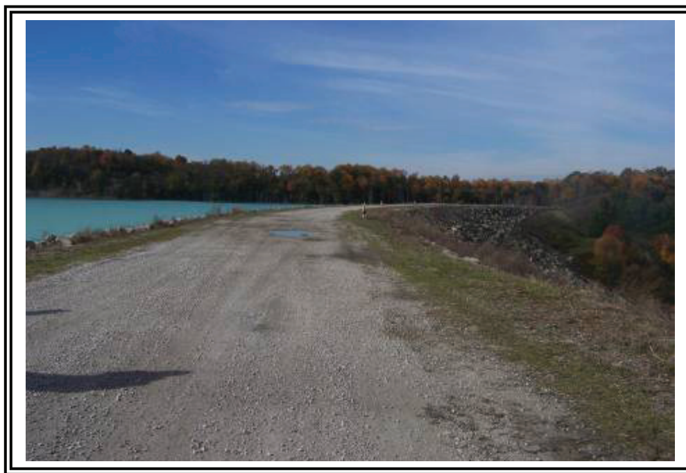
Dam crest, looking west.
