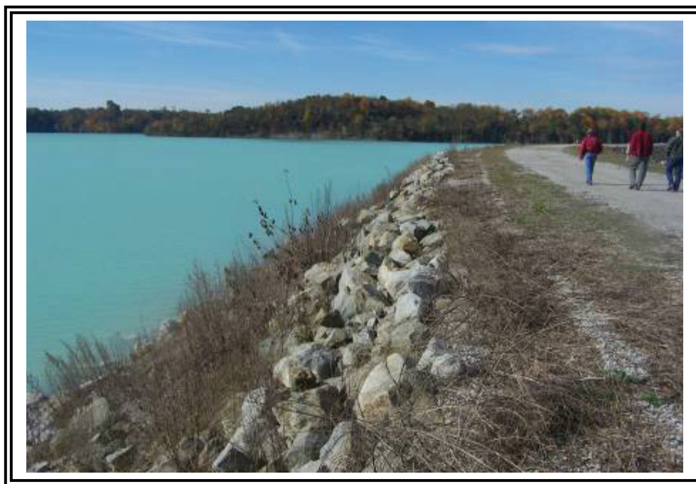
Upstream slope, looking southwest.
