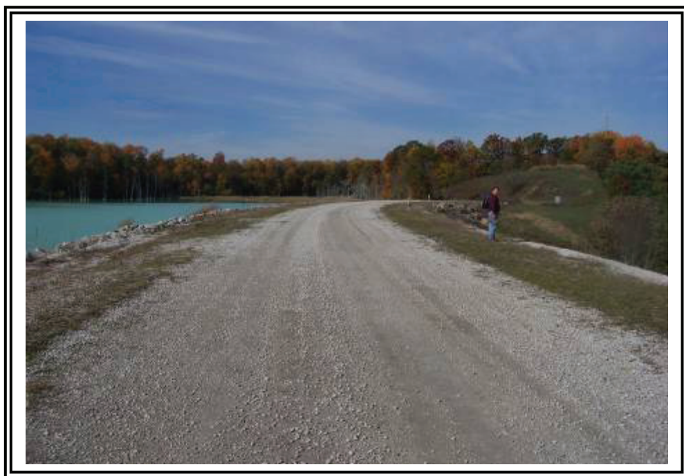
Dam crest, looking west.
