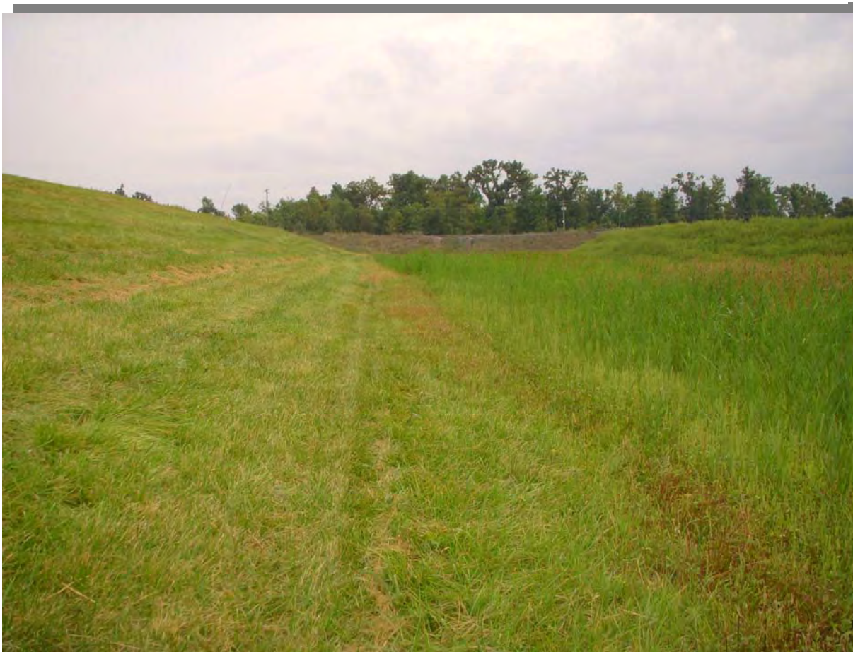
Photo 6 – View along outboard toe of south dike looking east. Note high vegetation in drainage swale beyond the toe.
