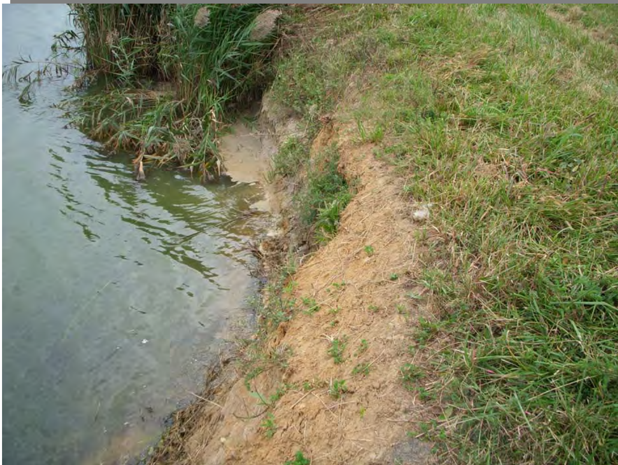
Photo 1 – Typical erosion of inboard slope on west side of pond.
