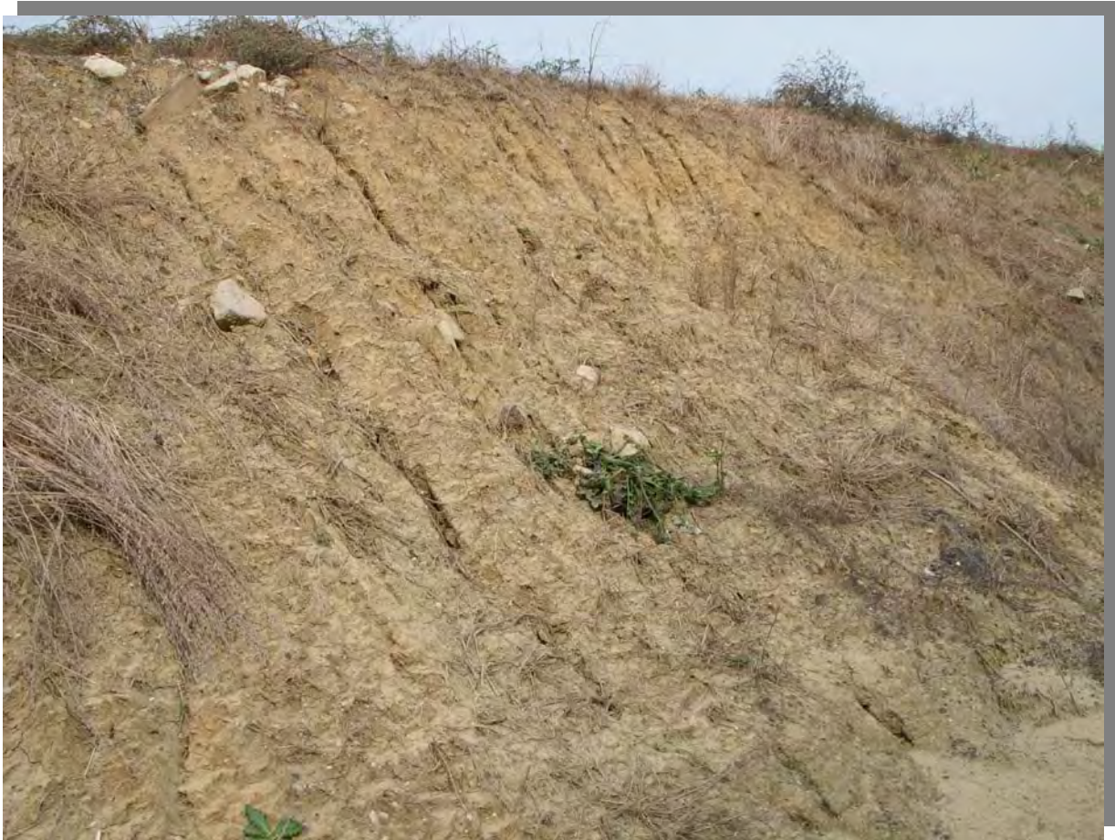
Photo 7 – East dike outboard slope impacted by excavation and erosion.
