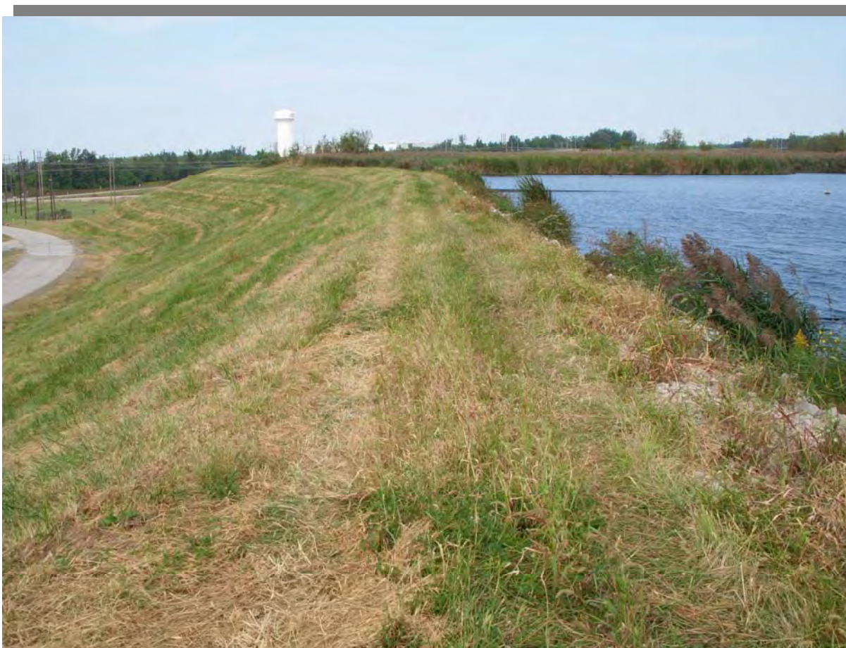
Photo 2 – View of south dike crest looking west.
