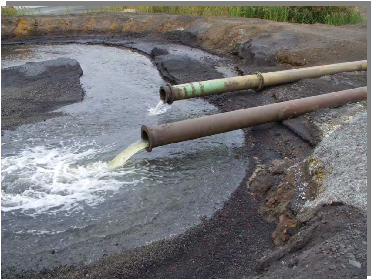
Photo 8 – Influent pipes discharging sludged bottom ash into pond.
