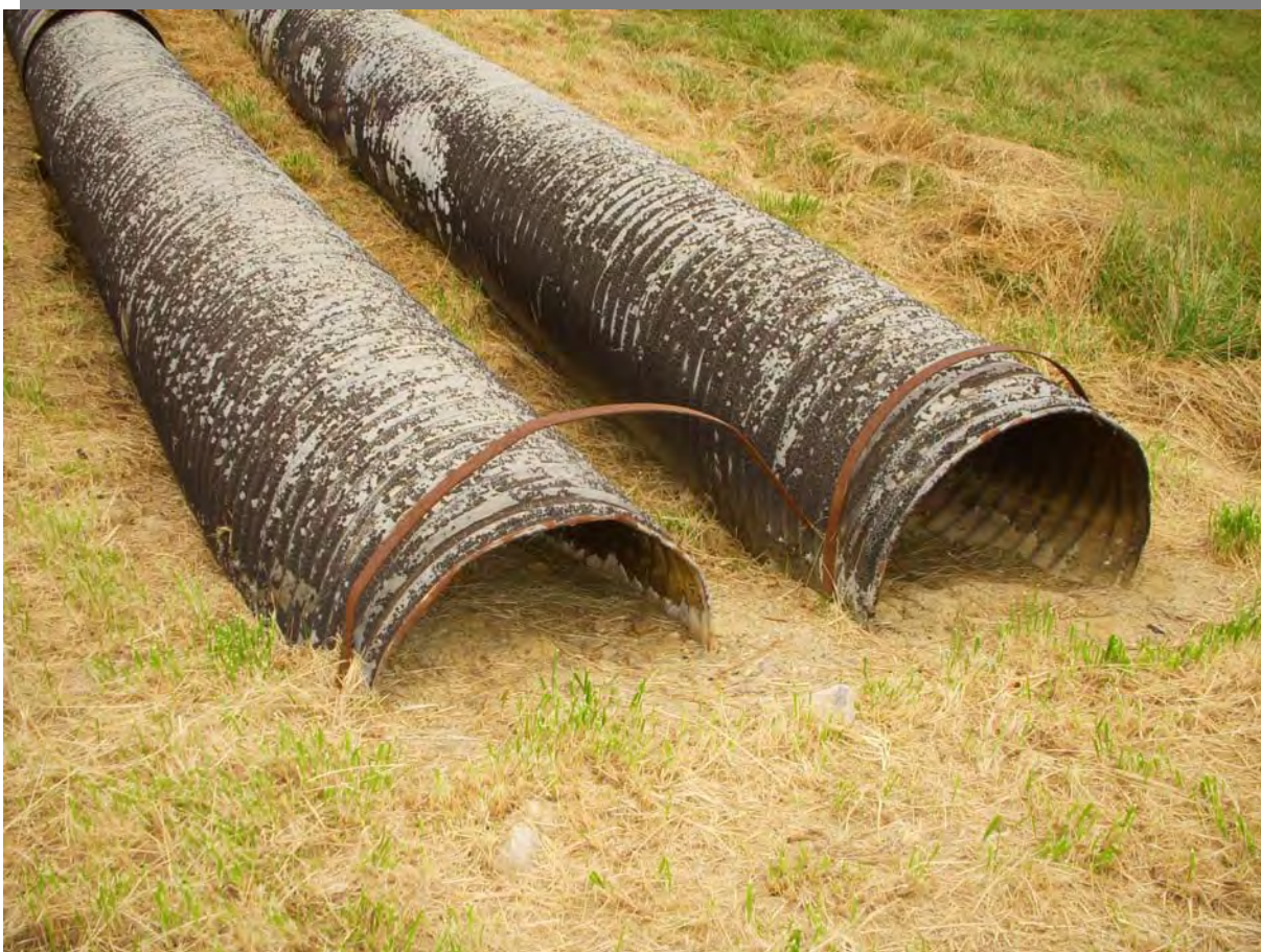
Photo 5 – Downstream end of emergency overflow pipes. Note siltation of outlet.
