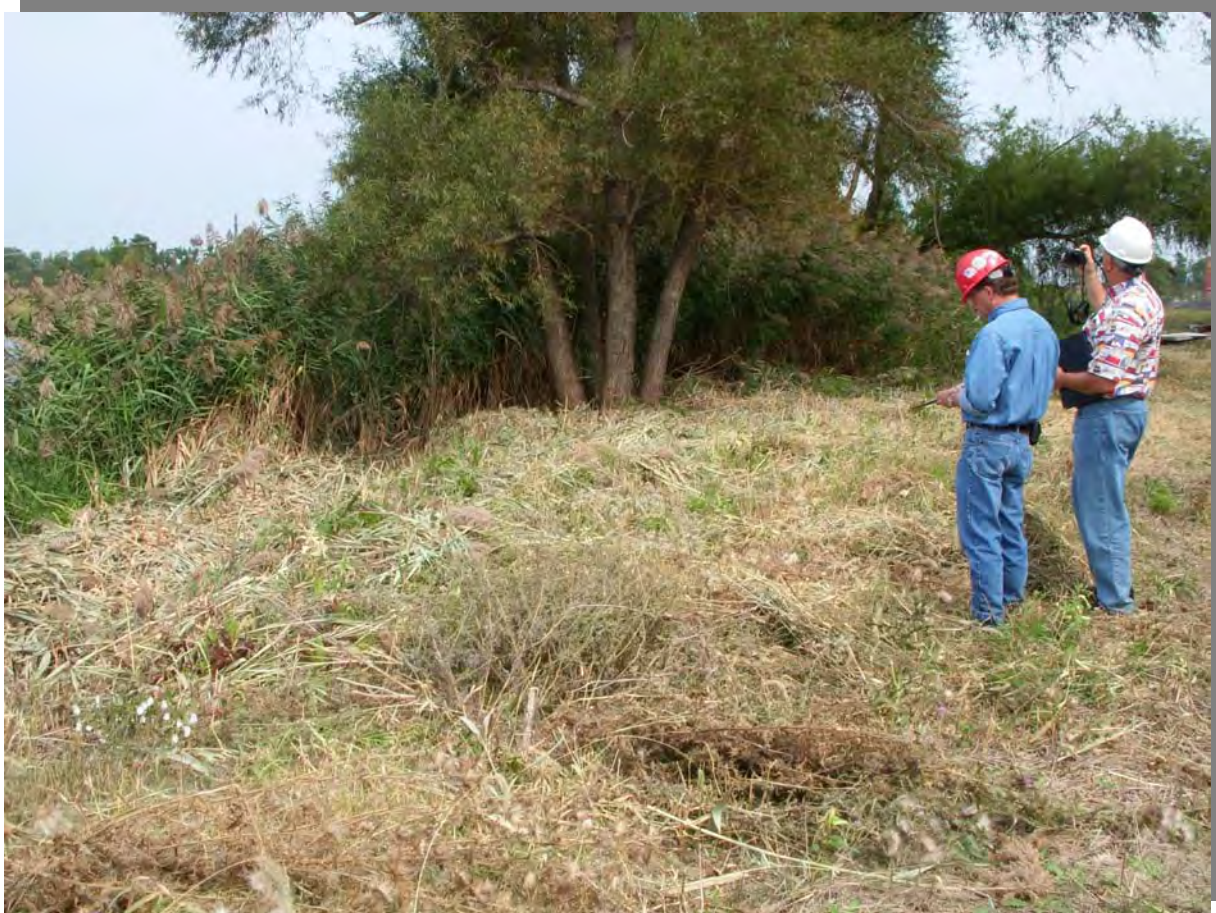
Photo 6 – East dike crest with willow tree.
