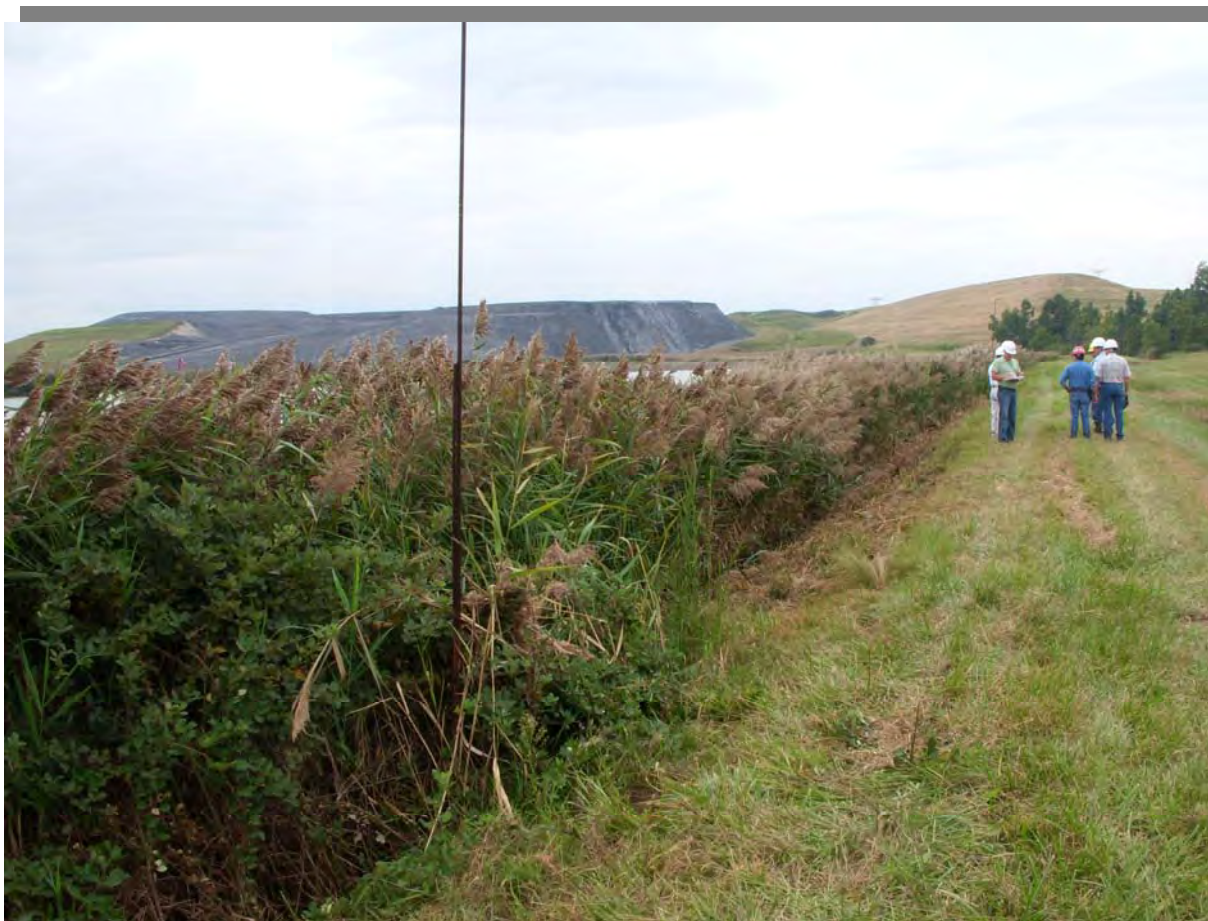
Photo 2 – Crest of low west dike looking south. Note heavy vegetation on inboard slope.
