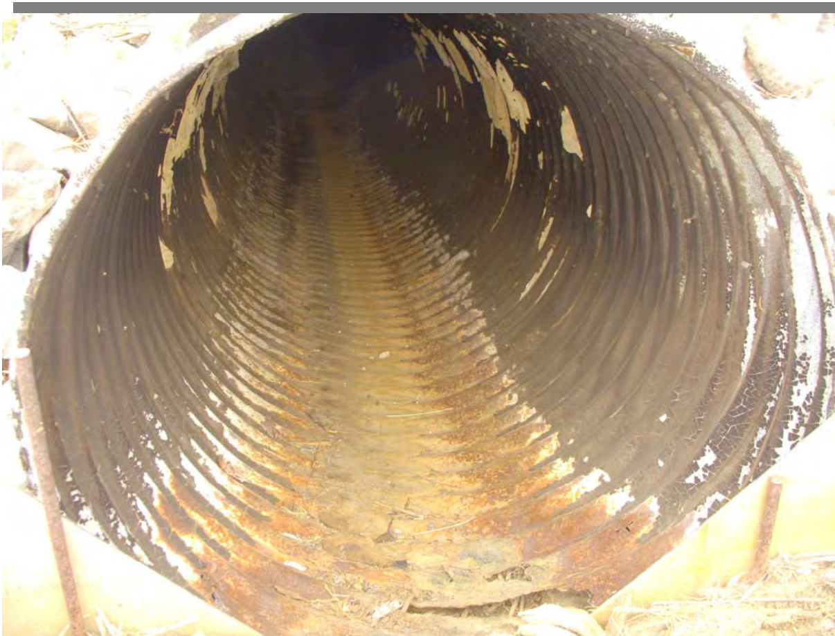
Photo 4 – View of deteriorated 30-inch CMP emergency overflow pipe at upstream end.
