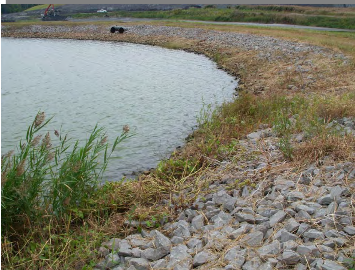
Photo 3 – Riprap-armored inboard slope of south dike. Note emergency overflow pipes in background.
