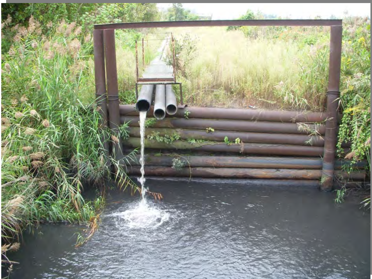
Photo 5 – Influent pipe discharging into northern ditch that parallels a portion of the northern inboard slope.
