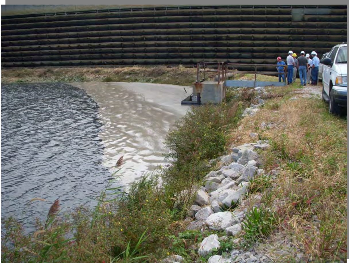
Photo 3 – View along inboard slope of south dike looking east. Note riprap armoring.
