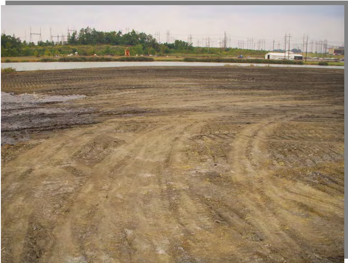
Photo 7 – View across the pond toward the west from the east side. Land in the foreground is former pond area that has been reclaimed with bottom ash.
