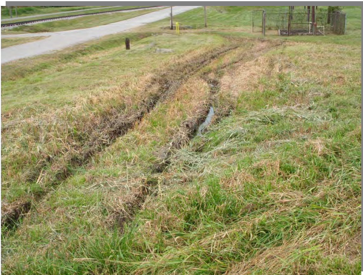
Photo 4 – Seepage and rutting along south outboard toe.
