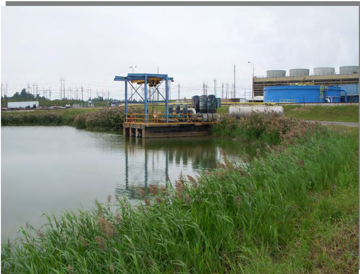
Photo 9 – View of pump station on incised inboard slope at the north end of the pond.
