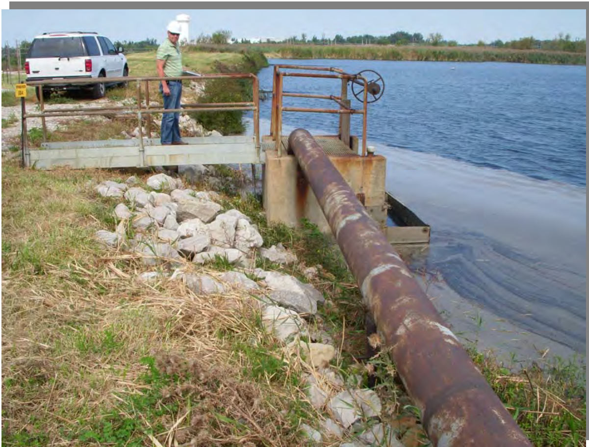
Photo 1 – View of pond outlet structure
