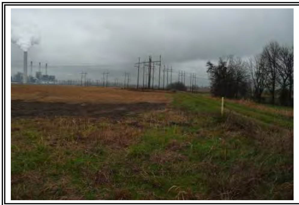
South dike inboard slope, looking east.
