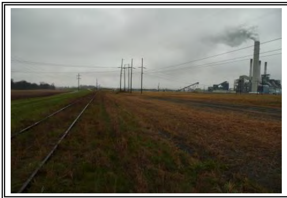
West dike inboard slope, looking north.
