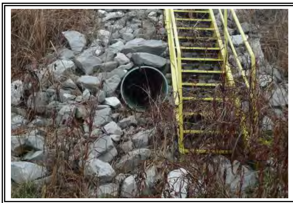
Outlet pipe on south dike.
