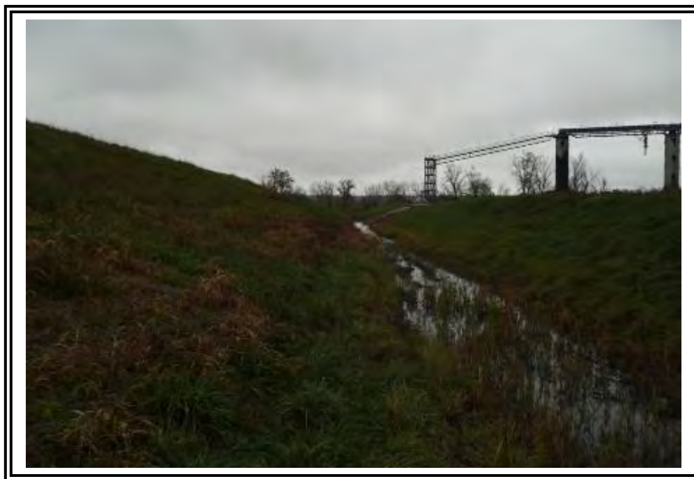
Standing water in drainage swale at toe of south dike.
