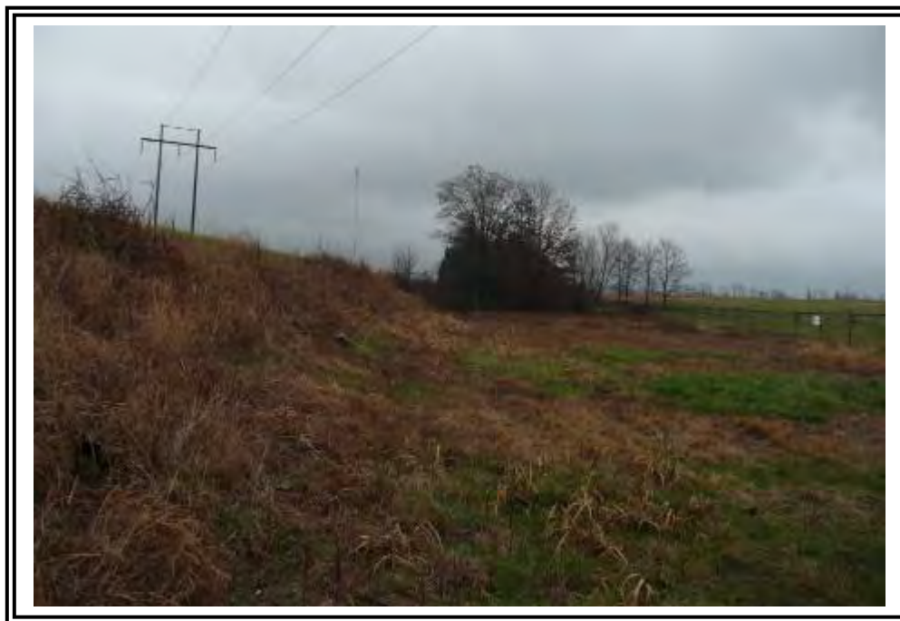
South dike outboard slope, looking east.
