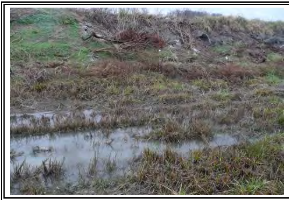
Poor drainage at toe of north dike where culvert under road has been blocked.
