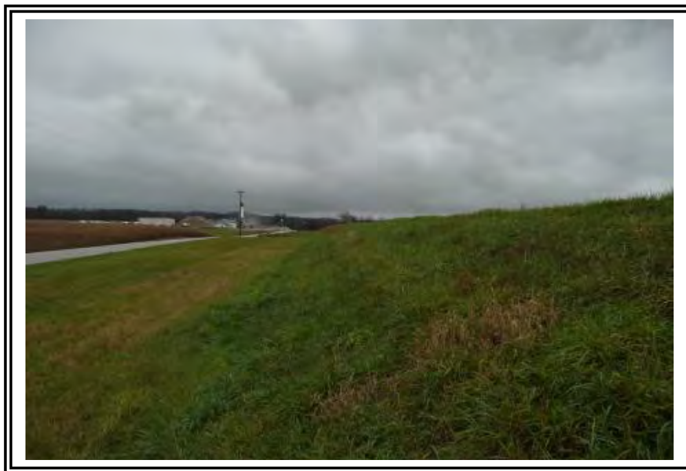
North dike outboard slope, looking east.
