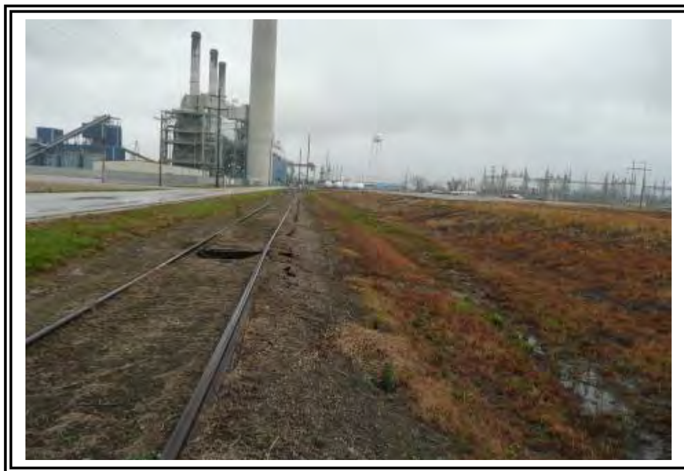
North dike crest area, looking east.
