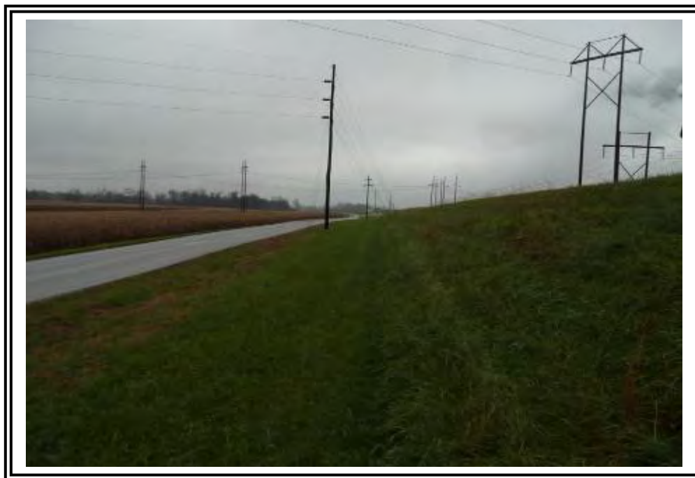
West dike outboard slope, looking north.
