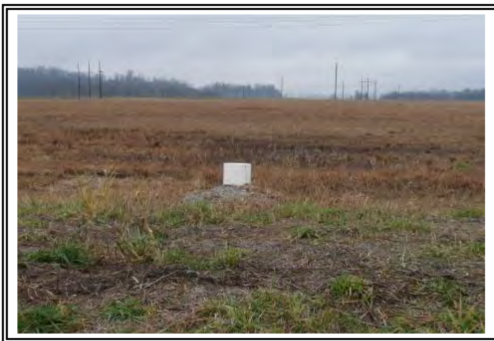
Outlet riser in pond area.
