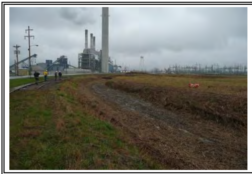
North dike inboard slope, looking east.
