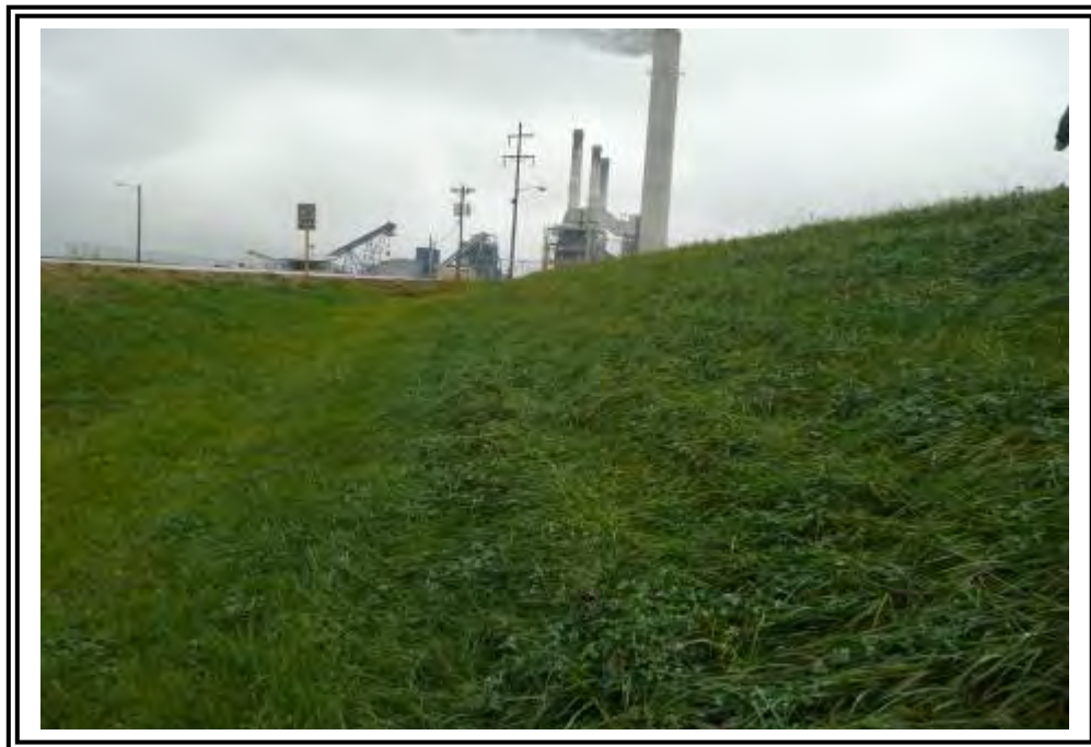
North dike outboard slope near facility driveway, looking east.
