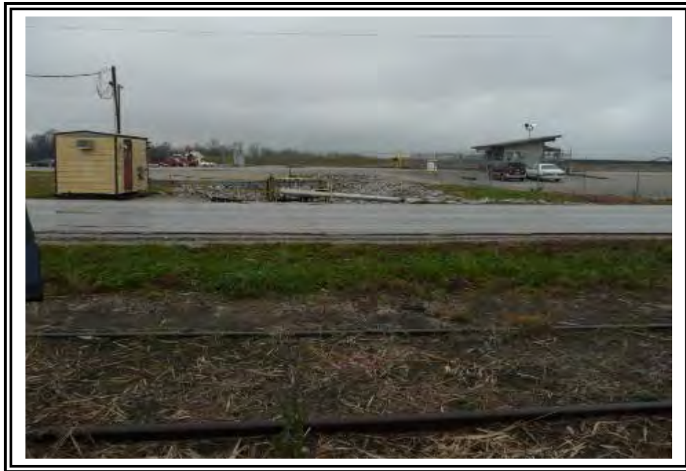
Looking north from north dike to reclaimed North Pond area.
