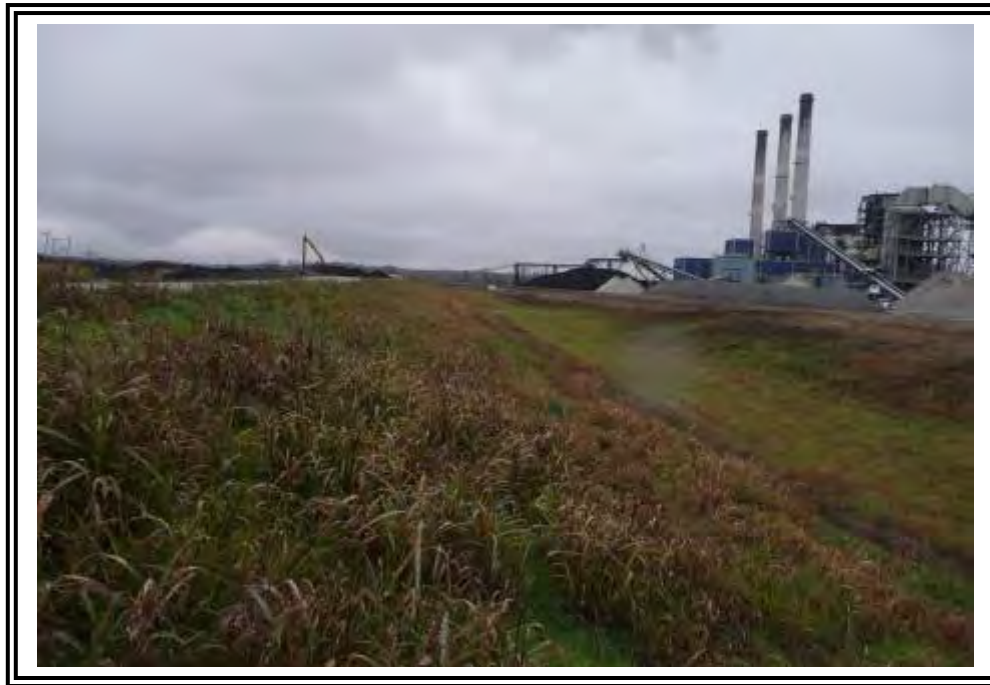
South dike outboard slope, looking east.
