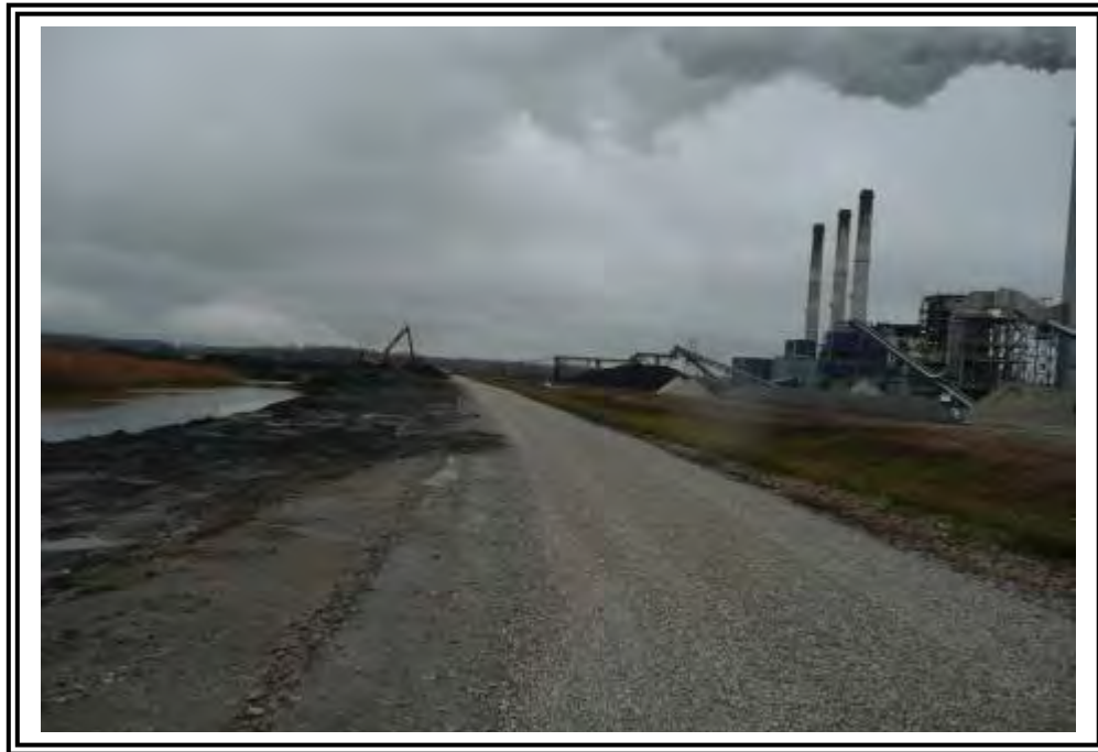
South dike inboard slope and crest at ash processing area, looking east. Note buildup of ash on inboard slope that widens crest area.
