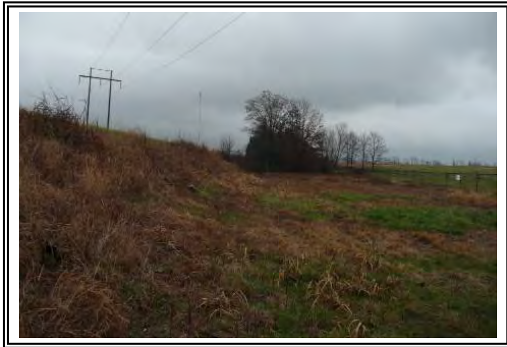
South dike outboard slope, looking east.
