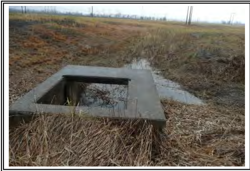
Old outlet structure to closed and reclaimed North Pond.
