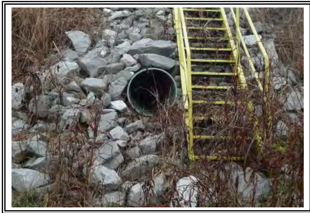
Outlet pipe on south dike.
