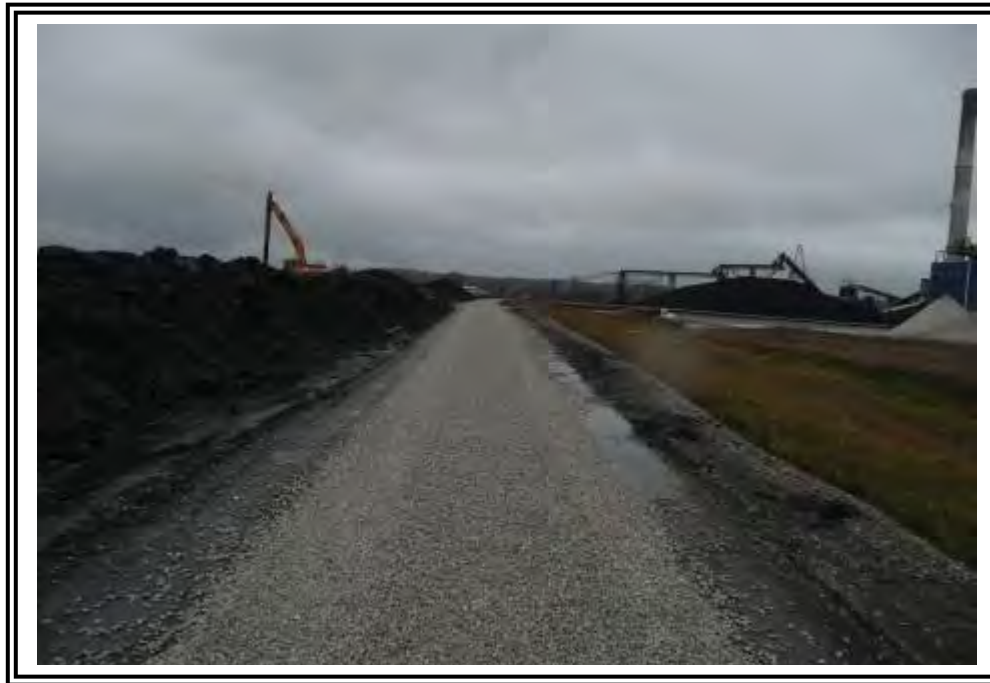
South dike crest looking east. Note standing water in puddles.
