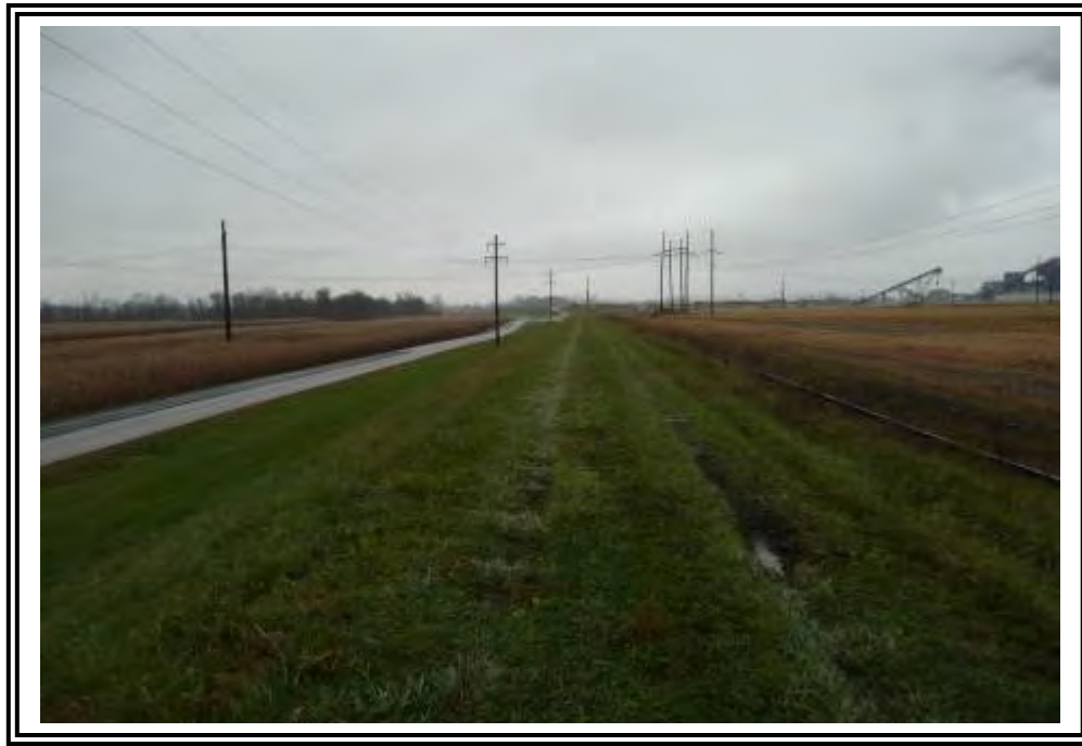
West dike crest, looking north.
