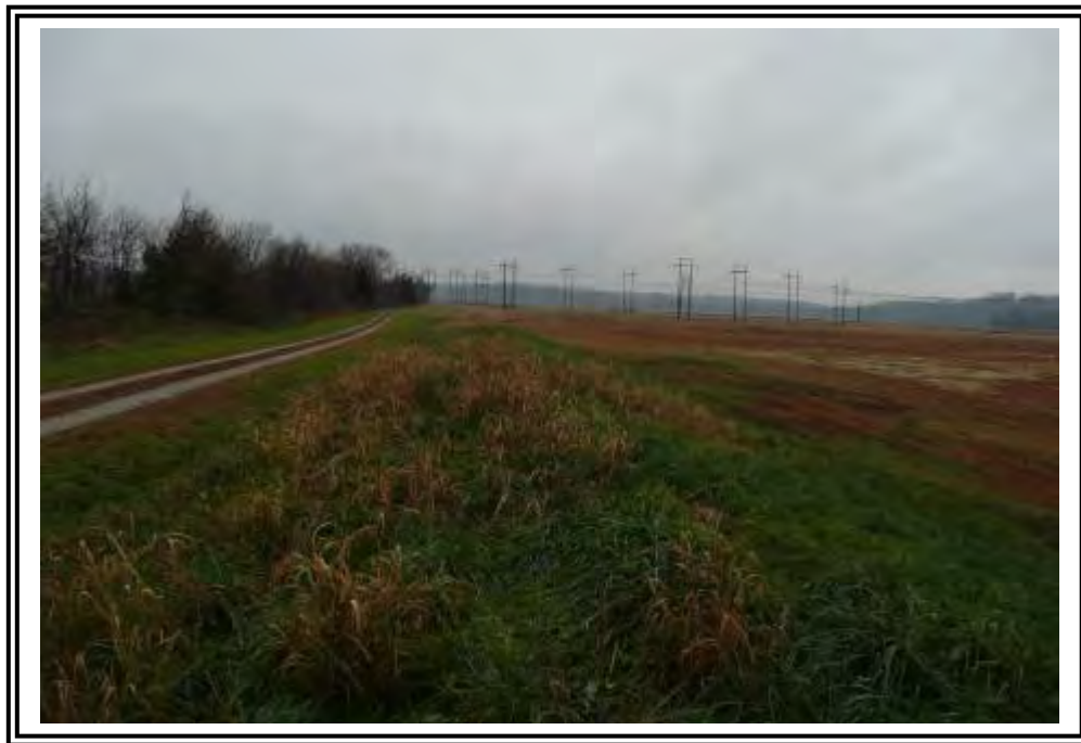
Looking west along south edge of pond from top of freeboard berm.
