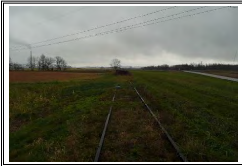
West dike crest, looking south along abandoned railroad spur.
