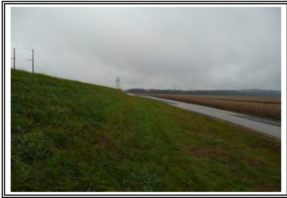
West dike outboard slope, looking south.
