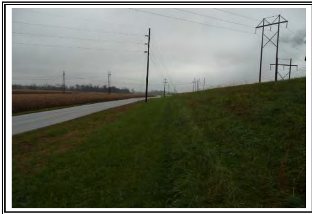
West dike outboard slope, looking north.
