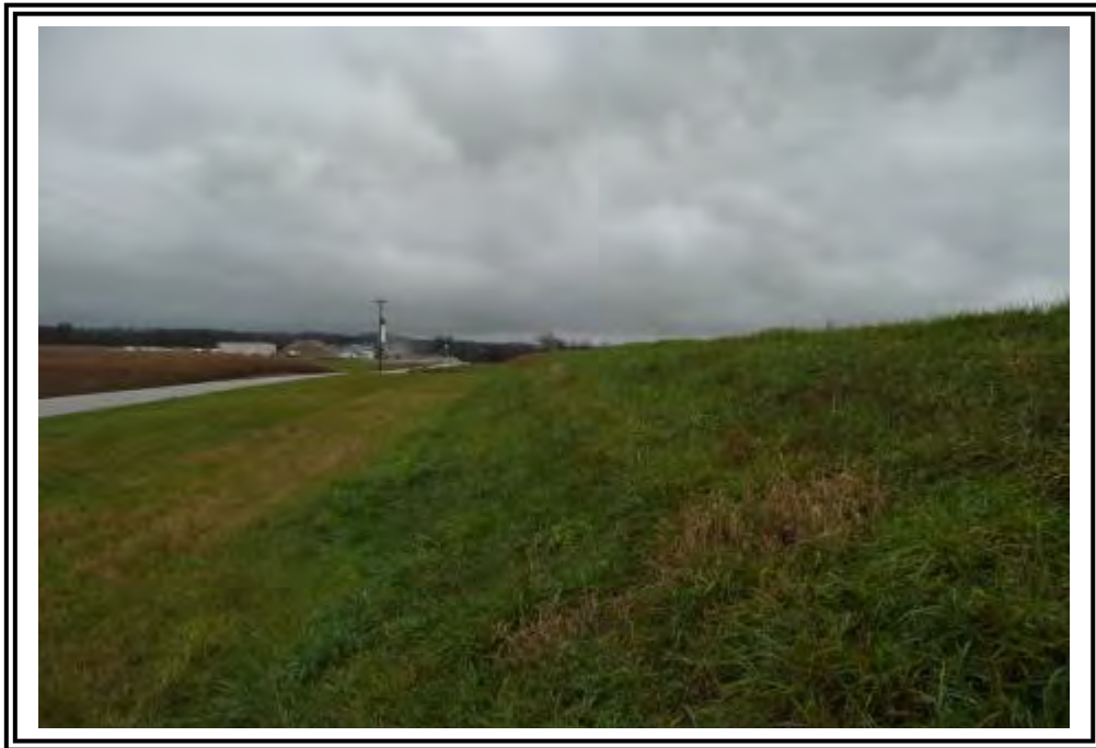
North dike outboard slope, looking east.
