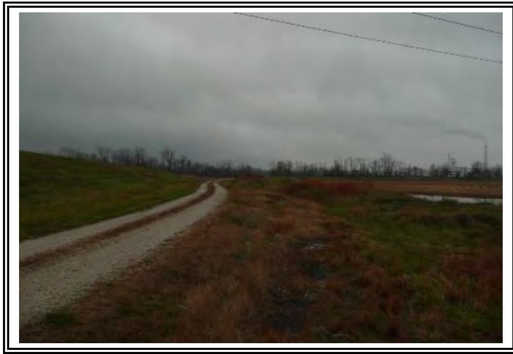
Access drive along east incised edge of pond, looking south. Interior berm built up to provide free board when pond is in use can be seen at right of photo.
