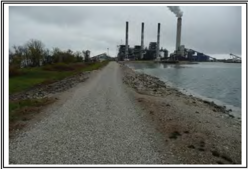
East dike crest, looking south. Note gravel crest surface.
