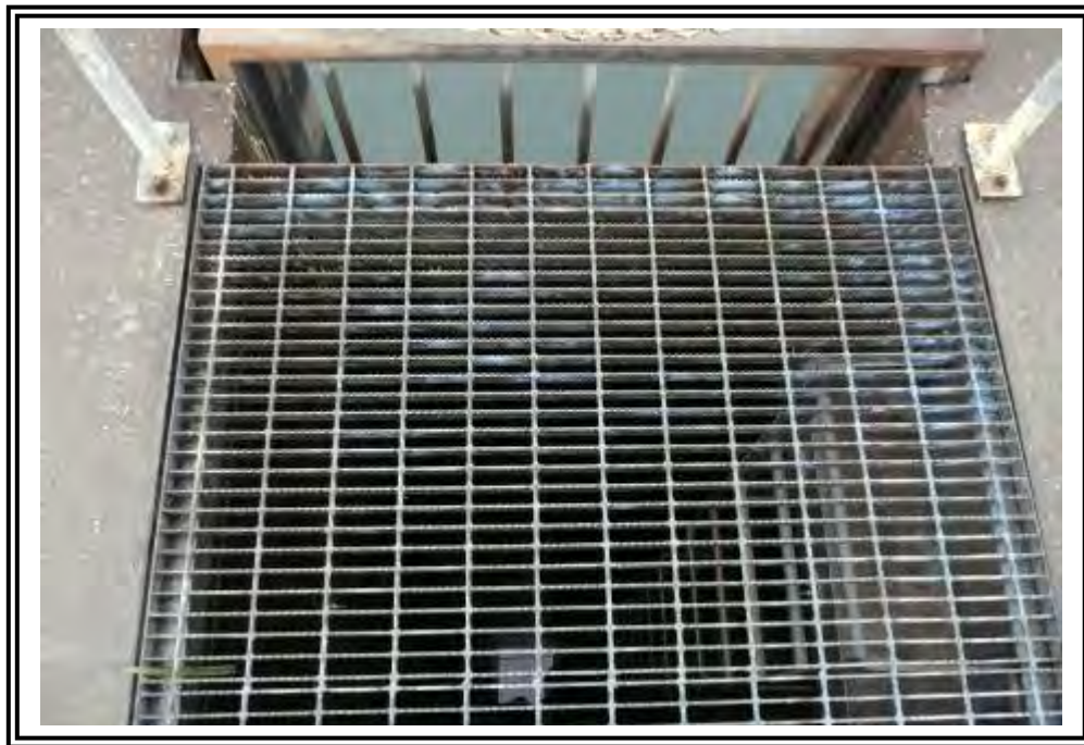
Concrete outfall structure.
