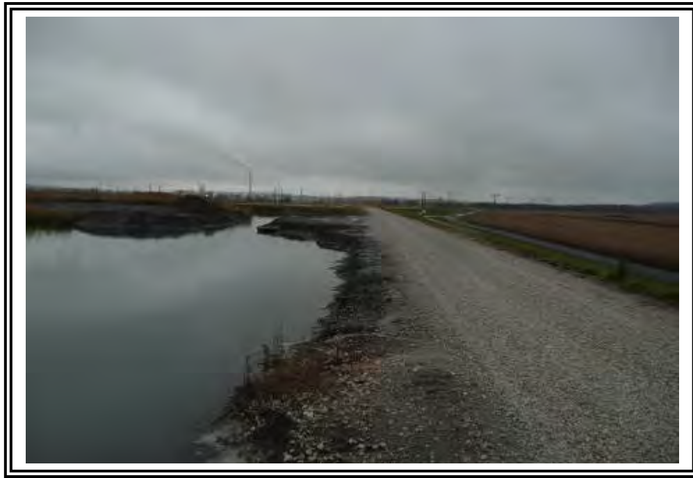
West dike inboard slope and crest, looking south.
