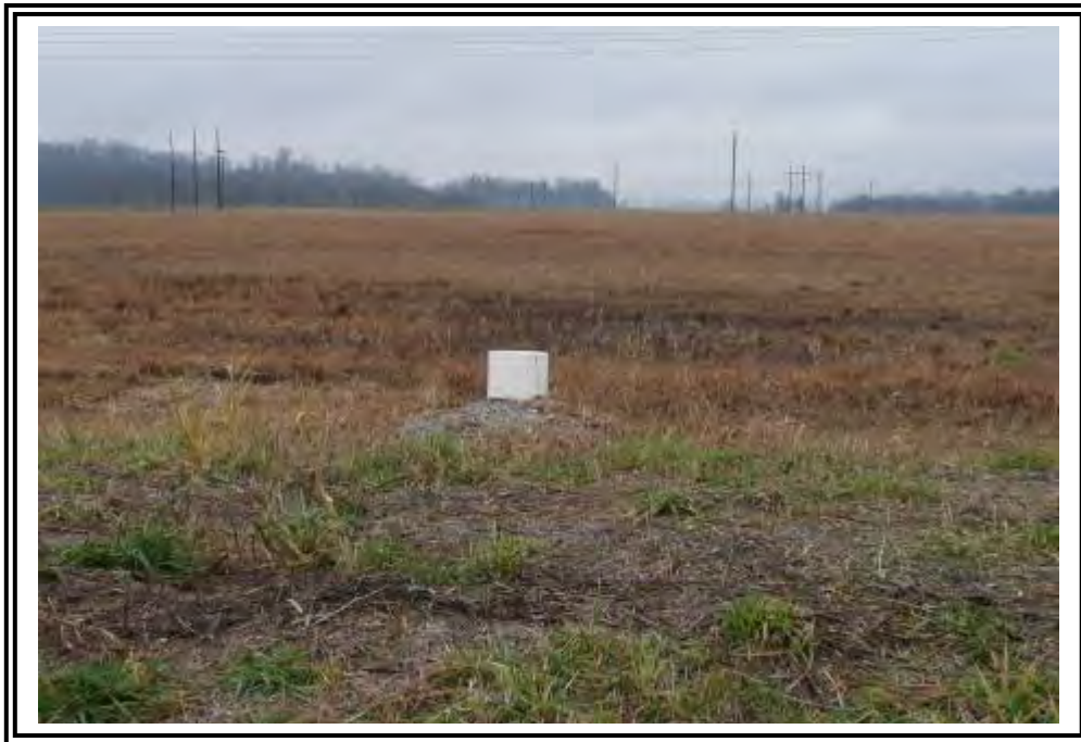
Outlet riser in pond area.
