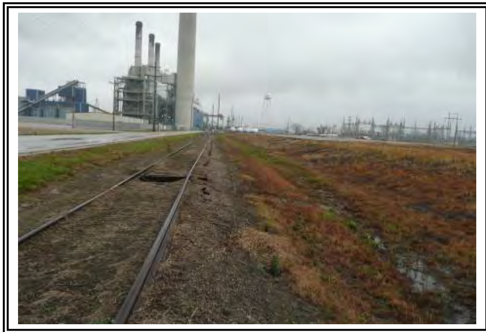
North dike crest area, looking east.
