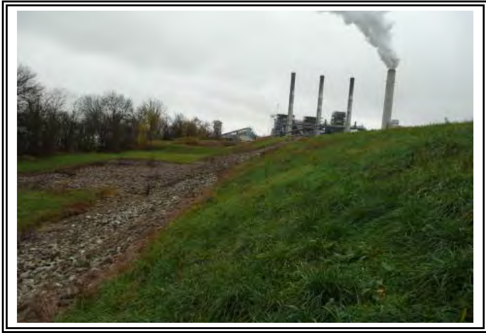
East dike outboard slope, looking south. Note rock toe drain.
