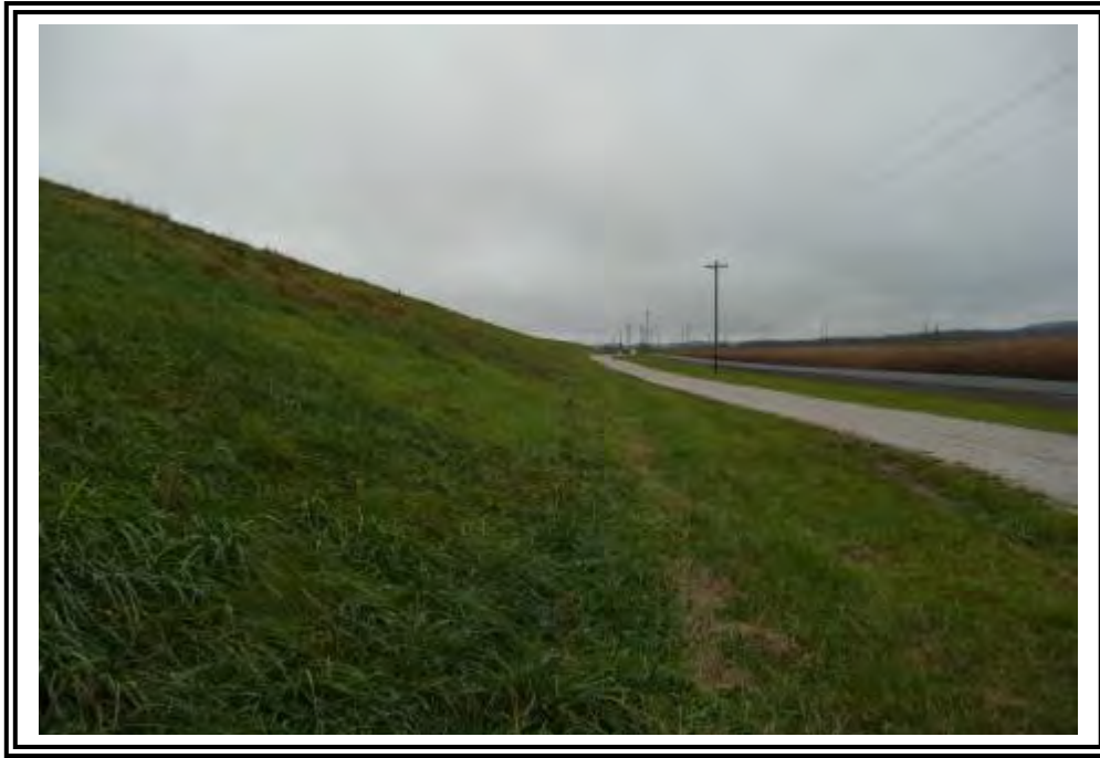
West dike outboard slope, looking south.
