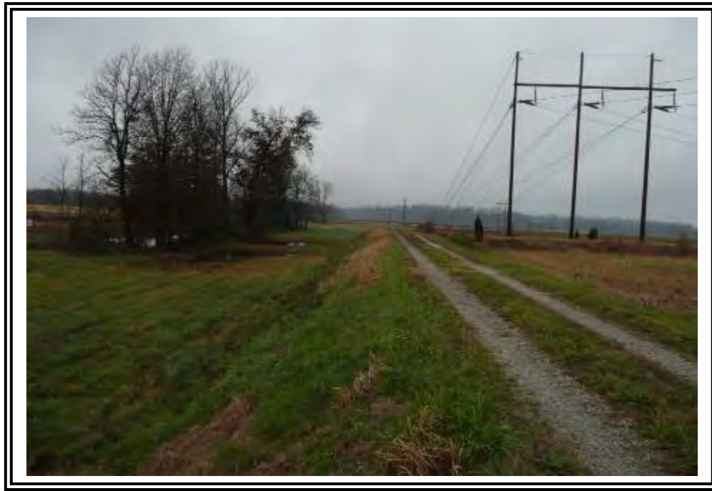
South dike crest area, looking west. Note standing water near toe area.
