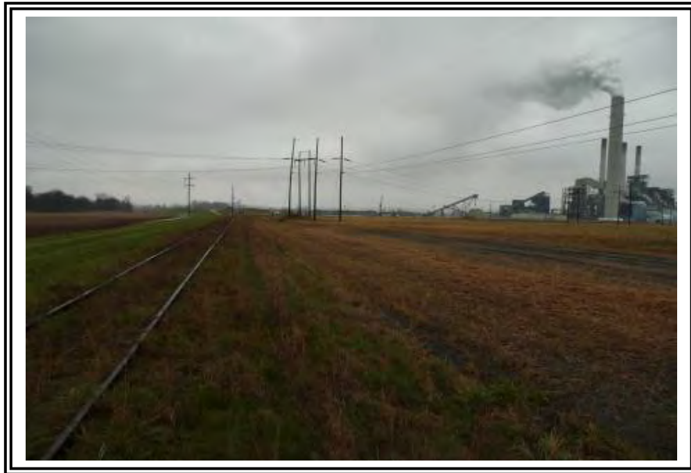
West dike inboard slope, looking north.
