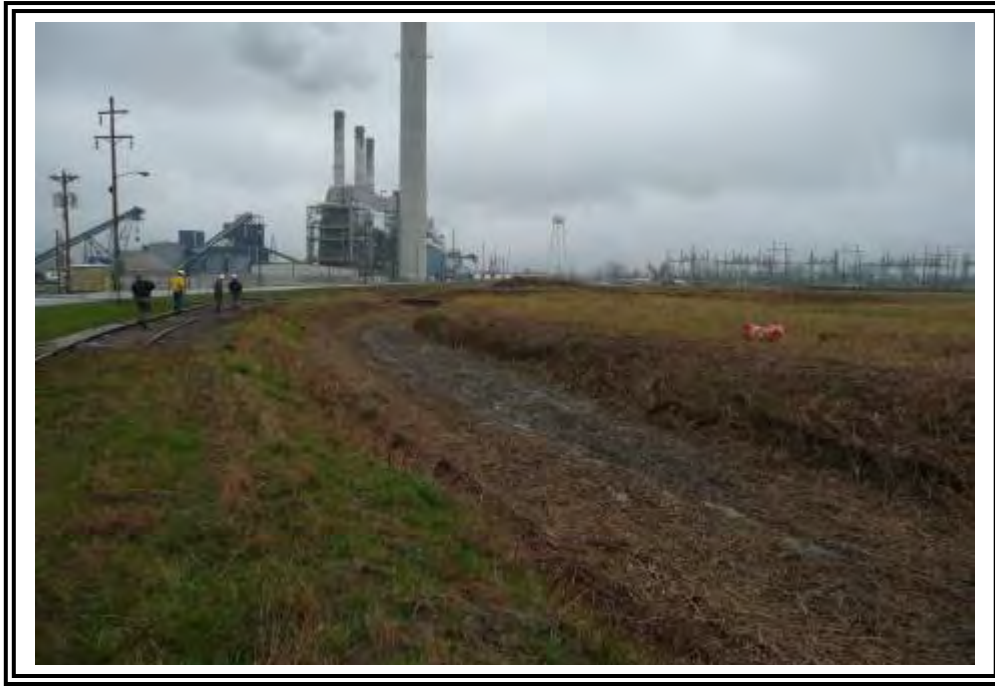
North dike inboard slope, looking east.
