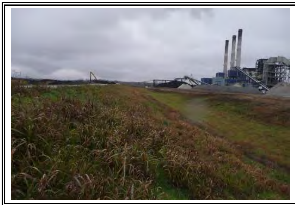
South dike outboard slope, looking east.
