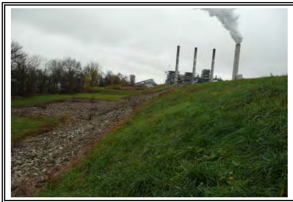
East dike outboard slope, looking south. Note rock toe drain.
