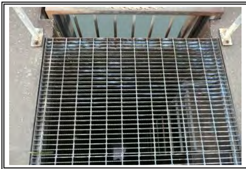
Concrete outfall structure.
