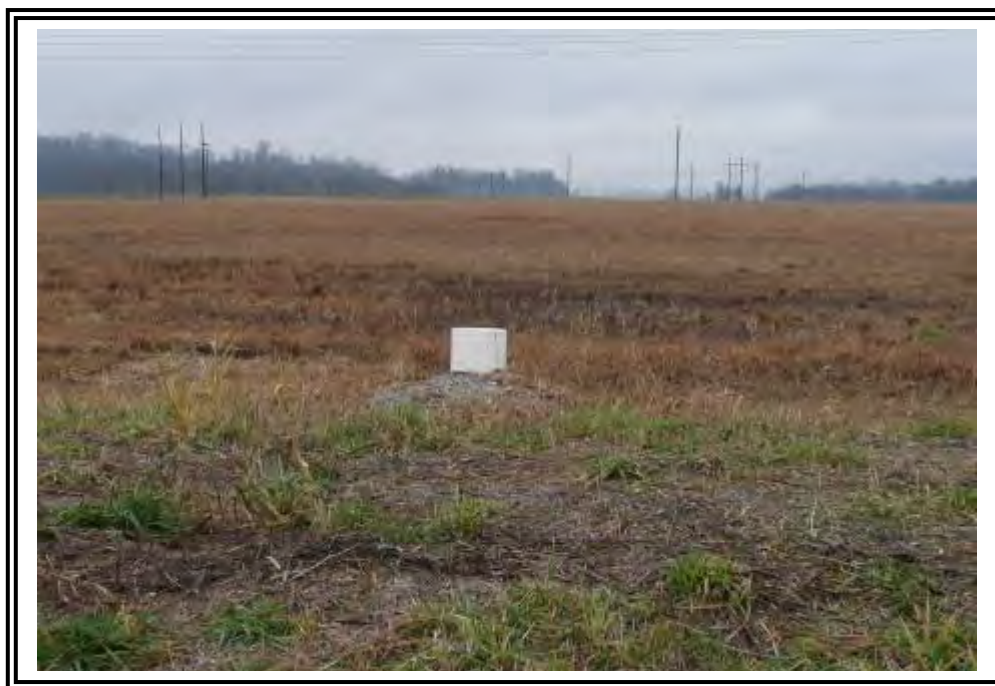
Outlet riser in pond area.
