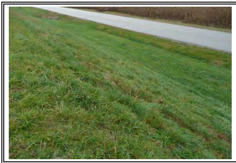
Mowing ruts in surface on west dike outboard slope.
