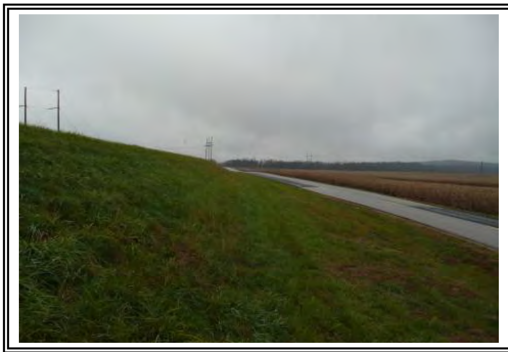
West dike outboard slope, looking south.
