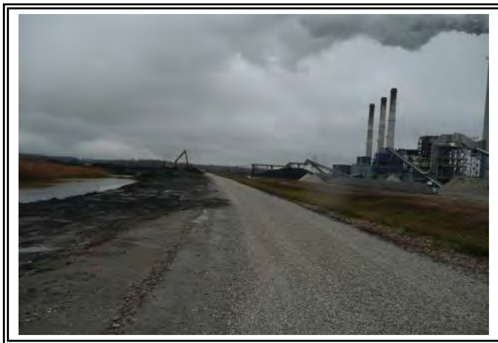
South dike inboard slope and crest at ash processing area, looking east. Note buildup of ash on inboard slope that widens crest area.
