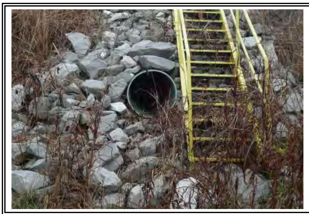
Outlet pipe on south dike.
