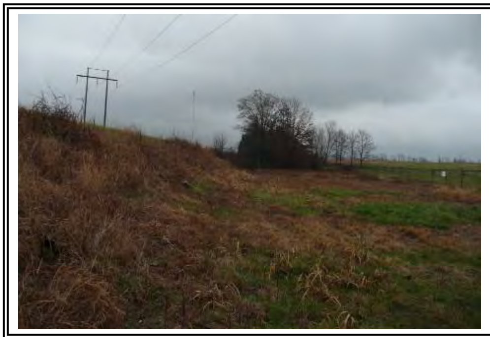
South dike outboard slope, looking east.
