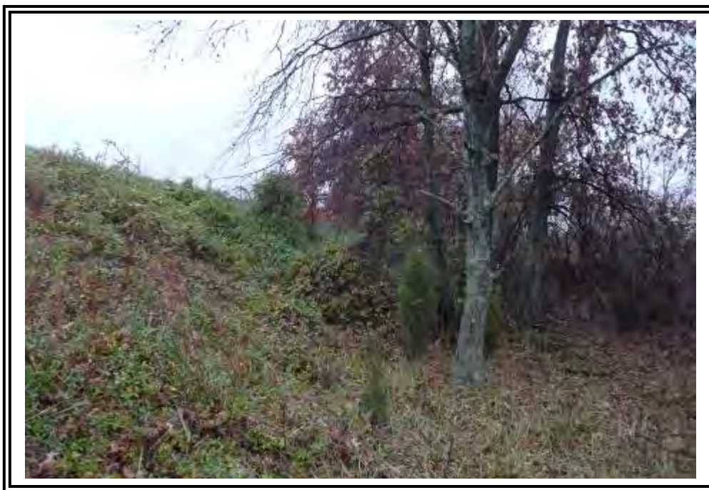
South dike outboard slope, looking east. Note trees and brush vegetation on slope and at slope toe.
