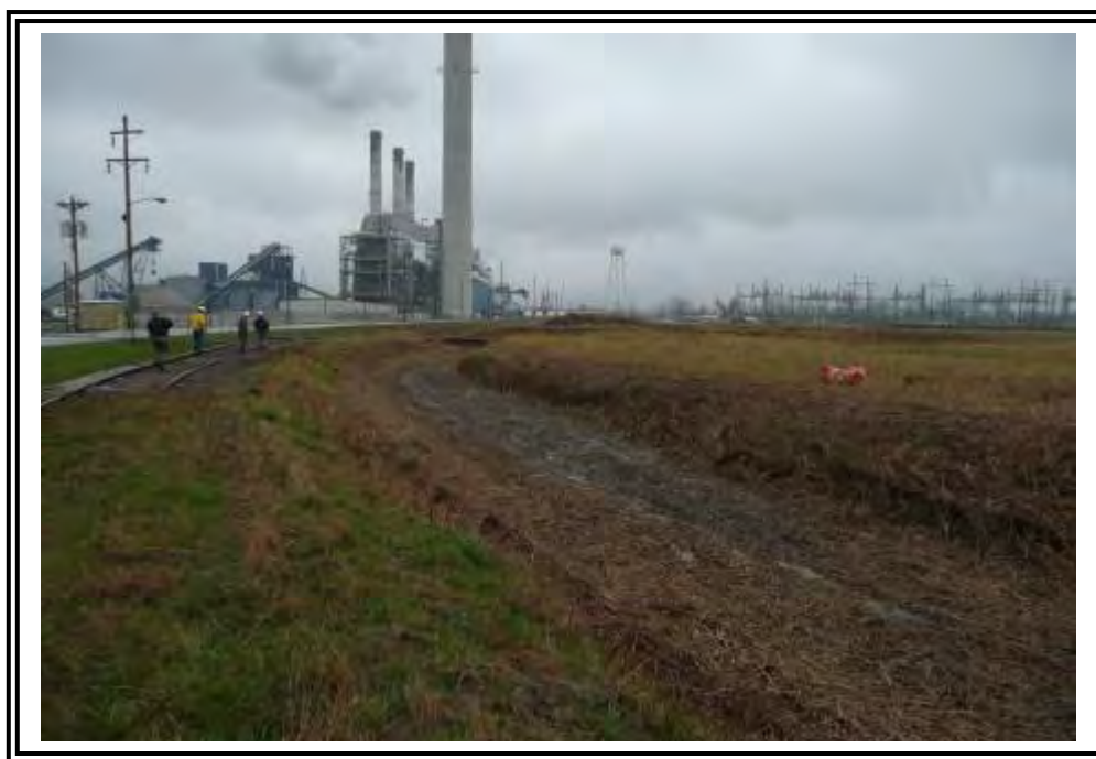
North dike inboard slope, looking east.
