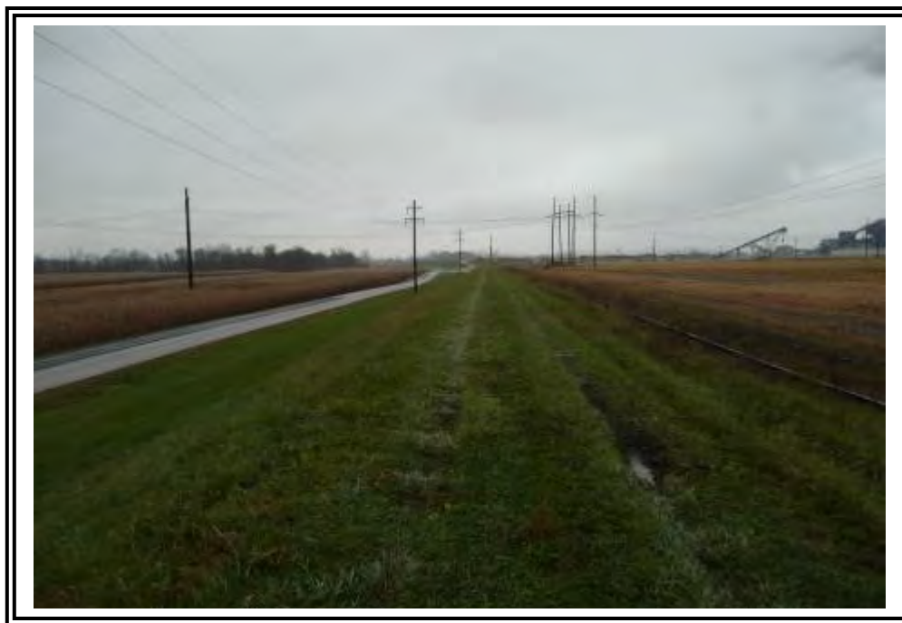
West dike crest, looking north.
