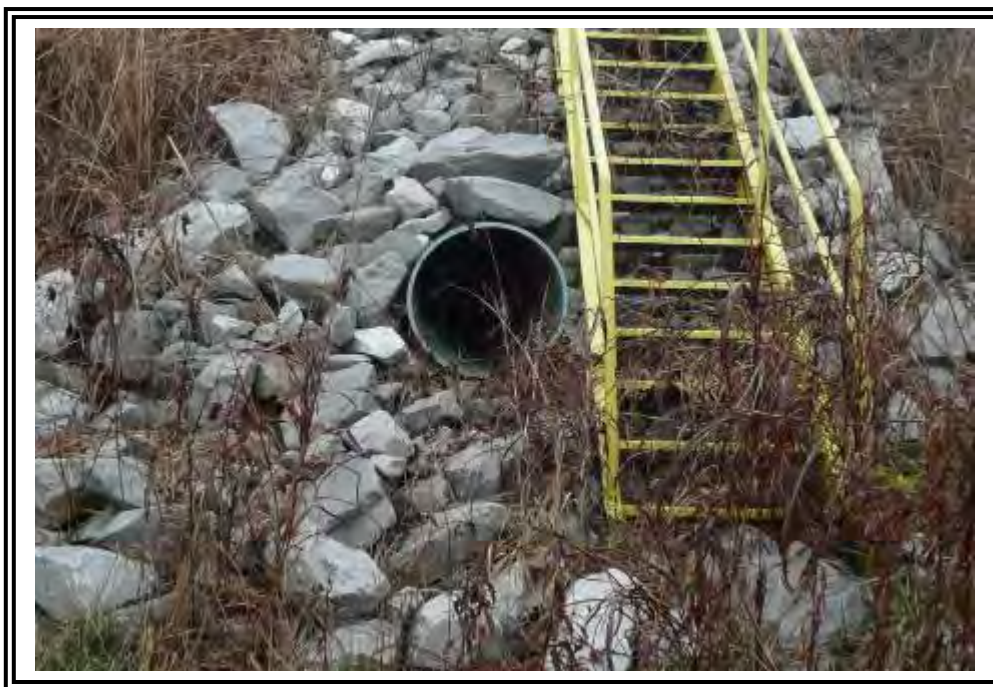
Outlet pipe on south dike.
