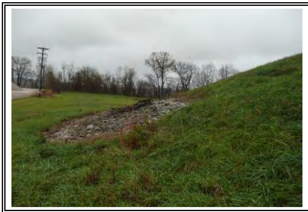
Rock toe drain at northeast corner of Ash Pond A, outboard slope.
