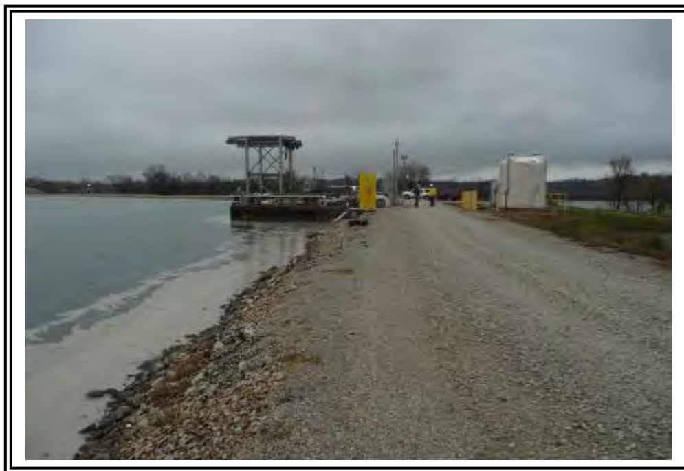
Recycle pump structure dam.
