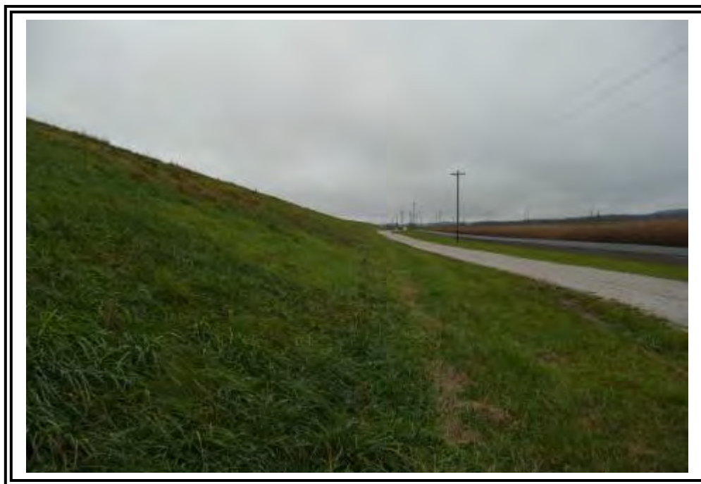
West dike outboard slope, looking south.
