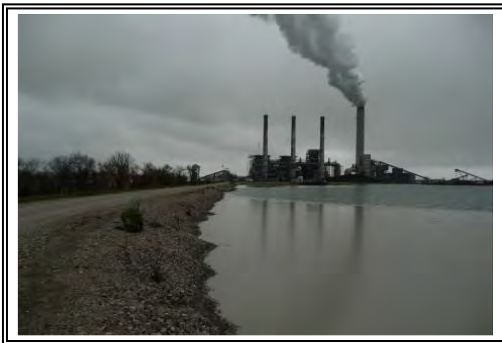
East dike inboard slope with rock surface, looking south. Note isolated woody vegetation.
