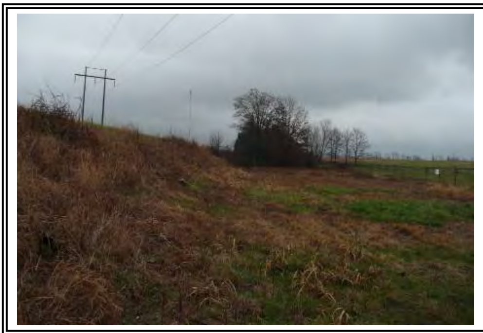
South dike outboard slope, looking east.
