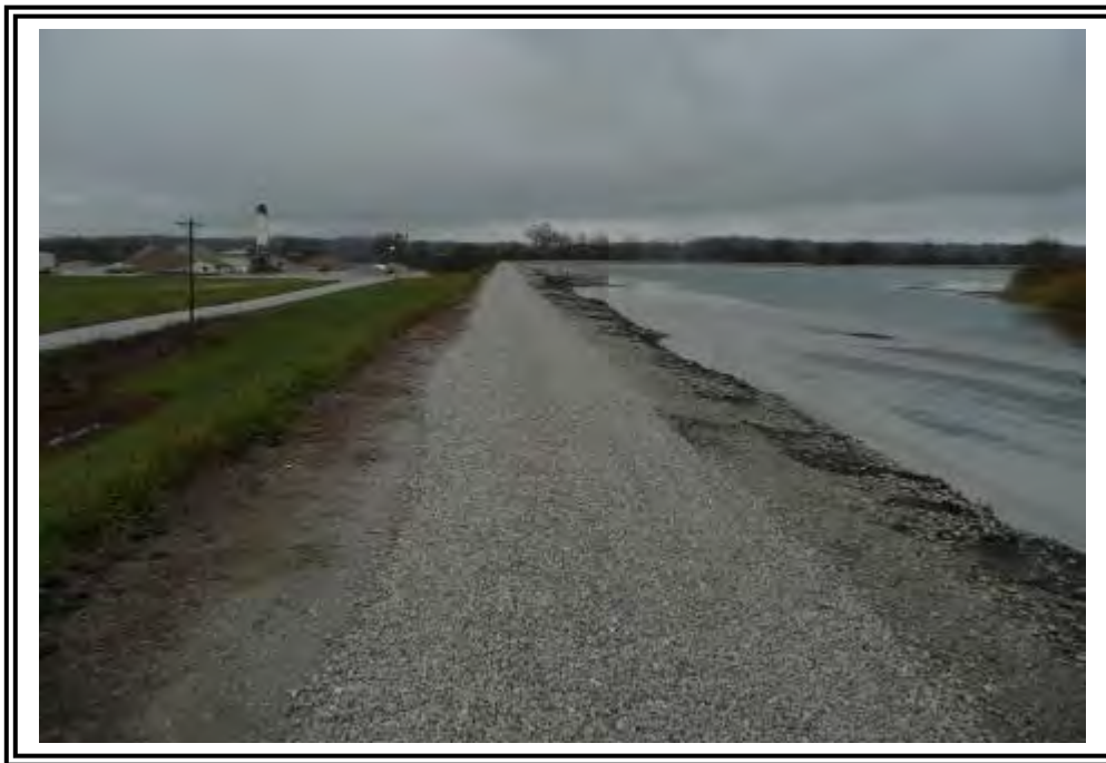
North dike crest looking east. Note wet area at toe of dike to left of photo.
