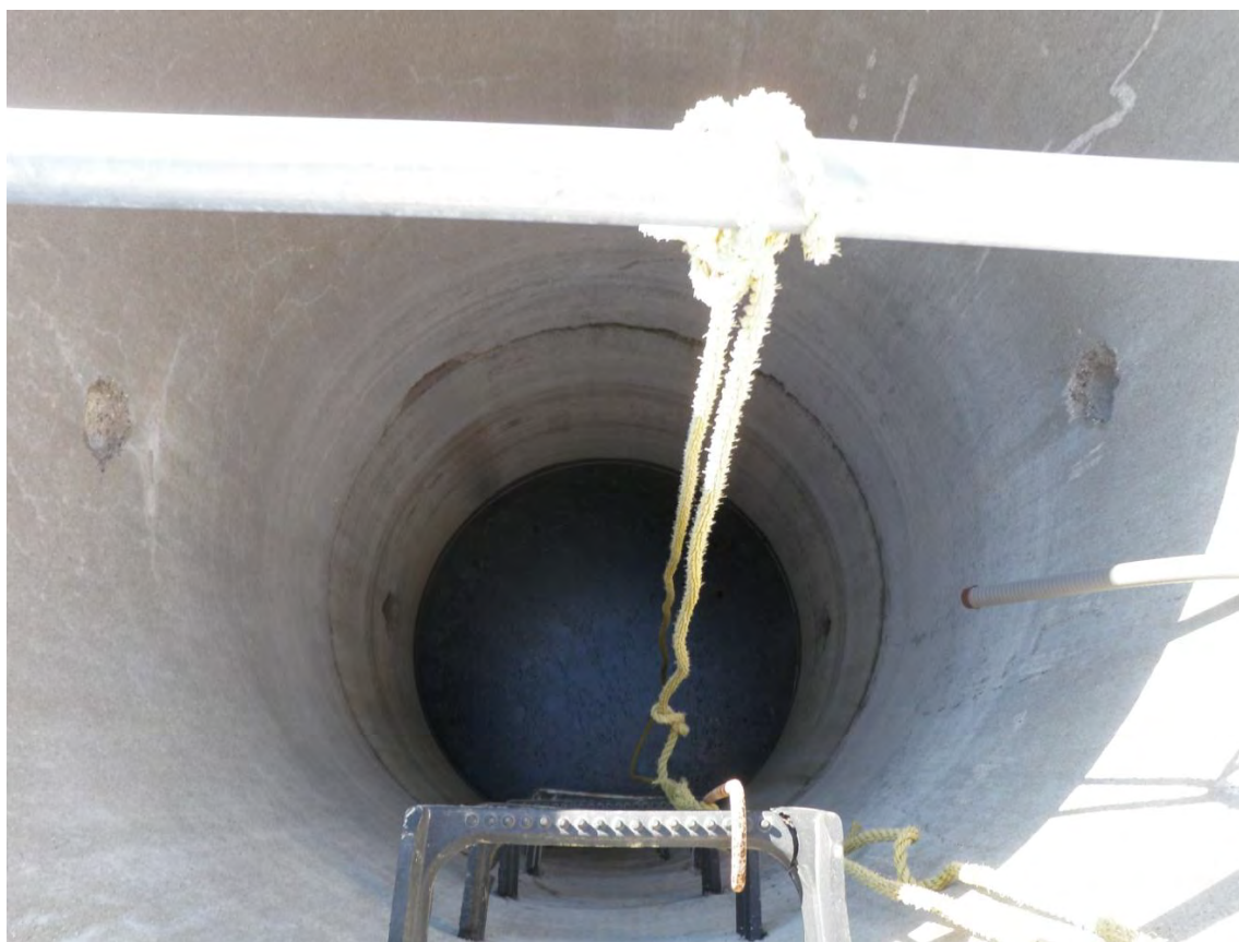
Photo 20: SDA Decantation Pond – Leachate Manhole
