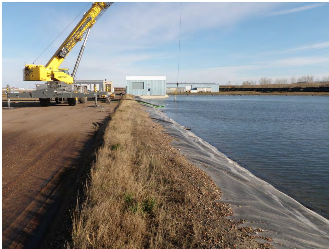
Photo 1: SDA Pond – West dike upstream slope and crest, looking north, note dredging operations
