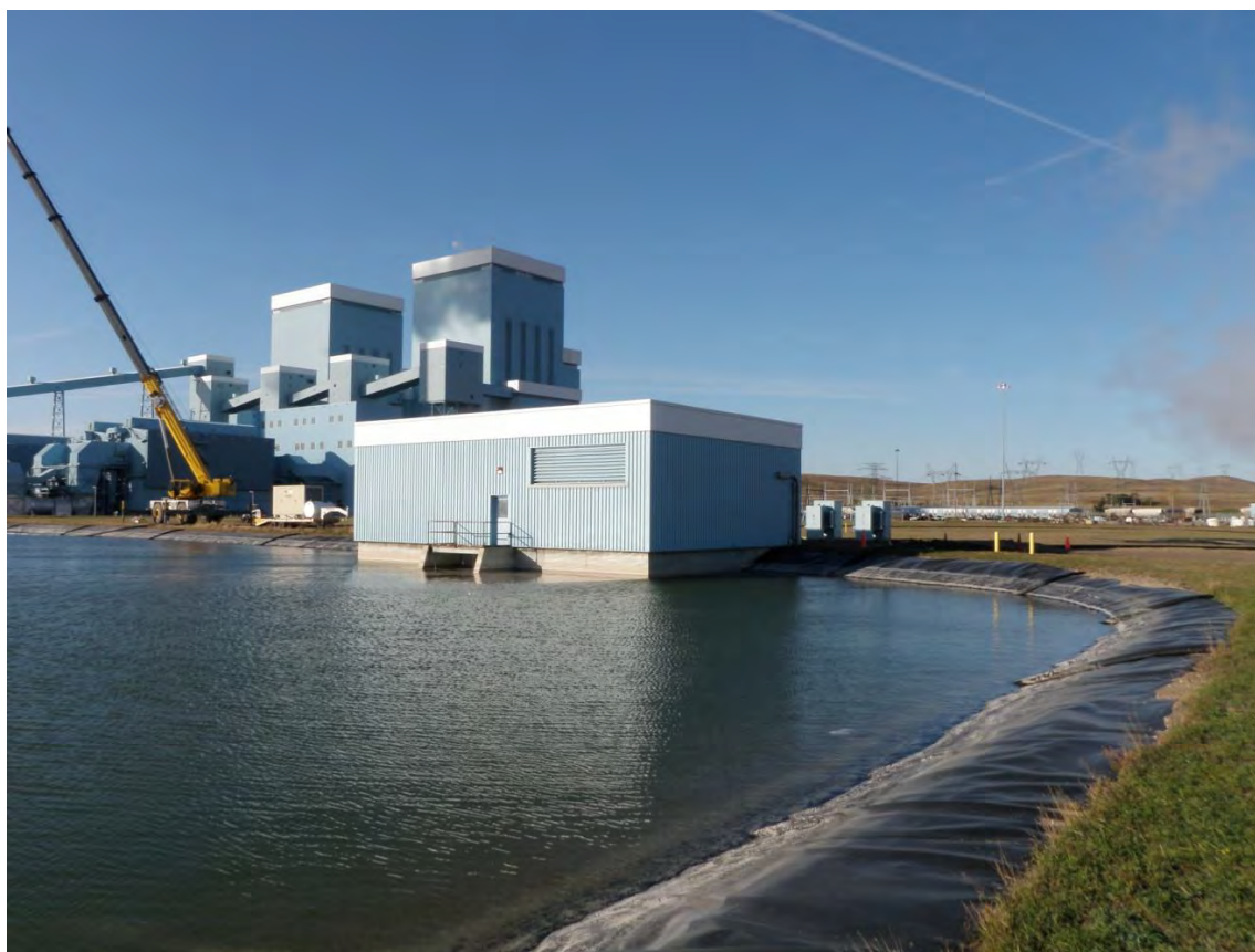
Photo 12: SDA Pond – Pump House, looking southwest
