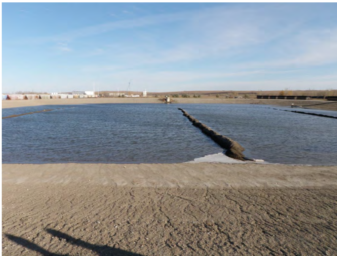
Photo 13: SDA Decantation Pond – Looking north across pond
