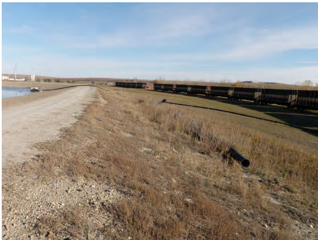
Photo 17: SDA Decantation Pond – East dike downstream slope, looking north, note inlet pipe over dam crest
