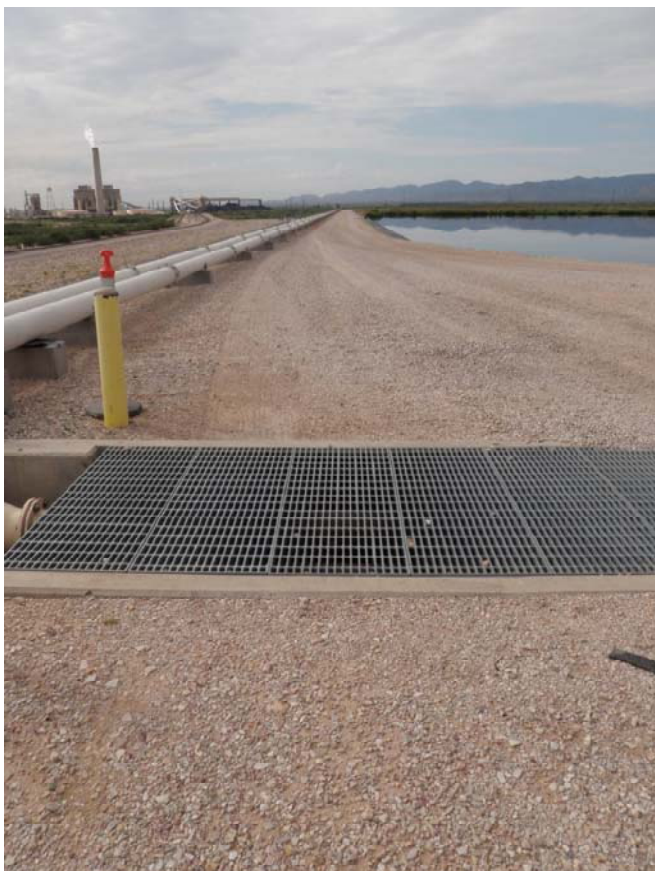
Photo 11: Crest of east embankment of Ash Pond 1 facing south. Pipelines convey slurried fly ash and residuals for disposal in the ash ponds. Note depressed pipe vault for traffic crossing.
