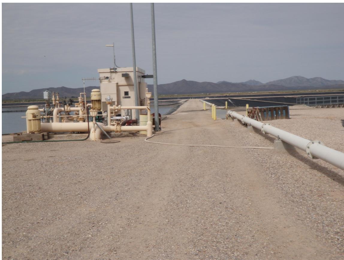
Photo 21: Crest and centralized recirculation pump station located at intersection of Ash Pond 1, 2, 3, & 4, looking west. Decant water is pumped back to the Cooling Tower Blowdown Pond.
