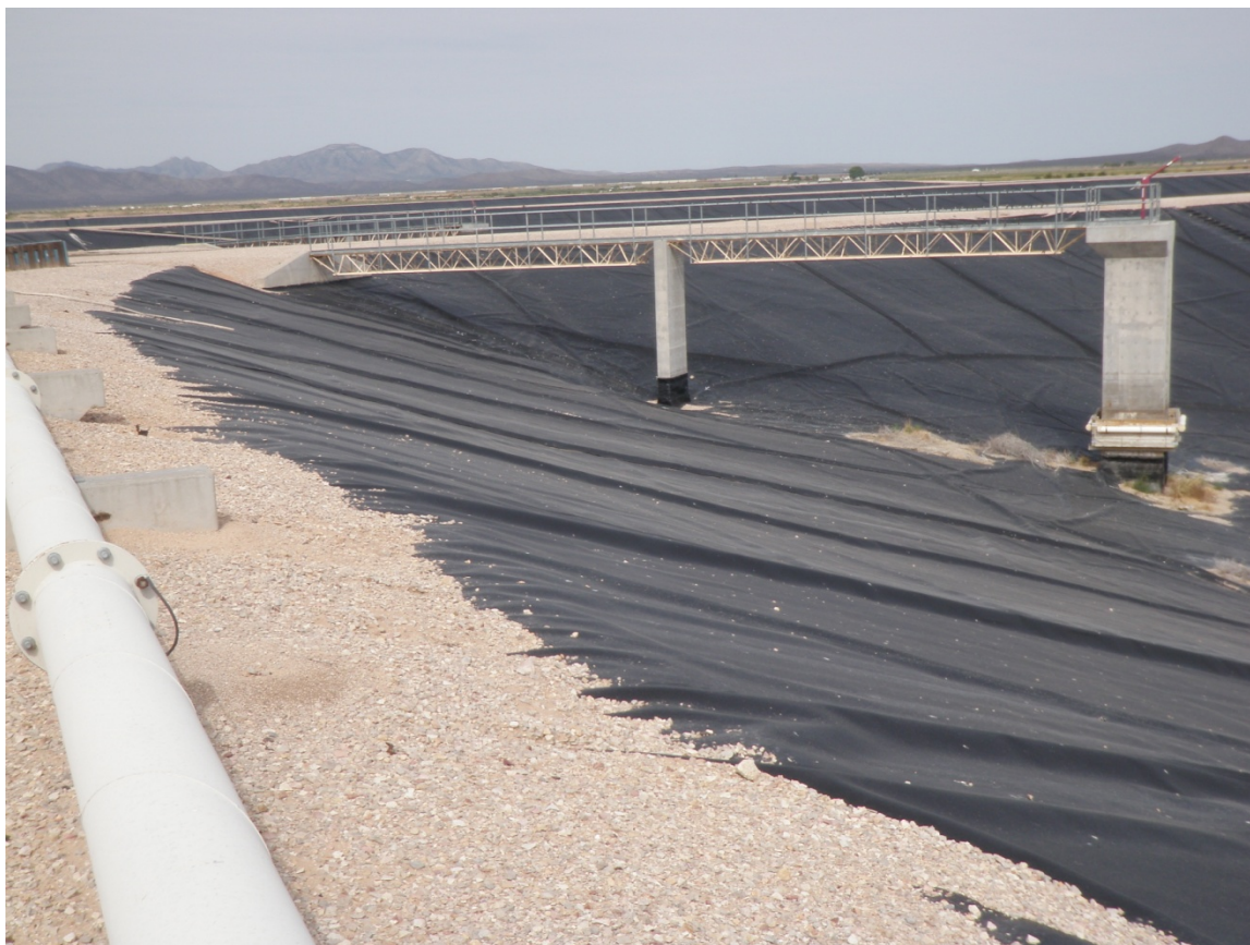
Photo 19: Ash Pond 4 decant drop inlet intake tower and access bridge, looking northwest. Note that Ash Pond 4 is nearly empty.
