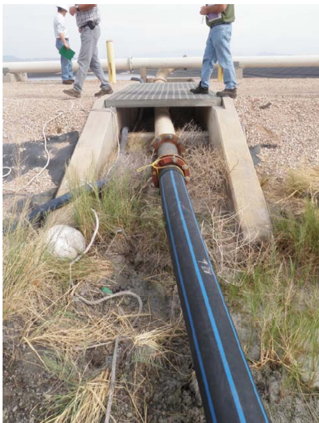
Photo 18: Pipe Vault in crest between Ash Pond 1 and Ash Pond 4 looking north. Note concrete backwall at north end of vault only.
