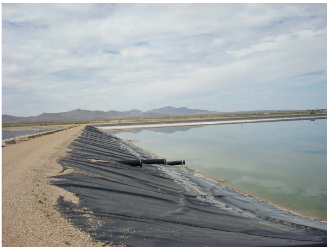
Photo 54: Upstream slope of the south embankment of Scrubber Sludge Pond 2, looking west. Note 3 HDPE pipes that connect Scrubber Sludge Pond 1 and Scrubber Sludge Pond 2. The pipes were closed with blind flanges at each end.
