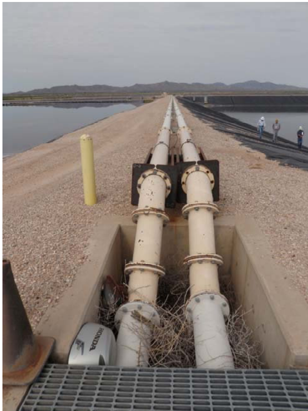
Photo 12: Crest of north embankment of Ash Pond 1 facing west. Note fly ash slurry pipelines.
