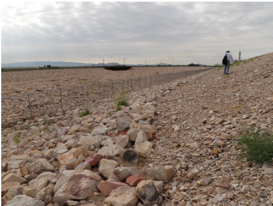
Photo 7: Downstream toe of east embankment of Ash Pond 4 facing south. Note granular rock slope protection and riprap in stormwater ditch at toe.
