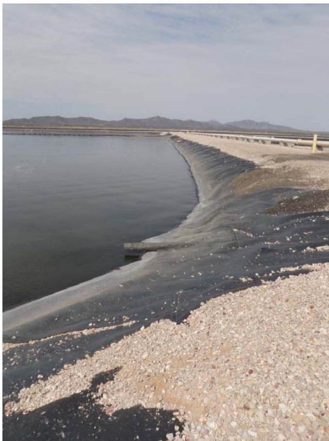
Photo 25: Upstream slope of north embankment of Ash Pond 2, looking west. Note the small pipe that drains a pipe vault.
