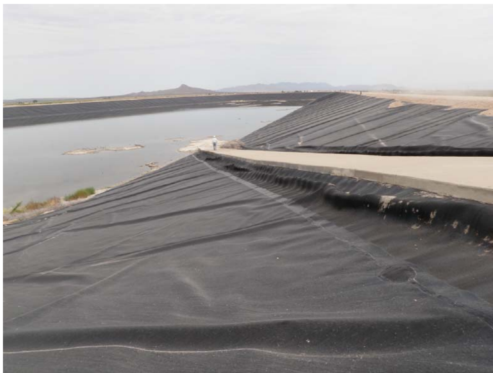
Photo 10: Upstream slope of east embankment of Ash Pond 4 facing north. Note the maintenance access concrete ramp. Pond is nearly empty.
