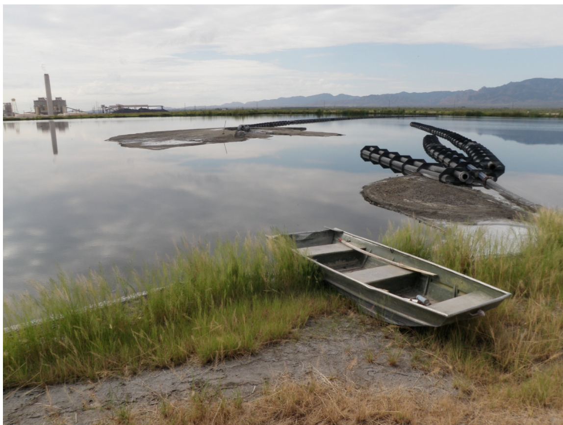
Photo 17: View of broken floating discharge pipe in Ash Pond 1. Occasional breaks occur in the slurried ash and residual discharge pipe due to pressure build-up, possibly associated with clogging.
