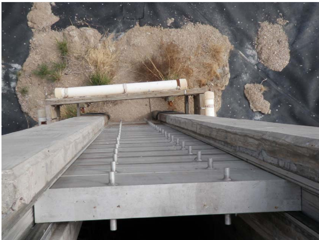
Photo 23: Exterior view of intake tower at Ash Pond 4, looking down. Note the aluminum stop logs that can be adjusted to control pond decant level.
