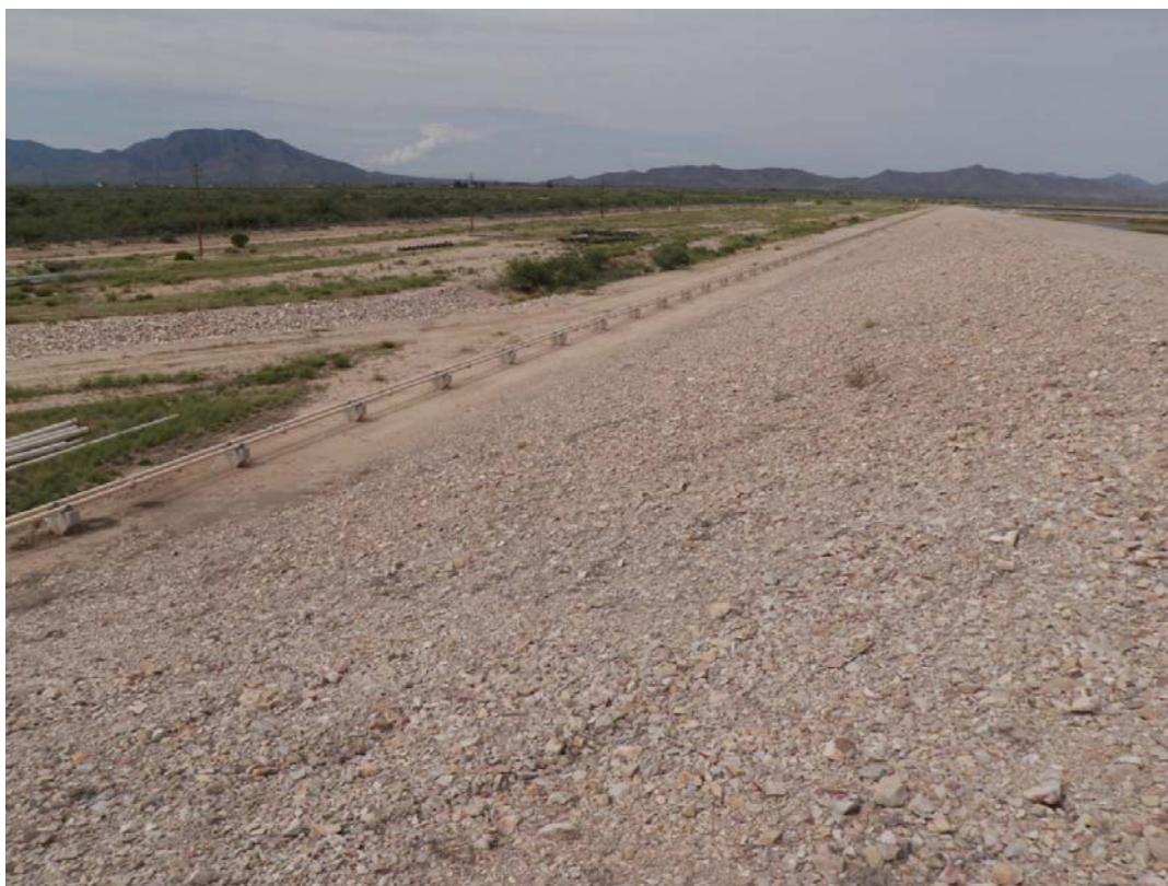
Photo 28: Downstream slope of south embankment of Ash Pond 1, looking west. Note pipes conveying slurried scrubber sludge to Scrubber Sludge Pond 1. Note riprapped stormwater channel located downstream of the embankment.
