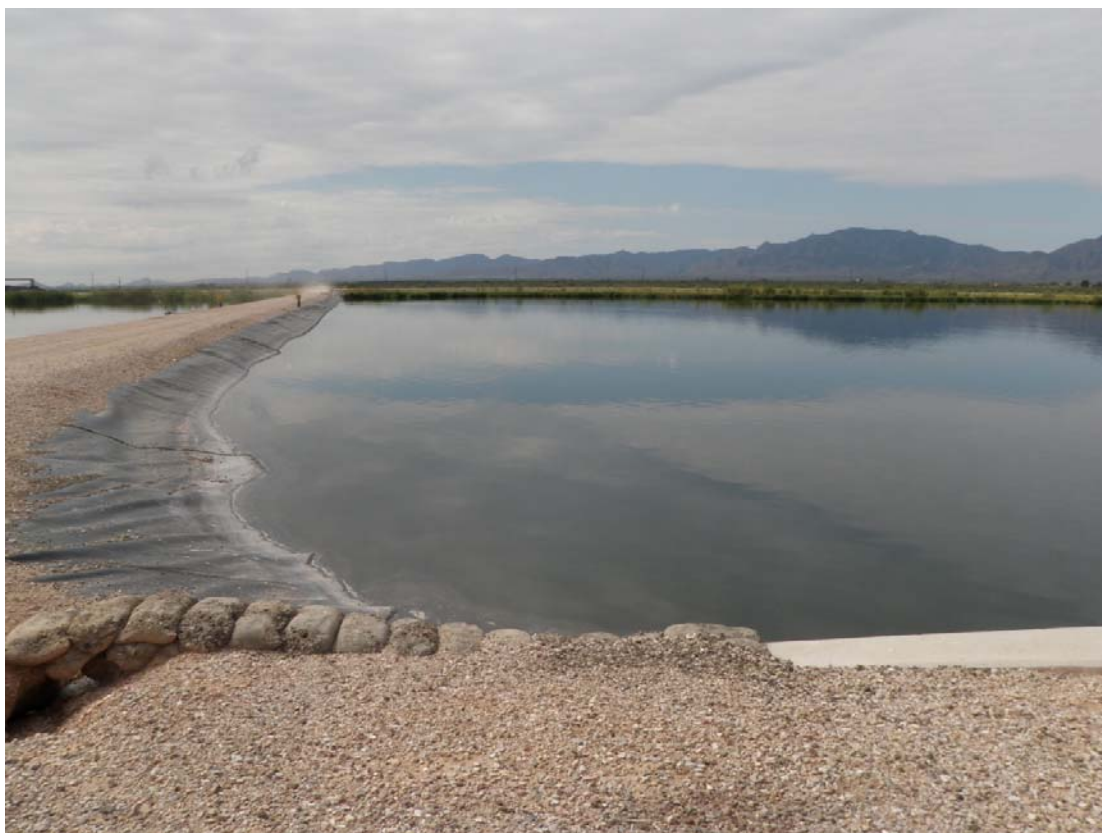
Photo 24: Upstream slope of embankment of Ash Pond 2, looking south. Note erosion of granular crest surface material from behind the wall formed of cement bags.
