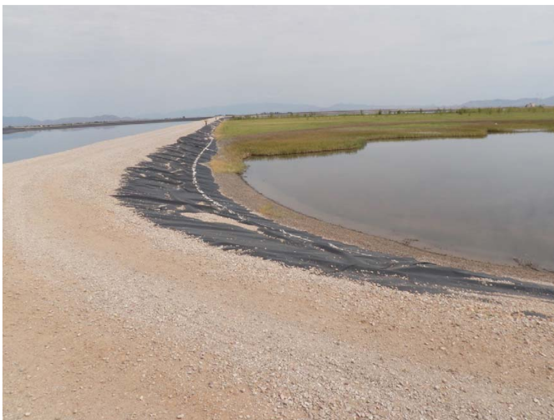
Photo 36: Ash Pond 2, upstream slope, looking north.
