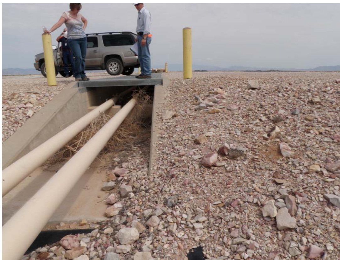
Photo 42: Pipe vault where pipes cross the crest to discharge into Scrubber Sludge Pond 1, looking north. Note the vault lacks a concrete headwall at the downstream end, which could provide a pathway to concentrate discharge of overtopping flows.
