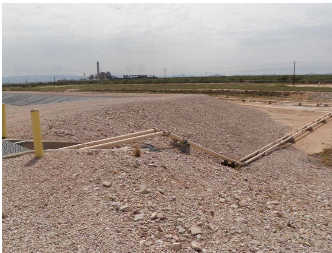
Photo 41: Pipes conveying scrubber sludge entering the facility at southwest corner of Scrubber Sludge Pond 1, looking southeast.
