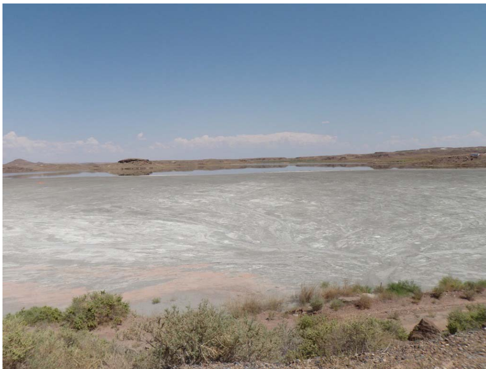
Photo 1: Fly Ash Pond - Overview looking north from embankment. Note downstream fly ash beach.
