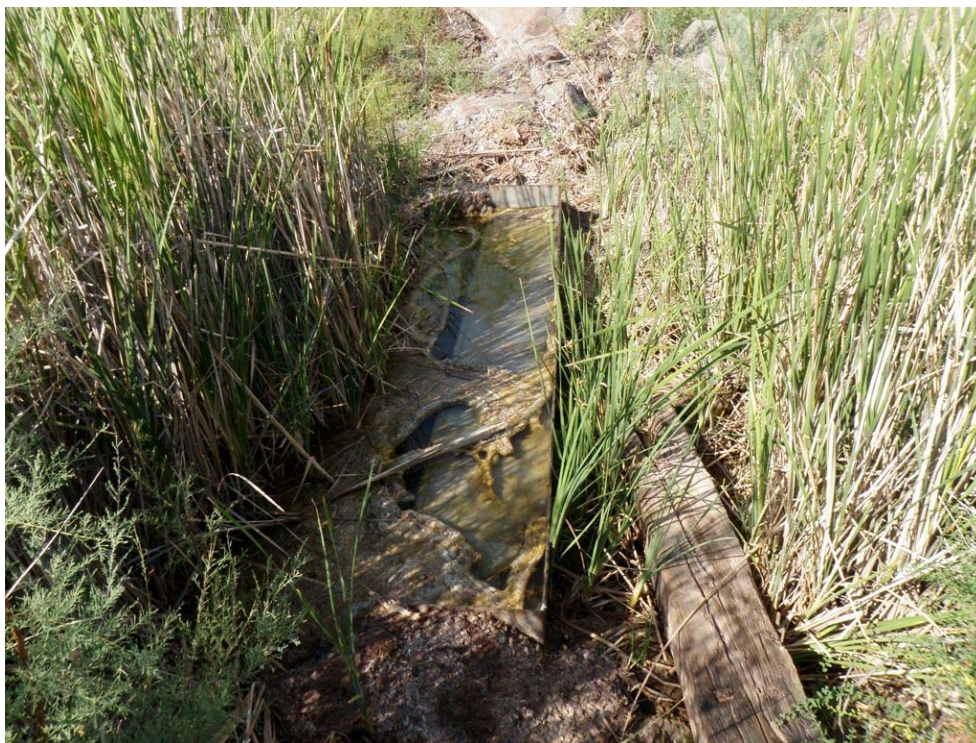
Photo 26: Bottom Ash Pond - Weir at West Abutment Seep.
