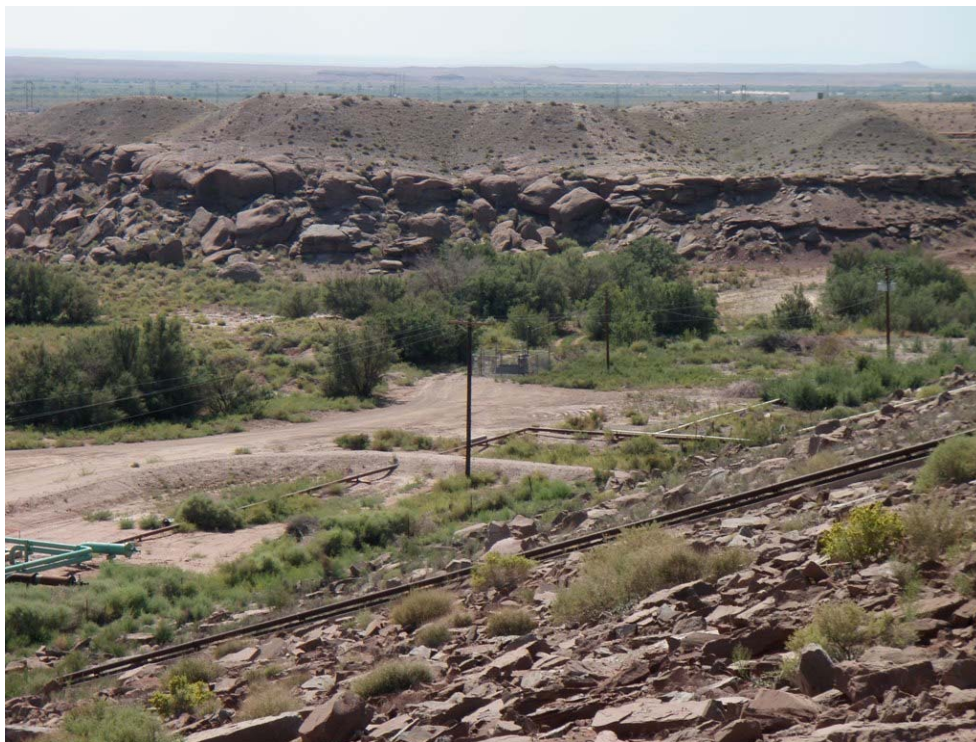
Photo 25: Bottom Ash Pond - West Abutment Seep from embankment crest. Siphon pipes (center) and siphon collection system (lower left) are also visible.
