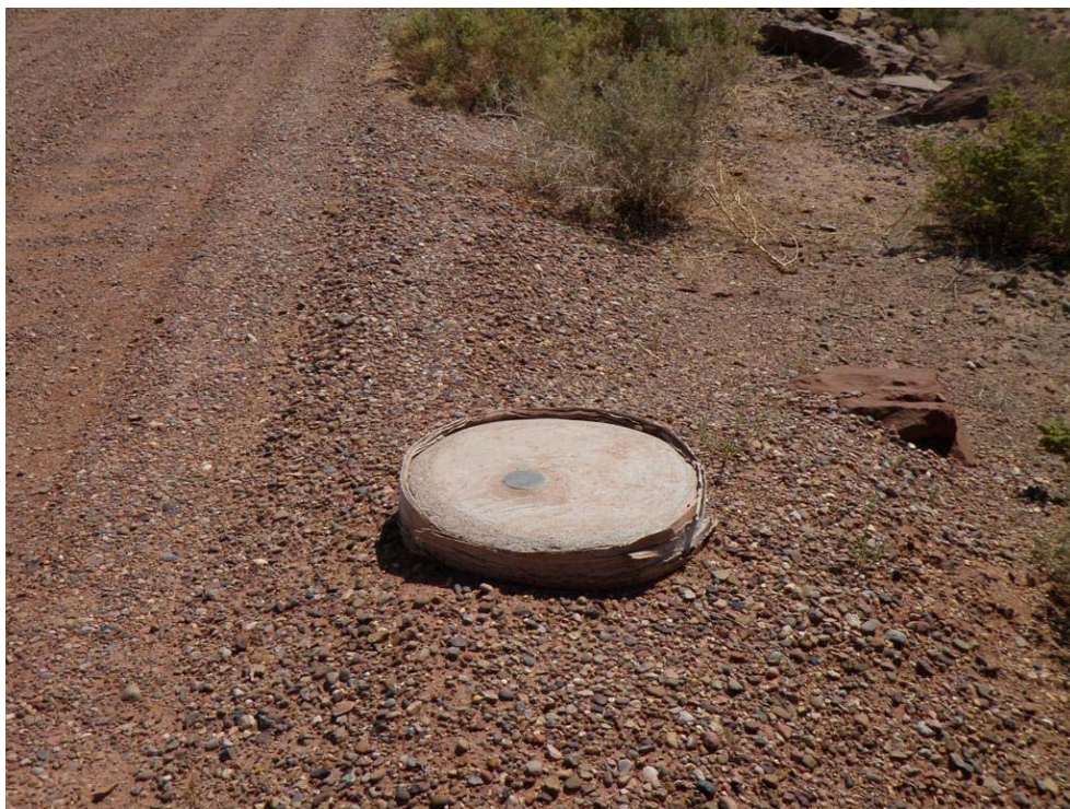
Photo 3: Movement monument on Fly Ash Pond Dam.
