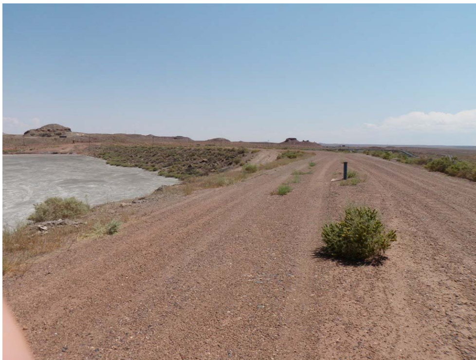
Photo 4: Crest of Fly Ash Pond Dam with piezometer, looking east at bend in embankment.
