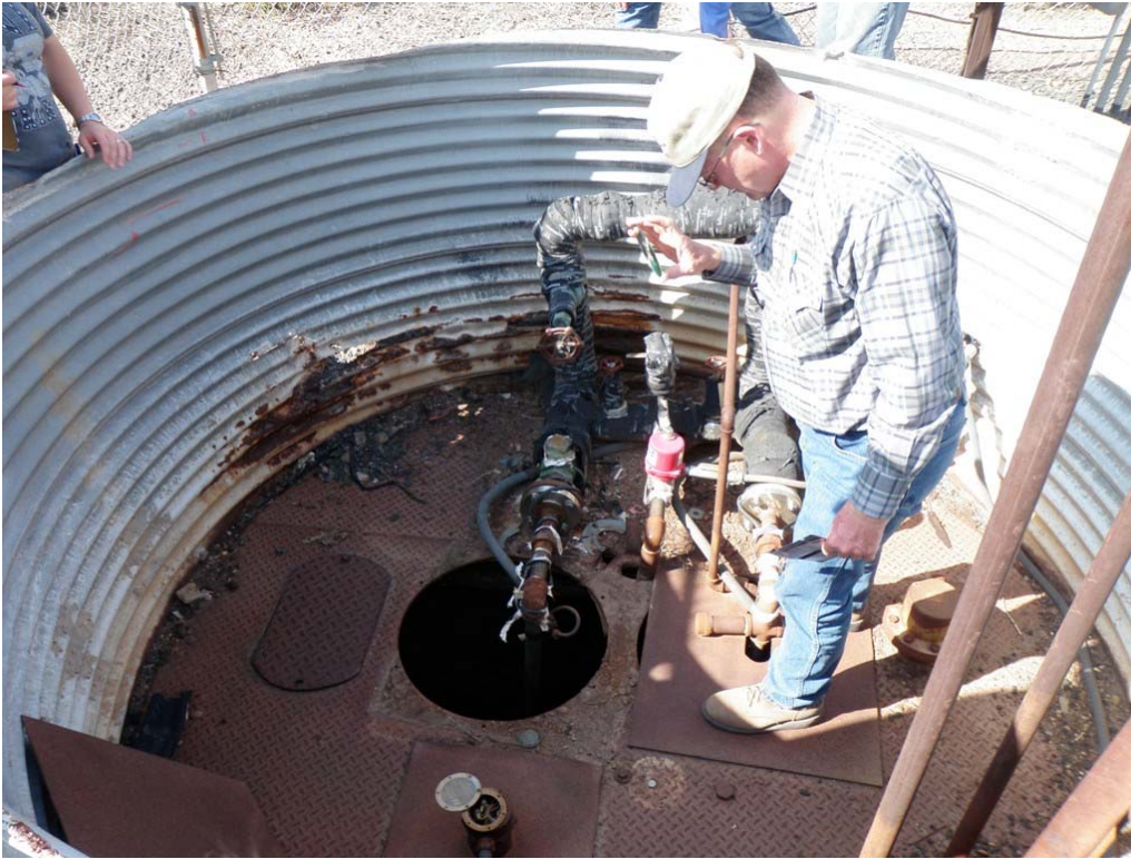
Photo 27 – Bottom Ash Pond: Seepage collection system at West Abutment Seep.
