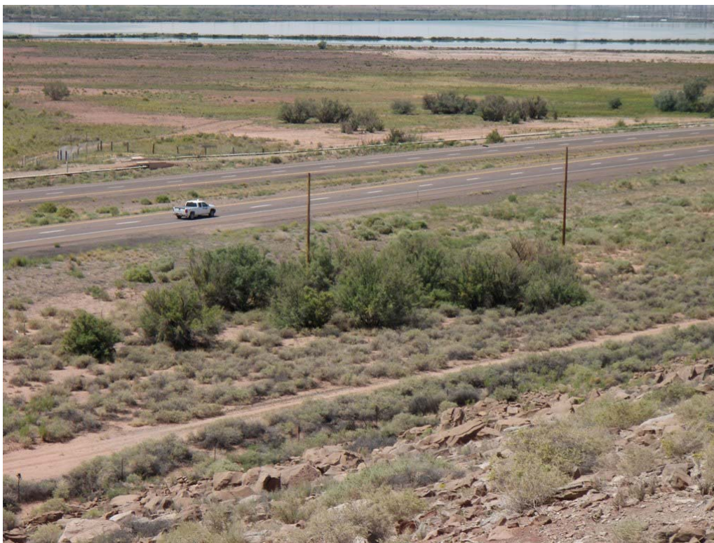
Photo 20 – Fly Ash Pond: Tamarisks near downstream toe indicating seepage.
