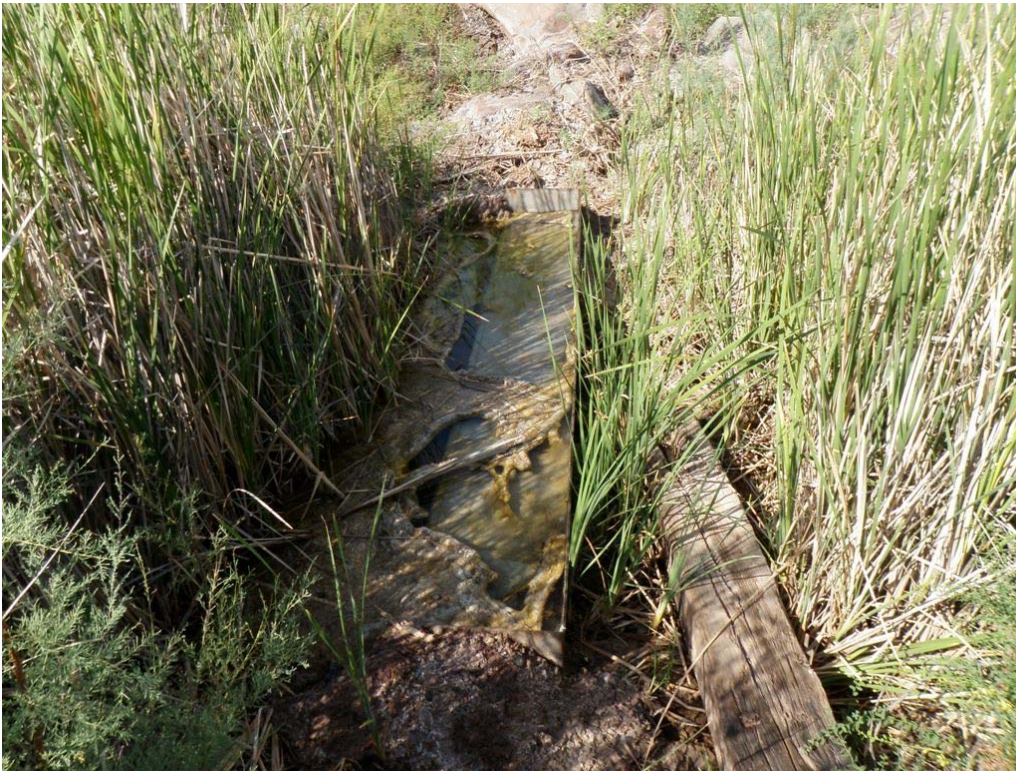
Photo 26 – Bottom Ash Pond: Weir at West Abutment Seep.
