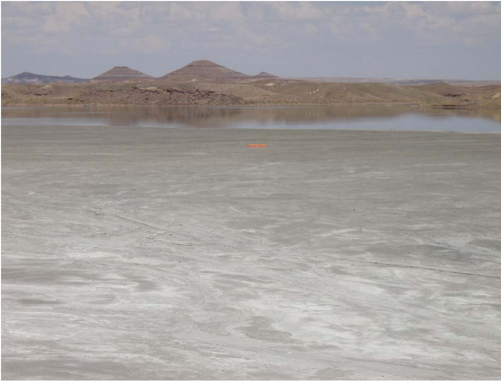
Photo 35 – Fly Ash Pond: Buoy marking 300-foot distance from area where cracks were observed in embankment crest. Fly ash beach must extend upstream of this distance.
