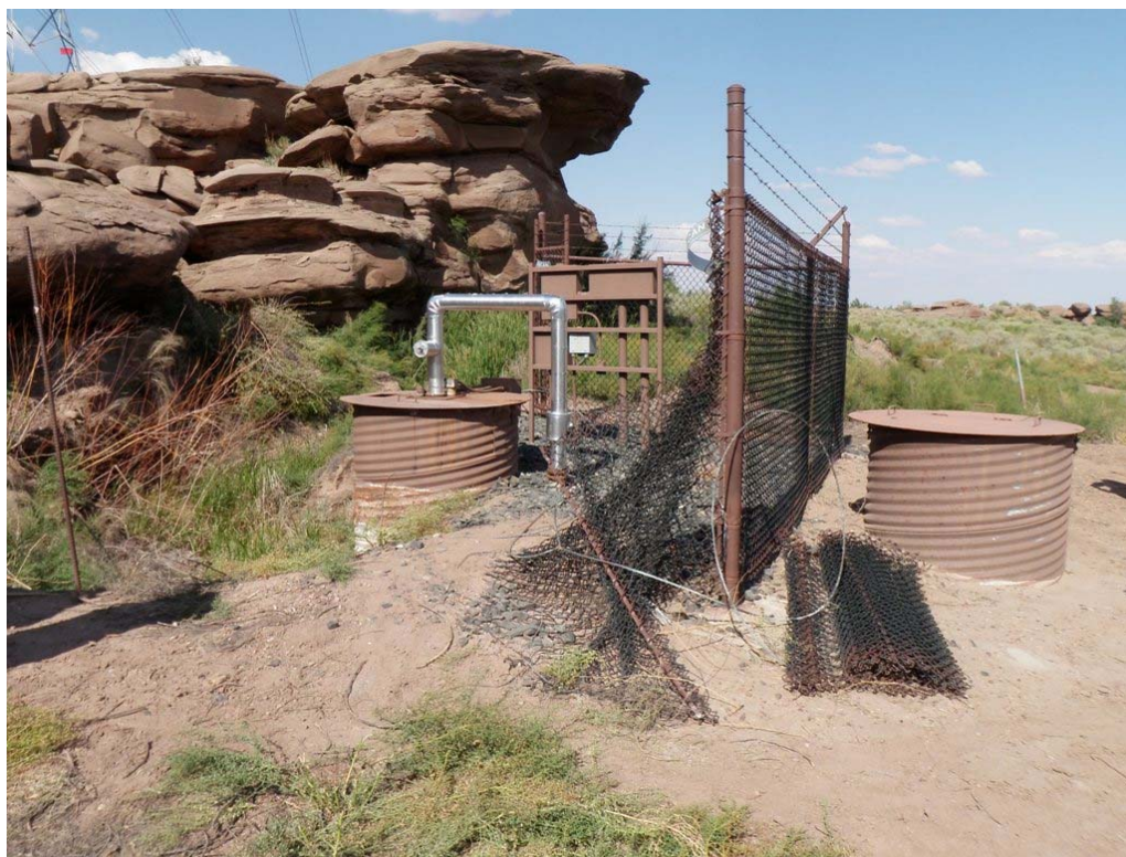
Photo 33 – Bottom Ash Pond: Seepage collection system for Petroglyph Seep.
