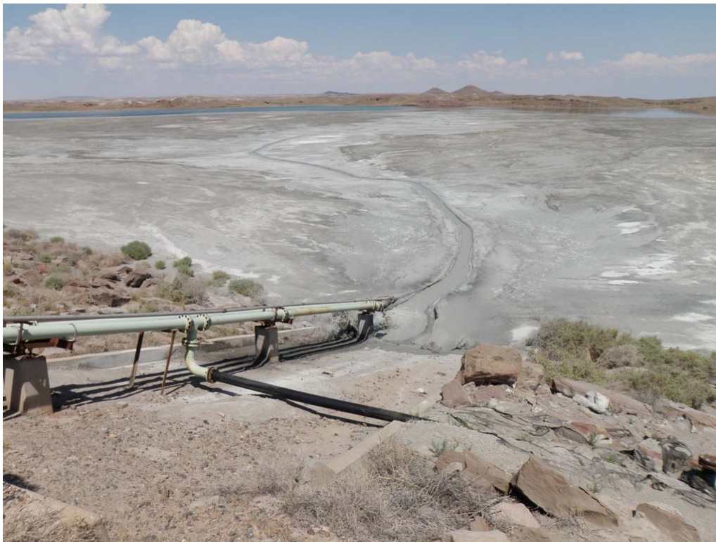
Photo 6 – Fly Ash Pond Dam: Slurry discharge point on upstream face.
