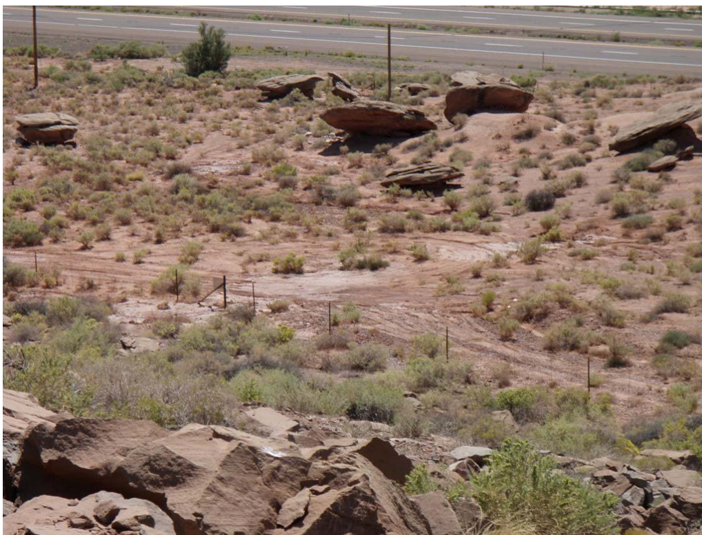
Photo 19 – Fly Ash Pond: Salt patch associated with seepage near right abutment toe (known as the “Hoodoo Salt Patch”).
