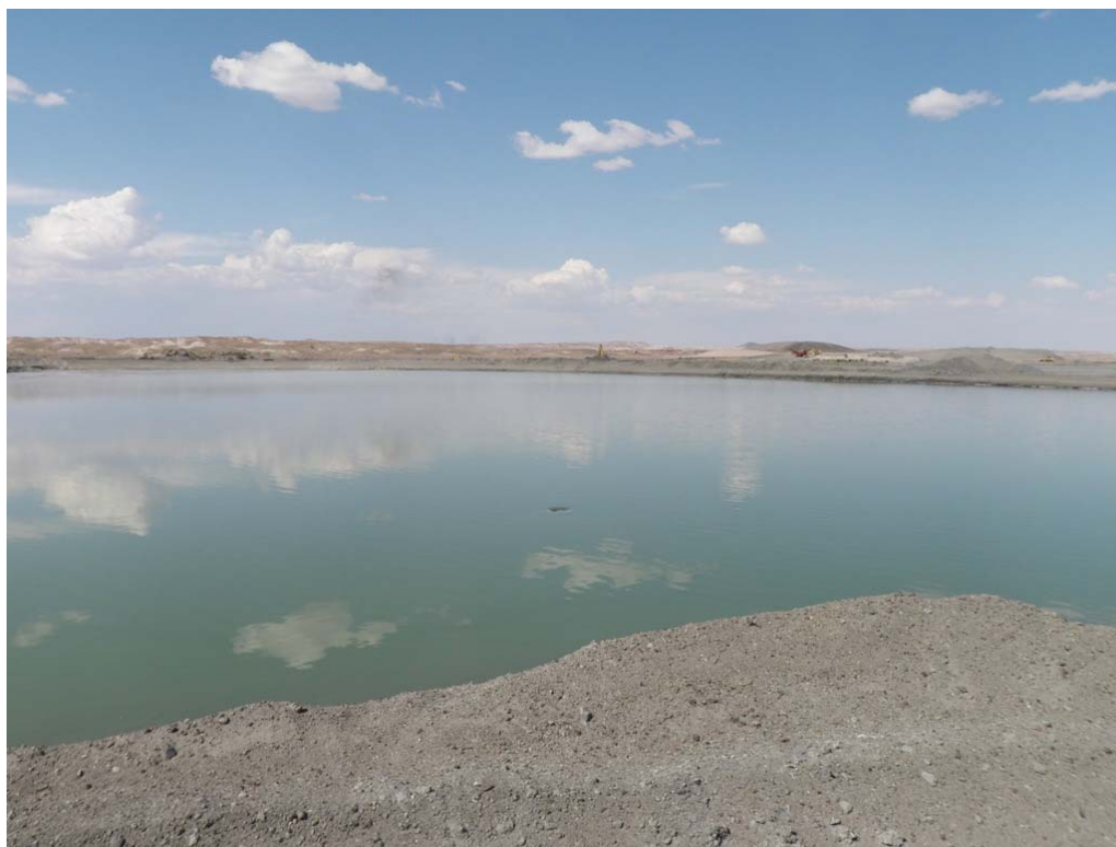
Photo 12 – Bottom Ash Pond: West cell, which is currently being filled with bottom ash slurry. Note vortex through which water flows to main reservoir.
