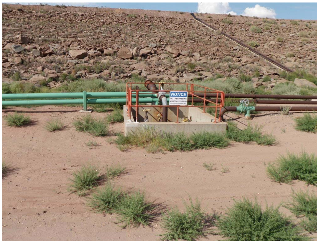
Photo 39 – Bottom Ash Pond: Siphon pipes extending along downstream slope, and siphon collection station.
