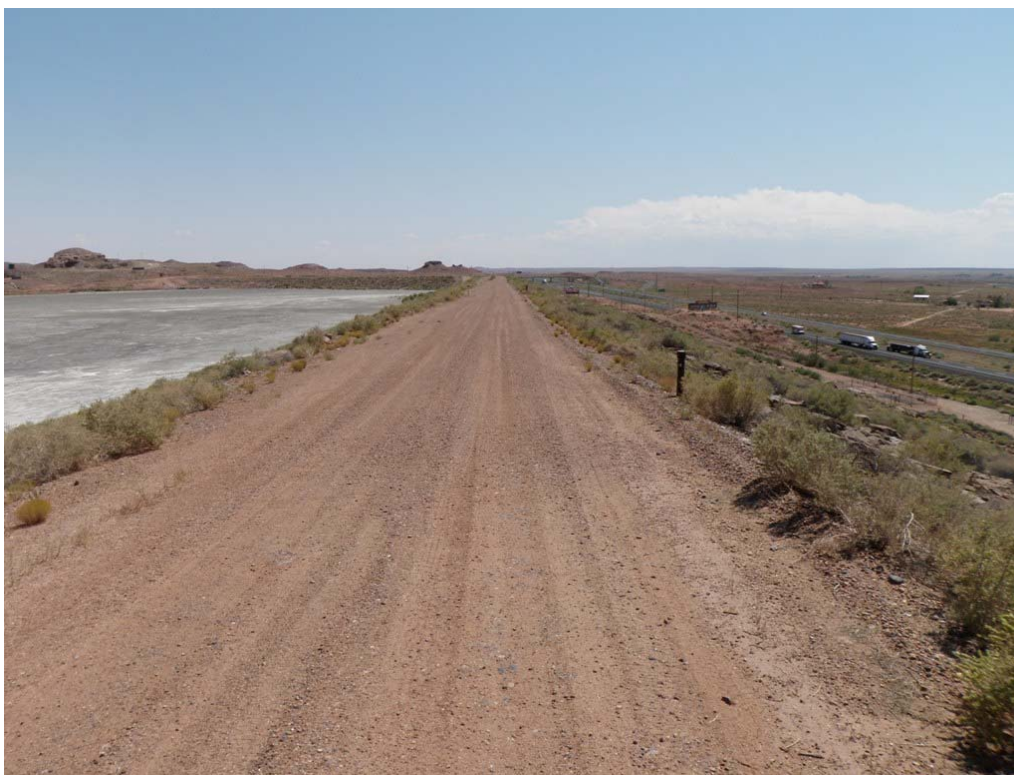
Photo 2 –Fly Ash Pond Dam: Crest of embankment with dirt road, looking east.
