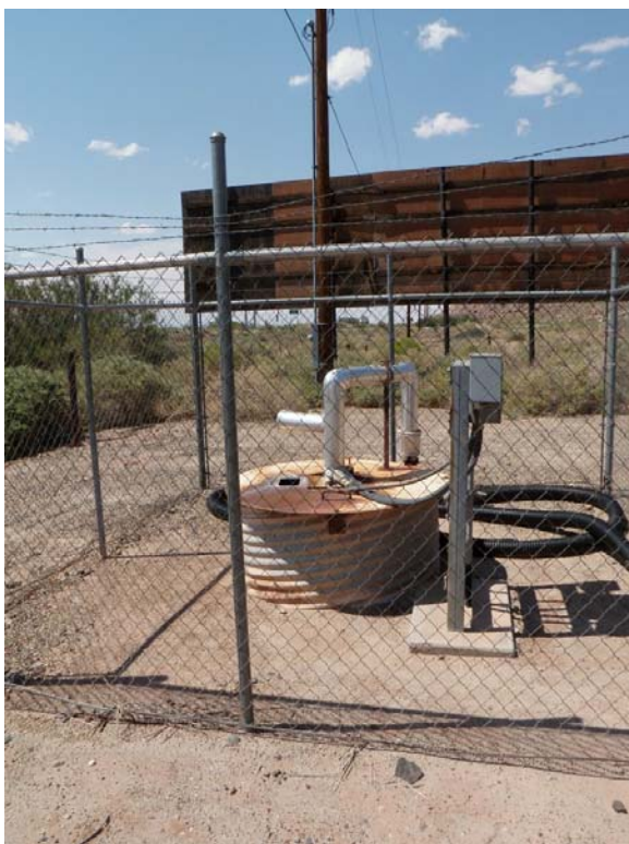
Photo 23 – Fly Ash Pond: Seepage collection system for Gironimo Seep.
