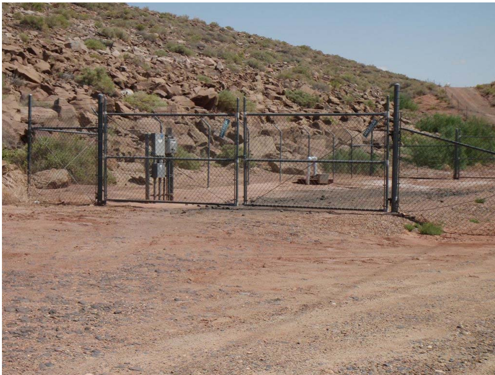
Photo 22 – Fly Ash Pond: Seepage collection system for Gironimo Seep.
