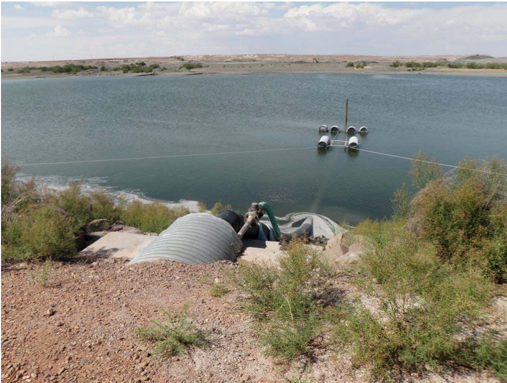
Photo 36 – Bottom Ash Pond: Floating siphon pipes to return water from main reservoir to power plant – upstream side of dam.
