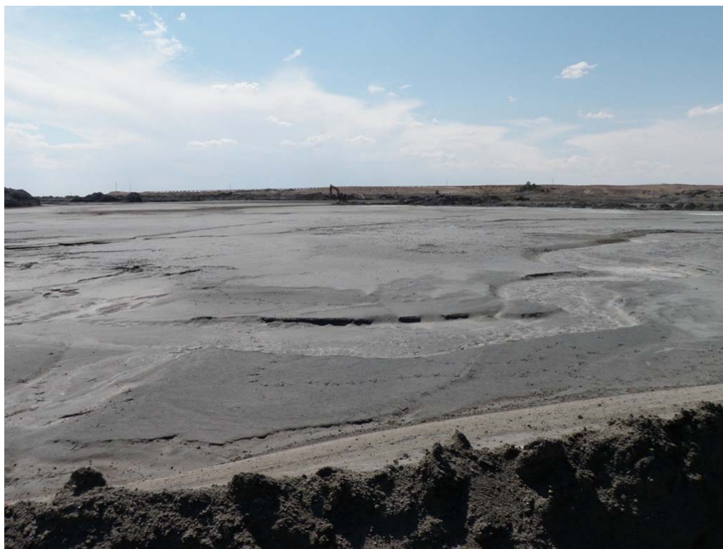
Photo 11 – Bottom Ash Pond: East cell with drained bottom ash. Note construction operations moving bottom ash to monofill.
