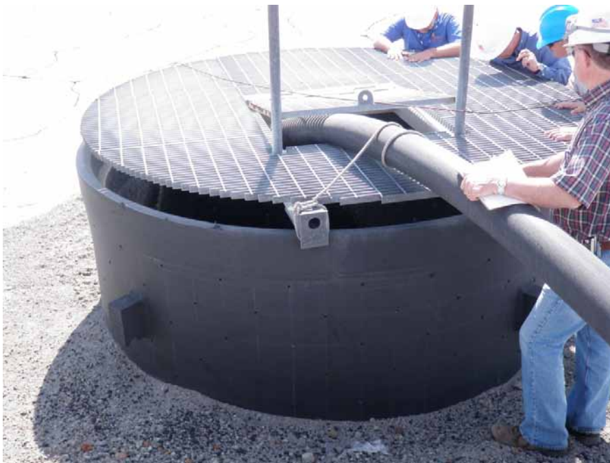
Photo 16 – LAI Decant drop inlet structure constructed of 8 ft diameter HDPE manhole. Small HDPE pipe is for water supply to construction of dam raise.
