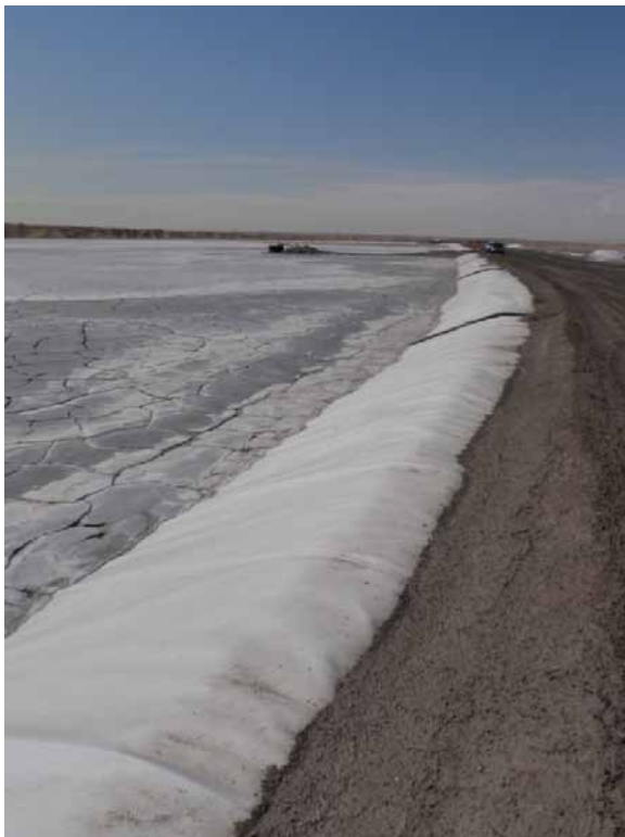
Photo 21 – LAI Upstream slope of west dam, looking right. Note berm to access decant drop inlet structure.
