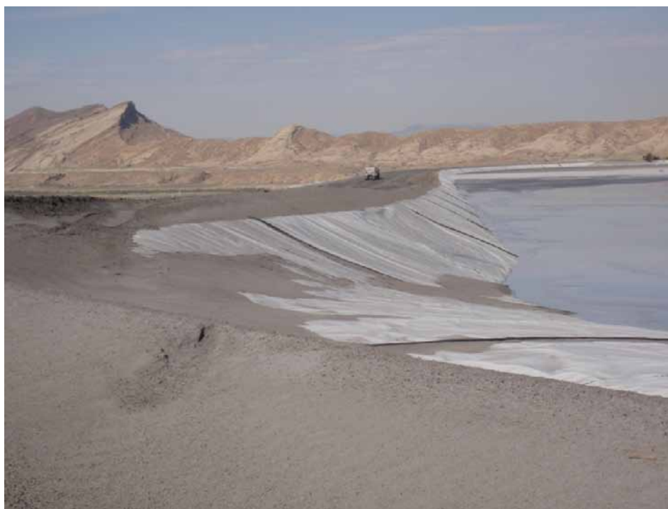
Photo 2 – LAI Upstream slope of south dam, looking to left. Note HDPE lining. Note lowest dam crest is on west side.
