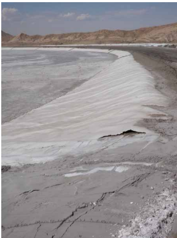
Photo 22 – LAI Upstream slope of north dam. Note tear in HDPE lining caused by construction equipment. APS has noted and plans immediate repair.
