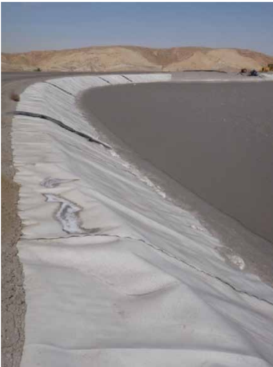
Photo 10 – LAI Upstream slope on south dam and southwest corner of impoundment. Note 'ash fill' placed on west upstream slope for pump to supply water for construction of LAI raise to El. 5258.
