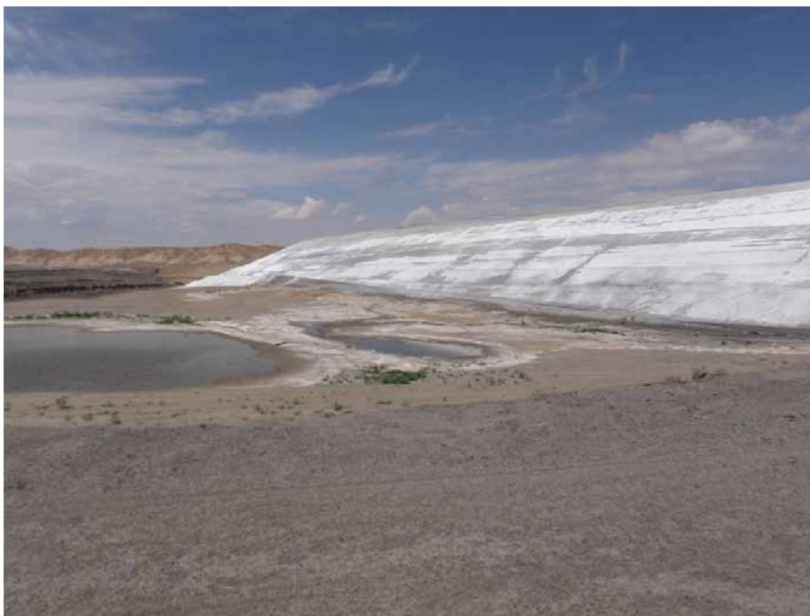
Photo 29 – LAI Downstream slope and toe of south dam, looking to right. Note ponded water near toe that results from seepage from old Pond #4 that underlies the LAI.
