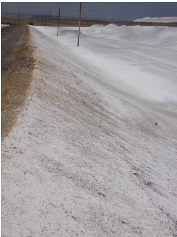
Photo 44 – LDWI Downstream slope of east dam, looking north. White material is lime applied as a dust control measure.
