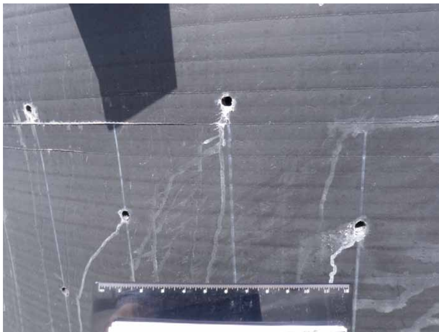
Photo 18 – LAI Close up view of 1/2" dia perforations in decant drop inlet.
