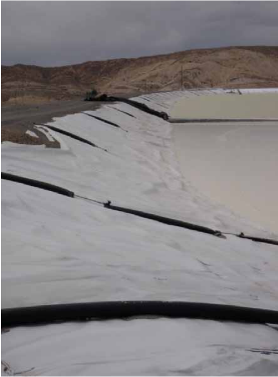
Photo 39 – LDWI Upstream slope of south dam. Note bladder dam used to divide reservoir to maintain depth of water over pumping system to convey water to power plant.
