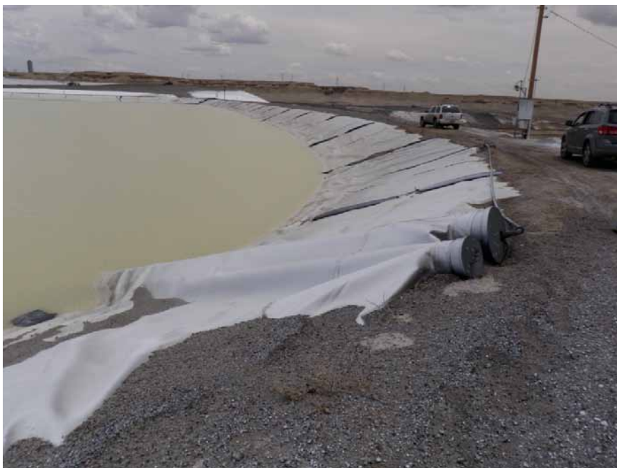
Photo 38 – LDWI southwest corner of impoundment. Note HDPE pipes used to monitor leak detection system between layers of HDPE lining. Power supply on pole is for automatic leak detection pump system.
