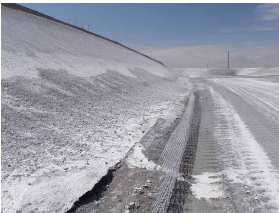
Photo 26 – LAI Downstream slope and toe of west dam, adjacent to LDWI. Note exposed geogrid strengthening layer that has been excavated for tie-in to dam raise fill.
