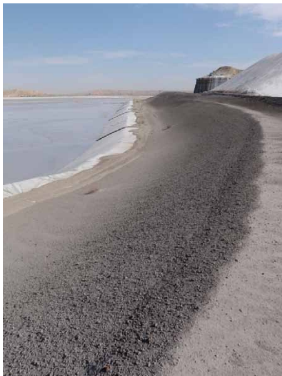
Photo 3 – LAI Upstream slope of east dam. East dam includes a rockfill zone. Note natural bluffs forming upslope side to east.
