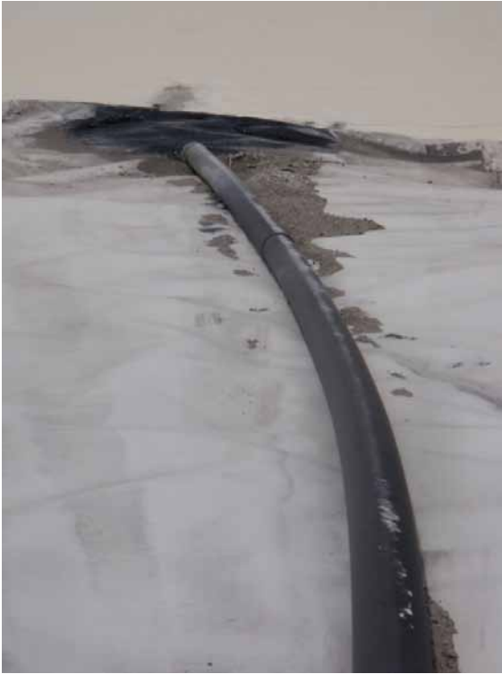
Photo 45 – LDWI Looking directly down slope at pipe from 8" perforated HDPE located in the LAI. Decant water collected by the perforated drain is pumped into the LDWI. Flow was observed to be a few gpm at the time of site visit.
