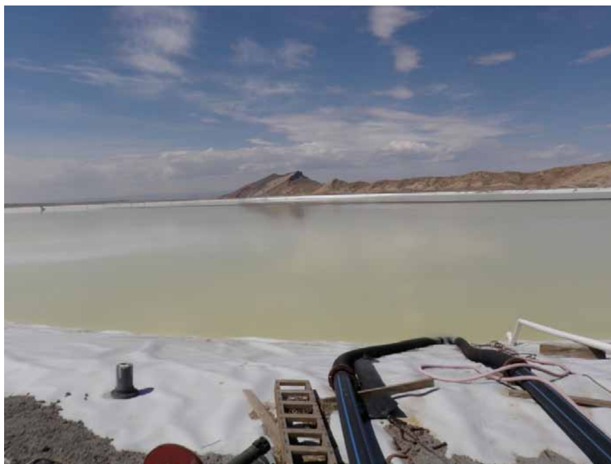
Photo 48 – LDWI Suction pipes for pumps recirculating water from LDWI back to power plant.
