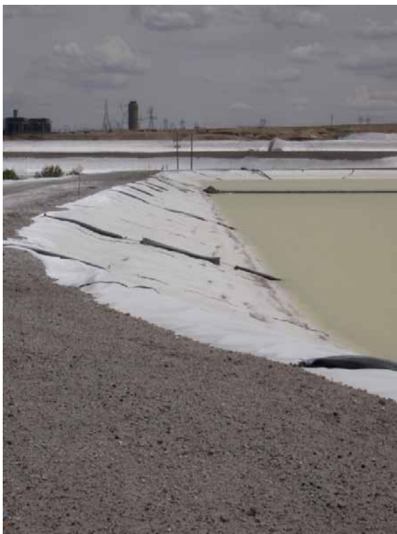
Photo 33 – LDWI upstream slope of north dam. Note dual HDPE lining.
