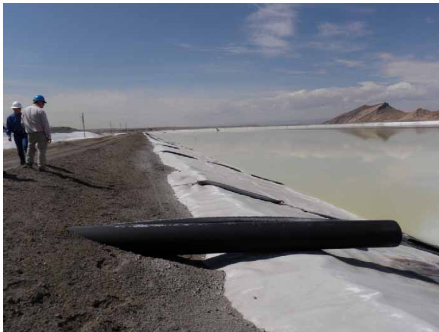
Photo 47 – LDWI Discharge end of 16" and adjacent 8" pipes with decant water from LAI.
