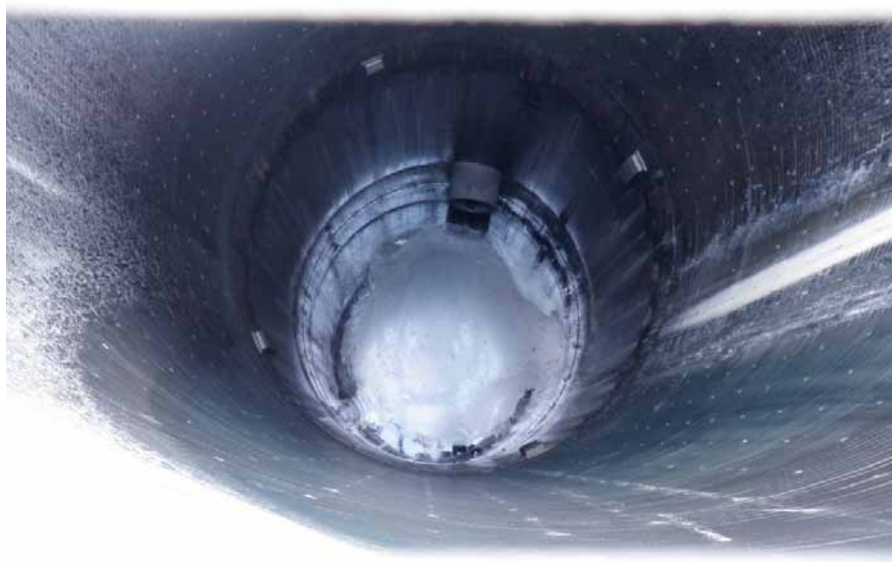
Photo 17 – LAI Looking down into decant drop inlet structure. Note perforations on sides of manhole and 16 inch diameter HDPE outlet pipe located above static water level. An 8 inch outlet pipe is submerged.
