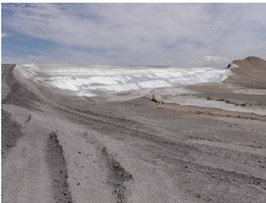
Photo 30 – LAI Downstream slope and toe of south dam, looking left toward the tie-in with natural weathered shale high ground.
