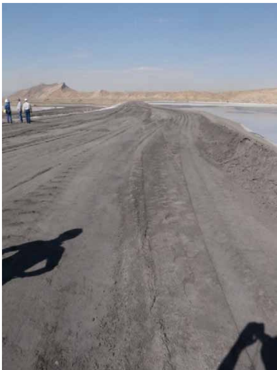
Photo 5 – LAI Dam crest on south dam, looking to left. Note small bottom ash 'berm' at slope crest for construction traffic safety.
