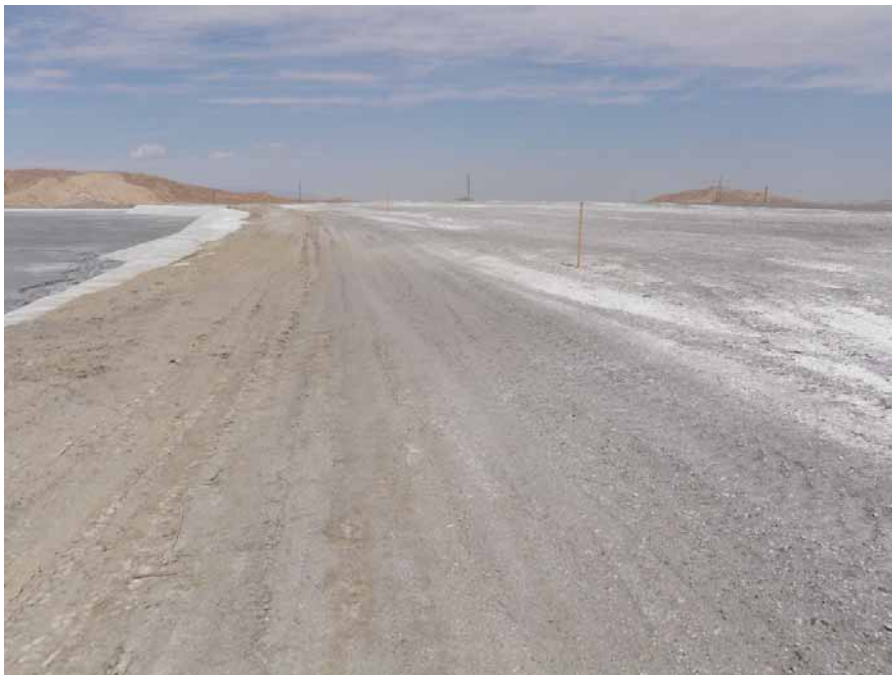
Photo 25 – LAI Crest of north dam. Note gradually sloping fill between impoundment and Pond #6 to right (out of service).
