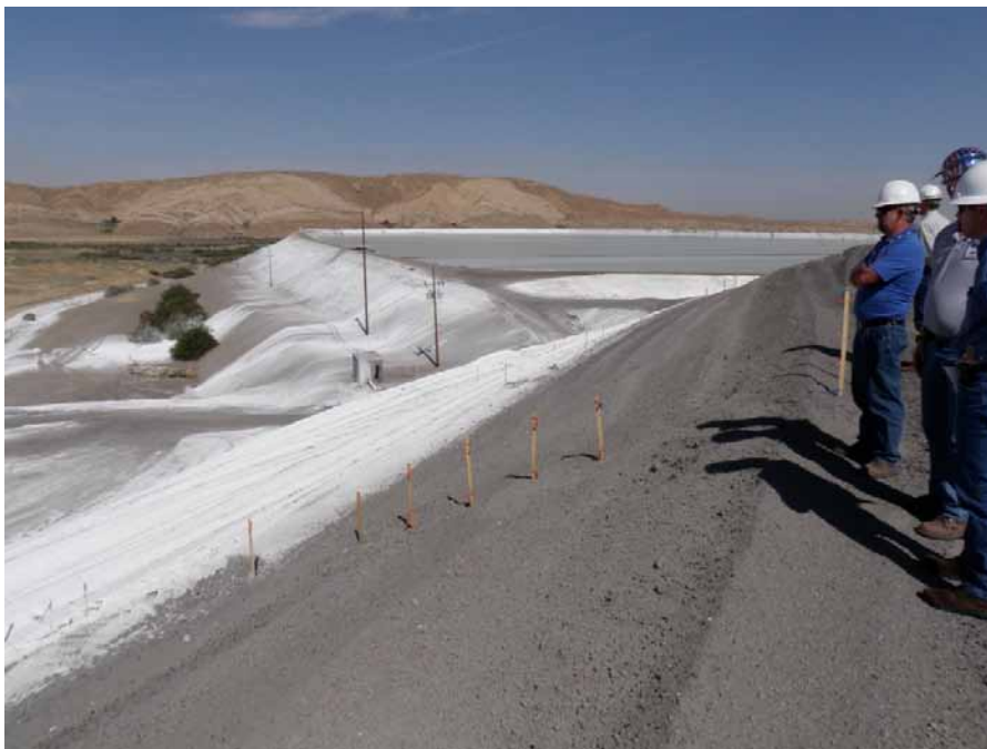
Photo 11 – LAI Downstream slope at southwest corner. Note LDWI at lower elevation in background and small pump station structure for decant water.
