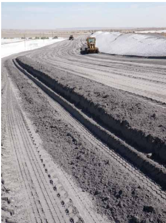
Photo 14 – LAI Widening the west dam in preparation for dam raise construction.
