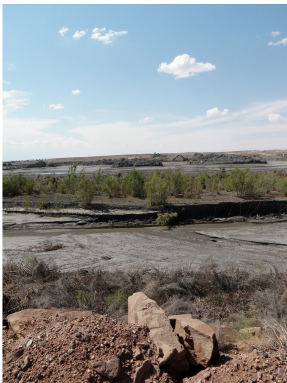
Photo 14: Bottom Ash Pond - Drainage way for overflow water from upstream cells to main reservoir.
