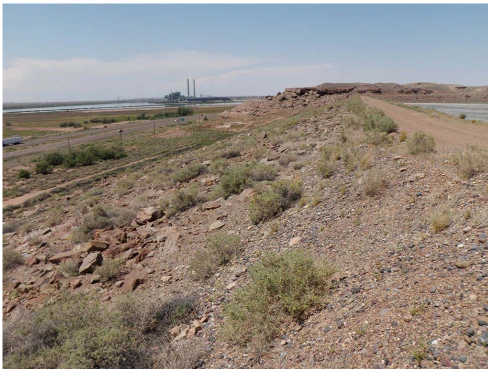
Photo 7: Fly Ash Pond Dam - Downstream slope, looking west. Note vegetation.
