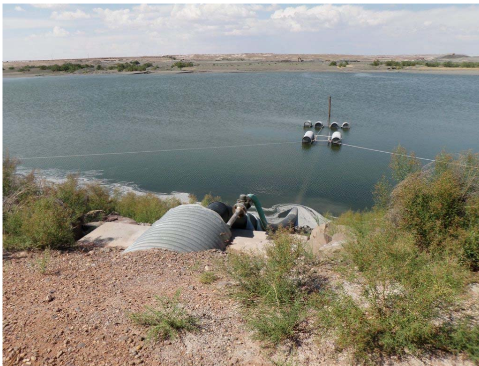
Photo 36: Bottom Ash Pond - Floating siphon pipes to return water from main reservoir to power plant – upstream side of dam.
