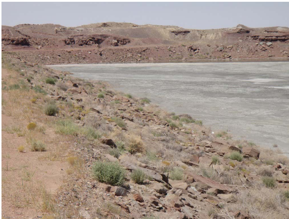
Photo 5: Fly Ash Pond Dam - Upstream slope, looking west. Note vegetation.
