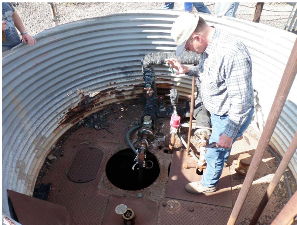
Photo 27: Bottom Ash Pond - Seepage collection system at West Abutment Seep.
