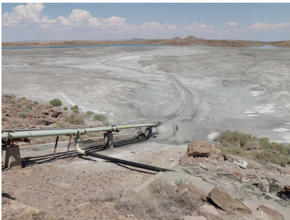
Photo 6: Fly Ash Pond Dam - Slurry discharge point on upstream face.
