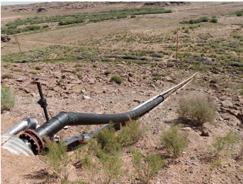
Photo 37: Bottom Ash Pond - Siphon pipes extending along downstream slope of dam.
