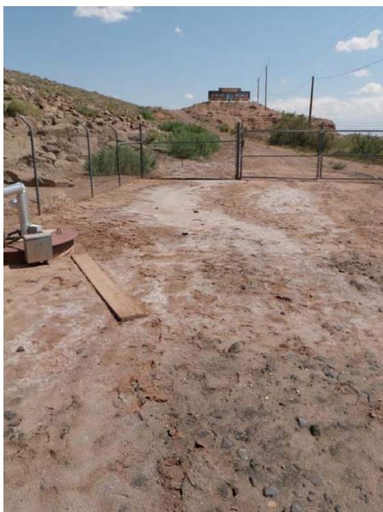
Photo 24: Fly Ash Pond - Hunt Seep area. Note seepage collection system on left. Also note the highway embankment seen on the top left of this photo.
