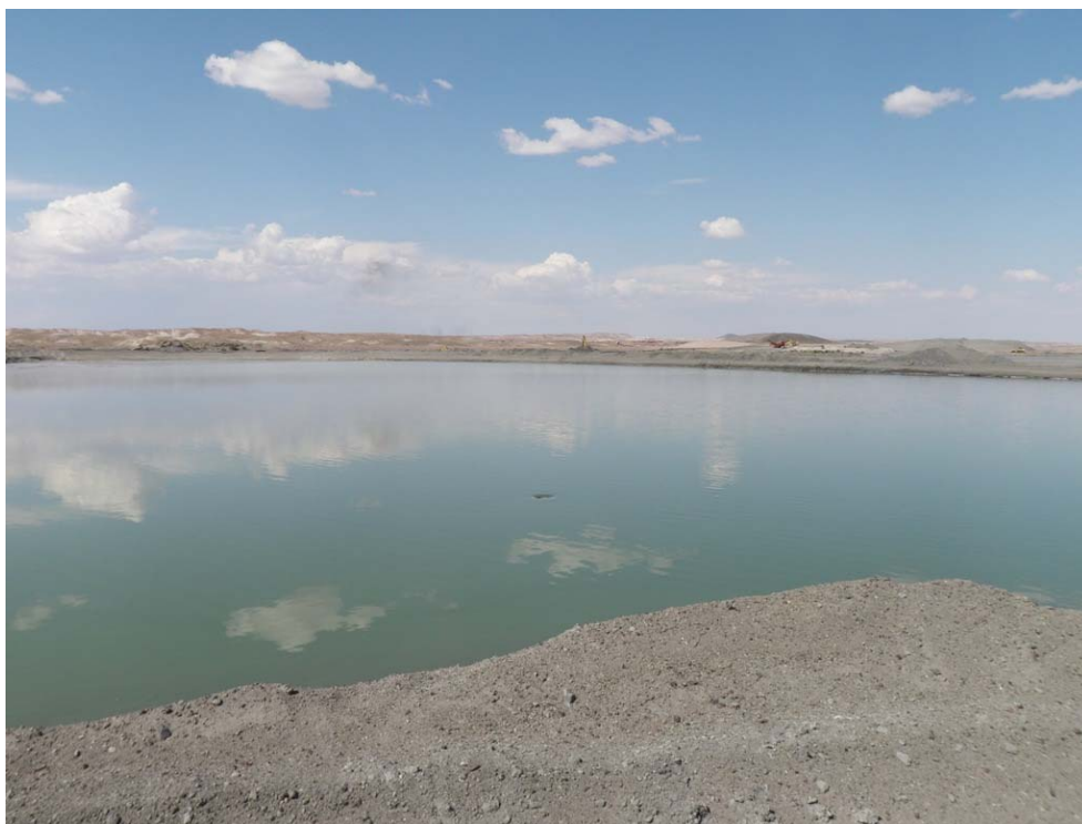
Photo 12: Bottom Ash Pond - West cell, which is currently being filled with bottom ash slurry. Note vortex through which water flows to main reservoir.
