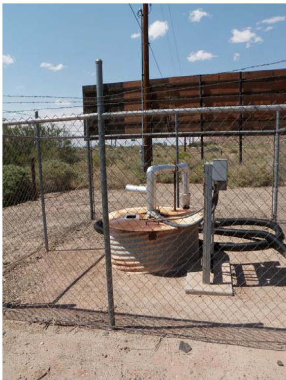
Photo 23: Fly Ash Pond - Seepage collection system for Geronimo Seep.
