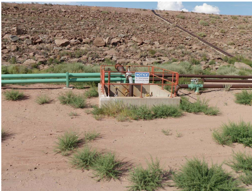
Photo 39: Bottom Ash Pond - Siphon pipes extending along downstream slope, and siphon collection station.
