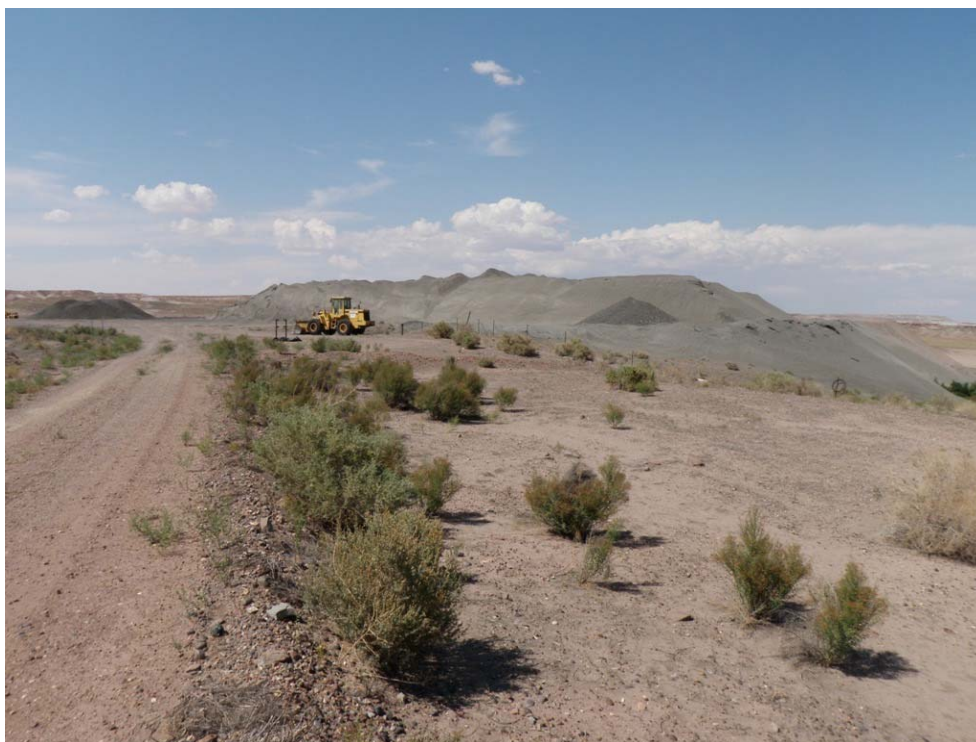
Photo 13: Bottom Ash Pond - Monofill for final storage of drained bottom ash.
