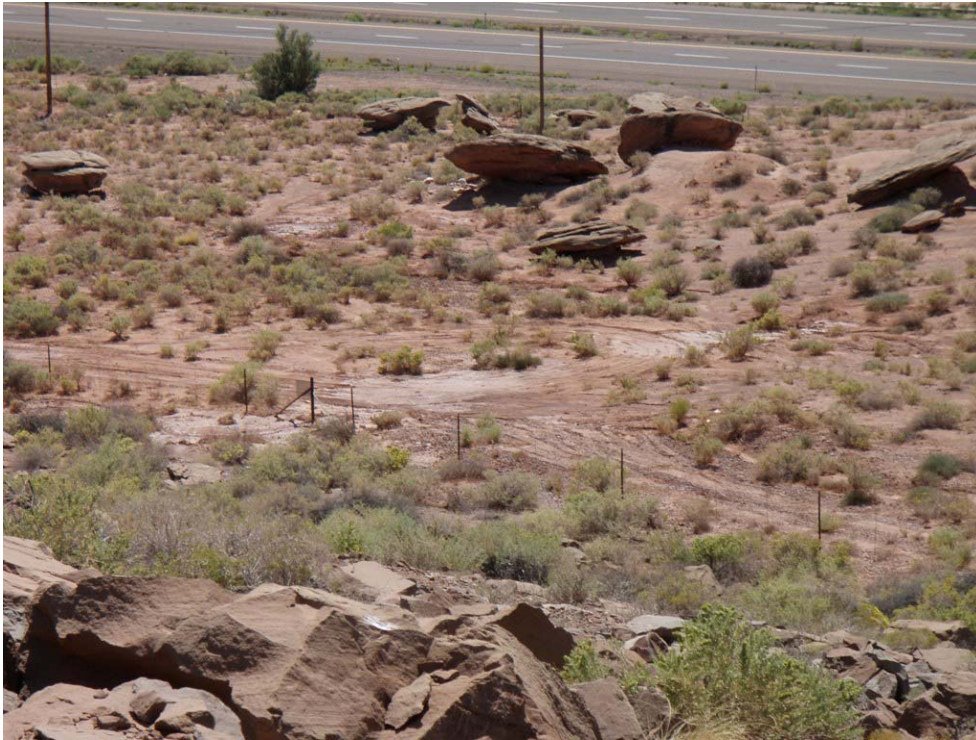
Photo 19: Fly Ash Pond - Salt patch associated with seepage near right abutment toe (known as the "Hoodoo Salt Patch").
