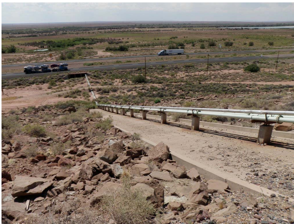
Photo 8: Fly Ash Pond Dam - Slurry pipes on downstream face.
