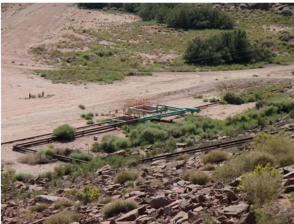
Photo 38: Bottom Ash Pond - Siphon collection station at toe of dam.
