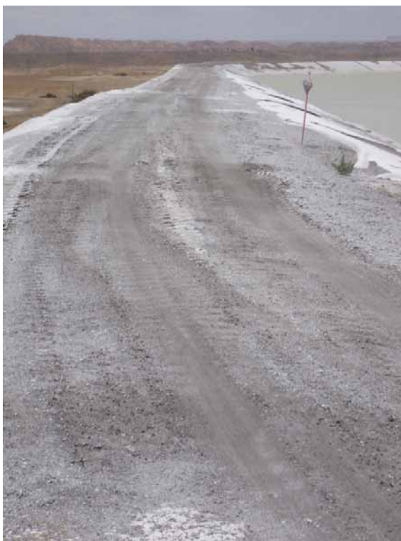
Photo 36 – LDWI Crest of west dam. Note areas of eroded crest material due to wind.
