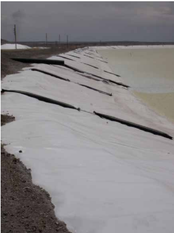
Photo 46 – LDWI Upstream slope of east dam, looking south. Note the 16 inch and 8 inch discharge pipes from the LAI decant intake that are routed across the top of the LDWI dam.
