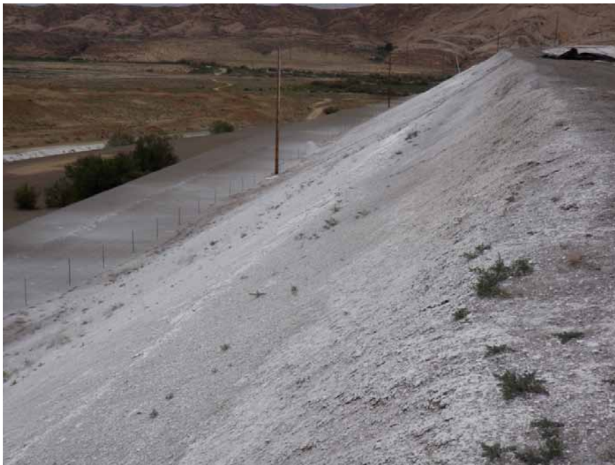
Photo 41 – LDWI Downstream slope of south dam.
