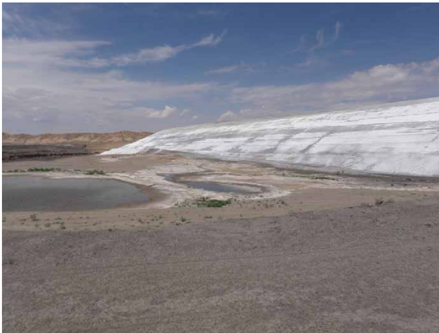
Photo 29 – LAI Downstream slope and toe of south dam, looking to right. Note ponded water near toe that results from seepage from old Pond #4 that underlies the LAI.
