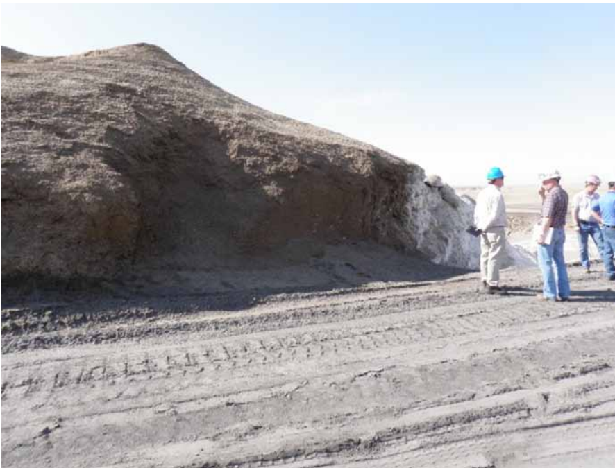
Photo 6 – LAI Exposed part of natural weathered shale that the south and east berm clay cores tie into for seepage control.
