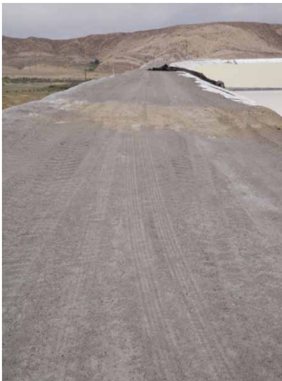
Photo 40 – LDWI Crest of south dam.
