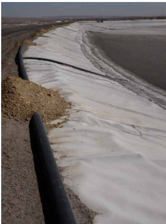
Photo 12 – LAI Upstream slope on west dam. HDPE pipe is to supply water for construction.
