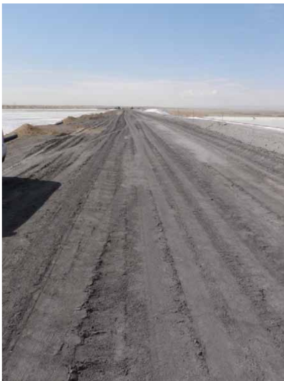
Photo 20 – LAI Crest of west dam, looking right.
