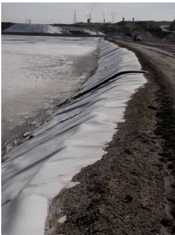
Photo 8 – LAI Upstream slope on south dam.
