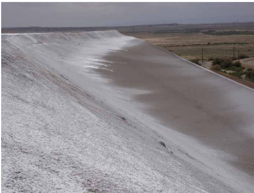
Photo 35 – LDWI downstream slope of west dam.
