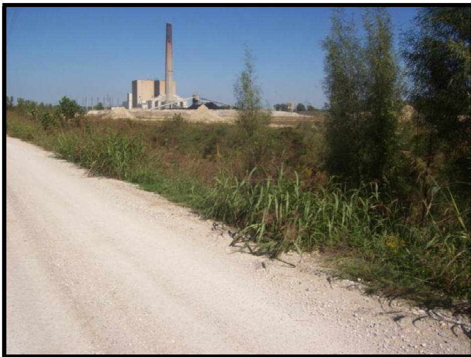
Figure 16: Vegetative growth adjacent to top of ash pond embankment, North. (A contract is in place to clear trees.)
