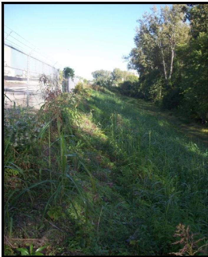
Figure 3: Ash pond external embankment with medium vegetation, Northwest.
