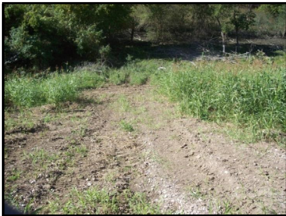
Figure 14: Heavily eroded area along exterior embankment of ash pond.
