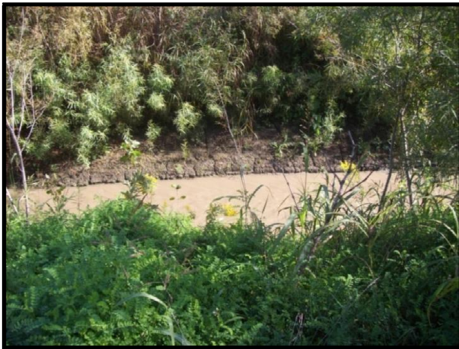
Figure 15: Downstream embankment of ash pond at Isle du Bois Creek. (High water noted during assessment. There is a 5' bench from toe of embankment to creek.)
