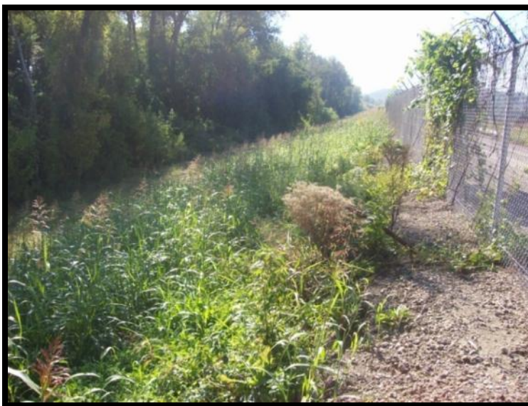
Figure 5.2.3-1: Ash pond external embankment with medium to heavy vegetative cover, Southeast.
