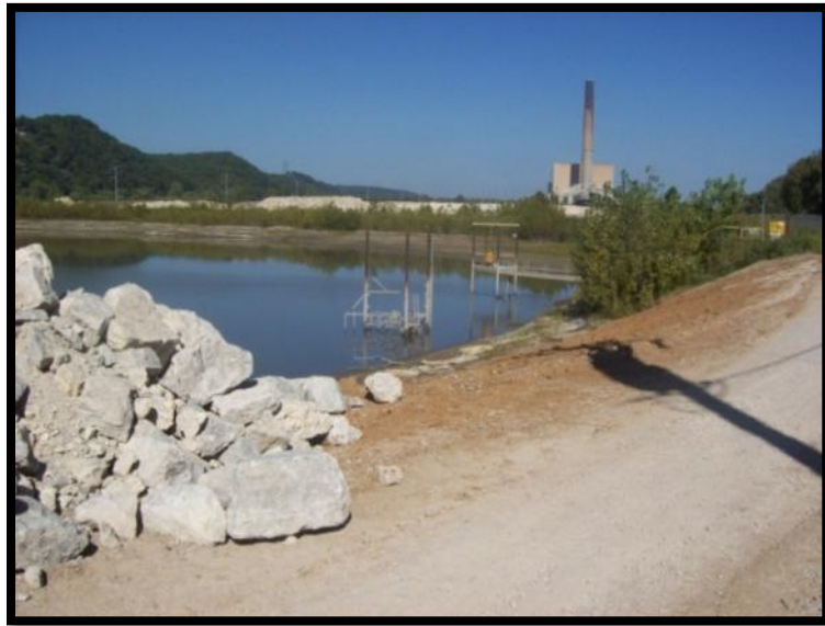
Figure 5.3.1-1: Ash pond inactive (left) and active (right) overflow structures, Northwest.
