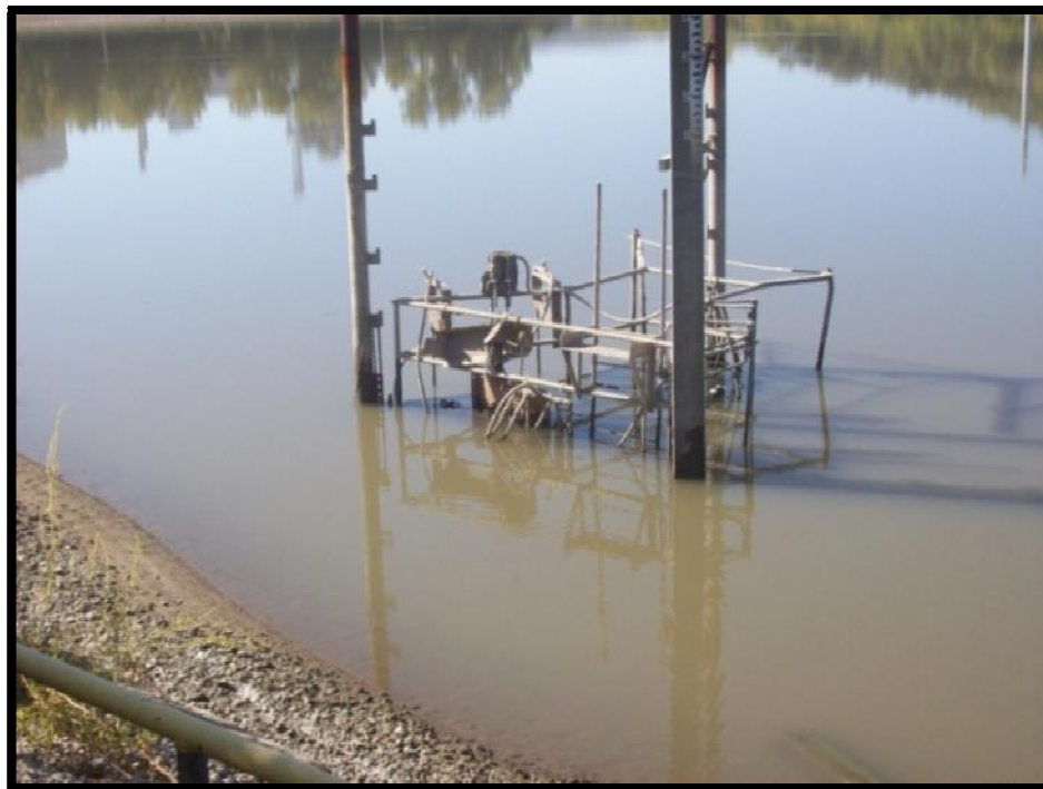
Figure 9: Inactive ash pond overflow structure.
