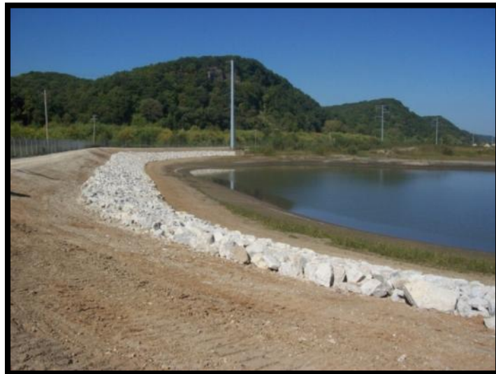
Figure 5.2.2-2: Riprap armored interior slope of ash pond.
