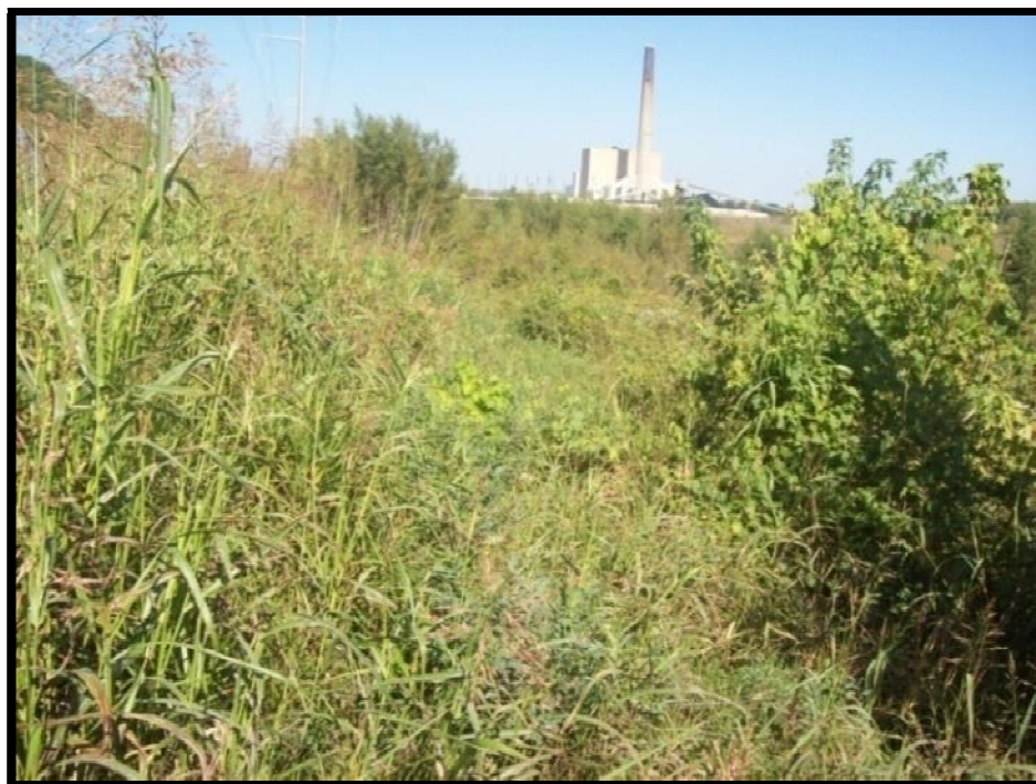
Figure 12: Ash pond exterior embankment with heavy vegetation, Northwest.
