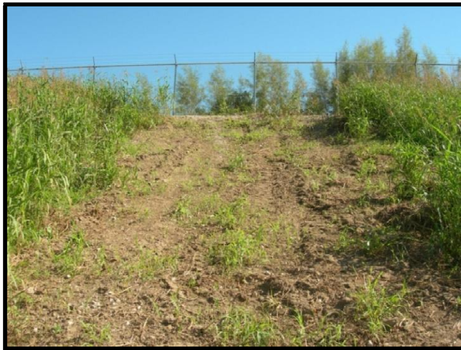
Figure 13: Ash pond exterior embankment erosion.
