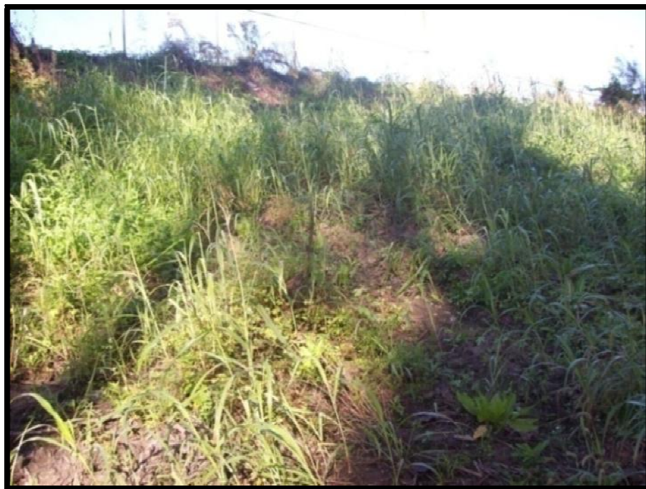
Figure 4: Ash pond external embankment with minimal ground cover and minor erosion from roadway runoff.
