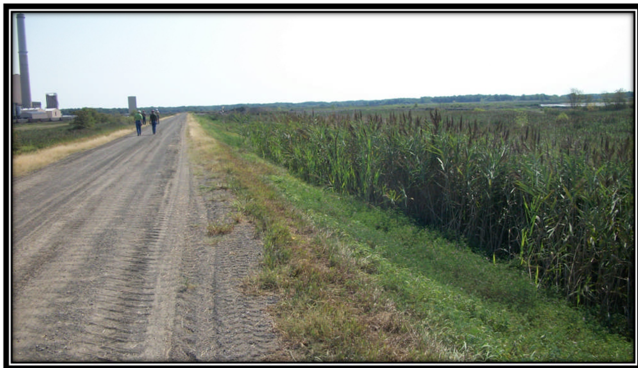
Photo 26 – Minor vegetation on upstream slope
