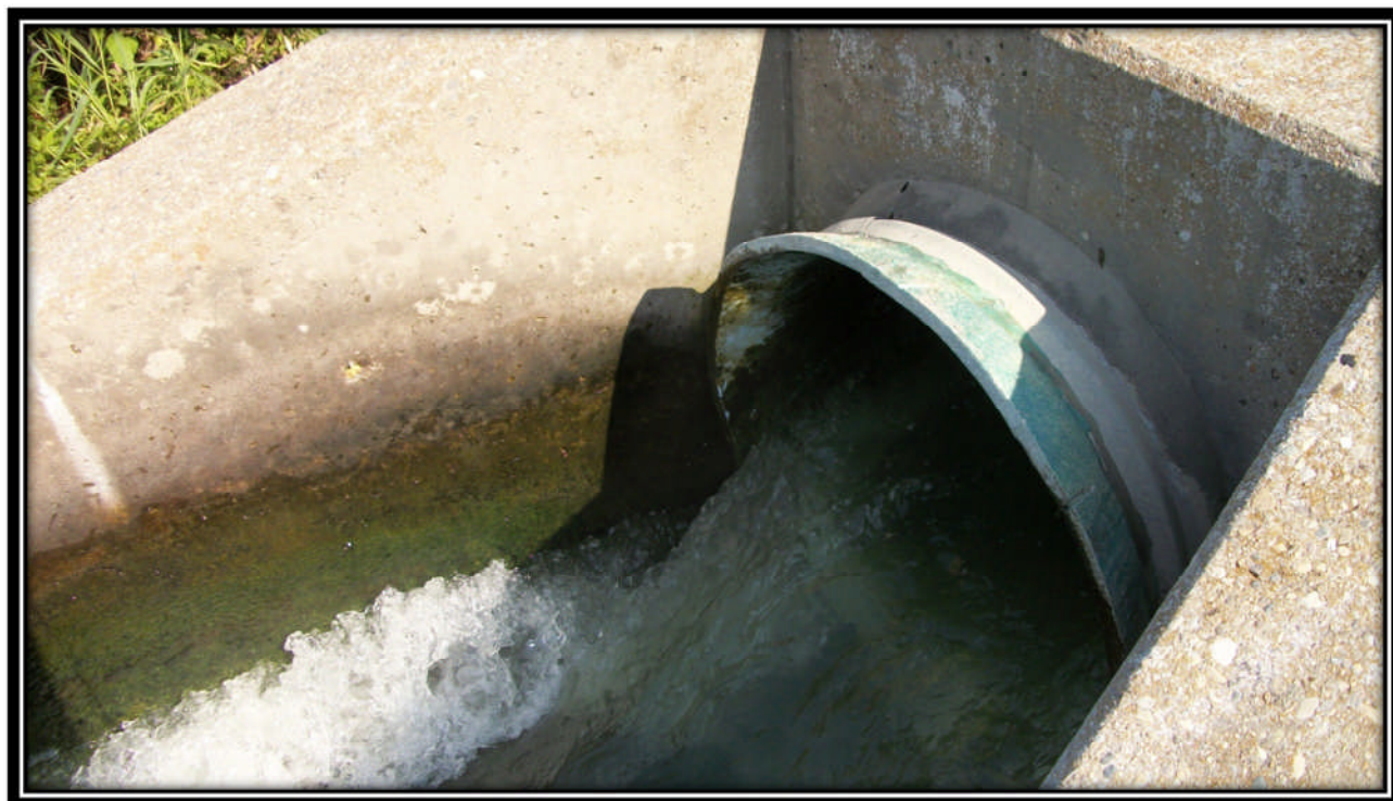
Photo 18 – CIPP lining slipped into CMP
