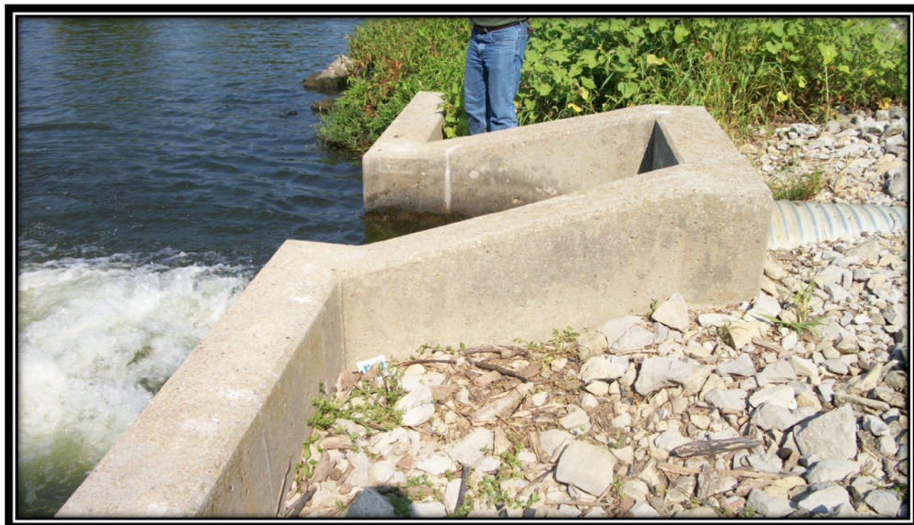
Photo 17 – CIPP lining slipped into CMP, discharging into Lake Newton
