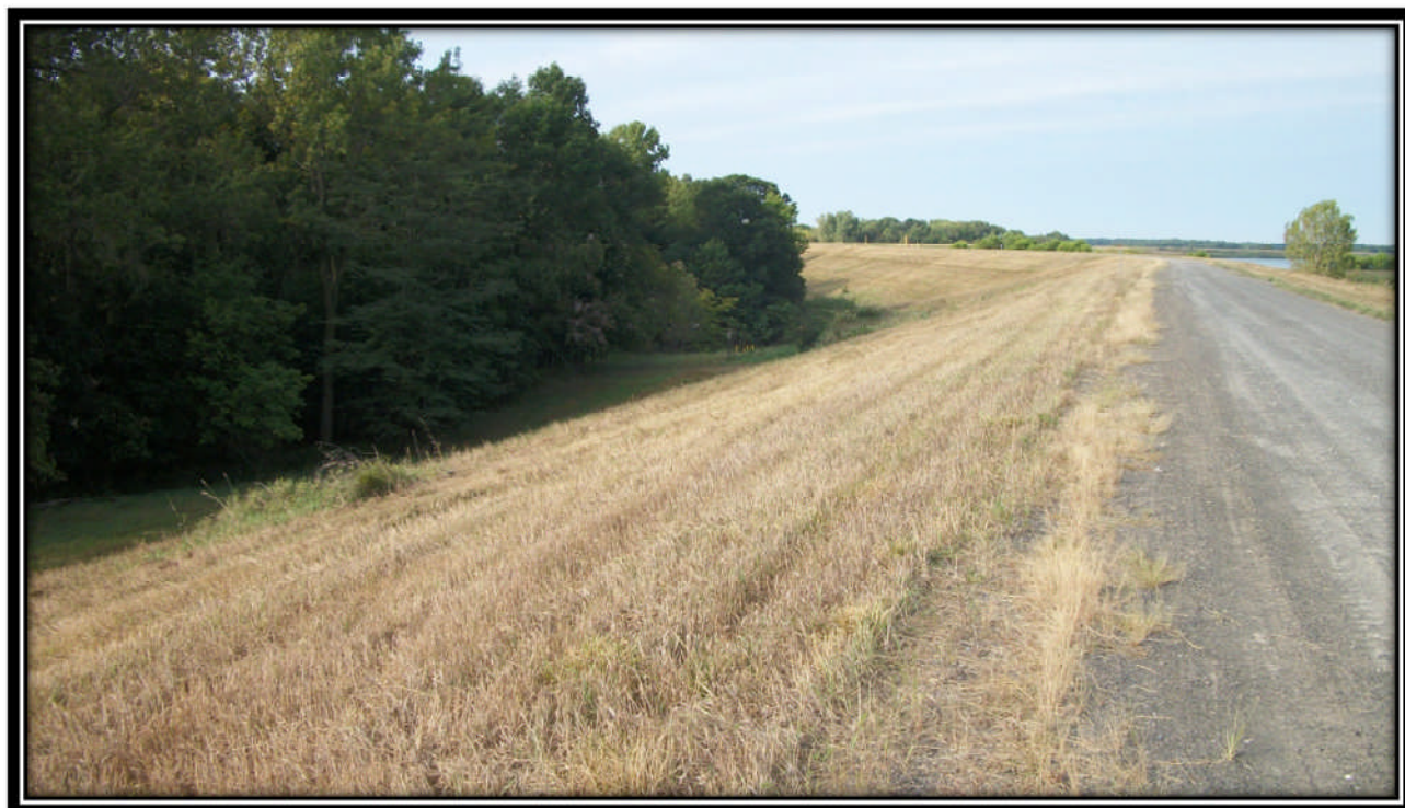
Photo 4 – Looking South along East embankment, vegetation on downstream slope
