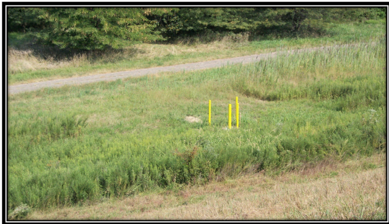
Photo 21 – Monitoring well on downstream toe
