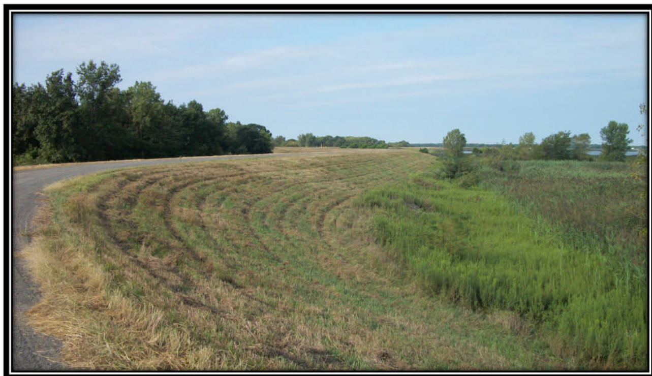
Photo 3 – Looking South along East embankment, vegetation on upstream slope
