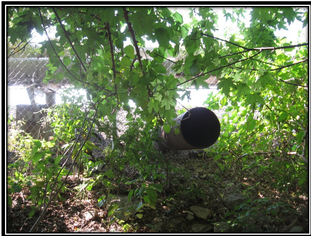
Photo 10 – Emergency Spillway Pipe for the Bottom Ash Pond
