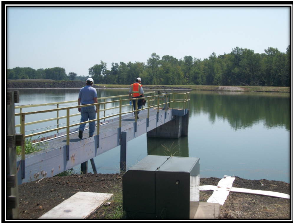
Photo 32 – Fly Ash Pond Outlet Works
