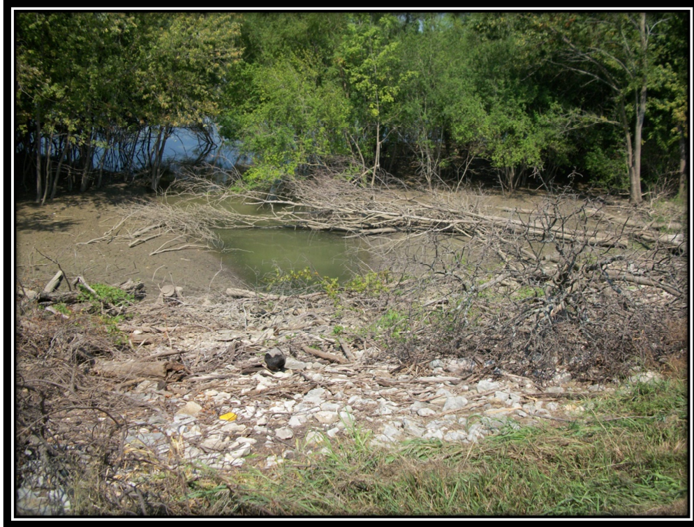
Photo 33 – Fly Ash Pond Outlet Works Pipe Outfall (Submerged)
