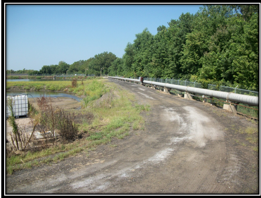
Photo 1 – Bottom Ash Pond Embankment Looking Southwest (Note Pipeline, Foundations and Fence)
