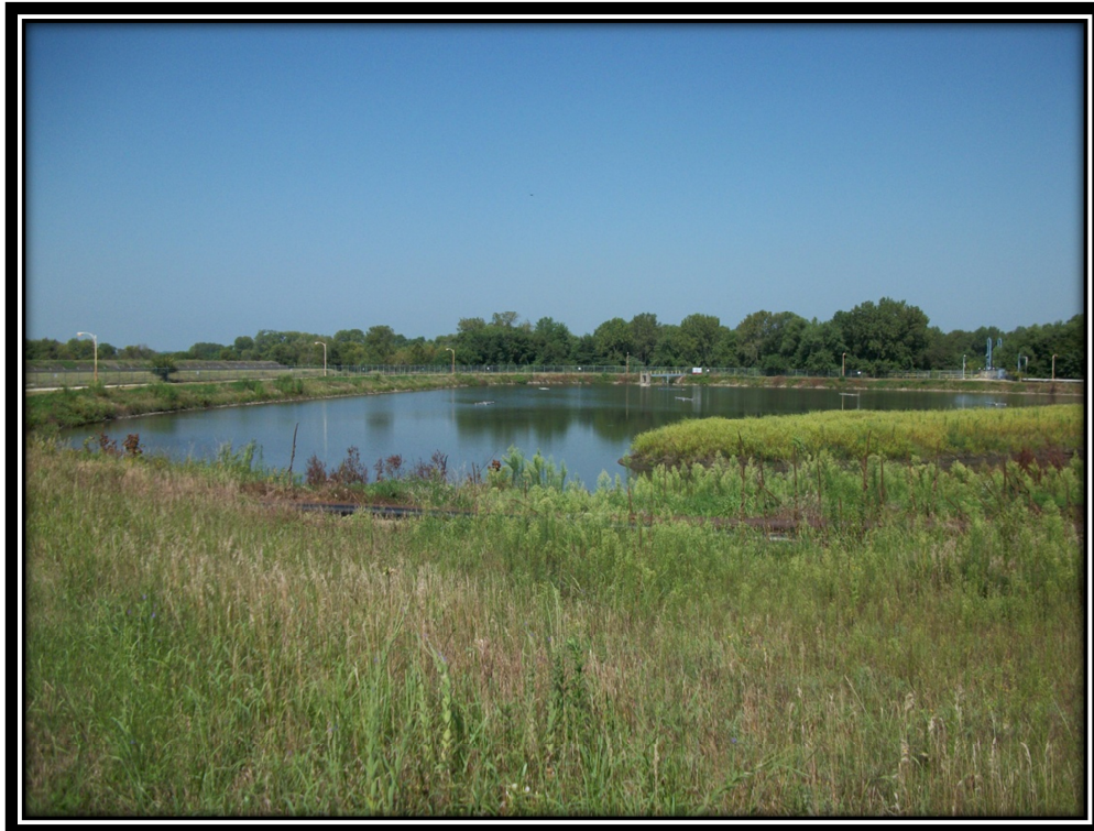
Photo 26 – General Photograph of the Bottom Ash Pond (Note Settling Channel and Main Pond)
