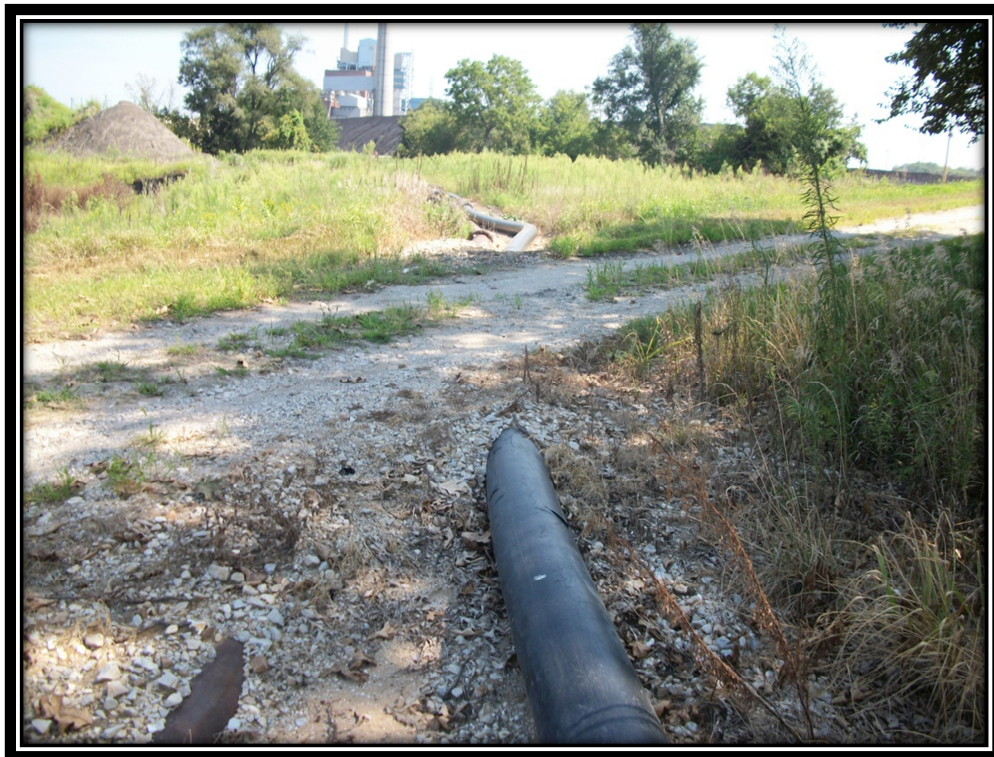
Photo 24 – Sluice Pipe Penetrations through Crest of Bottom Ash Pond Embankment
