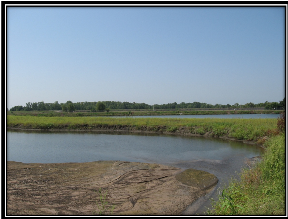
Photo 6 – Settling Channel of Bottom Ash Pond near Inlet
