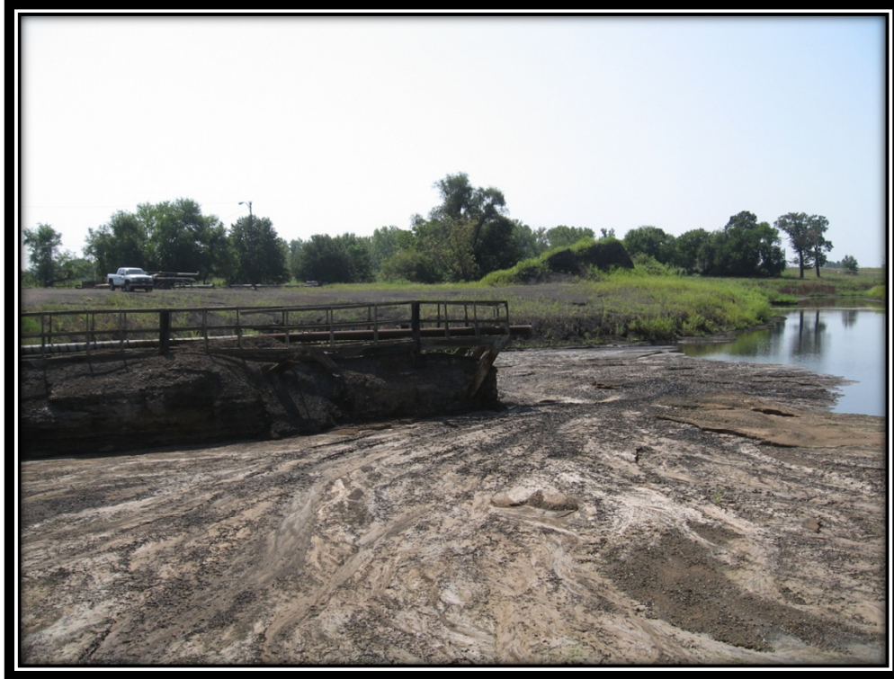
Photo 5 – Bottom Ash Pond Inlet Piping
