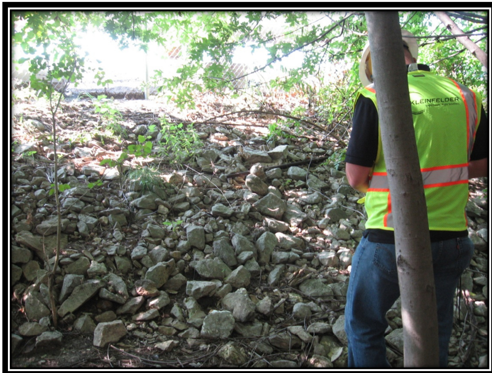
Photo 8 – Riprap on Downstream Slope of Bottom Ash Pond (Typical)
