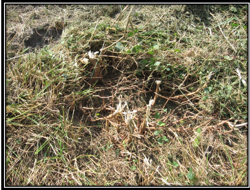
Photo 35 – Mowed Woody Vegetation on Downstream Slope of Fly Ash Pond (Note Intact Root System)
