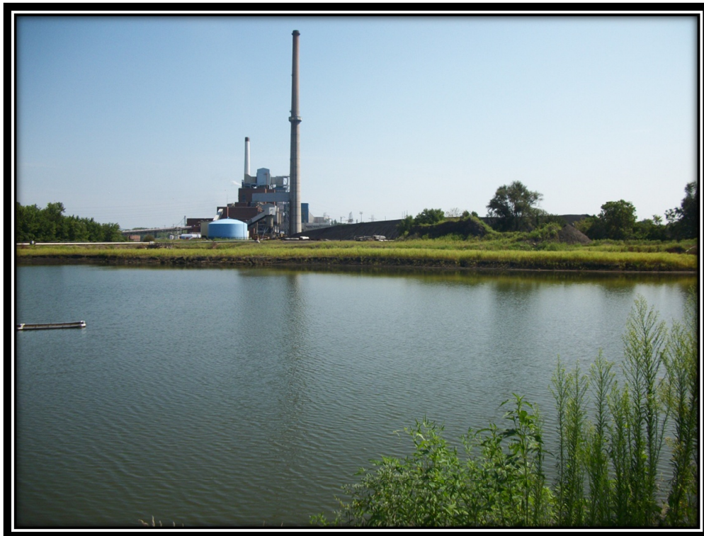
Photo 22 – General Photo of Bottom Ash Pond Looking Northeast
