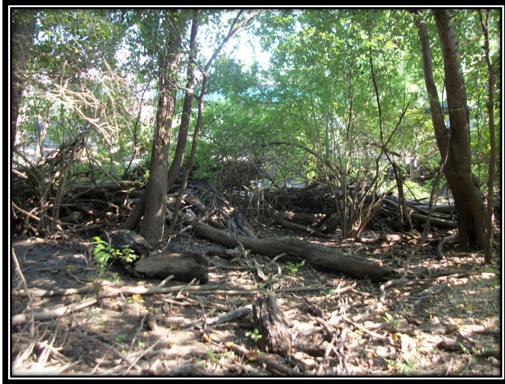
Photo 17 – Debris Pile and Heavy Vegetation at the Downstream Toe of the Bottom Ash Pond (Typical)
