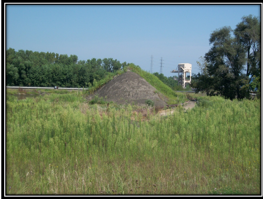
Photo 27 – Stockpile of Bottom Ash Recovered from the Bottom Ash Pond
