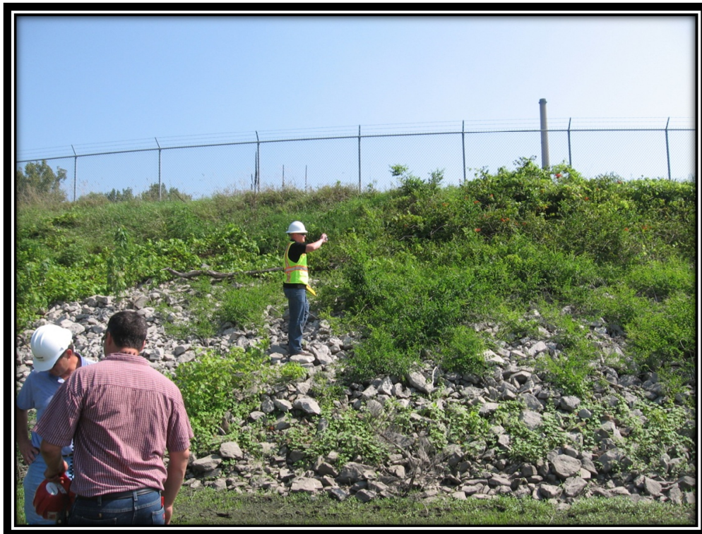
Photo 20 – Riprap on Downstream Slope of Bottom Ash Pond (Note Fence at Crest)
