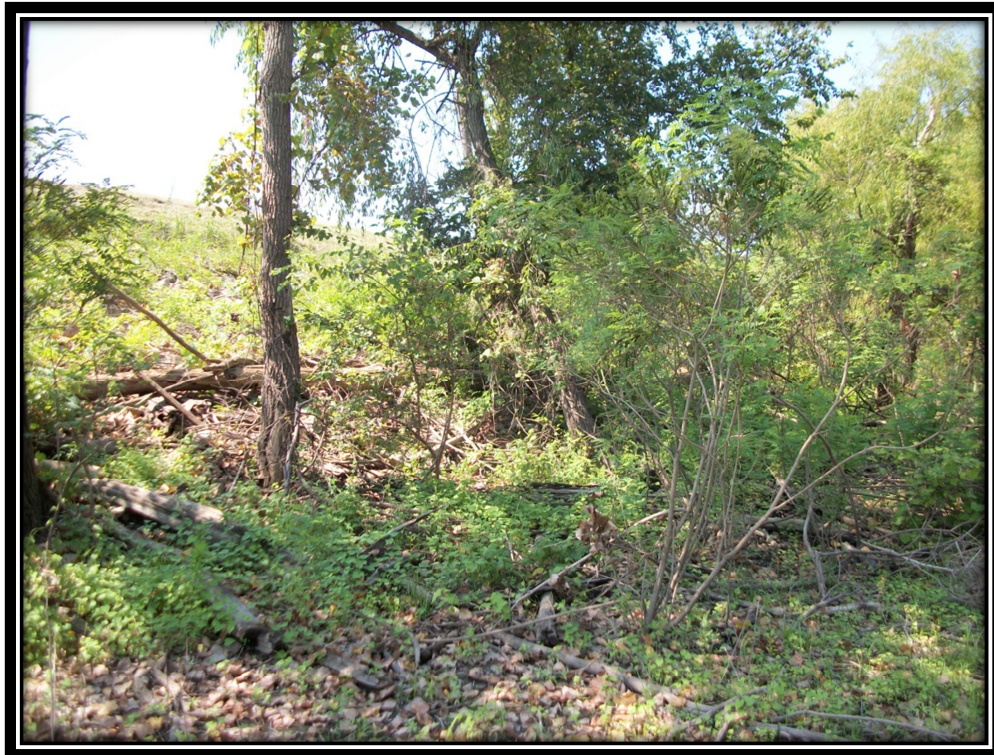
Photo 30 – Vegetation on the Downstream Slope and Toe of the Fly Ash Pond
