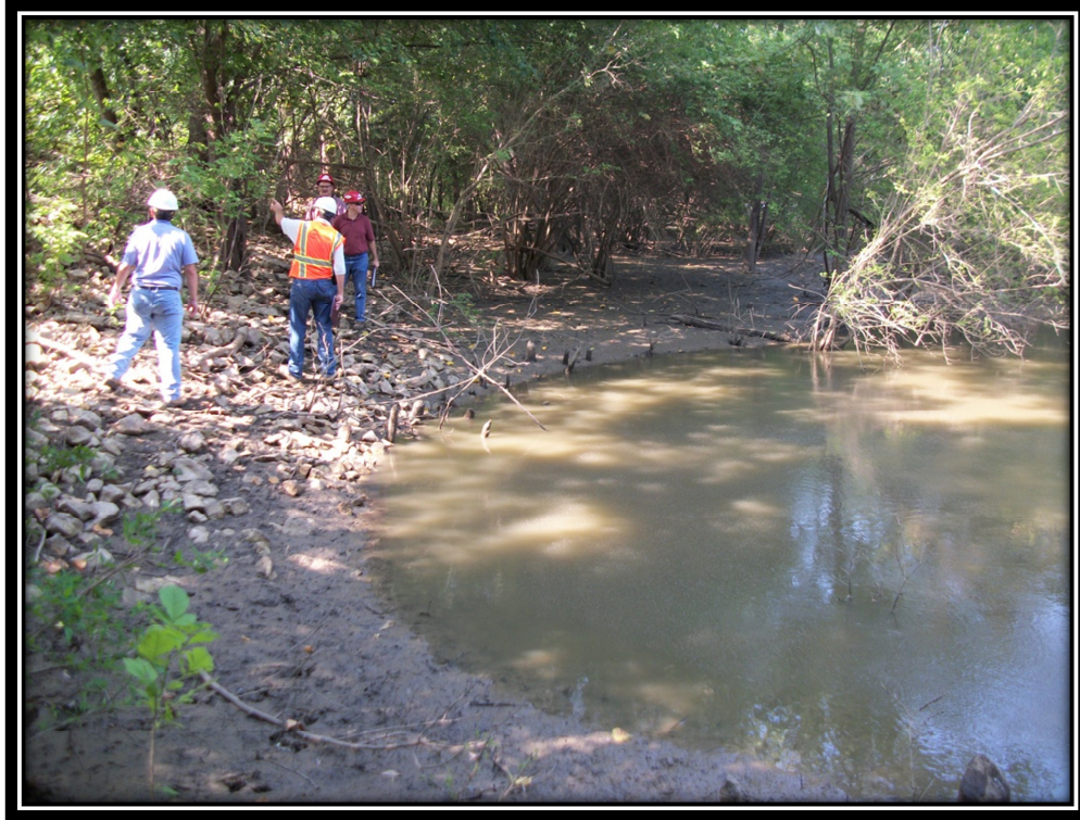
Photo 15 – Bottom Ash Pond Outlet Piping Outfall (Submerged)
