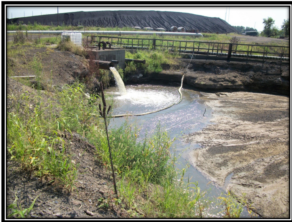
Photo 4 – Bottom Ash Pond Inlet Piping (Note Coal Stockpile in Background)
