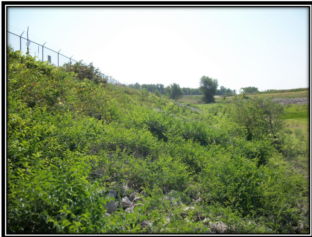
Photo 18 – Vegetated Riprap on the Bottom Ash Pond Southwest Embankment
