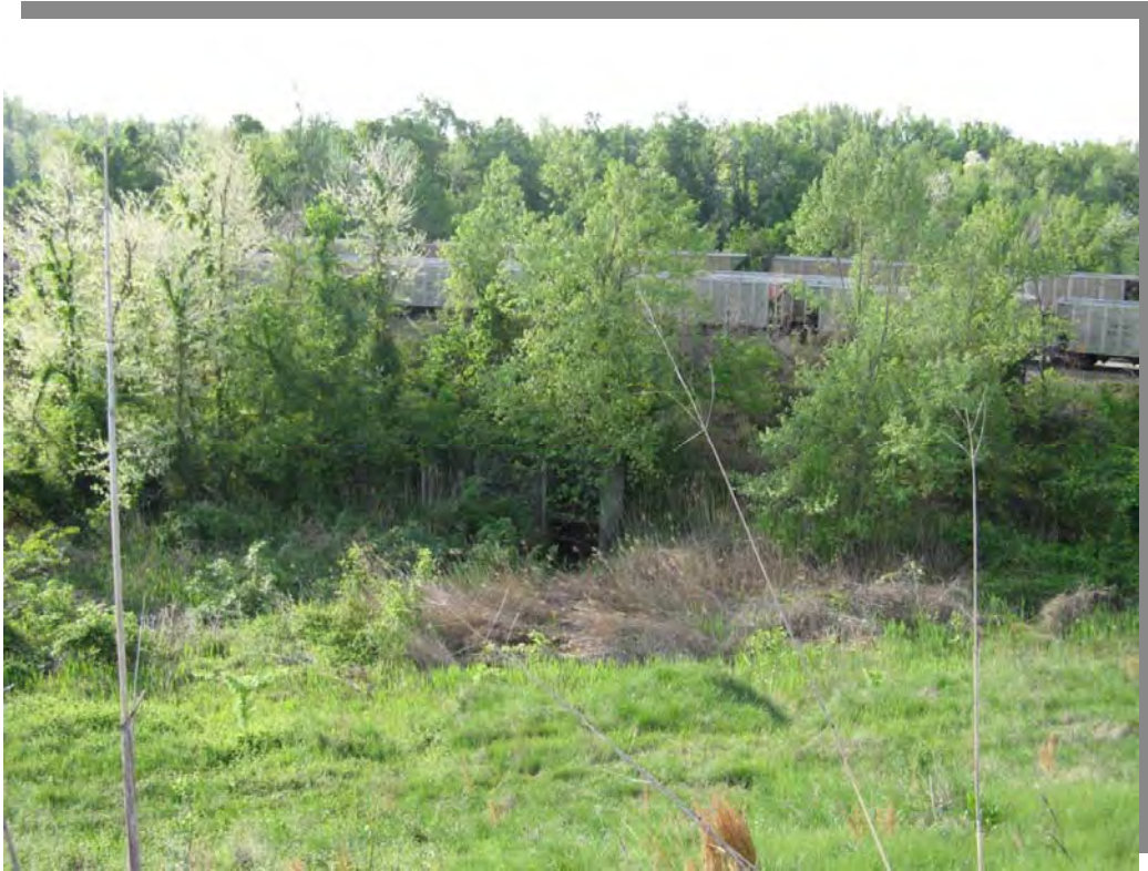
Photo 25 – Ash Pond outlet channel pass-through below EEI railroad siding.
