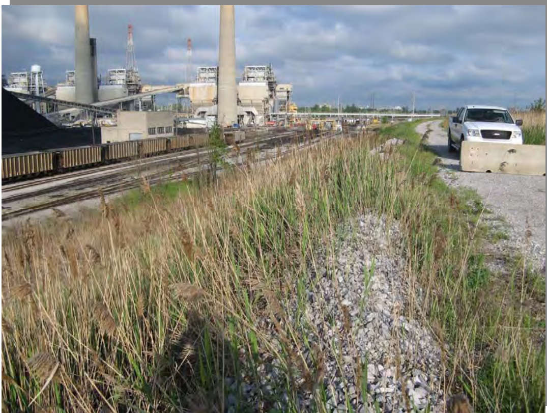
Photo 18 – Outboard slope of southern embankment of Southern Pond. Note Jersey barrier blocking vehicular access to eastern embankment.
