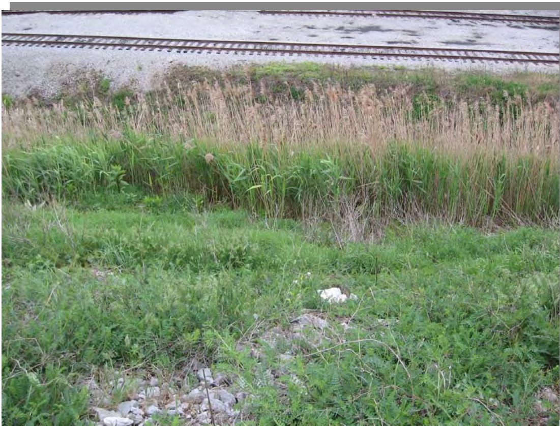
Photo 8 – Outboard slope of Northern Pond near the northern end. Note reedy grasses at toe.
