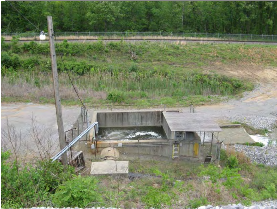
Photo 9 – pH balance outlet structure. Note HDPE pipe running parallel to toe (Southern Pond discharge) joining with concrete pipe (Northern Pond discharge) outside of structure.
