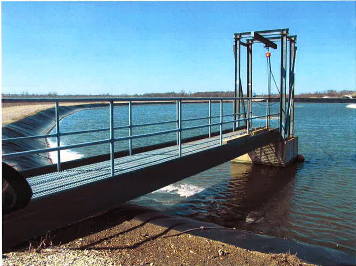
Photo #6 – Ash Pond B – Outlet structure
