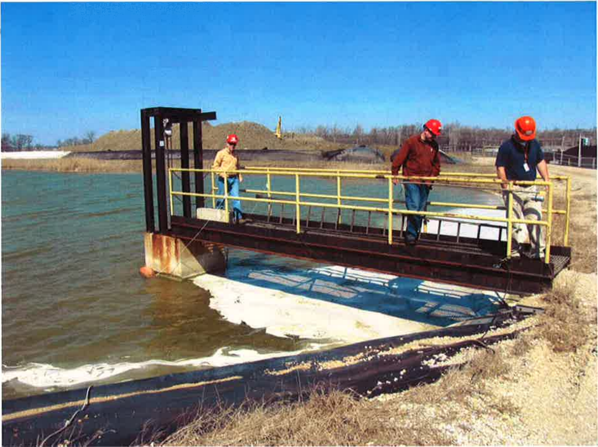
Photo #5 - Ash Pond A – Outlet structure
