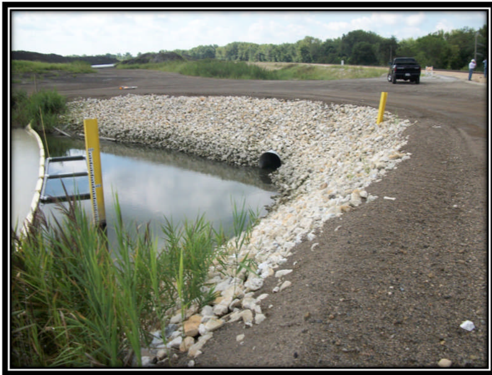
Photo 33 – Outlet Piping from Pond 1 into Clarification Pond Inlet Channel
