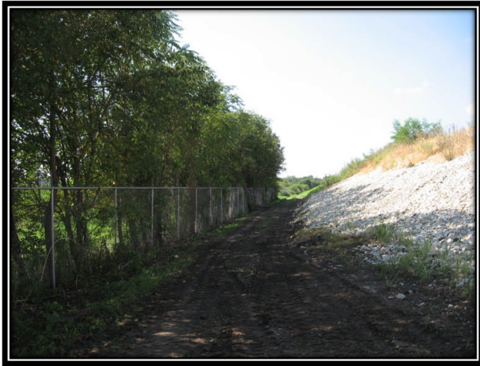
Photo 9 – Cleared Toe of Downstream Slope (Note Riprap and Minor Rutting)
