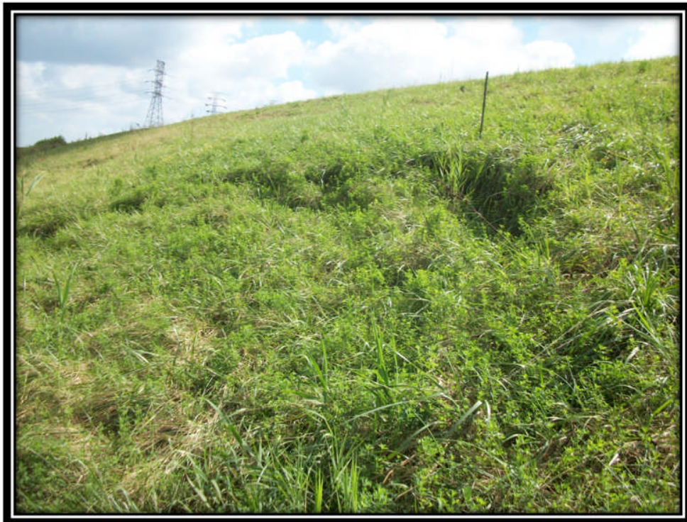
Photo 36 – Scarp on Western Pond 1 Downstream Slope (Note Post for Observational Purposes)
