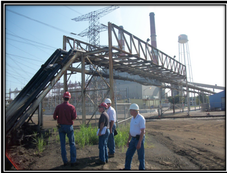
Photo 2 – Elevated Sluice Pipe Structure
