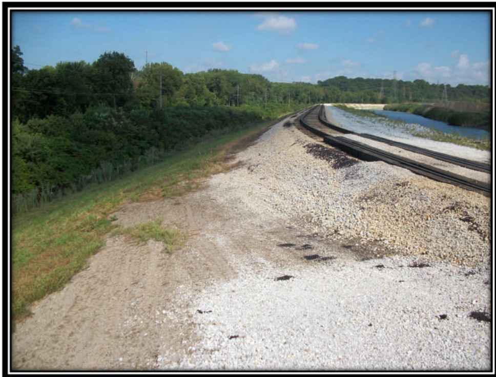
Photo 24 – Original Embankment with Raised Railroad Embankment Improvements Visible
