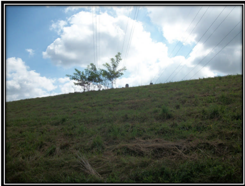
Photo 32 – Small Diameter Vegetation Growing on Crest
