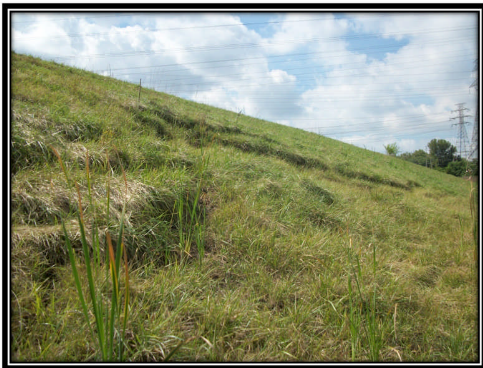
Photo 38 – Scarp on Western Pond 1 Downstream Slope
