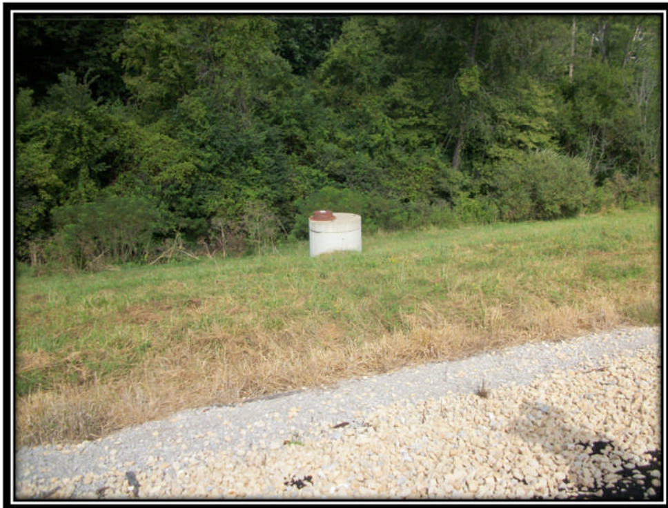
Photo 28 – Waste Water Sewer Line Manhole in Downstream Slope (Near Toe of Original Embankment)
