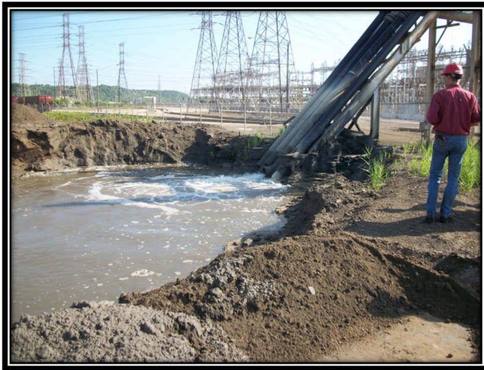
Photo 1 – Sluice Pipes at the Inlet to the Ash Pond
