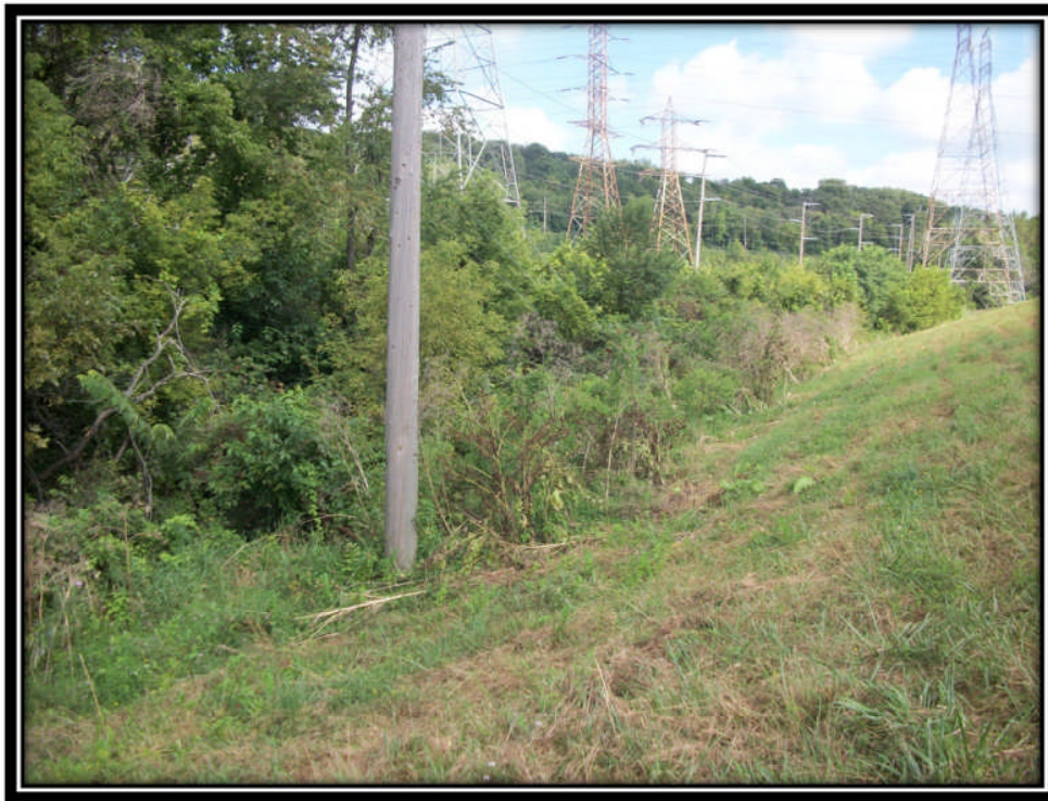
Photo 29 – Electric Line Penetration near Toe of Downstream Embankment
