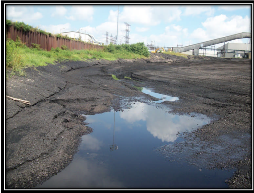
Photo 45 – Storm Water Channel between Coal Pile and Floodwall (Possible Seep Location)
