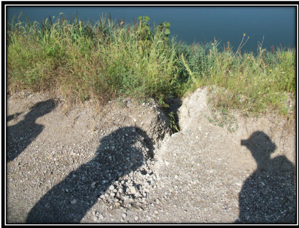
Photo 13 – Minor Erosion on Crest of Clarification Pond (Typical of Ash Pond and Clarification Pond)
