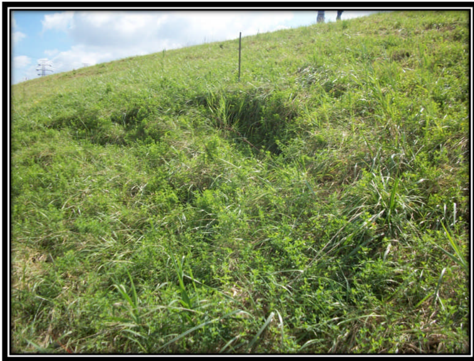
Photo 37 – Scarp on Western Pond 1 Downstream Slope Approximately 18"-24" Deep
