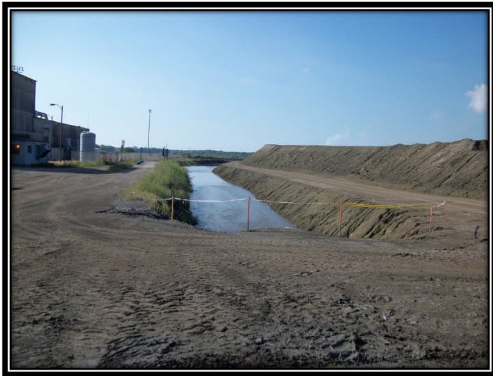
Photo 3 – Active Ash Pond Settling Channel
