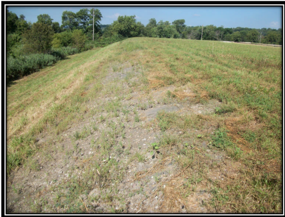
Photo 20 – Sparse Vegetation on Crest and Downstream Slope of Southern Embankment
