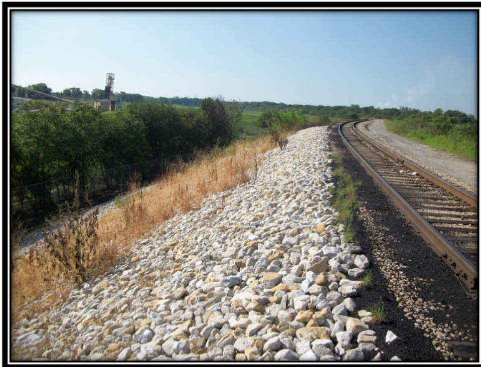
Photo 12 – Riprap and Railroad Tracks at Crest of Clarification Pond Embankment
