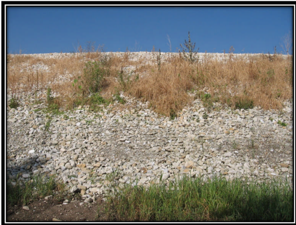
Photo 10 – Vegetated Riprap on Embankment Slope (Typical)
