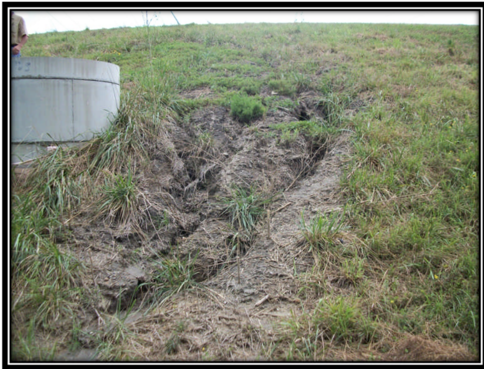
Photo 31 – Erosion Greater Than 12” Present at Sides of Waste Water Sewer Manhole
