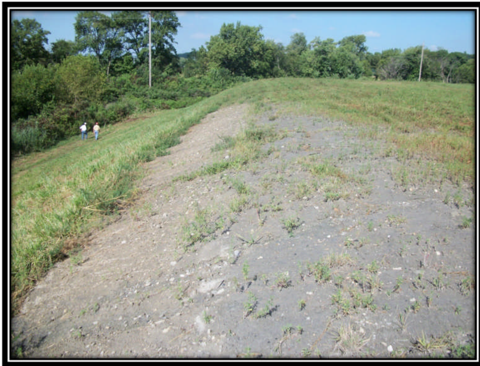
Photo 19 – Sparse Vegetation on Crest and Downstream Slope of Southern Embankment
