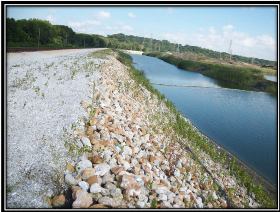
Photo 26 –Clarification Pond Inlet Channel with Riprap (Note Ash Pond Settling Channel Inlets)
