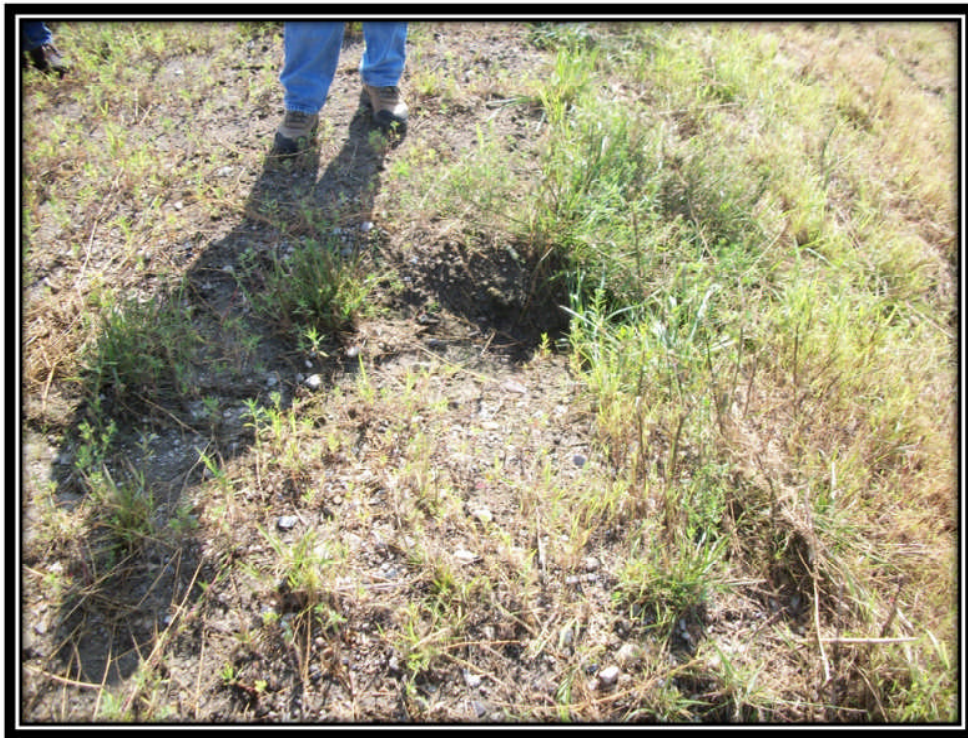
Photo 21 – Erosion on Southern Downstream Slopes and Crest (Typical)
