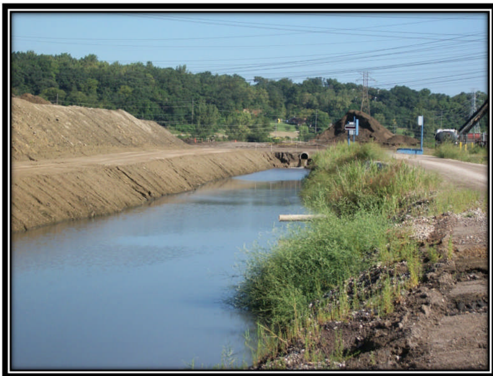
Photo 4 – Active Intake Pipe and Ash Settling Channel
