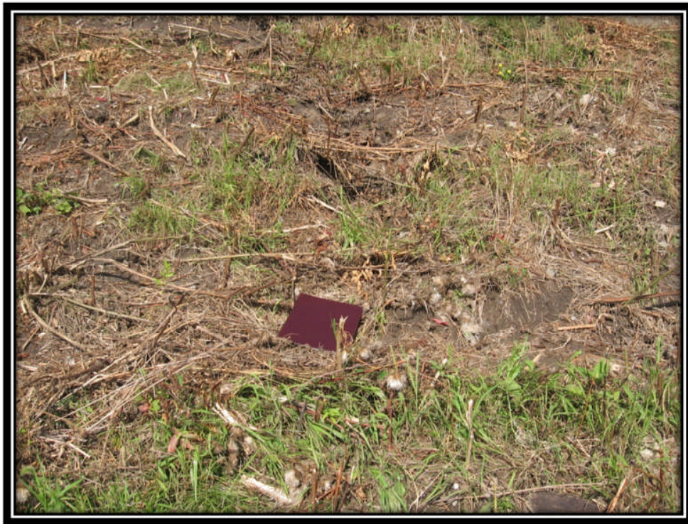
Photo 15 – Area of Sparse Vegetation and Erosion on Embankment Slope and Toe
