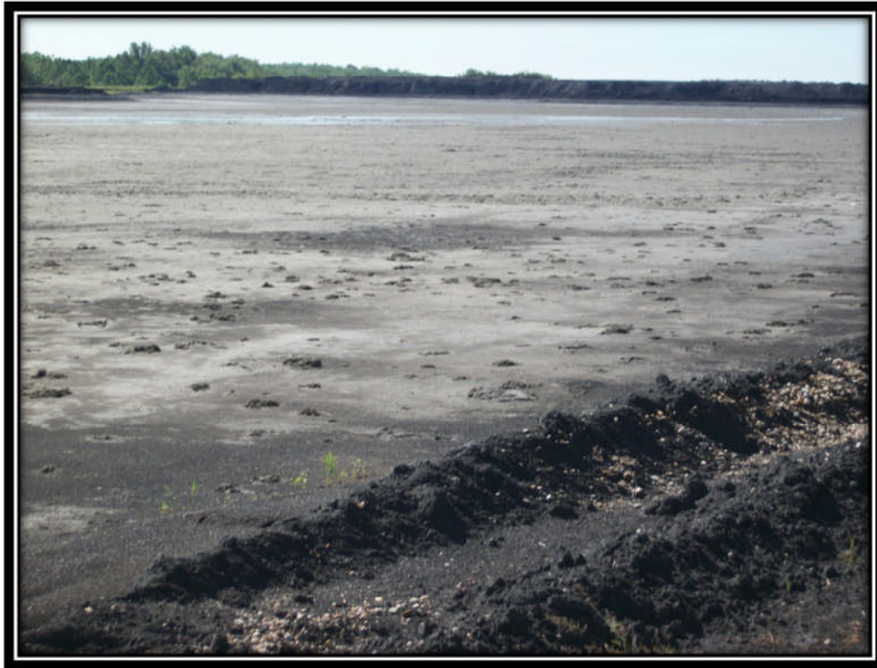
Photo 23 – Ash Pond 2 in the Process of being Drained and Decommissioned
