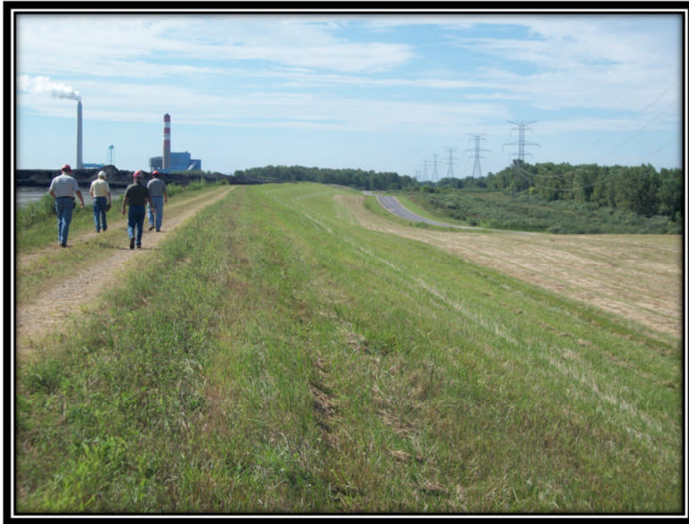
Photo 31 – Western Embankment Crest of Ponds 1 and 2 (Typical)
