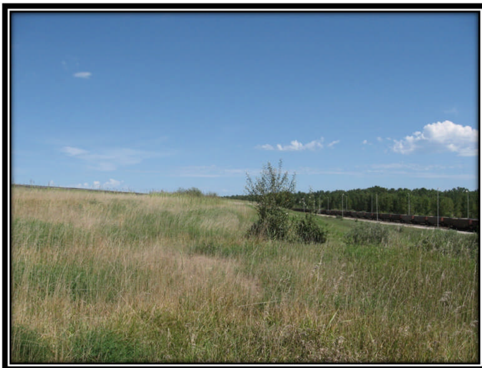
Photo 40 – Woody Vegetation on Eastern Slope of Pond 1 Embankment (Note Lack of Mowing)
