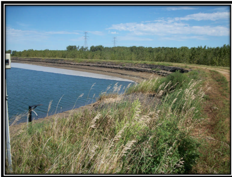
Photo 18 – Northeast Corner of Ash Pond 2 (Note Draw Down and Current Freeboard)
