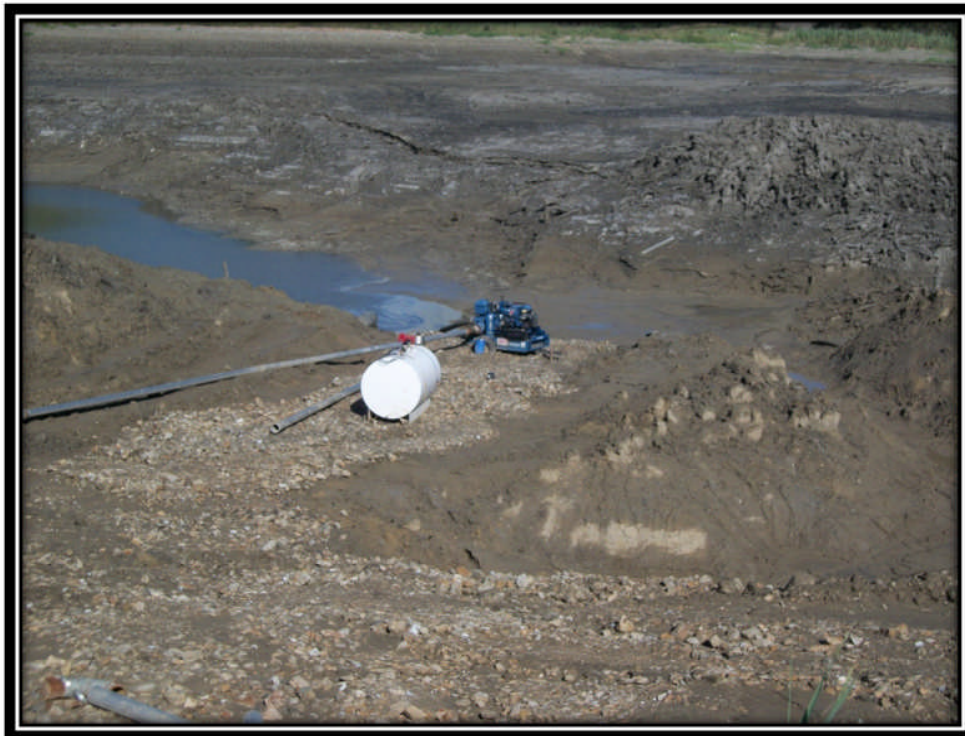
Photo 8 – Pumping Operations to Remove Remaining Water from Recycle Pond
