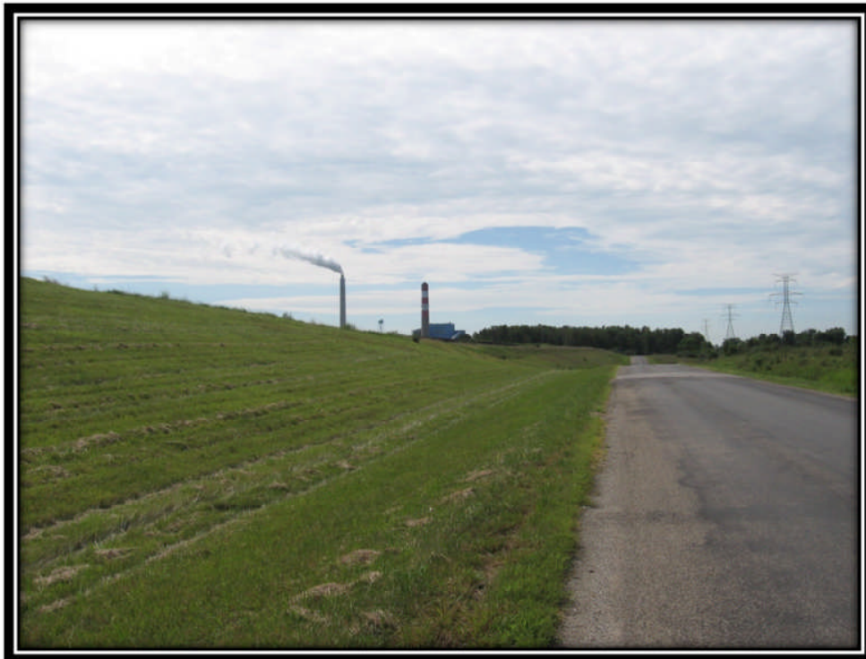
Photo 36 – Typical Western Embankment of Ponds 1 & 2 Looking South
