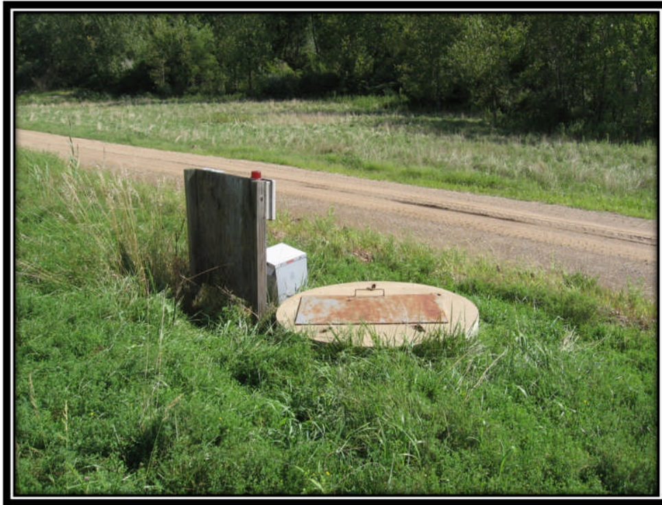
Photo 13 – Pump Station at Seepage Blanket
