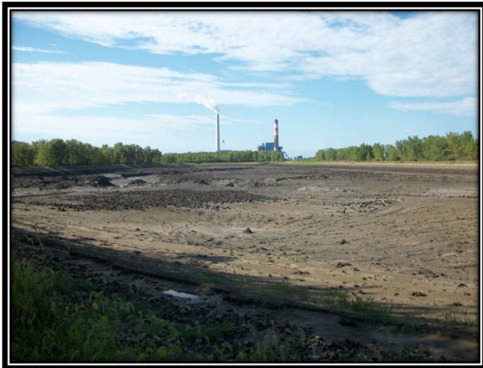
Photo 2 – Typical Condition of Recycle Pond in the Process of Being Decommissioned Looking South
