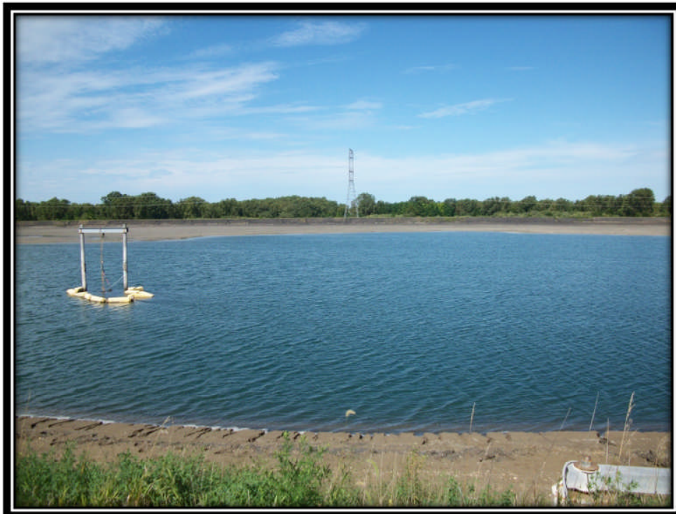
Photo 14 – Outlet Works of Pond 2 and Remaining Impoundment Level
