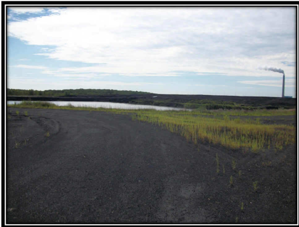
Photo 26 – Junction of Ash Ponds 1 and 2 Looking Southeast
