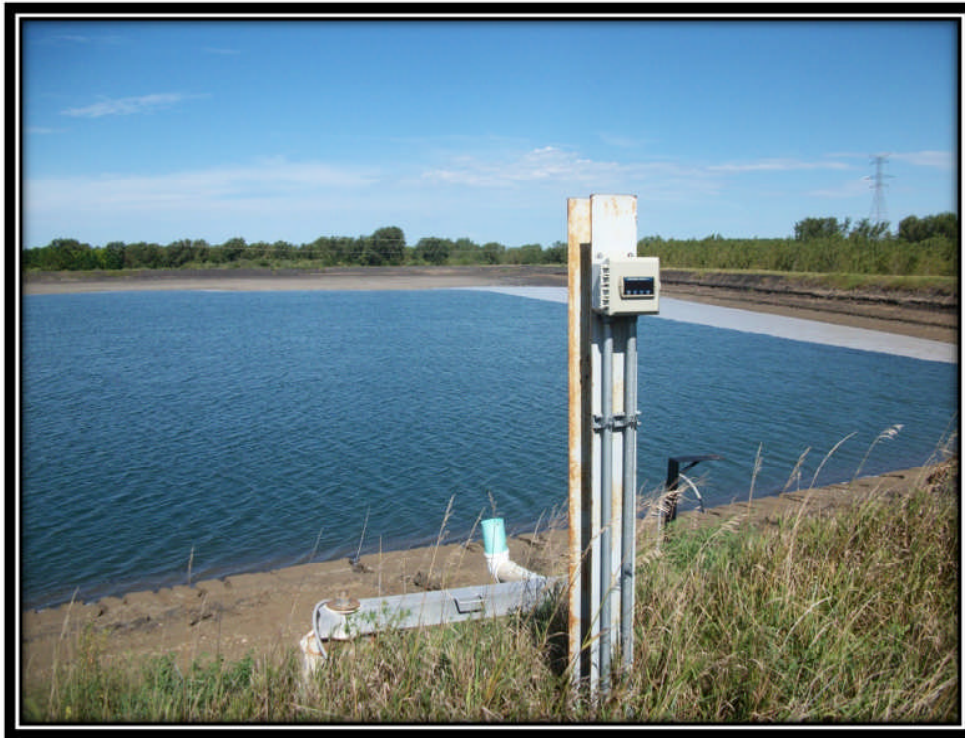
Photo 17 – Electric Control Penetration in Crest near Pond 2 Outlet Works and Seepage Blanket
