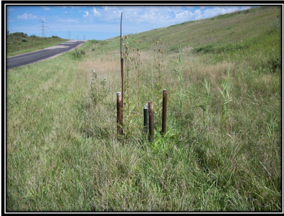
Photo 35 – Monitoring Well at the Downstream Toe of the Western Embankment of Pond 1
