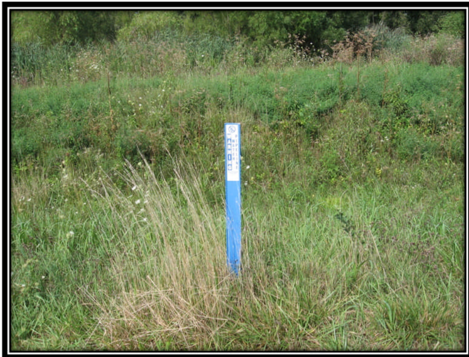
Photo 28 – Buried Water Line Marker at Junction of Ponds 1 and 2 at Toe of Western Embankment
