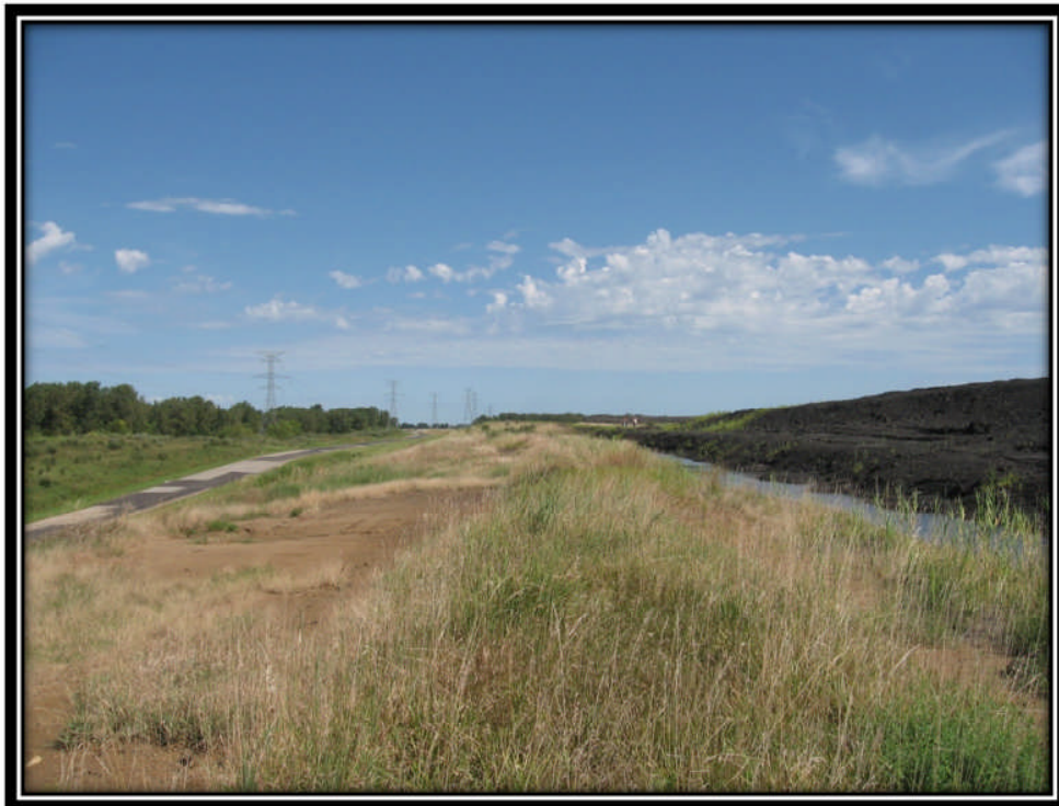
Photo 32 – Ash Pond 1 Crest and Settling Channel from Western Embankment Crest Looking North
