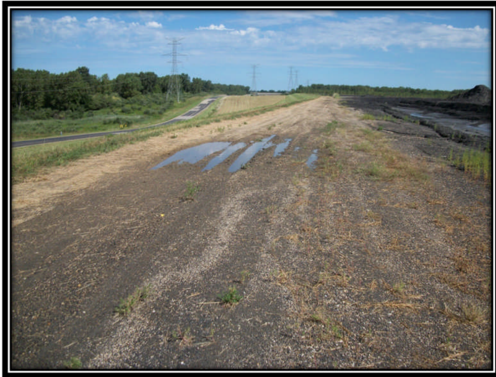
Photo 25 – Slight Rutting and Ponding of Storm Water on Western Embankment Crest (Typical)
