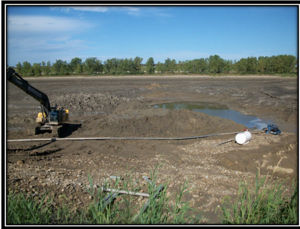
Photo 7 – Pumping Operations to Remove Remaining Water from Recycle Pond
