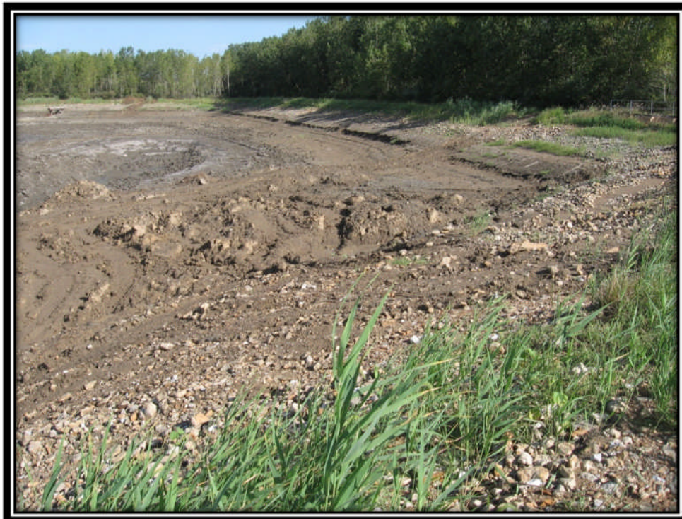
Photo 4 – Recycle Pond Looking Northwest (Note Inlet Pipe in Background)
