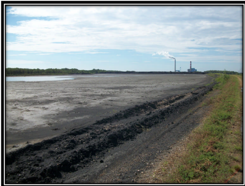
Photo 24 – Ash Pond 2 in the Process of being Drained and Decommissioned
