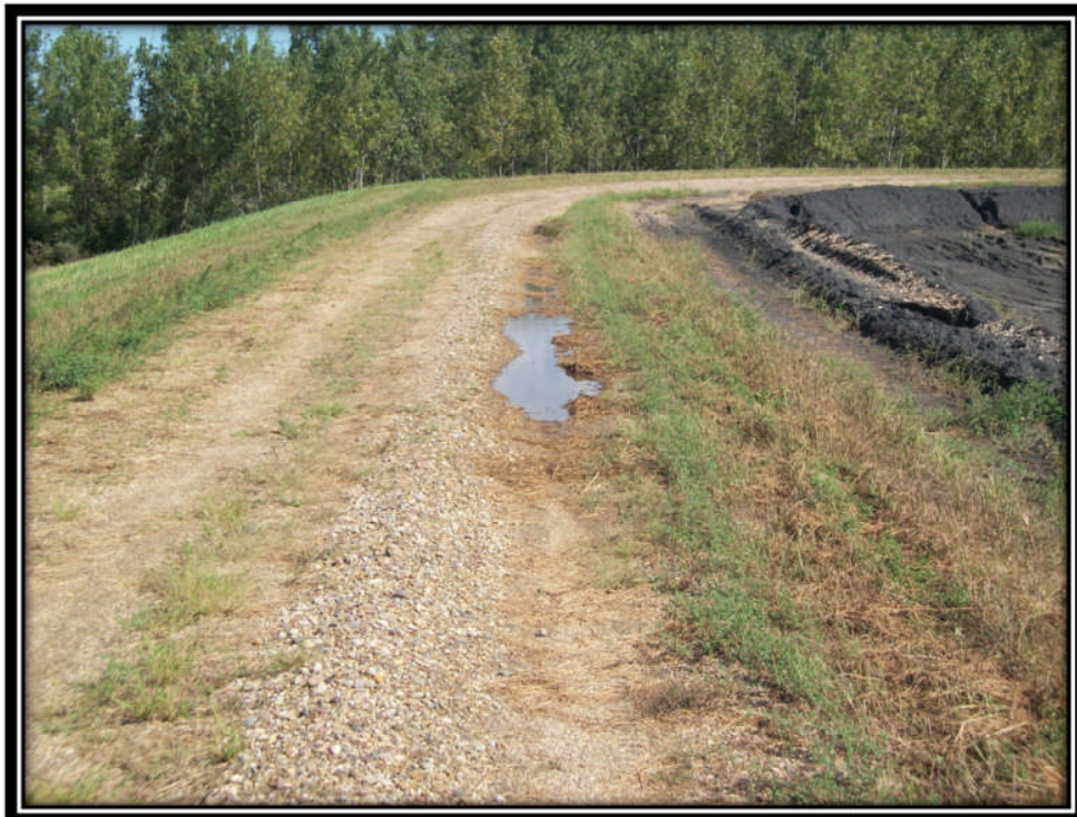
Photo 22 – Slight Rutting and Ponding of Storm Water on Western Crest of Pond 2
