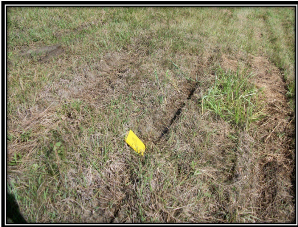
Photo 10 – Possible Slight Seepage Area near Eastern Embankment Toe (Note Rutting)
