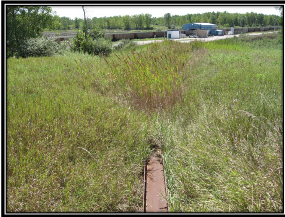
Photo 41 – Tall Grass and Similar Vegetation on Eastern Slope of Pond 1 Embankment (Note Debris)
