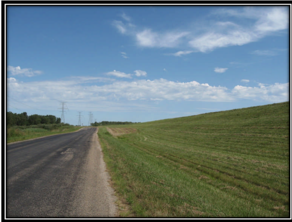
Photo 37 – Typical Western Embankment of Ponds 1 & 2 Looking North
