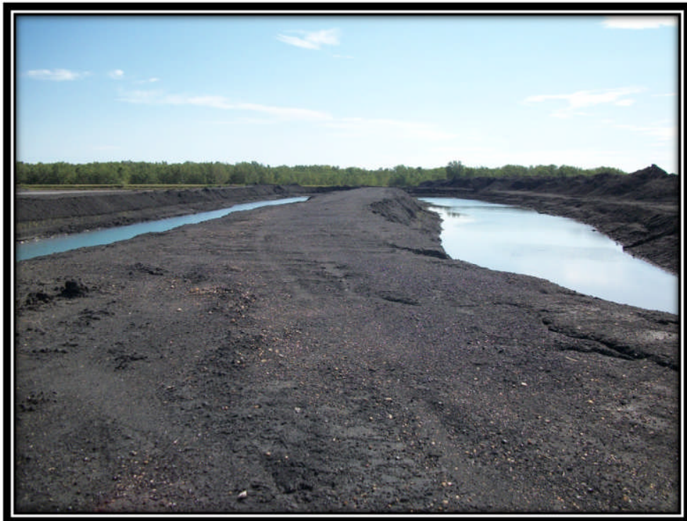
Photo 30 – Ash Pond 1 Settling Channel
