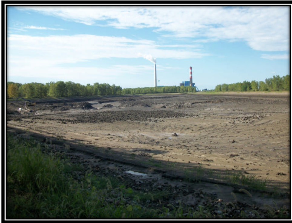
Photo 3 – Typical Condition of Recycle Pond (Note Pumping Operations in Background)
