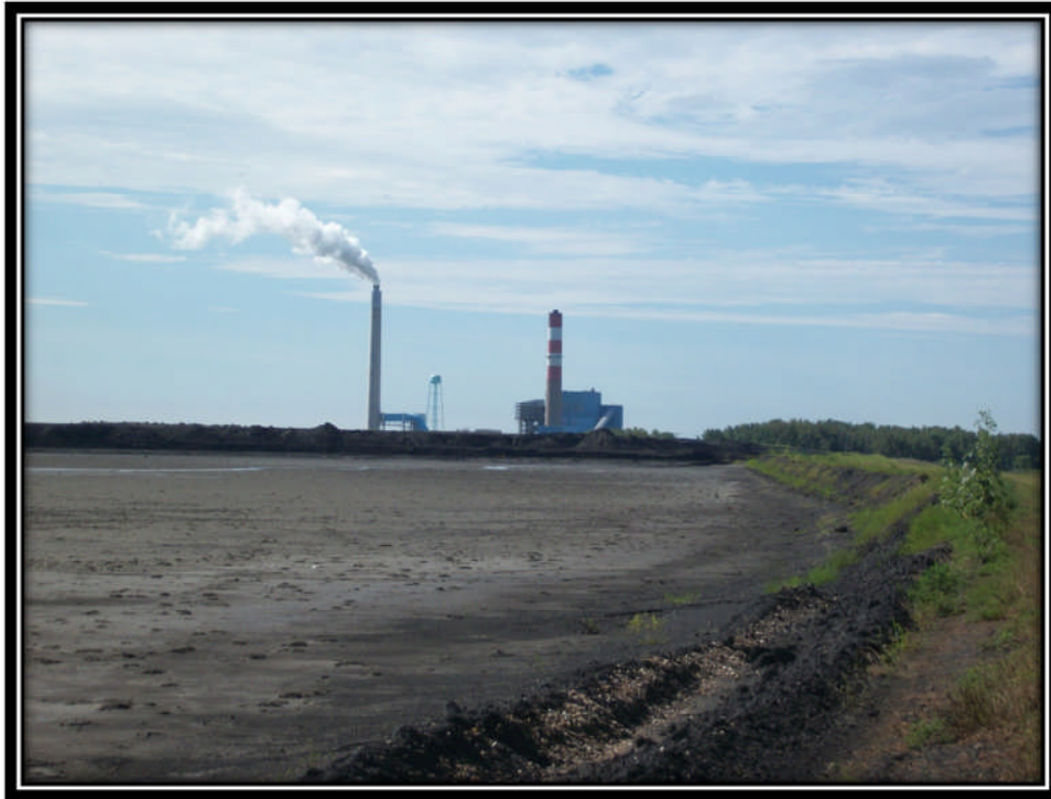
Photo 21 – Ash Pond 2 Looking South along the Western Upstream Embankment
