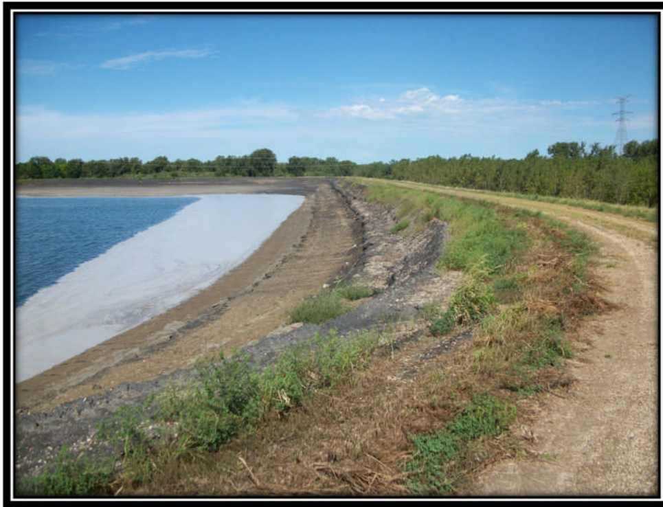
Photo 19 – Typical Upstream Slope of Northern Embankment of Pond 2 Looking West
