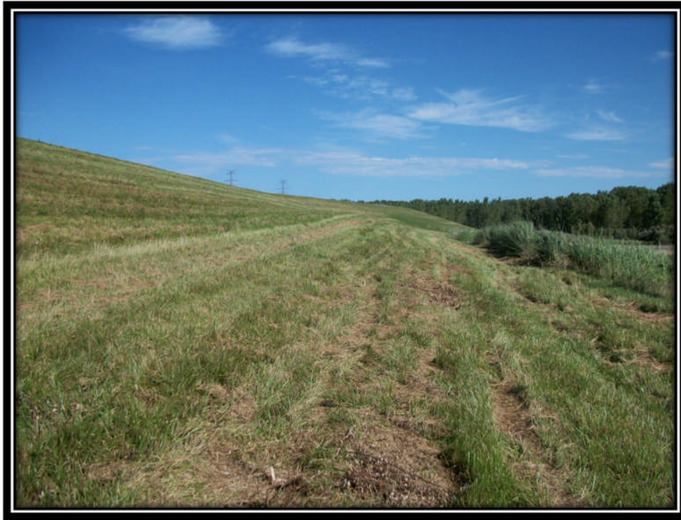
Photo 9 – Eastern Embankment Pond 2 (Note Drainage Blanket and Benched Section in Background)
