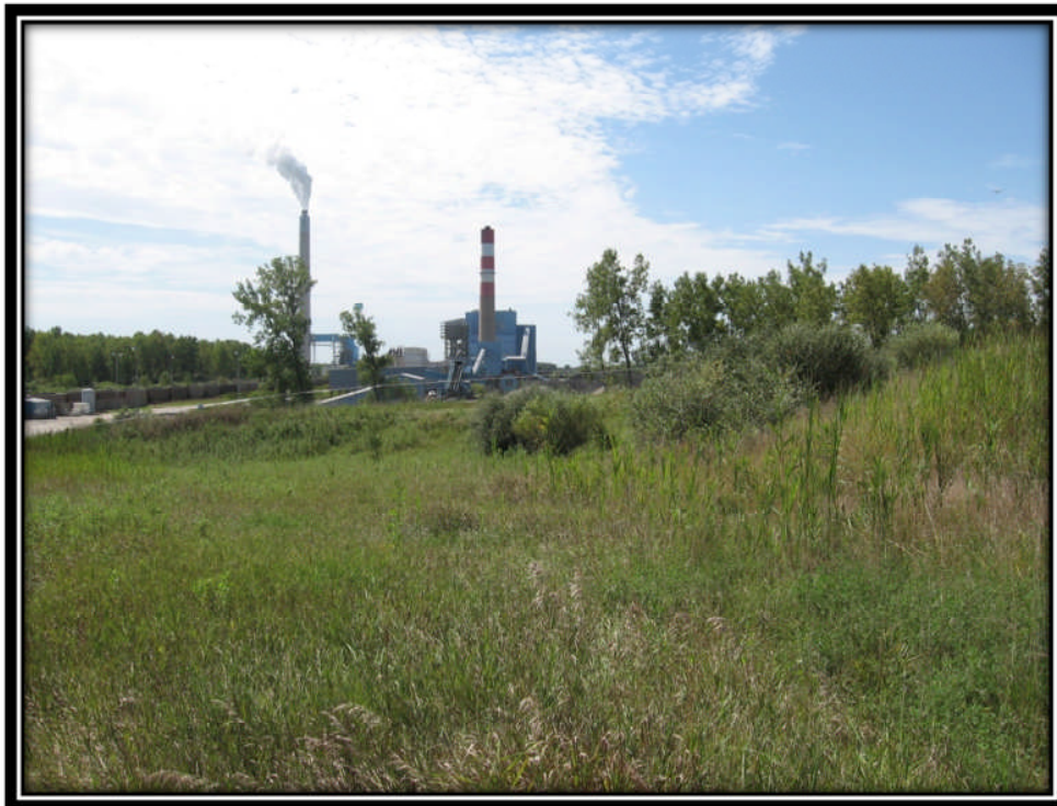
Photo 42 –Vegetation on Eastern Slope of Pond 1 Embankment (Note Lack of Mowing)
