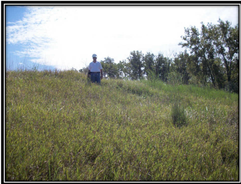
Photo38 – Surface Erosion Approximately 2' deep by 3' Wide on the Southwestern Corner of Pond 1
