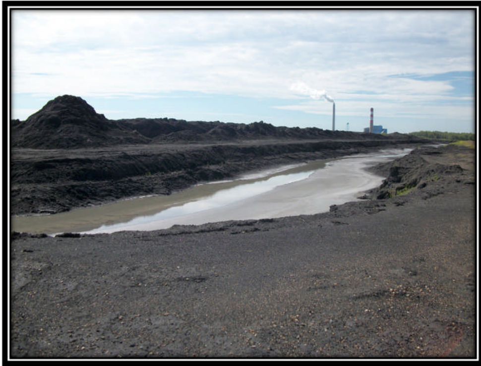
Photo 29 – Ash Pond 1 Settling Channel
