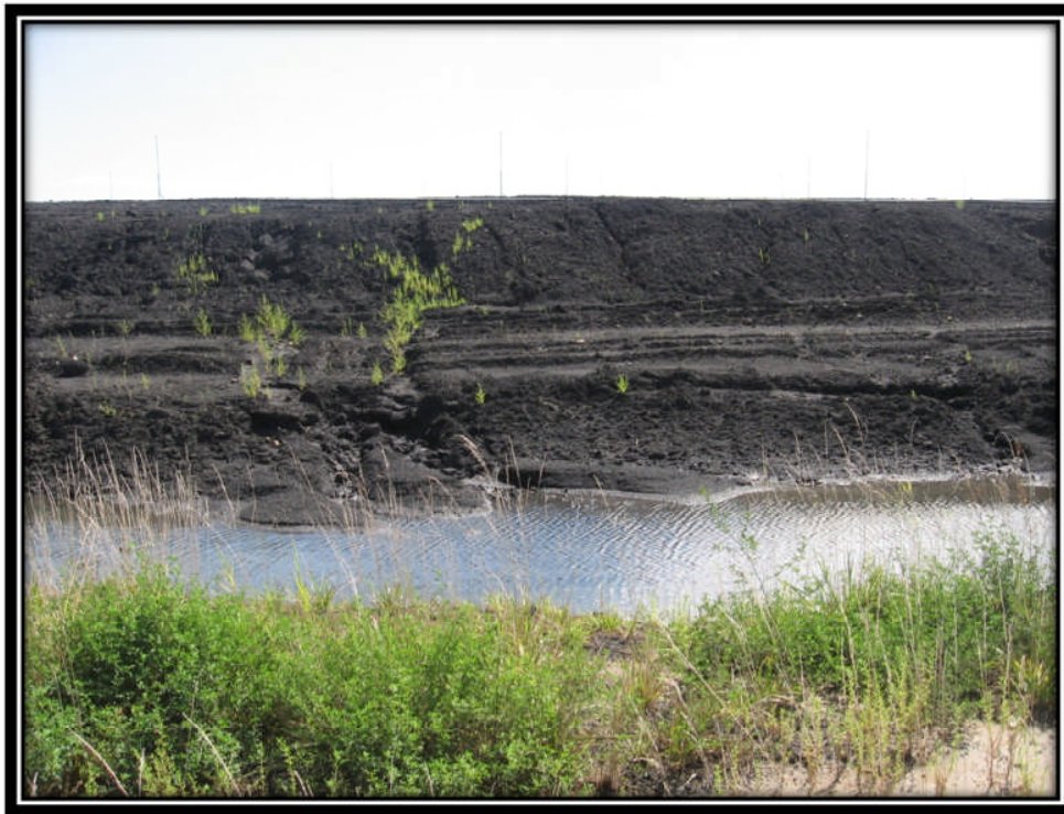
Photo 33 – Ash Pond 1 Settling Channel from Western Embankment Crest Looking East
