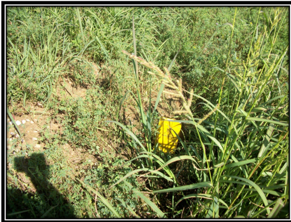
Photo 12 – Surface Erosion near Toe of Eastern Embankment of Ash Pond 2
