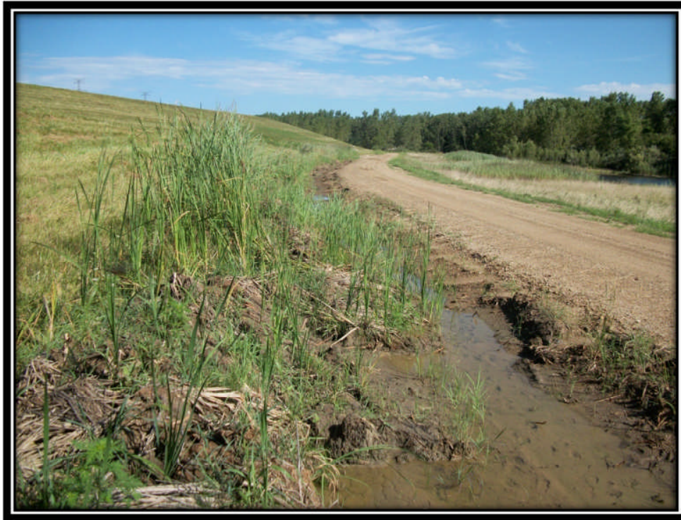
Photo 11 – Ponding of Storm Water at Toe of Eastern Embankment between Road and Ash Pond 2
