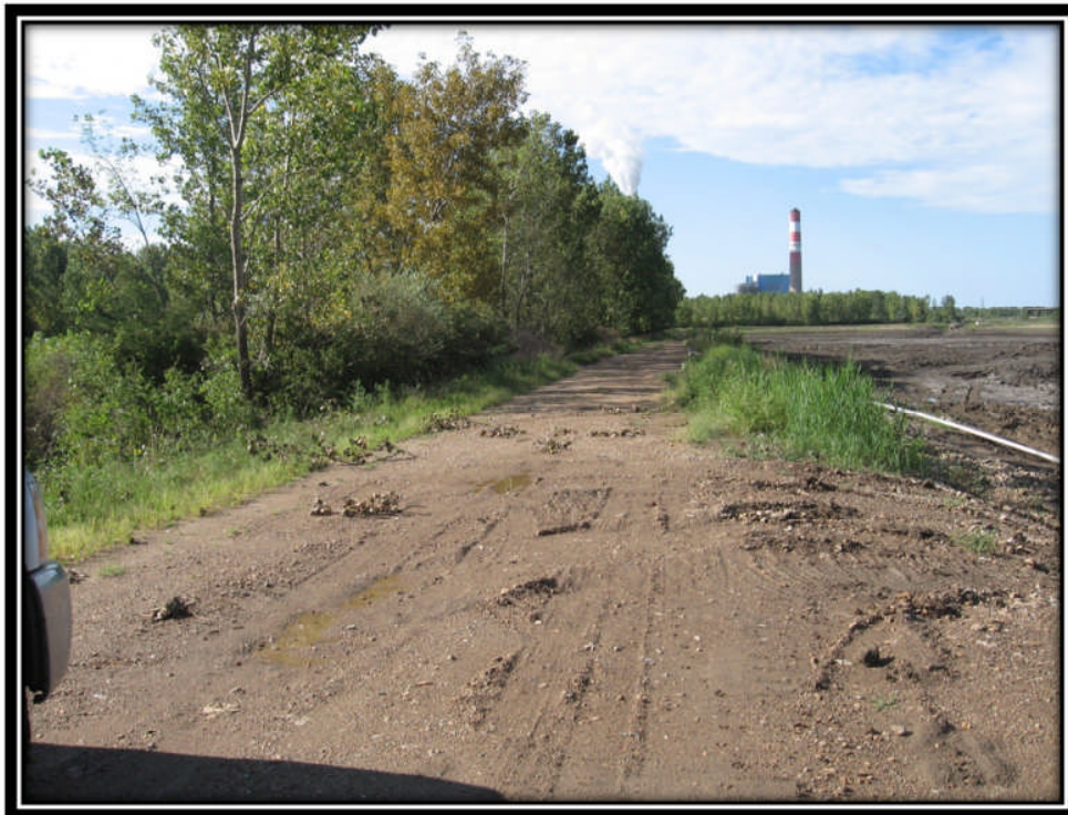
Photo 6 – Typical Crest Condition of Recycle Pond
