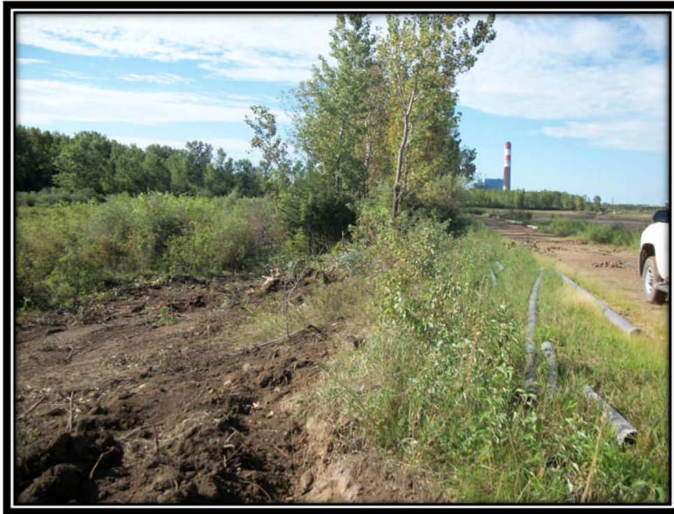
Photo 5 – Clearing Operations in Preparation of Recycle Pond Decommissioning
