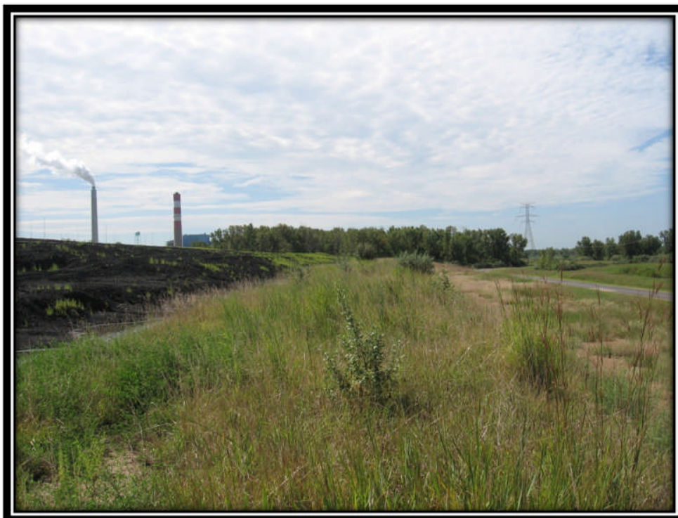
Photo 34 – Ash Pond 1 Crest and Settling Channel from Western Embankment Crest Looking South
