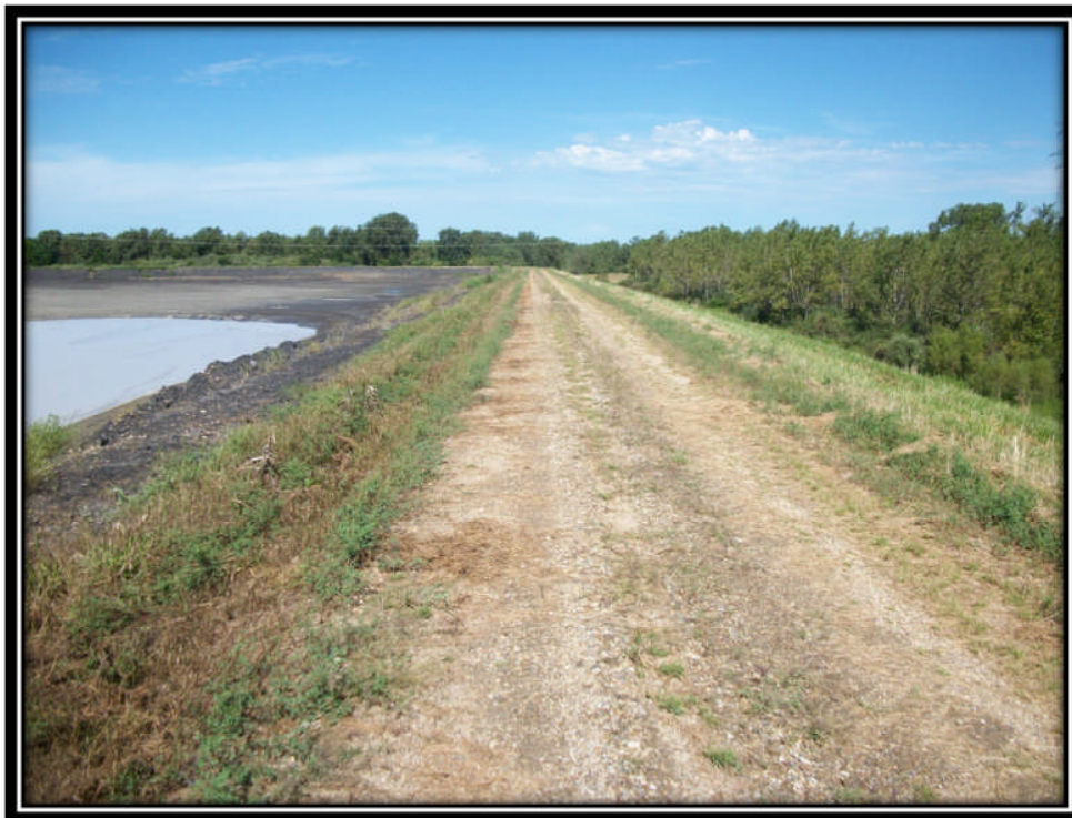
Photo 20 – Northern Embankment of Pond 2 Looking West Showing the Typical Crest Condition
