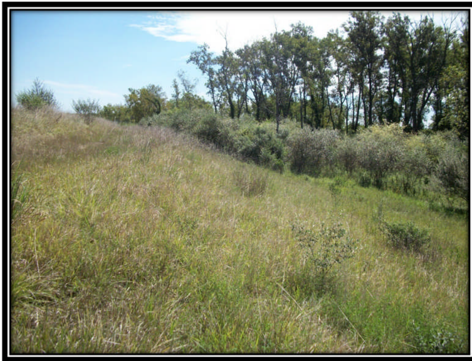
Photo 39 – Vegetation Greater than 1" in Diameter on the Southern Embankment of Pond 1 (Typical)
