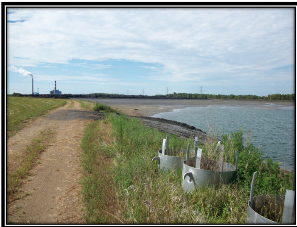
Photo 16 – Pond 2 Crest Looking South with Outlet Pipe Risers in Foreground
