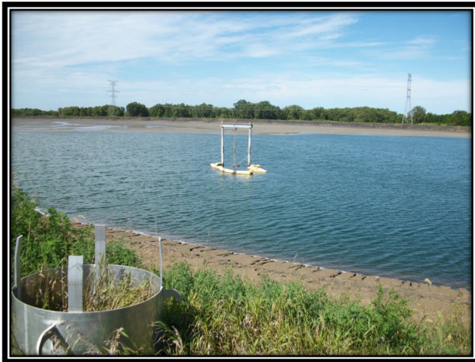
Photo 15 – Outlet Works of Pond 2 with Outlet Pipe Risers in Foreground
