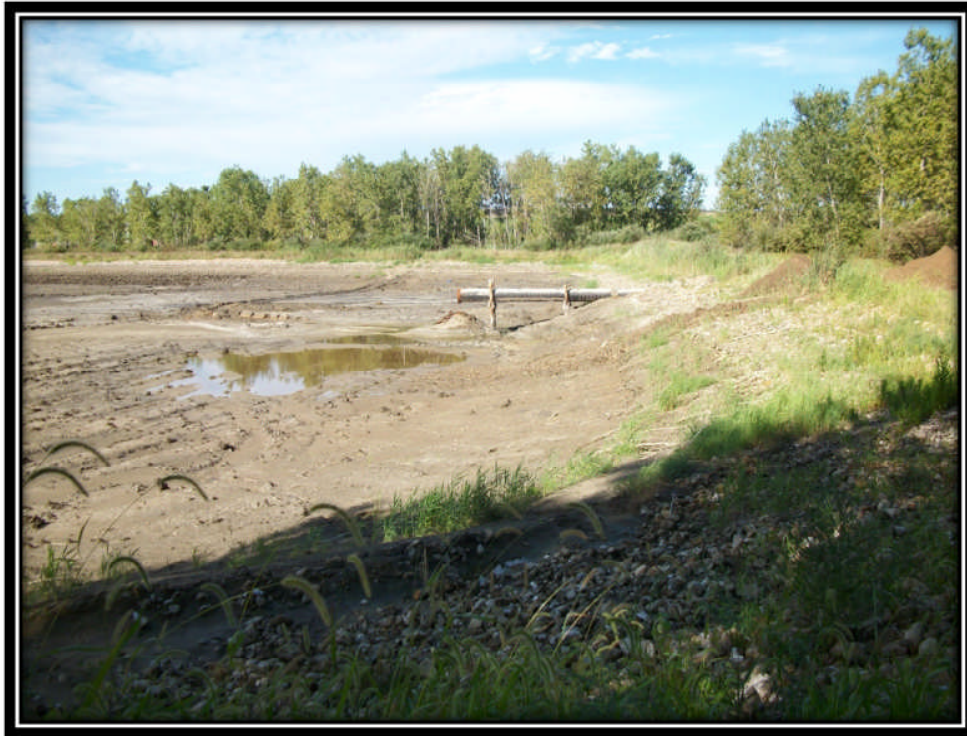
Photo 1 – Recycle Pond Inlet Pipe
