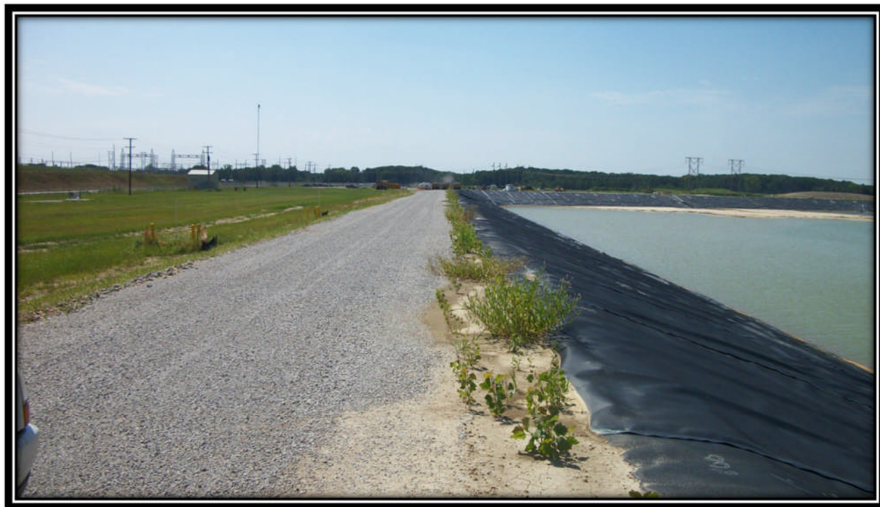
Photo 32 – Looking West along South embankment
