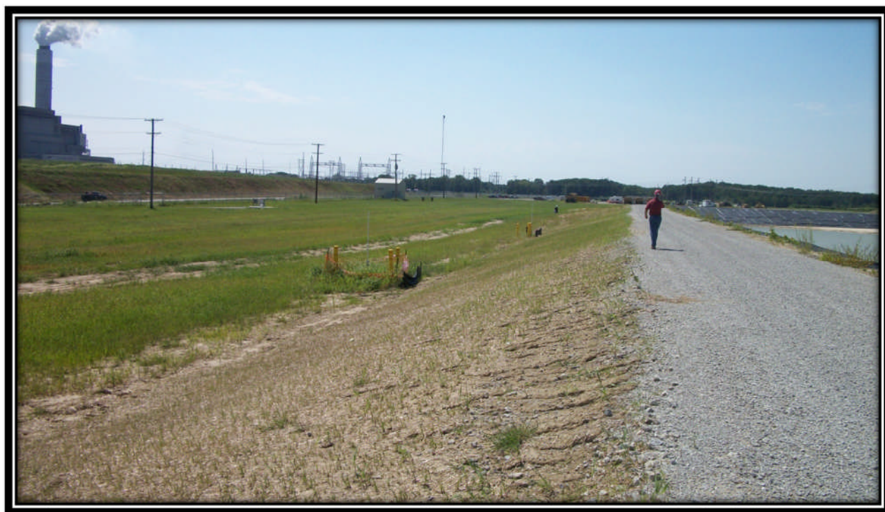
Photo 36 – Looking West along downstream slope of South embankment
