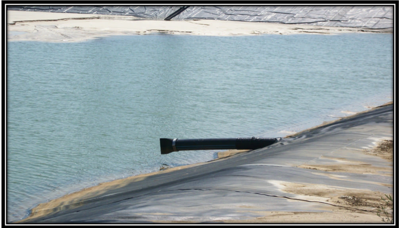
Photo 41 – Pipe between larger and smaller pond
