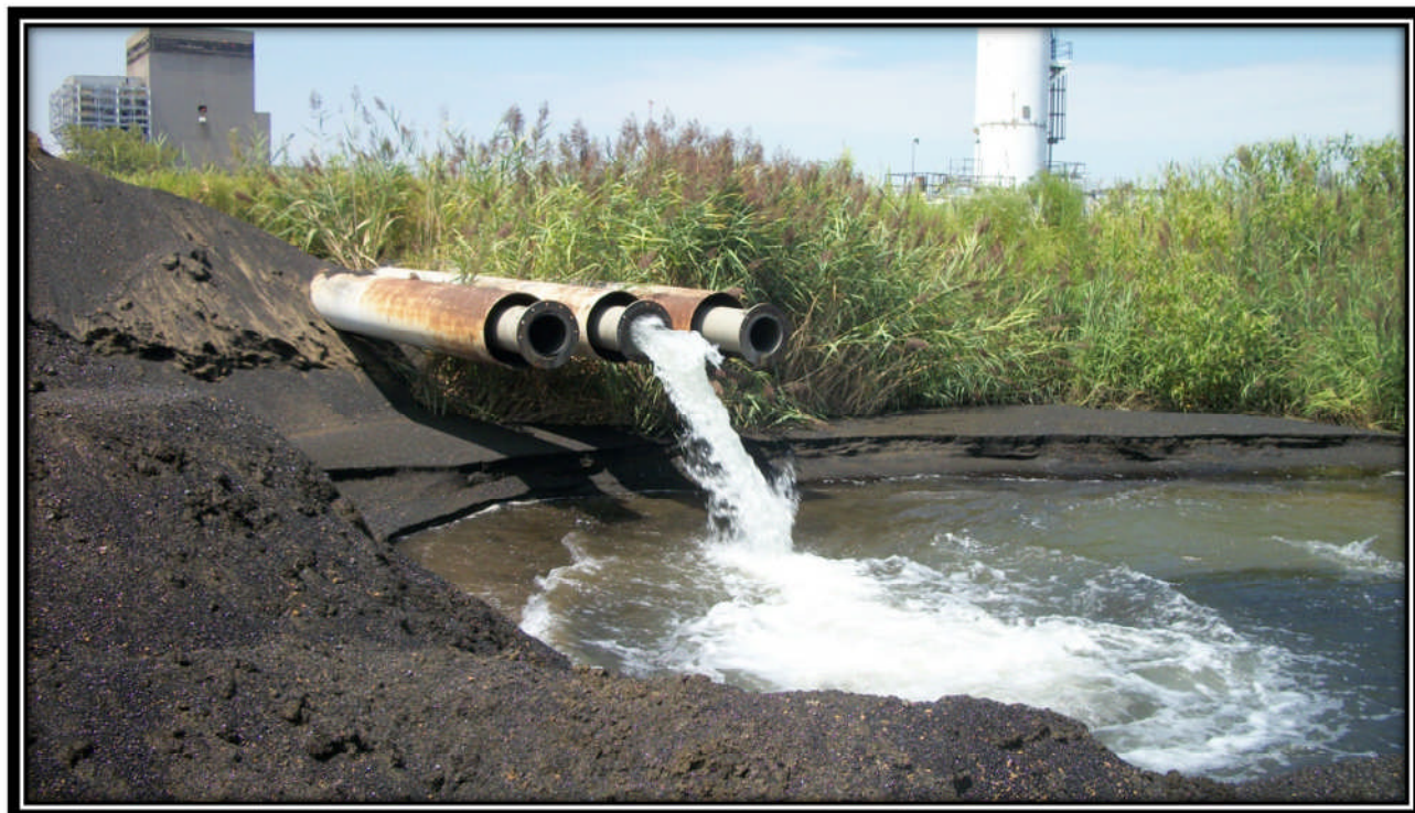
Photo 31 – Ash pond discharge outlet pipes
