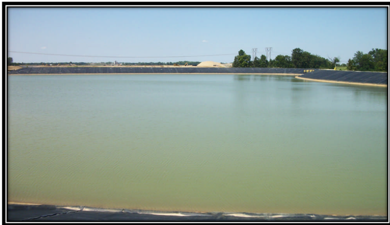
Photo 34 – Looking North from South embankment
