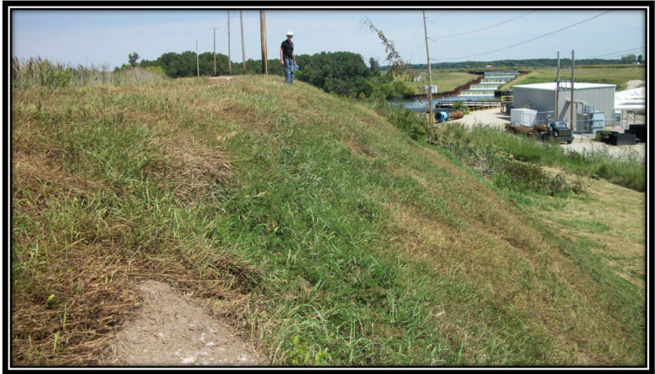
Photo 11 – East embankment looking North with minimal scarps
