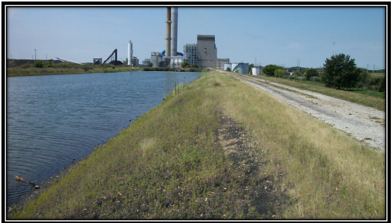
Photo 20 – Looking West along North embankment at the upstream slope
