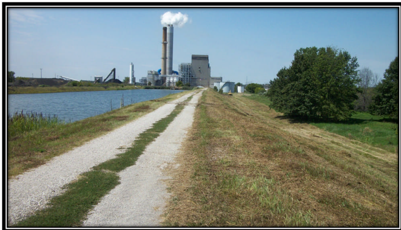
Photo 18 – Looking West along North embankment at the crest
