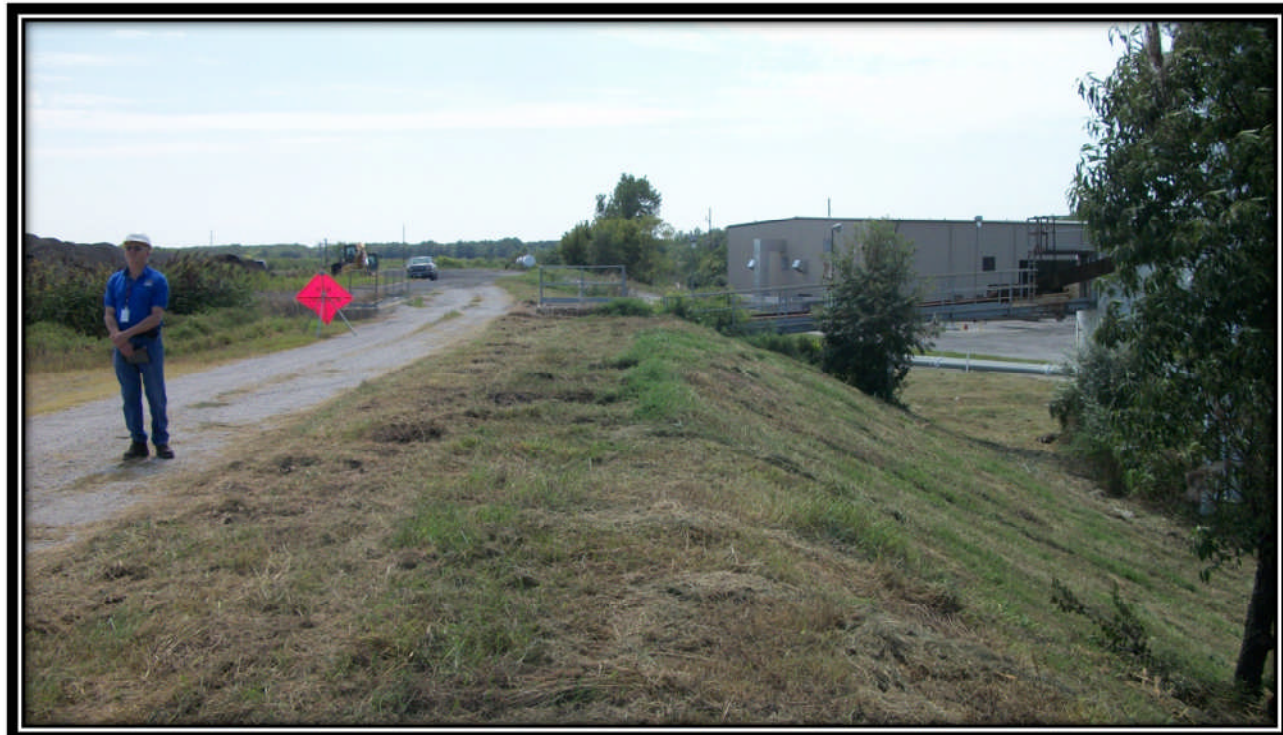
Photo 29 – Looking South along West embankment
