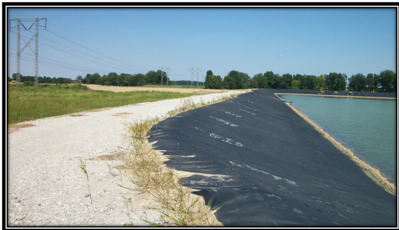
Photo 38 – Looking East along North embankment
