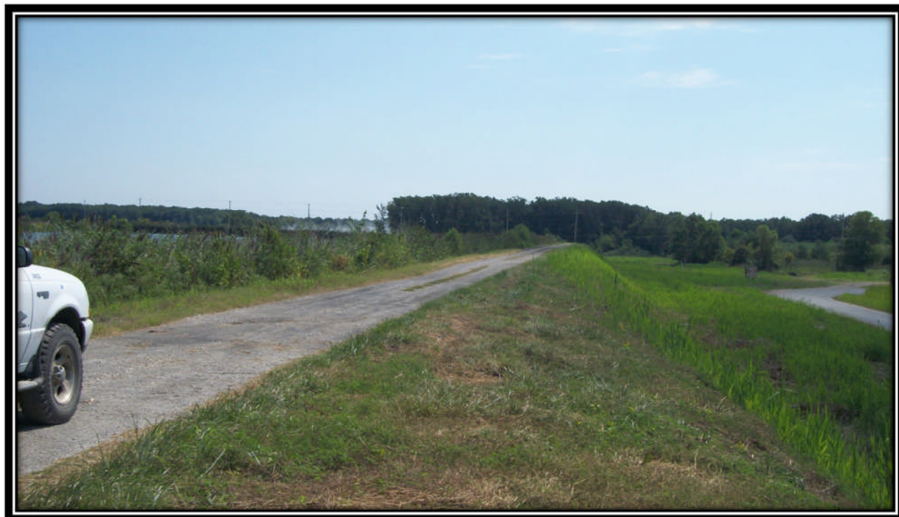
Photo 1 – Looking East along South embankment
