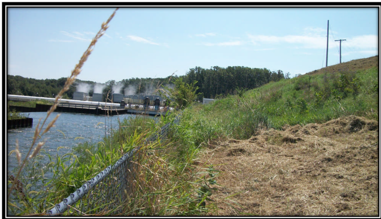
Photo 16 – Downstream of Northeast corner to sheetpile wall
