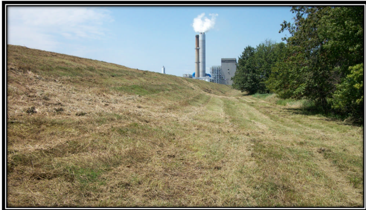
Photo 17 – Looking West along North embankment at the downstream slope
