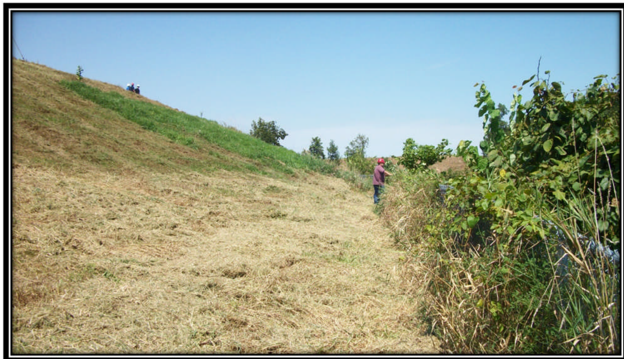
Photo 15 – Downstream of Northeast corner to sheetpile wall
