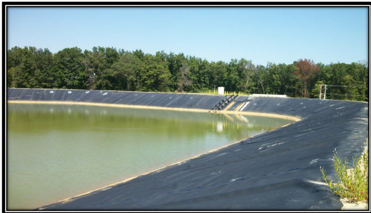
Photo 33 – Looking East from South embankment
