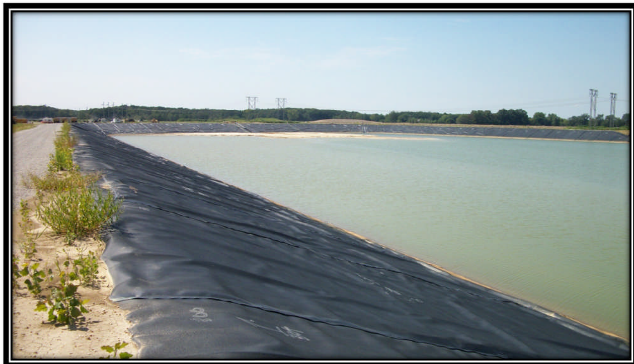
Photo 35 – Looking West from South embankment
