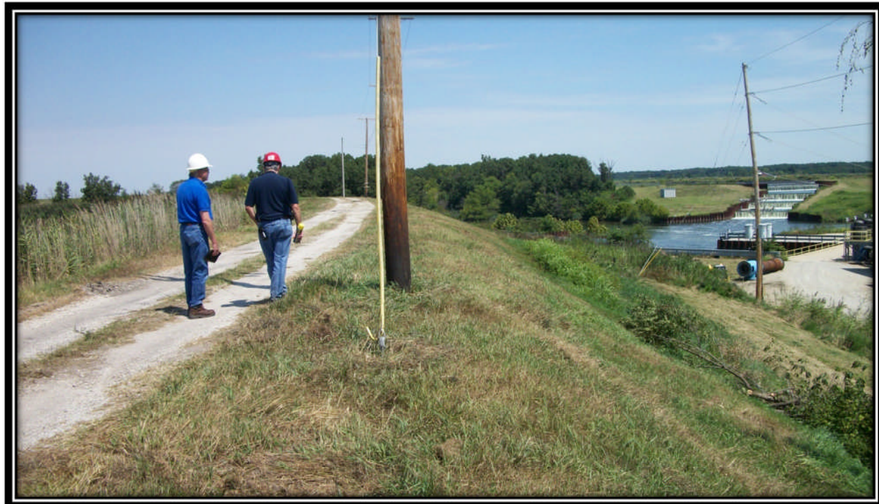
Photo 13 – Looking North on East embankment
