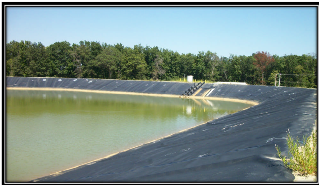
Photo 33 – Looking East from South embankment
