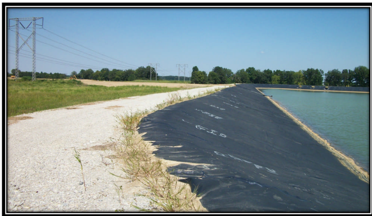
Photo 38 – Looking East along North embankment
