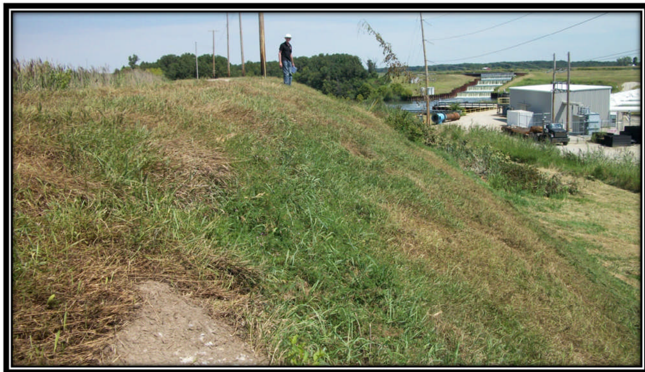
Photo 11 – East embankment looking North with minimal scarps
