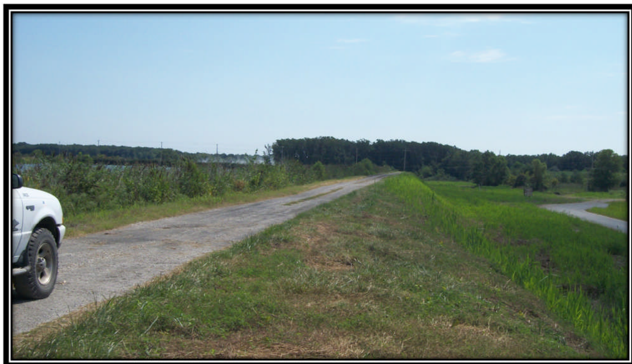
Photo 1 – Looking East along South embankment
