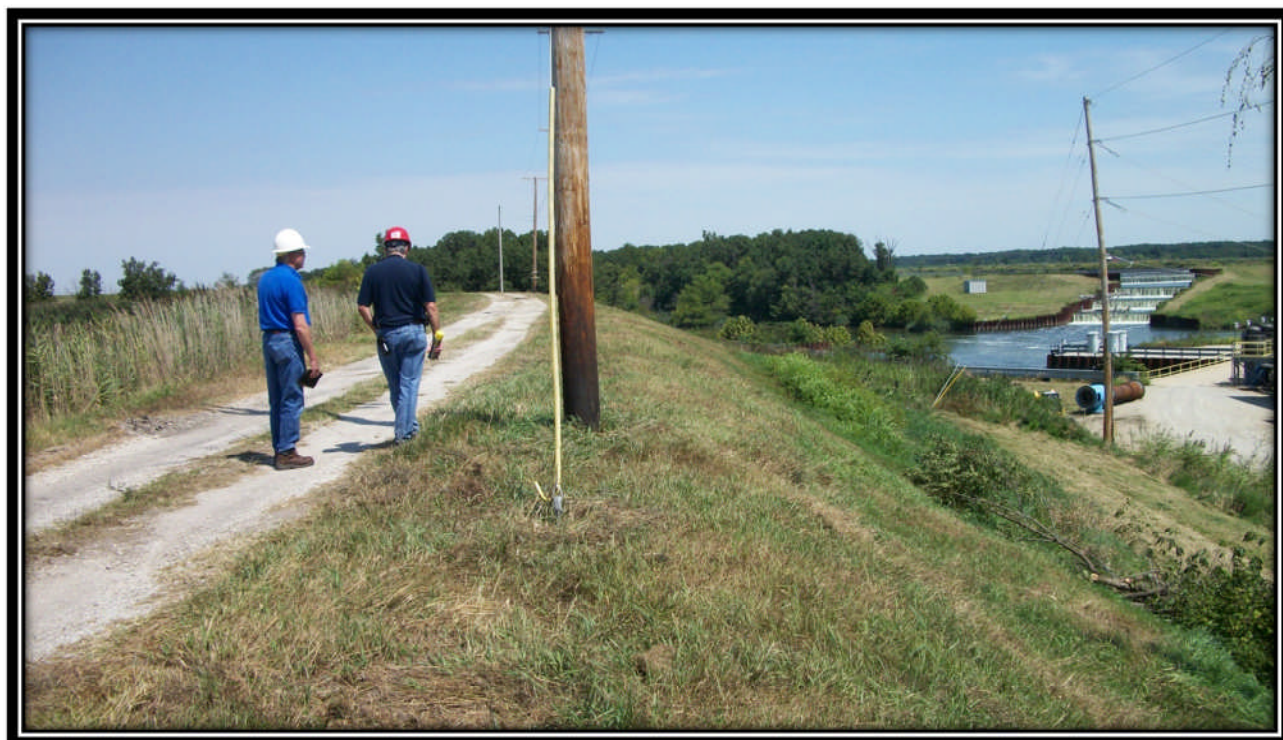
Photo 13 – Looking North on East embankment
