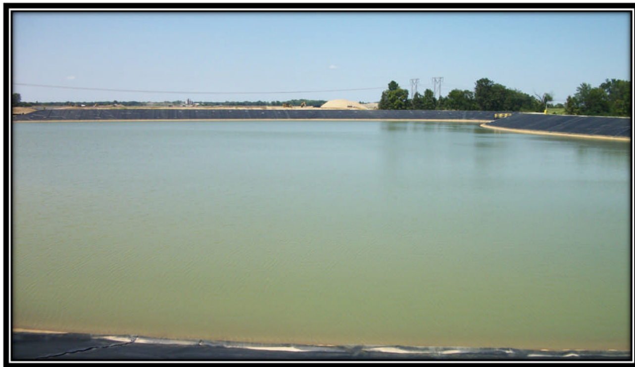
Photo 34 – Looking North from South embankment
