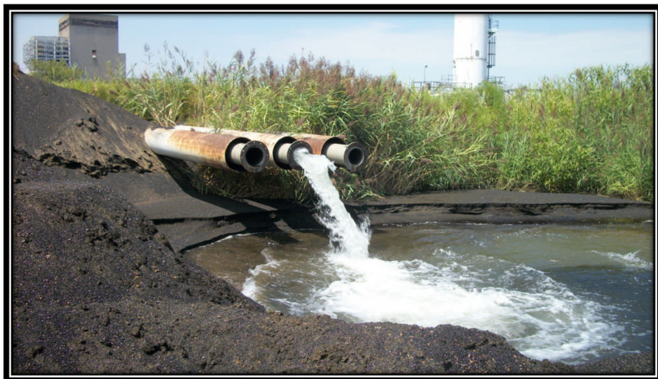
Photo 31 – Ash pond discharge outlet pipes
