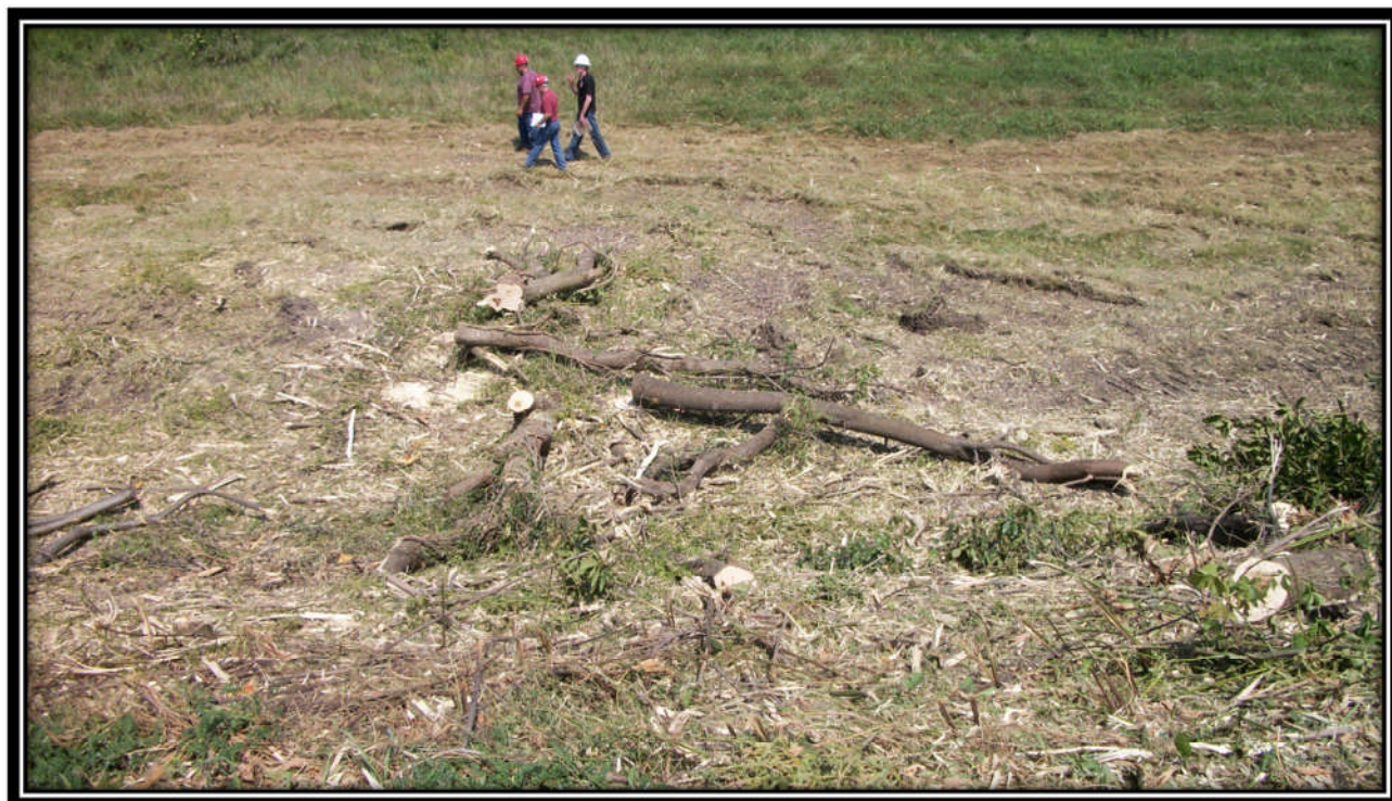
Photo 22 – Debris on downstream slope of North embankment
