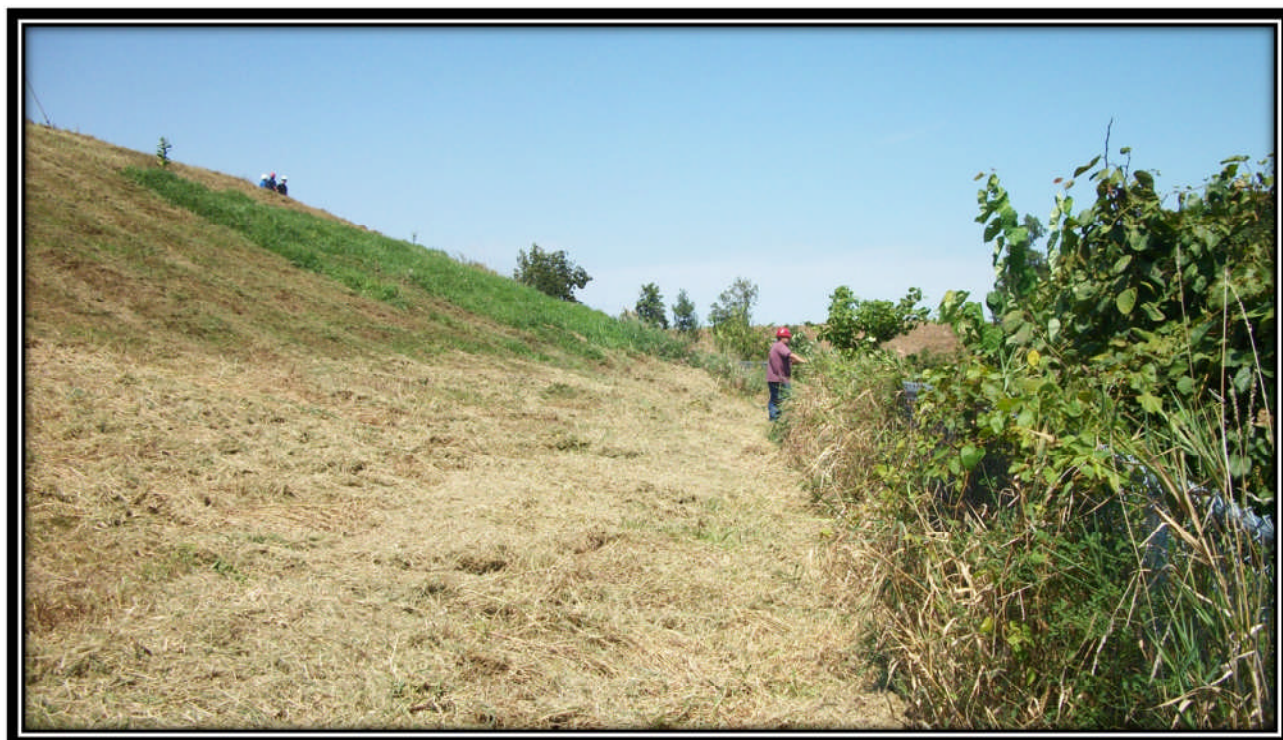
Photo 15 – Downstream of Northeast corner to sheetpile wall
