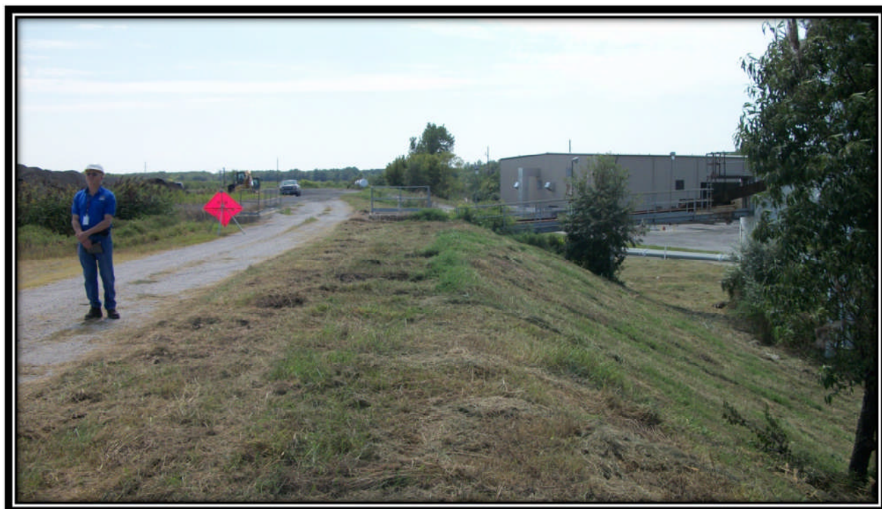
Photo 29 – Looking South along West embankment
