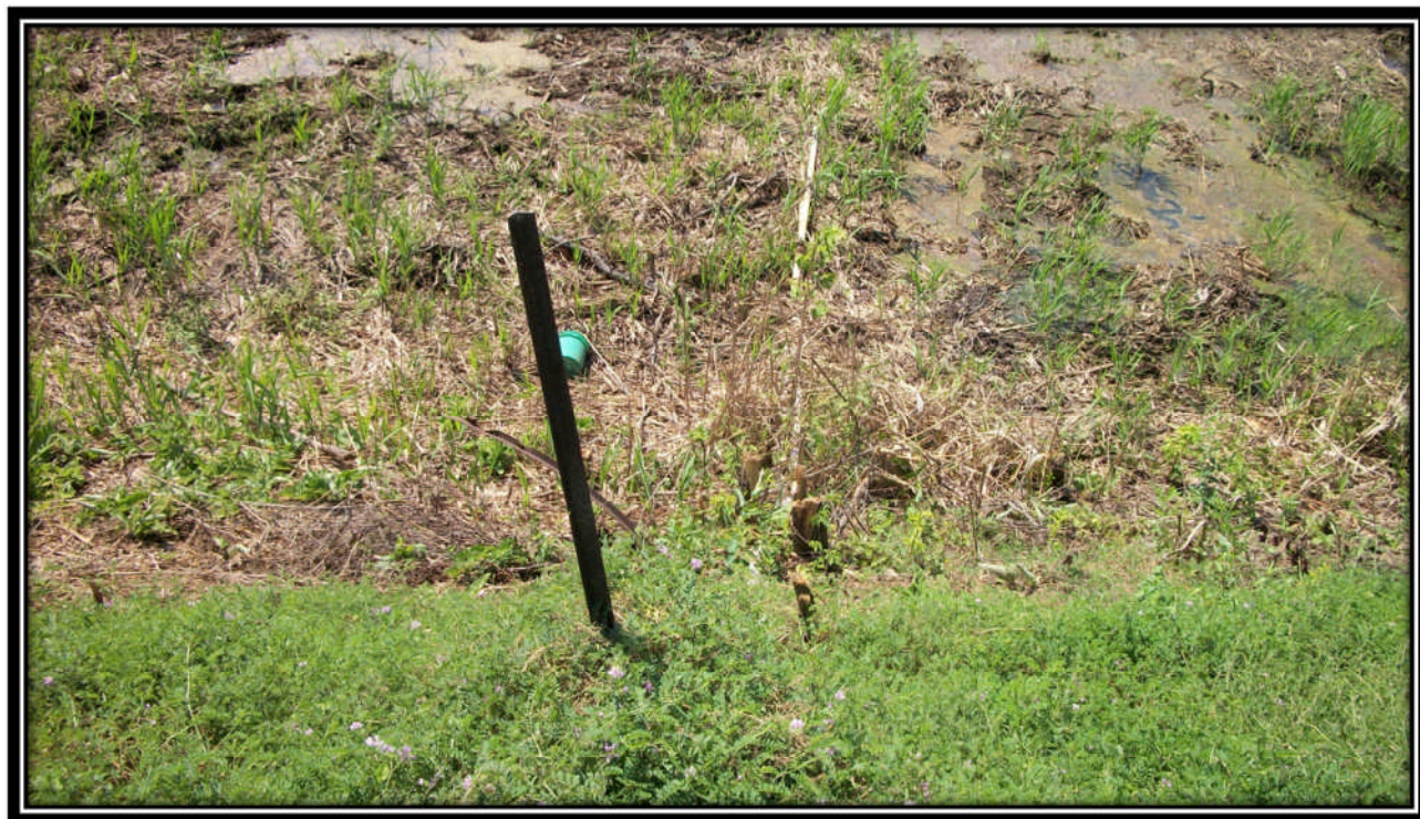
Photo 9 – Abandoned pump crossing
