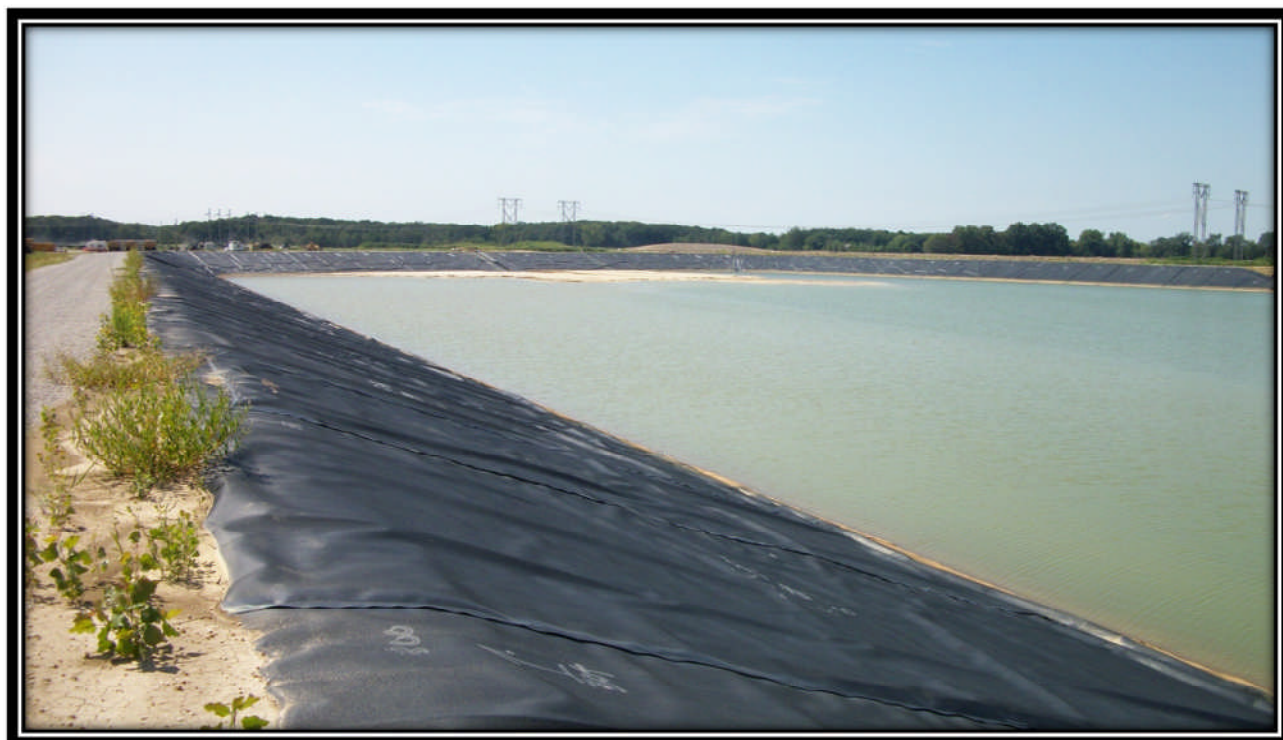
Photo 35 – Looking West from South embankment
