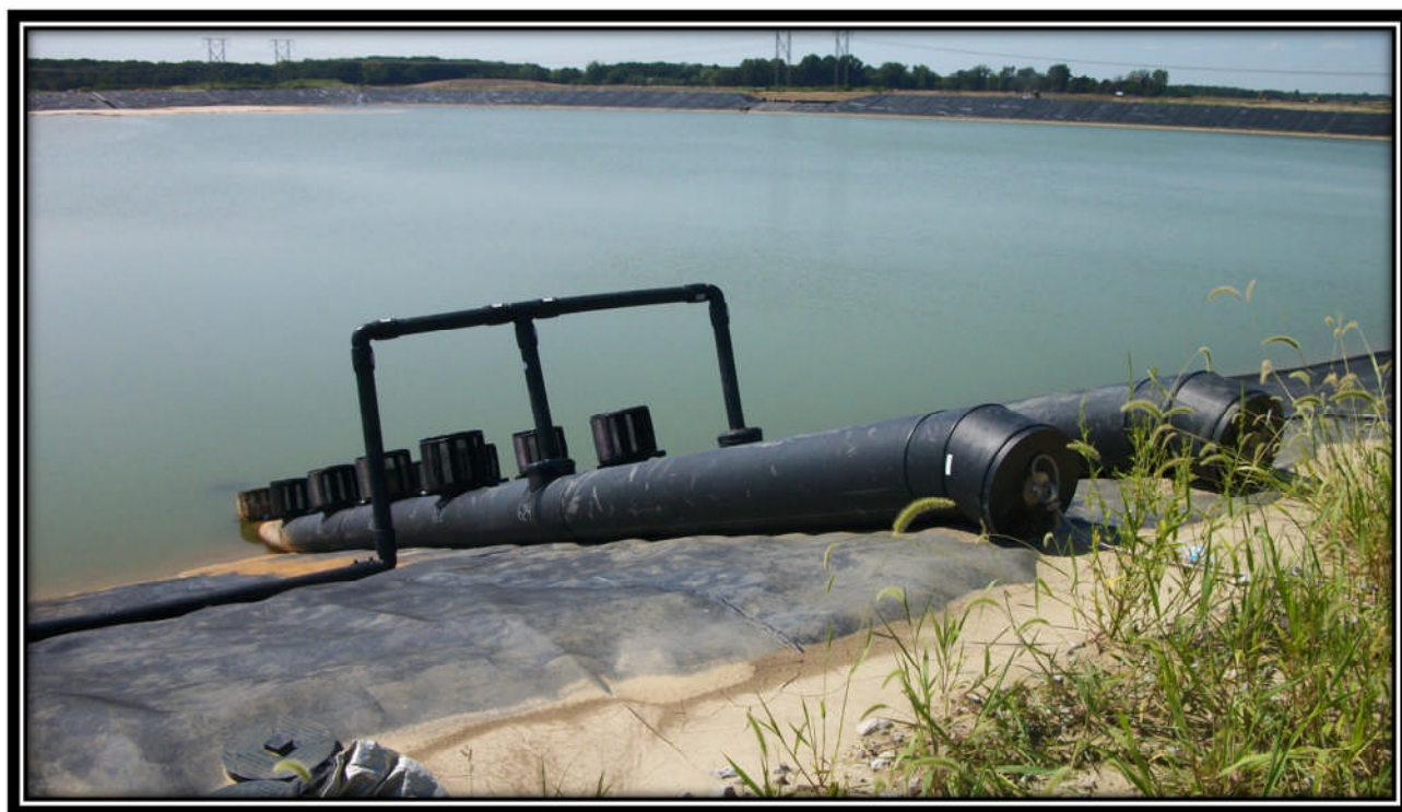
Photo 46 – Inlet of recirculation system
