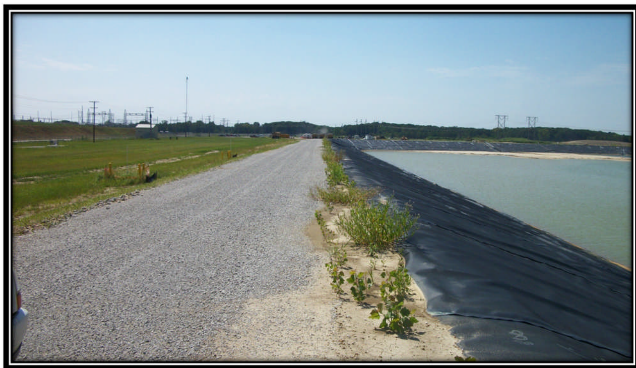
Photo 32 – Looking West along South embankment
