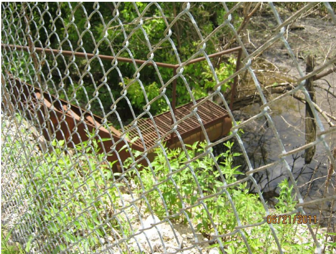
Photograph 2 Outboard Slope at Stability Analysis Cross-Section at SB-3
