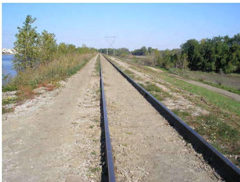
Figure 5.4.1-1: Zero Liquid Discharge Pond East Dike Crest View South to North
