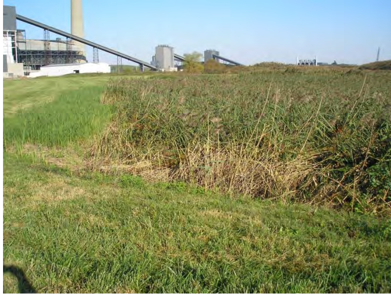
Figure 5.2.4-1: Main Ash Pond South Dike Crest at Western Abutment
