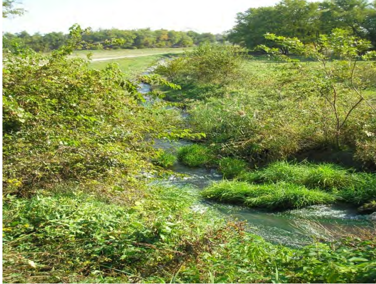
Figure 5.5.2-2: Main Ash Pond Spillway Drainage Ditch from Outfall to Des Moines River.
