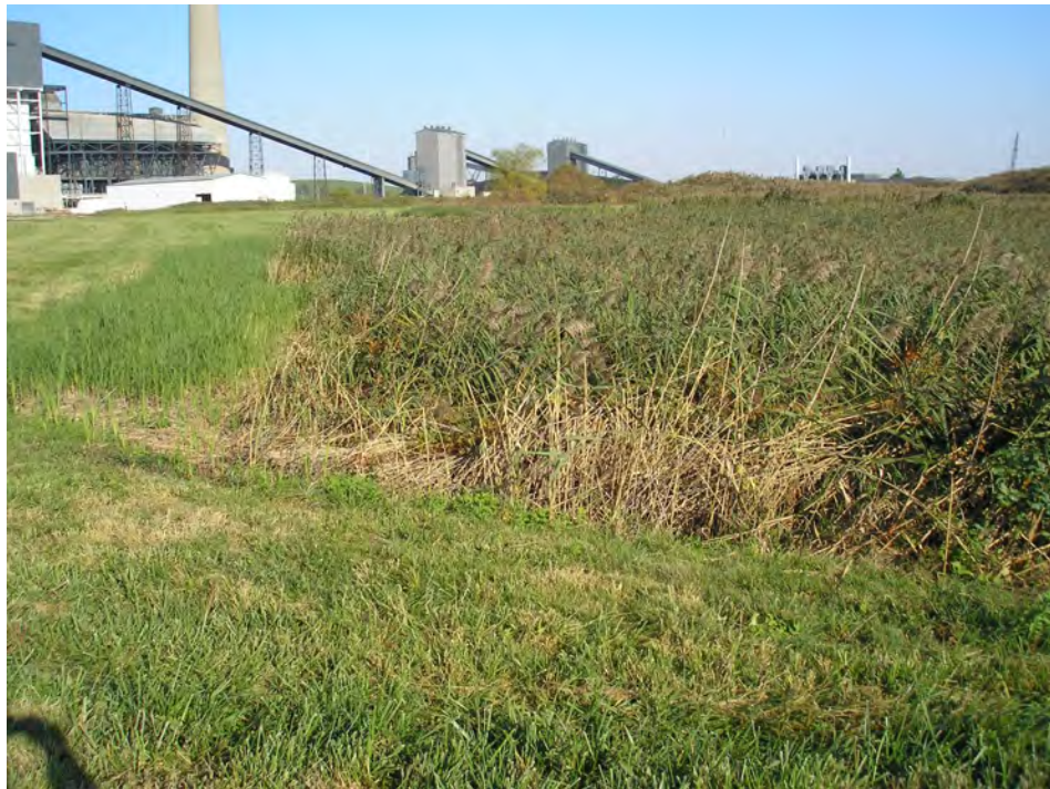
Photograph 1: Main Ash Pond South Dike West Abutment
