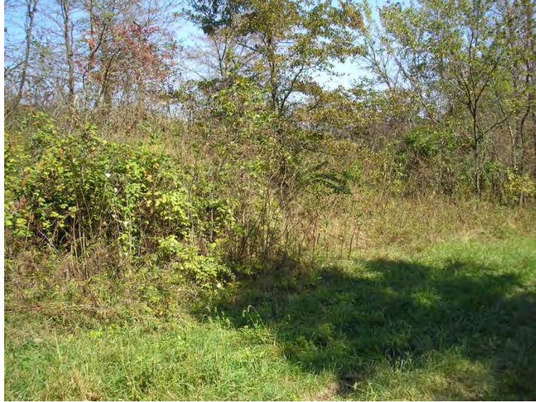
Figure 5.2.3-4: Main Ash Pond South Dike Down-Gradient Toe
