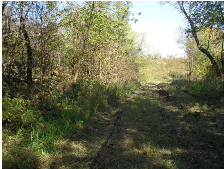
Figure 5.2.3-5: Wet Area at Main Ash Pond South Dike Down Gradient Toe
