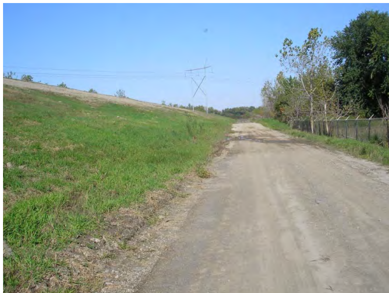
Figure 5.4.3-3: Zero Liquid Discharge Pond East Dike Toe,
