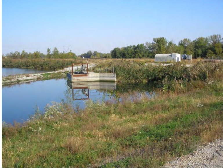
Figure 5.5.1-1 Main Ash Pond Primary Spillway Riser Structure
