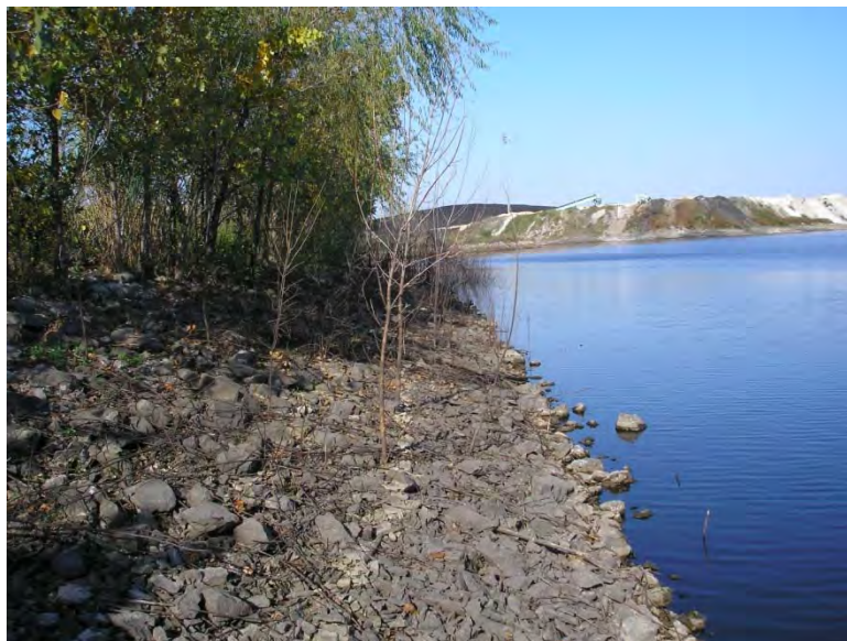
Figure 5.3.3-1: Main Ash Pond North Dike Down-Gradient Slope
