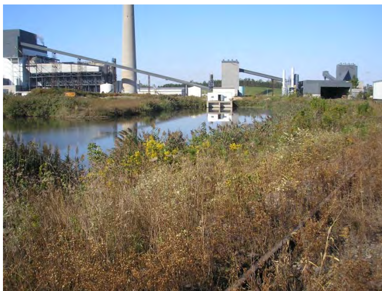
Figure 5.3.4-1: Main Ash Pond North Dike Up-Gradient Slope West Abutment
