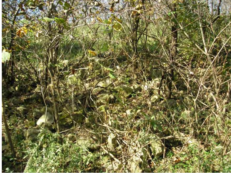
Figure 5.2.3-3: Main Ash Pond South Dike Down-Gradient Slope Riprap Armoring
