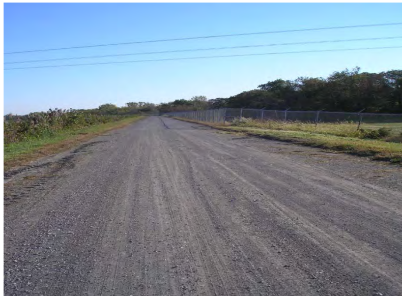
Figure 5.2.1-1: Main Ash Pond South Crest Viewing West to East
