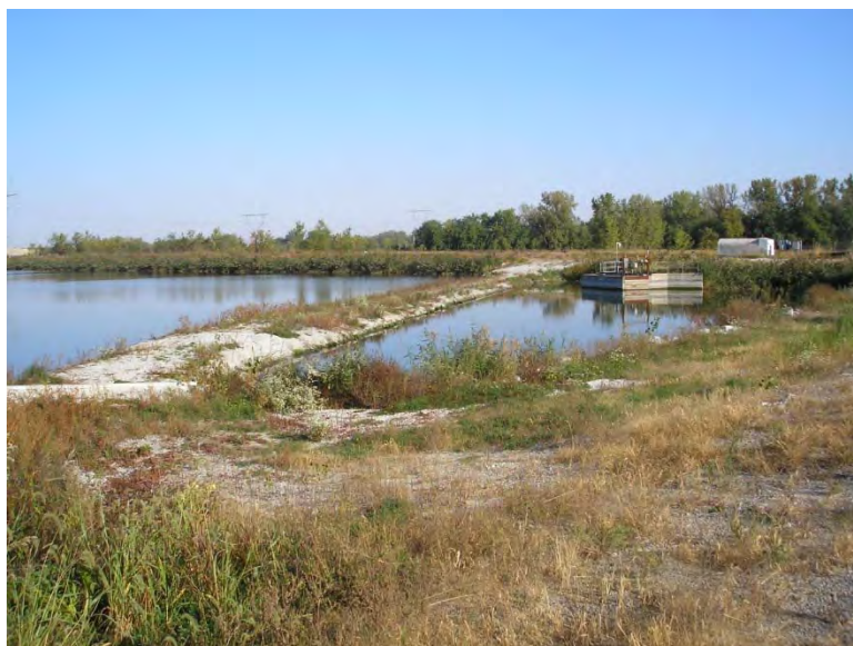
Figure 8.1-1: Low Dike and Final Settling Basin within Main Ash Pond
