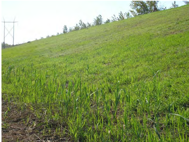
Figure 5.4.3-1: Zero Liquid Discharge Pond: East Bank Down-Gradient Slope
