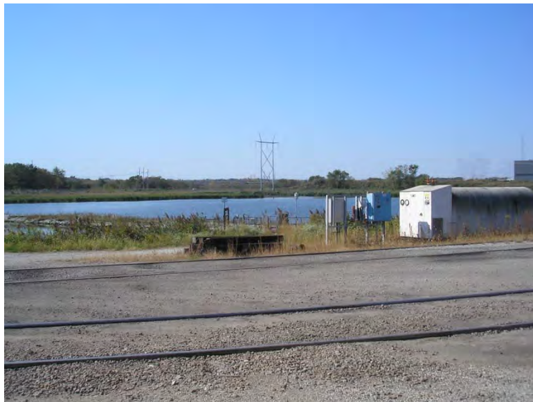
Figure 5.2.4.2: Main Ash Pond South Dike Groin Crest at East End
