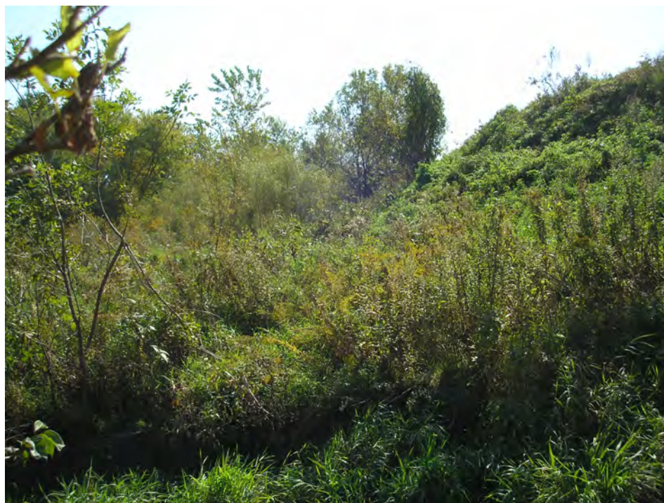
Photograph 4: Main Ash Pond South Dike West End Down-Gradient Slope
