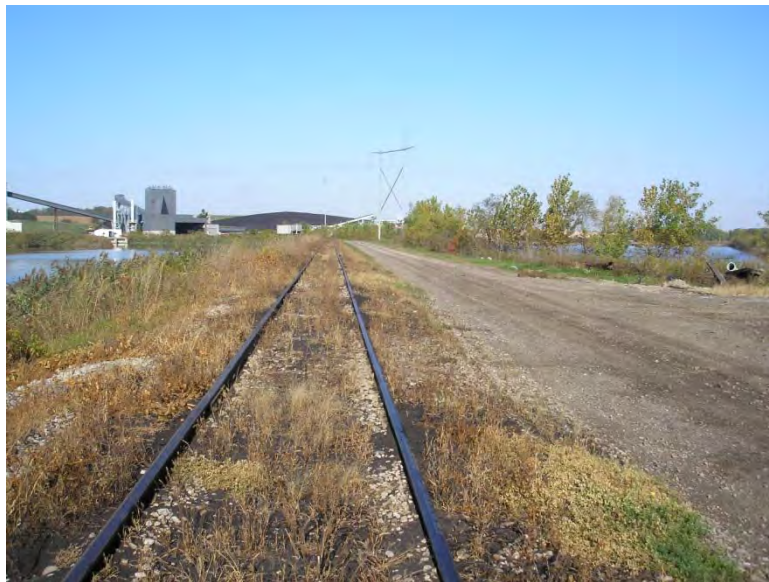
Figure 5.3.1-1: Main Ash Pond North Dike Crest View East to West
