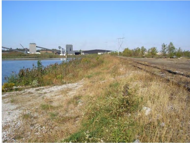
Figure 5.3.2-1: Main Ash Pond Up-Gradient Slope View East to Wet
