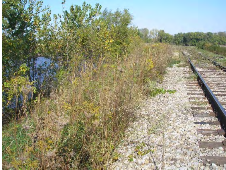
Figure 5.4.2-1: Zero Liquid Discharge Pond East Dike Up-Gradient Slope
