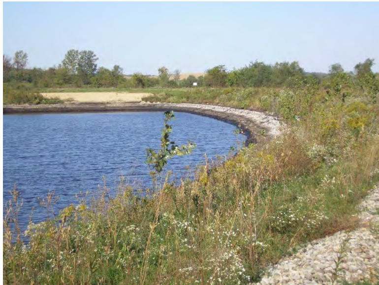
Figure 5.4.4-1: Zero Liquid Discharge Pond East Bank North Abutment Area
