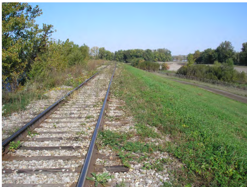
Photograph 6: Zero Liquid Discharge Pond East Dike Crest and Down-Gradient Slope
