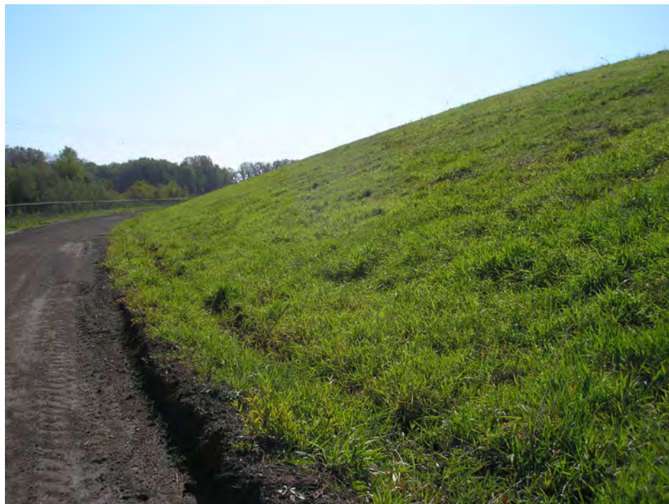
Photograph 7: Zero Discharge Pond East Dike Down-Gradient Slope at North Groin
