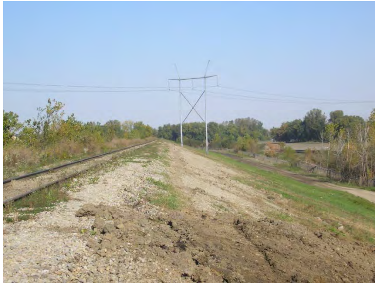
Figure 5.4.3-2: Zero Liquid Discharge Pond East Dike: Re-graded/Re-seeded Area at Top of Down-Gradient Slope
