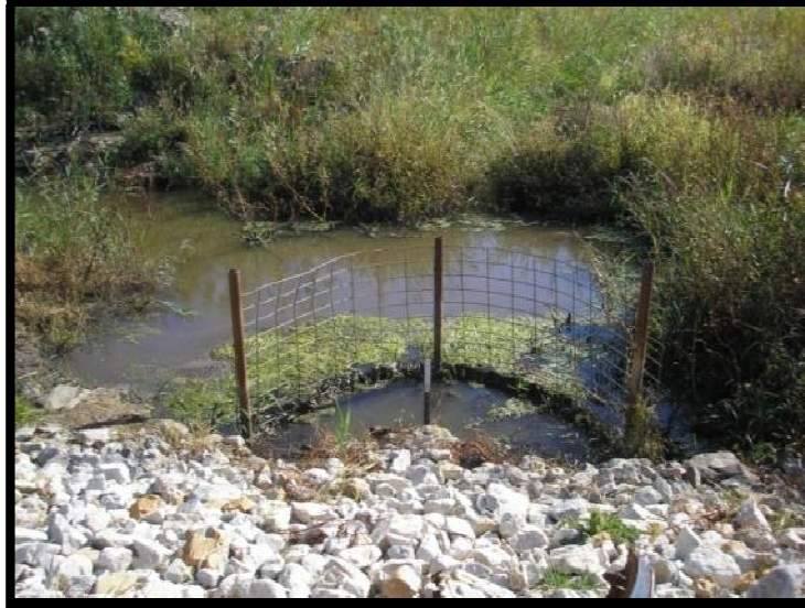
Figure 8.1-3: Economizer Ash Pond Spillway Inlet
