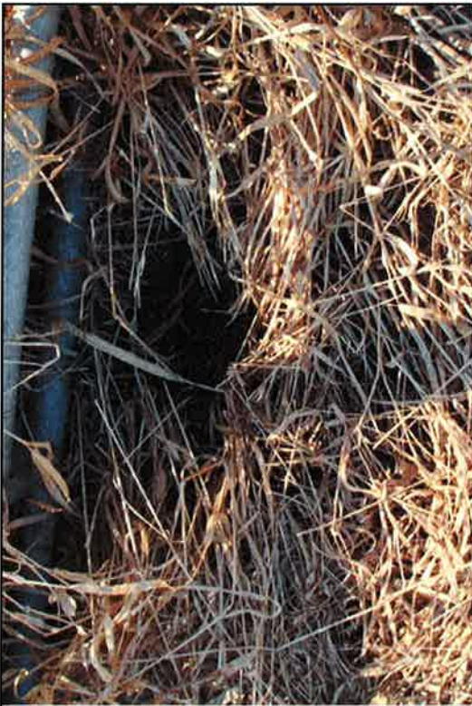
BGS - Ash Pond No.1 Pic #5
