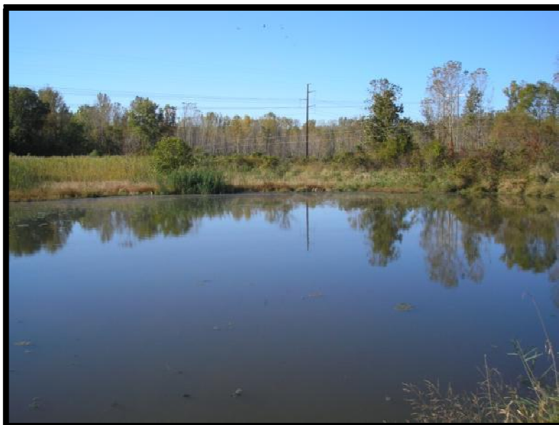
Figure 5.3.2-3: Bottom Ash Pond Upstream Slopes South and West Dikes
