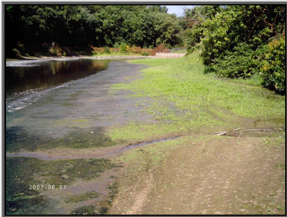
Photo 4) West – Facility Discharge Channel; Continuous Wet Ground after Dry Weather
