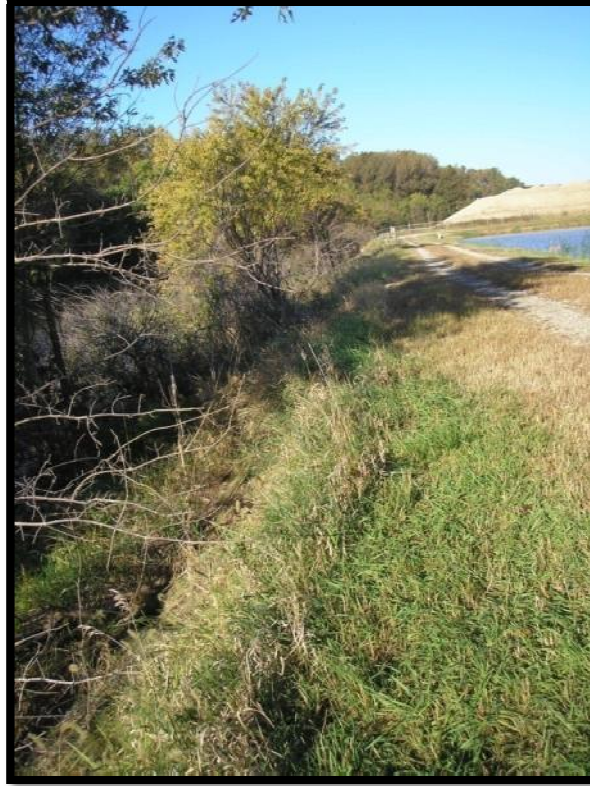
Figure 5.2.3-1: Ash Seal Pond South Dike Outside Slope
