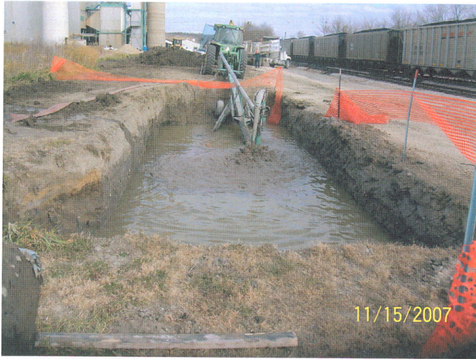
Photograph of bentonite slurry mixing in process.
