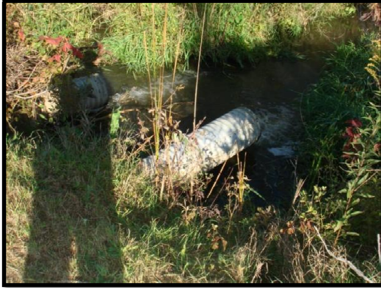
Figure 5.7.2-1: Bottom Ash Pond Spillway Outlet Conduits
