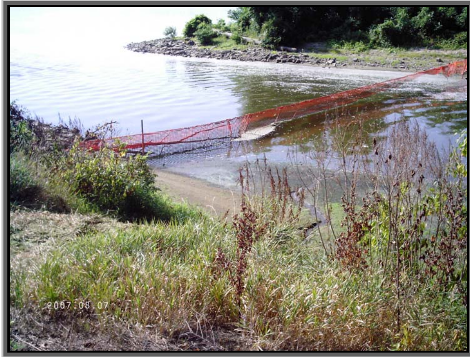
Photo 1) Southeast – Facility Discharge Channel Toward the Mississippi River
