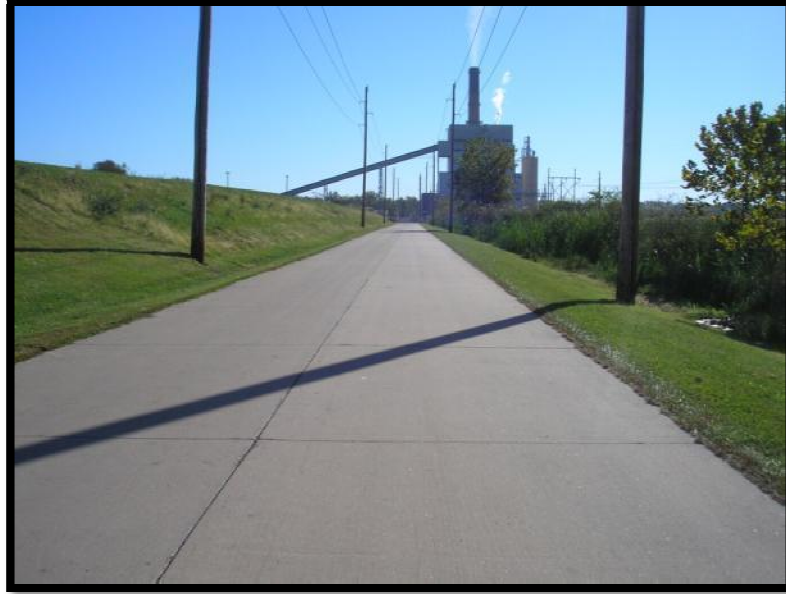
Figure 5.3.1-1: Bottom Ash Pond North Dike Crest
