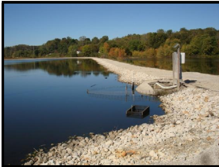
Figure 8.1-4: Ash Pond 1 Primary Spillway Riser
