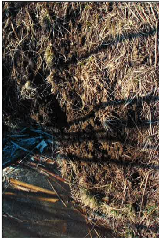
BGS - Ash Pond No.1 Pic #7
