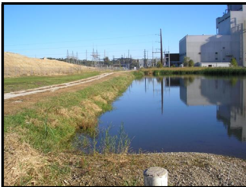
Figure 5.2.3-3: Eco-Stone Storage Pile over Outside Slope Ash Seal Pond West Dike
