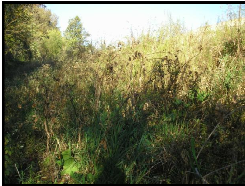
Figure 5.3.3-1: Bottom Ash Pond Downstream Slope South Dike
