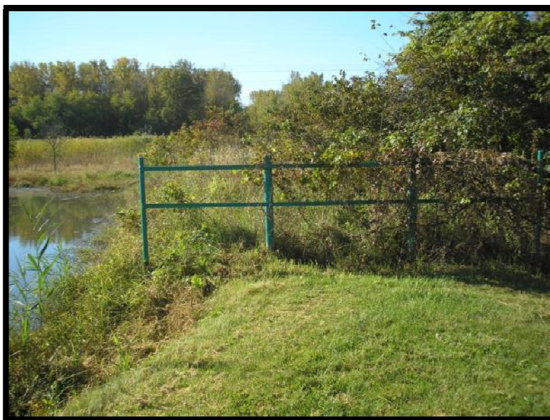
Figure 5.3.1-3: Bottom Ash Pond North End of West Dike
