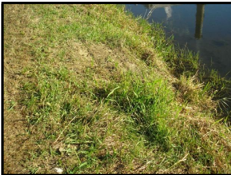
Figure 5.2.2-1: Ash Seal Pond Typical Inside Slope Vegetation Cover
