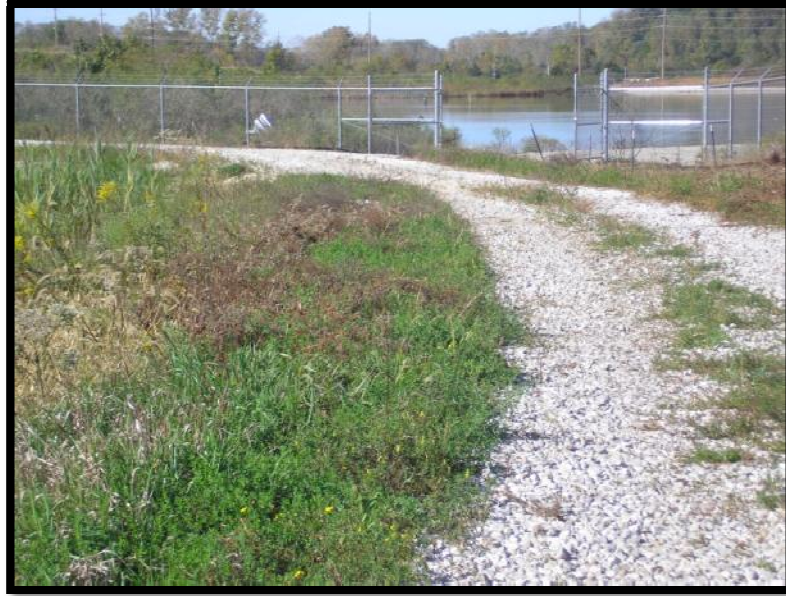
Figure 5.4.4-1: Economizer Ash Pond Crest and Upstream Slope
