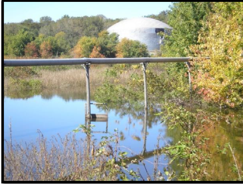
Figure 5.7.1-5: Ash Pond 2 Top of Spillway Stop Log Device
