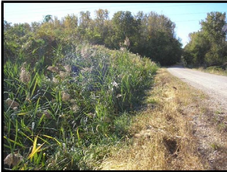
Figure 5.3.3-3: Bottom Ash Pond West Dike Downstream Slope
