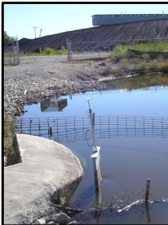
Figure 5.7.1-4: Ash Pond 1 Spillway Location
