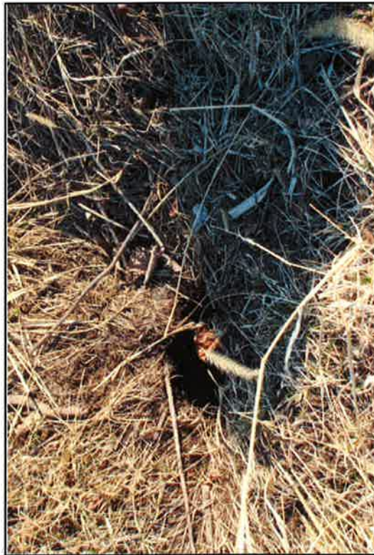
BGS -Ash Pond No.1 Pic #15
