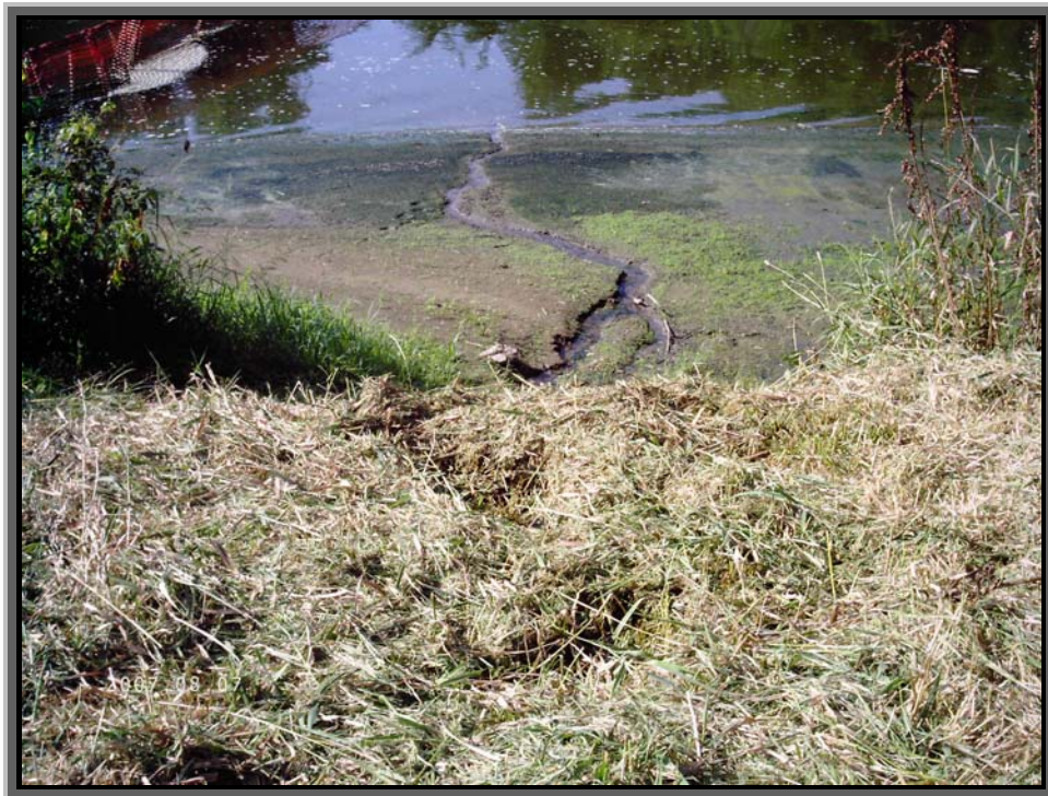
Photo 2) South – Seep Location in from Berm
