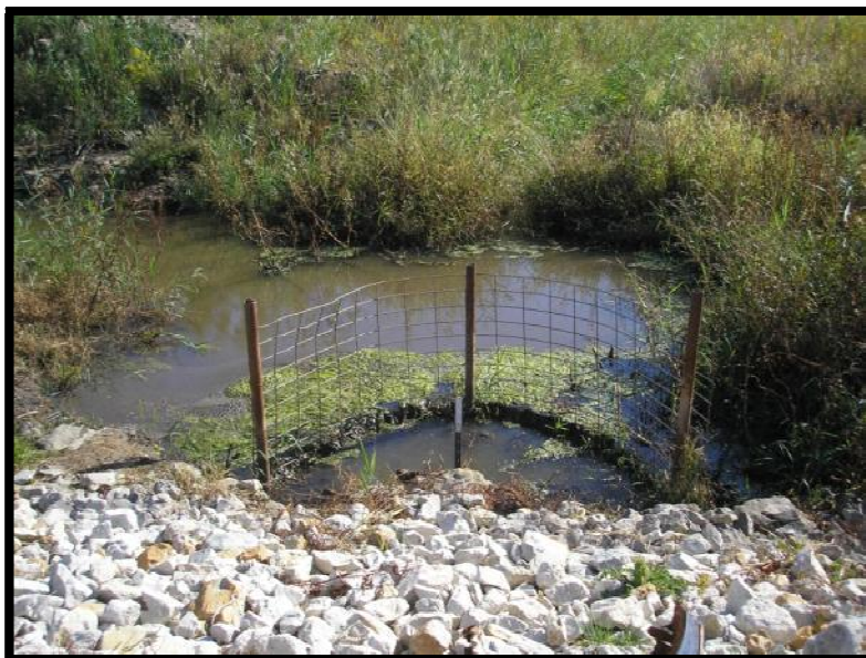
Figure 5.7.1-3: Economizer Ash Pond Spillway Location
