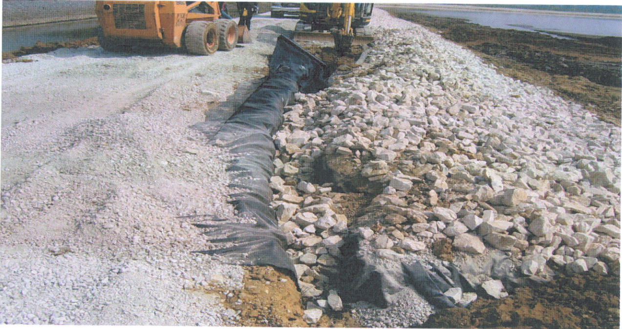
Notching geotextile fabric into top and inside slope
