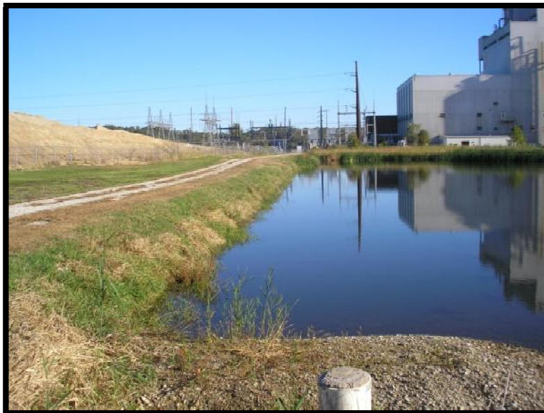
Figure 5.3.2-2: Dry Fly Ash Storage Pile on Bottom Ash East Dike Upstream Slope
