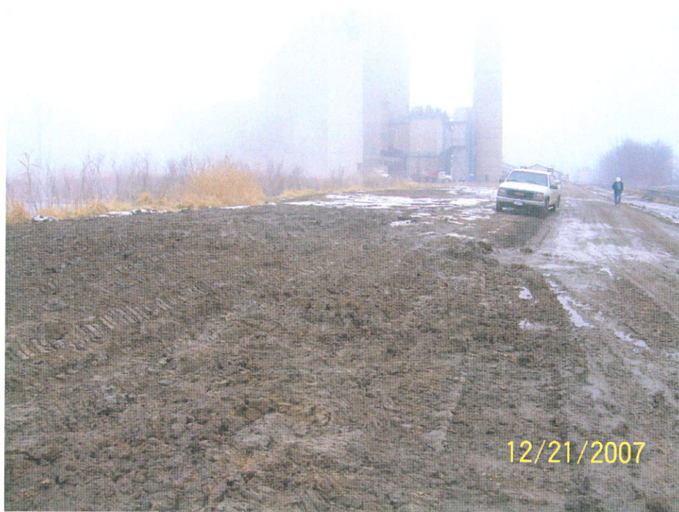
Photograph of filled-in mixing area.
