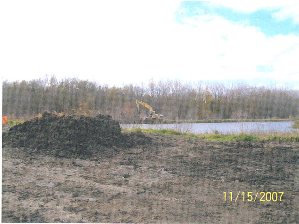
Looking across ash pond at excavator digging slurry trench in ash pond berm.
