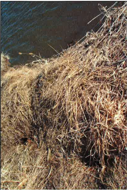
BGS - Ash Pond No.1 Pic #13
