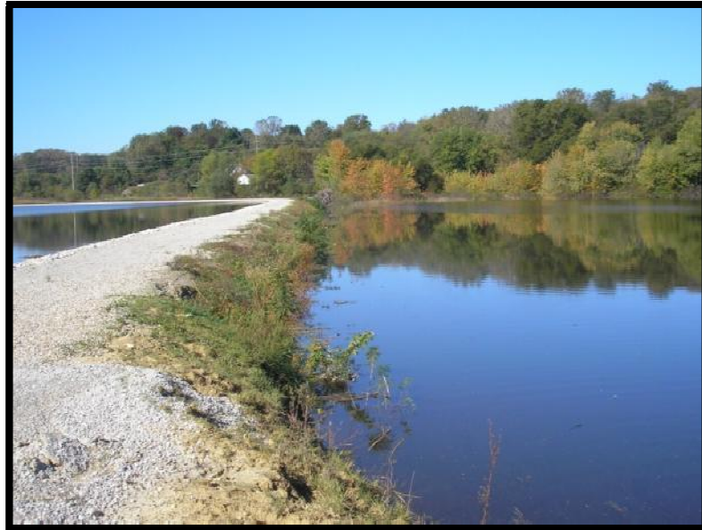
Figure 5.5.3-1: Ash Pond 1 Dike Eastern and Central Section Downstream Slope
