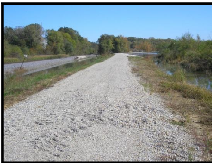
Figure 5.5.1-1: Ash Pond 1 Crest at Southwest End
