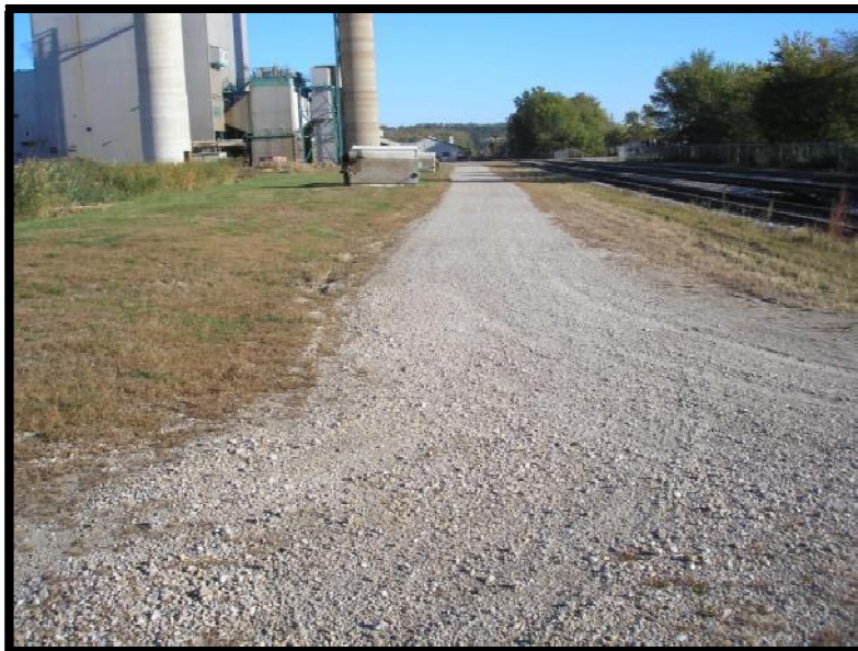
Figure 5.2.1-1: Ash Seal Pond East Dike Crest
