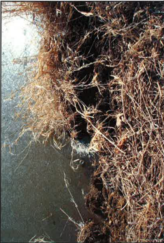
BGS - Ash Pond No.1 Pic #17
