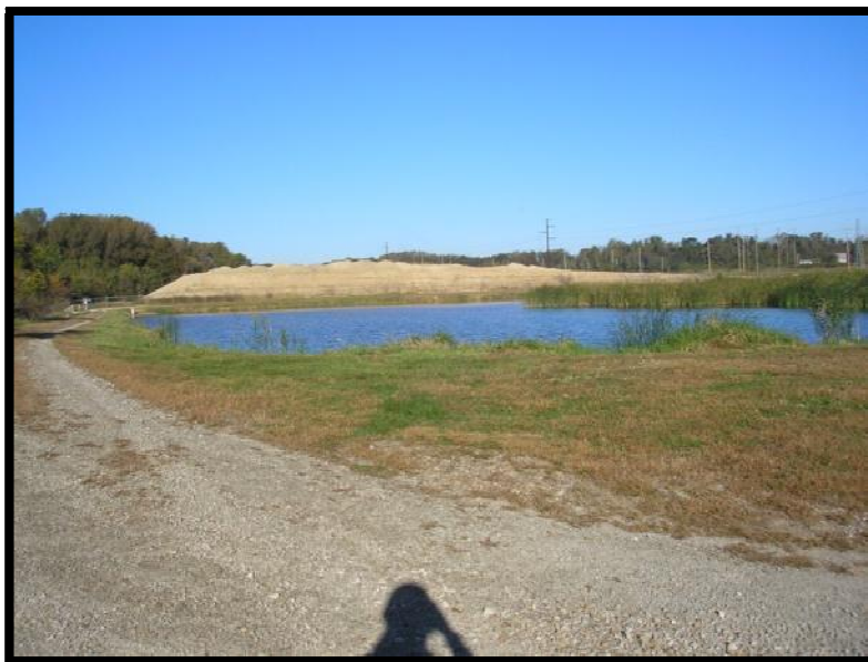
Figure 5.2.1-2: Ash Seal Pond South Dike Crest
