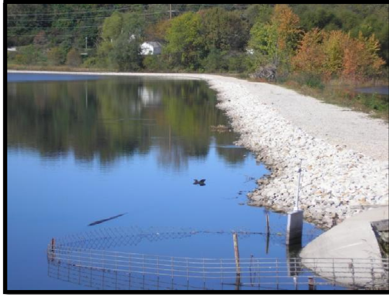
Figure 5.5.2-1: Ash Pond 1 Embankment Upstream Slope
