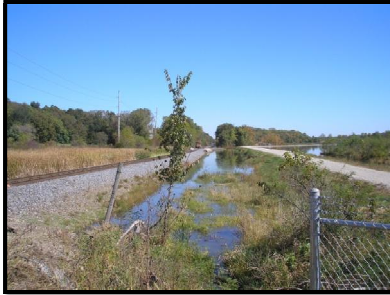
Figure 5.5.4-1: Ash Pond 1 West Abutments
