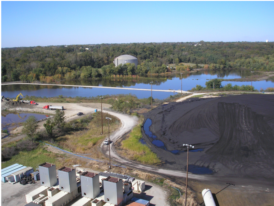
Photograph 6: Rooftop View of Ash Pond 1 Ash Pond 1 Upstream Dike Abutment Located at Construction Equipment. Ash Pond 1 Downstream Dike Located Above Downstream Dike.
