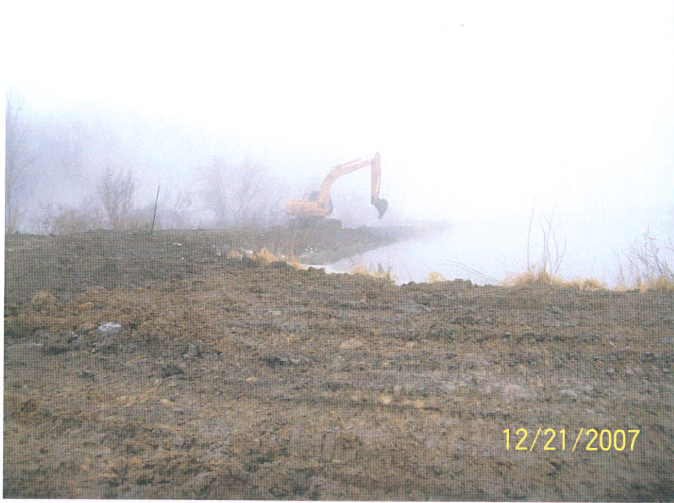
Photograph of final cap placement.
