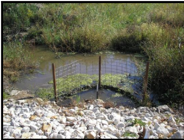
Figure 5.4.4-2: Economizer Ash Pond West Abutment and Pipe Spillway Invert
