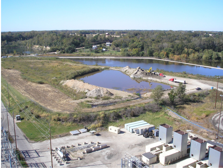
Photograph 5: Rooftop View of Economizer Ash Pond. Economizer Ash Pond in Foreground. Ash Pond 1 in Background
