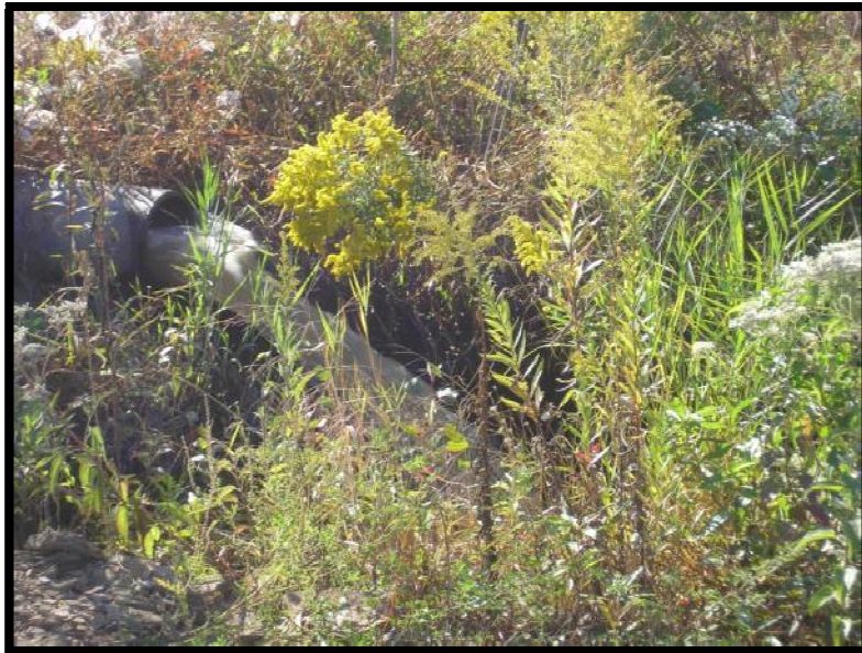
Figure 5.7.2-2: Economizer Ash Pond Spillway Outlet Conduits
