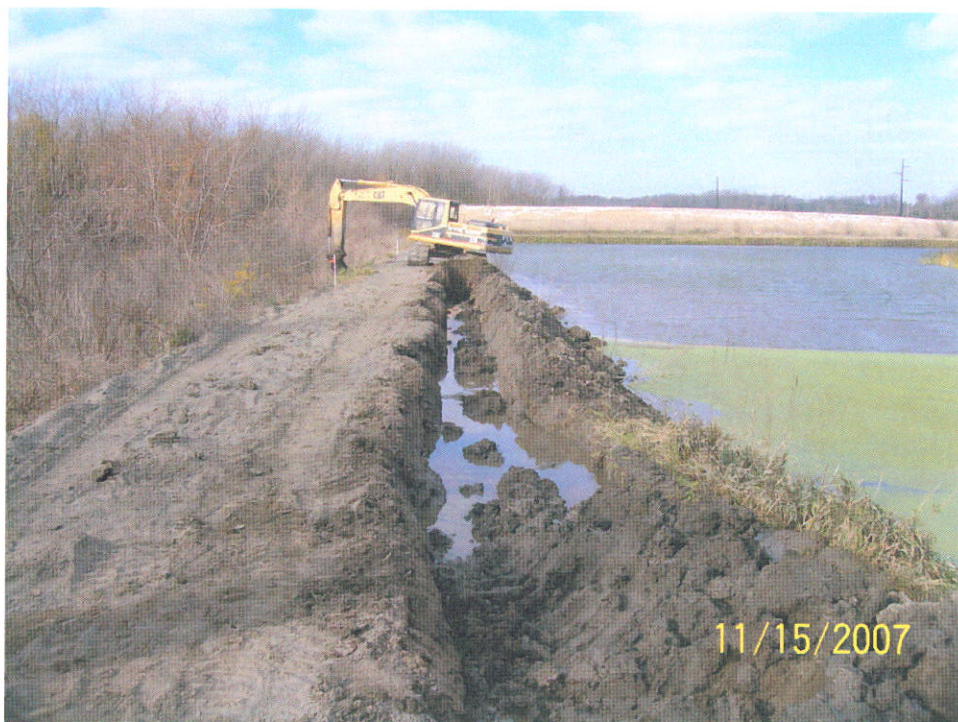
Photograph of slurry trench in berm along ash pond. Standing water is simply the bentonite slurry at the top of the trench.
