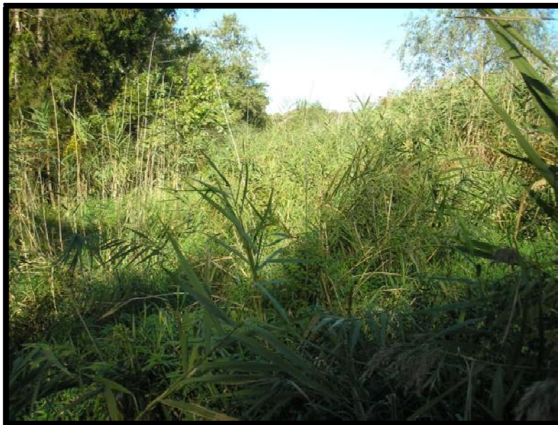
Figure 5.3.1-2: Bottom Ash Pond South Dike Crest.
