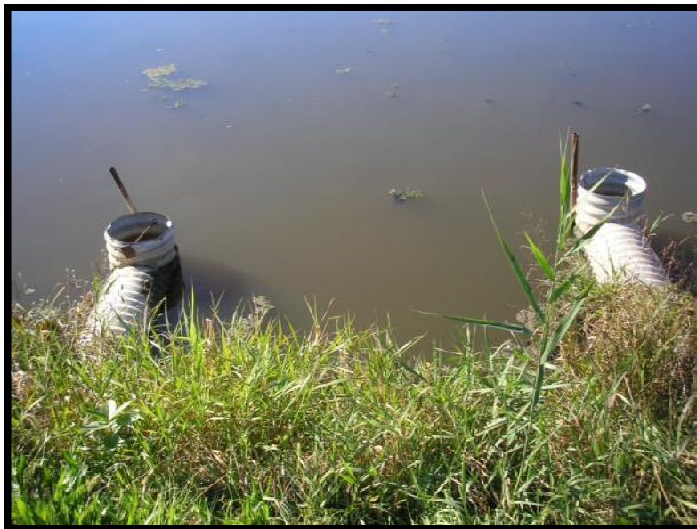
Figure 5.7.1-2: Bottom Ash Pond Primary Spillway Structure
