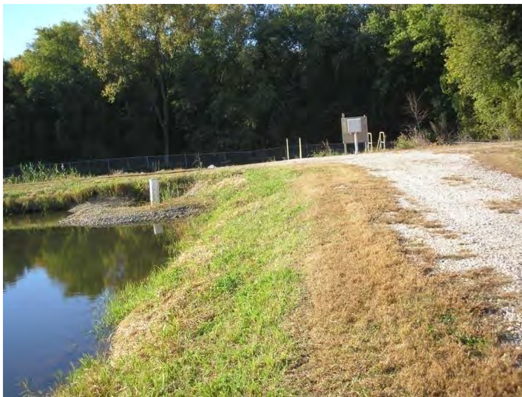
Figure 8.1-1: Ash Seal Pond Interior Low Dike and Spillway Riser
