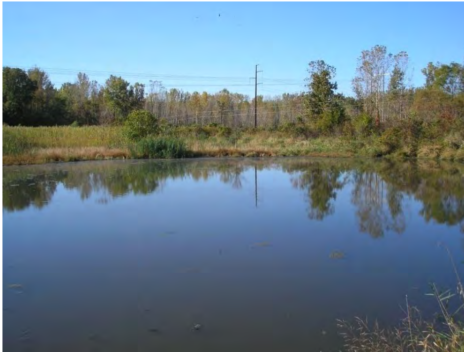
Figure 5.3.2-2: Bottom Ash Pond Upstream Slopes South and West Dikes
