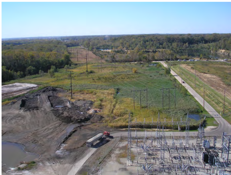
Photograph 4: Rooftop View of North Side of Bottom Ash Pond
