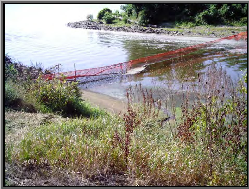
Photo 1) Southeast – Facility Discharge Channel Toward the Mississippi River
