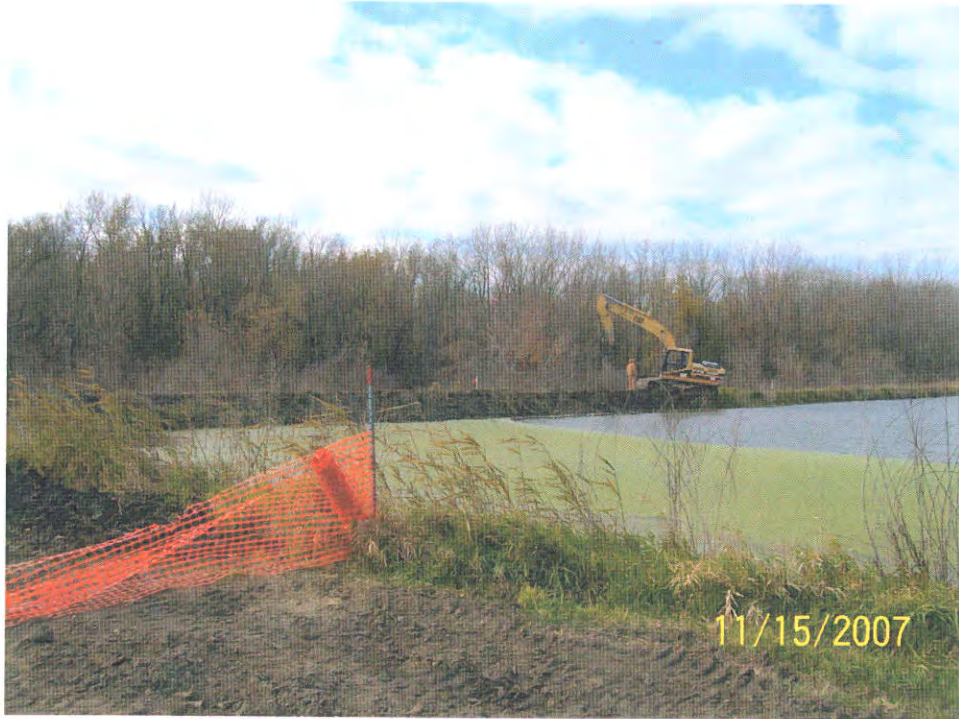
Another photo looking across the ash pond at the excavator digging the slurry trench.
