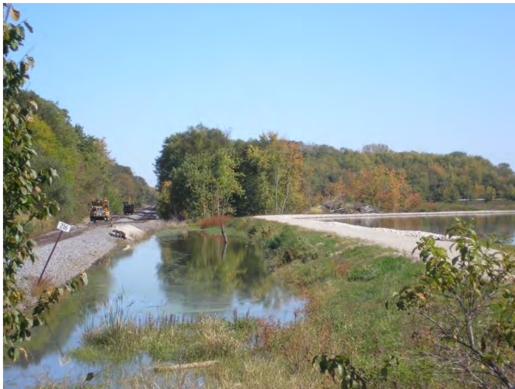
Figure 2.5-1: Railroad Right-of-Way Along West Boundary of Ash Pond 1.
