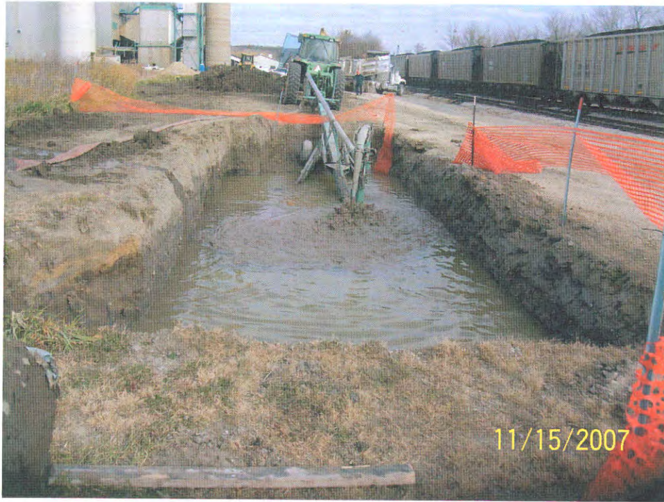
Photograph of bentonite slurry mixing in process.
