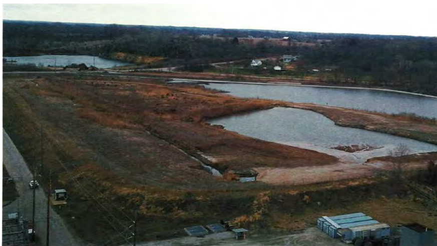
Figure 10.4.1-2: Economizer Ash Pond with Stockpile and Construction Equipment Removed. (Photo courtesy of Burlington Generating Station)
