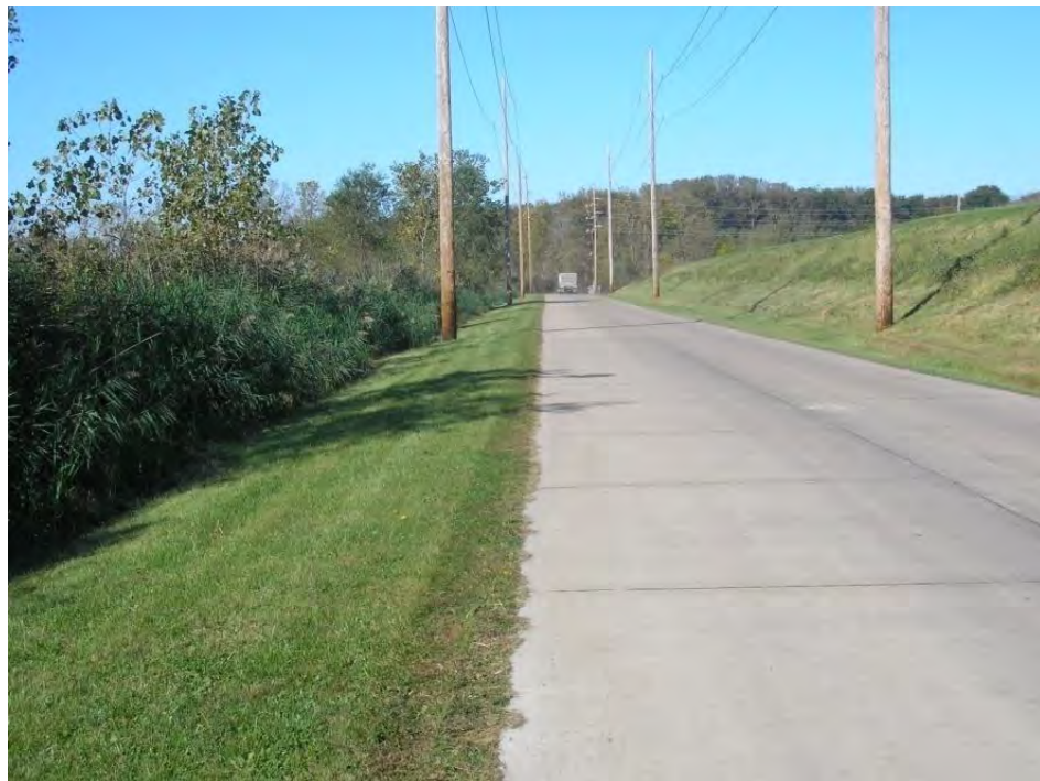
Figure 5.3.2-1: Bottom Ash Pond North Dike Upstream Slope
