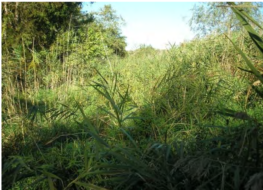
Figure 5.3.1-2: Bottom Ash Pond South Dike Crest.
