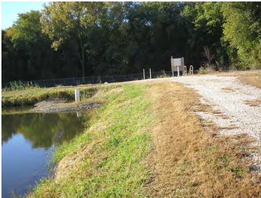
Figure 5.7.1-1: Ash Seal Pond Primary Spillway Structure.
