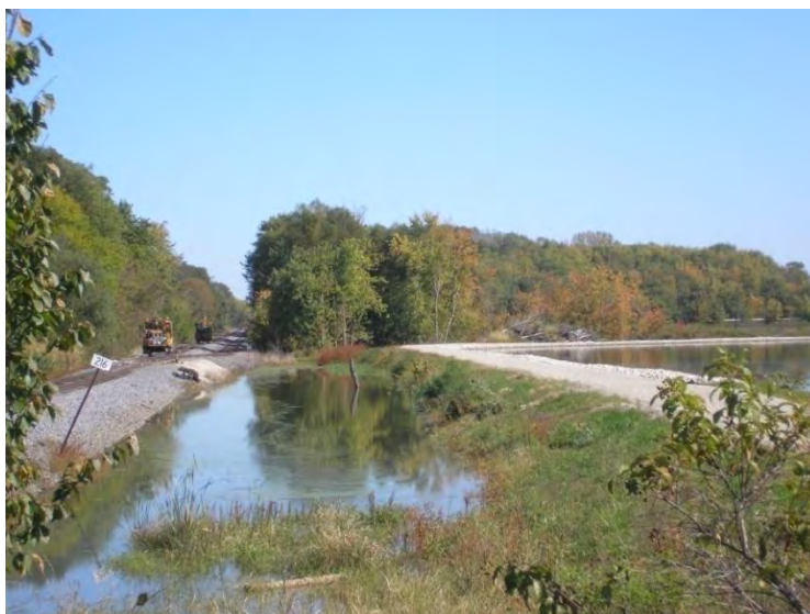
Figure 5.5.3-2: Ash Pond 1 West Section Downstream Slope
