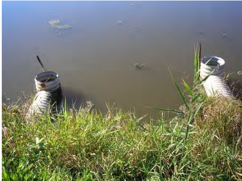
Figure 5.7.1-2: Bottom Ash Pond Primary Spillway Structure
