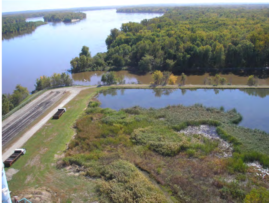
Photograph 1: Rooftop View of East Side of Ash Seal Pond
