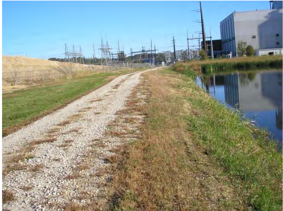
Figure 5.2.1-3: Ash Seal Pond West Dike Crest and Inside Slope
