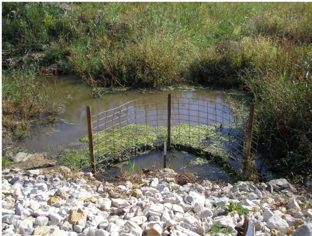
Figure 8-1-3: Economizer Ash Pond Spillway Inlet
