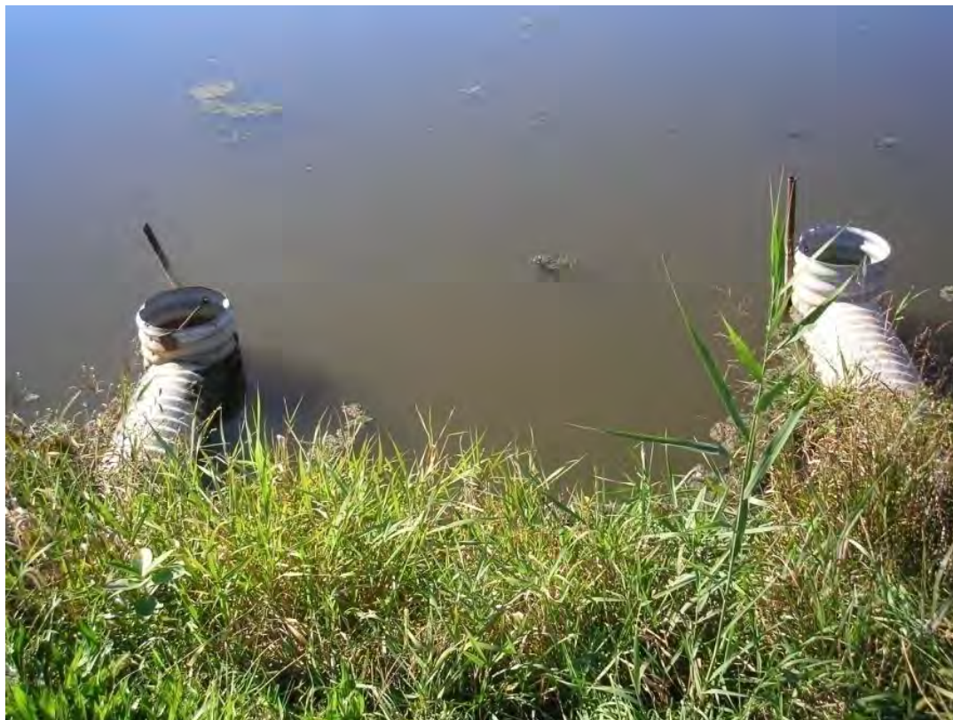
Figure 8.1-2: Bottom Ash Pond Primary Spillway Inlet
