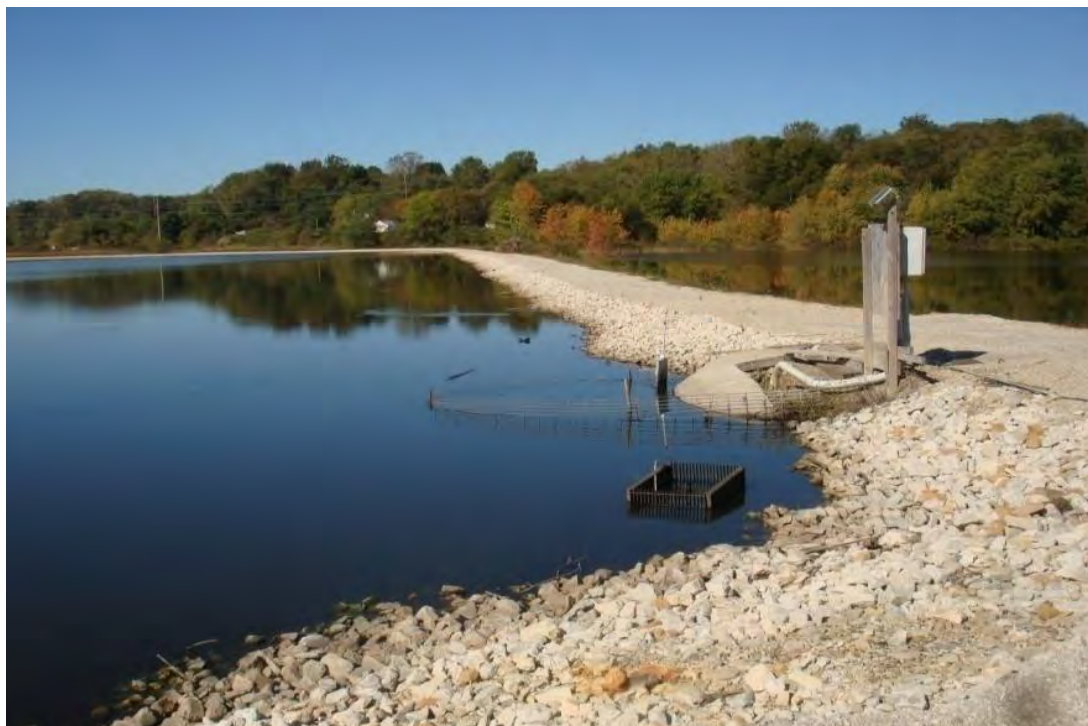
Figure 8.1-4: Ash Pond 1 Primary Spillway Riser
