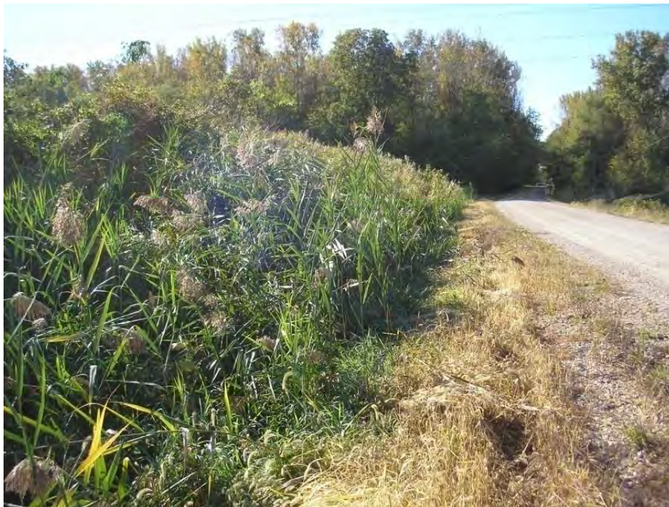
Figure 5.3.3-3: Bottom Ash Pond West Dike Downstream Slope
