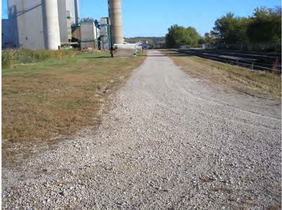
Figure 5.2.1-1: Ash Seal Pond East Dike Crest
