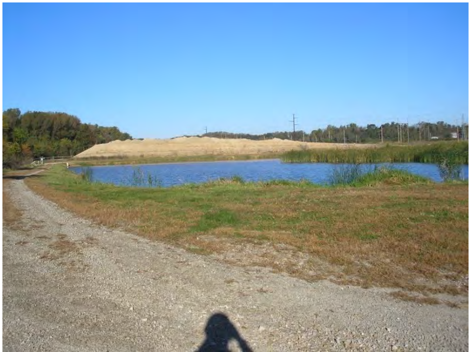
Figure 5.2.1-2: Ash Seal Pond South Dike Crest
