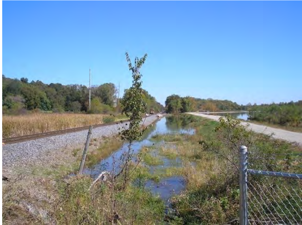
Figure 5.5.4-1: Ash Pond 1 West Abutment
