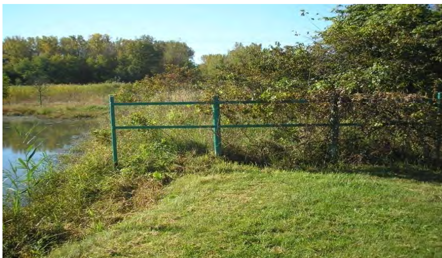
Figure 5.3.1-3: Bottom Ash Pond North End of West Dike
