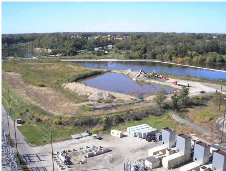
Photograph 5: Rooftop View of Economizer Ash Pond. Economizer Ash Pond in Foreground. Ash Pond 1 in Background
