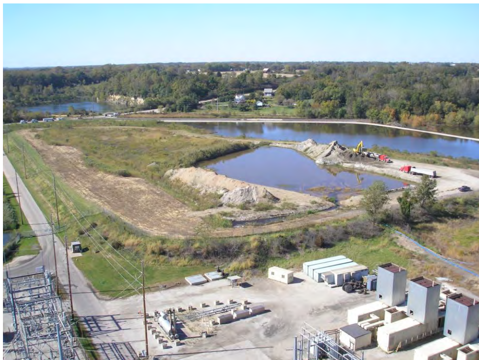
Figure 5.4.1-1: Overhead View of Economizer Ash Pond Crest with Dredging Equipment.
