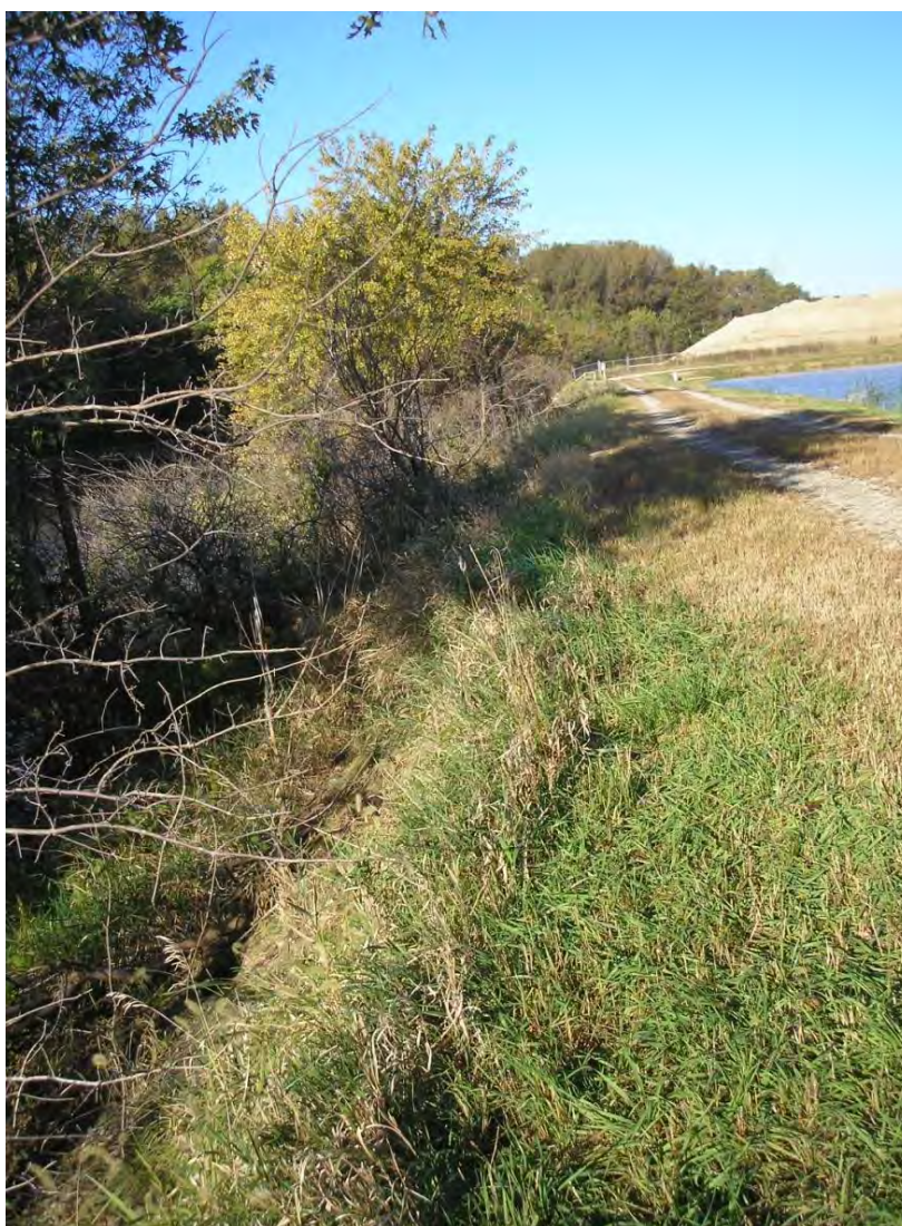
Figure 5.2.3-1: Ash Seal Pond South Dike Outside Slope
