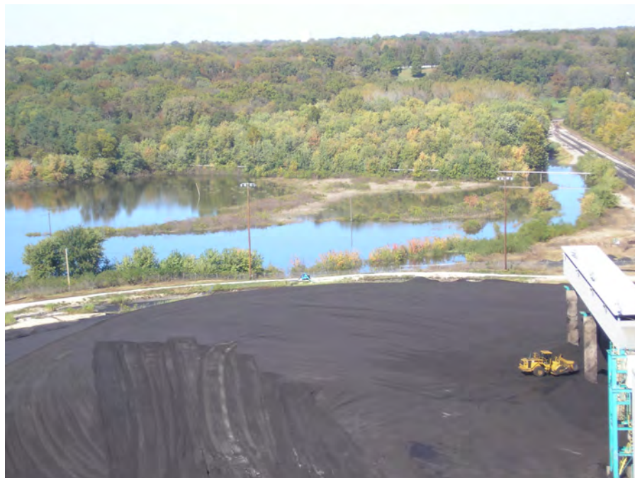
Photograph 7: Rooftop View of Ash Pond 2. Downstream Dike Located beneath Pipe Crossing in Upper Right. Dike Inundated by Flood Water from Mississippi River
