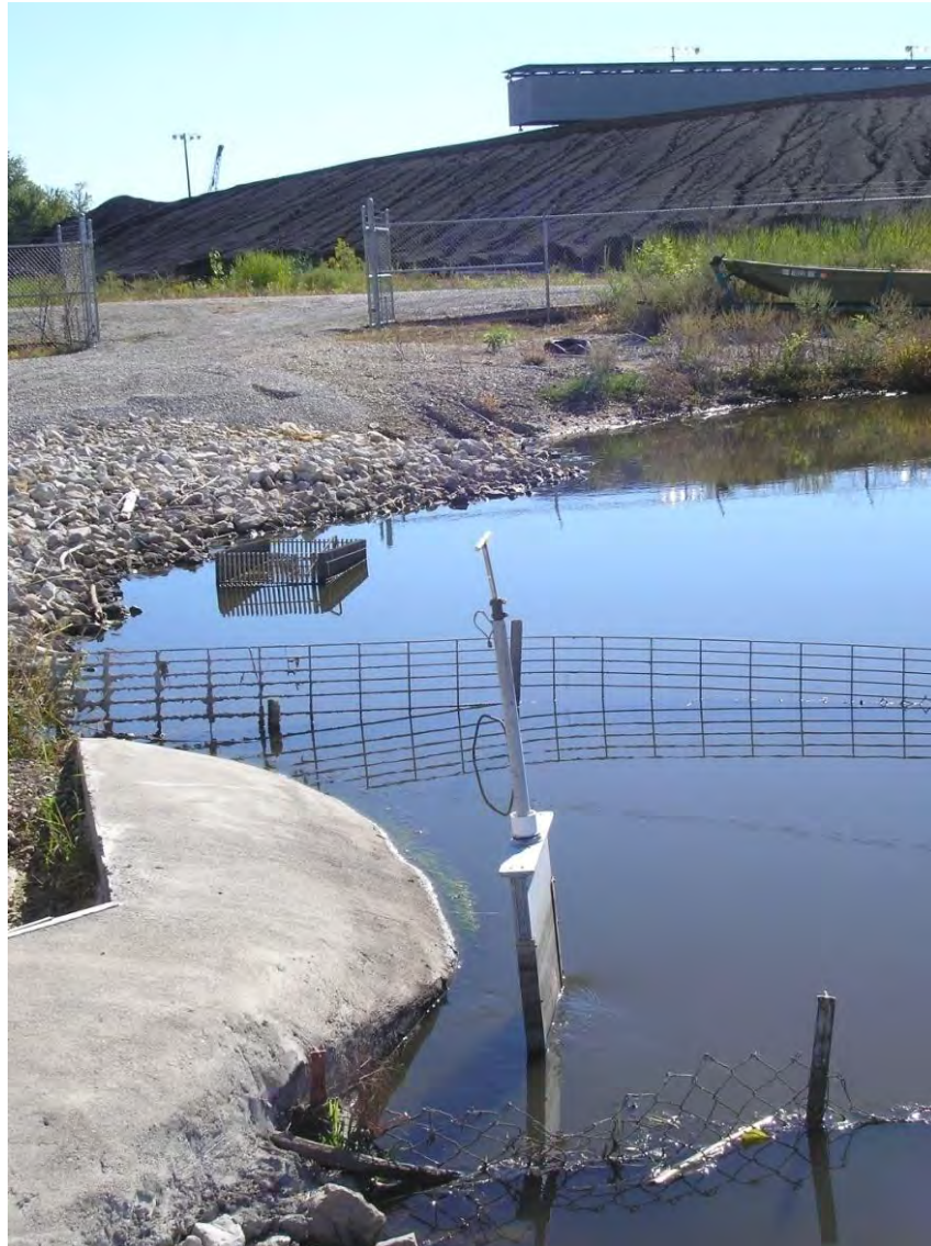
Figure 5.7.1-4: Ash Pond 1 Spillway Location
