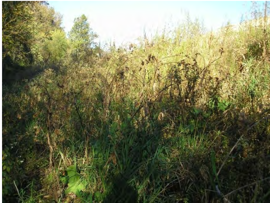
Figure 5.3.3-1: Bottom Ash Pond Downstream Slope South Dike
