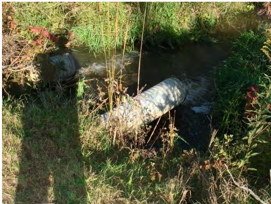
Figure 5.7.2-1: Bottom Ash Pond Spillway Outlet Conduits
