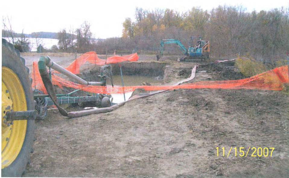
Photograph of bentonite slurry mixing pit. The Mississippi River is at background left and the ash pond is at far right.
