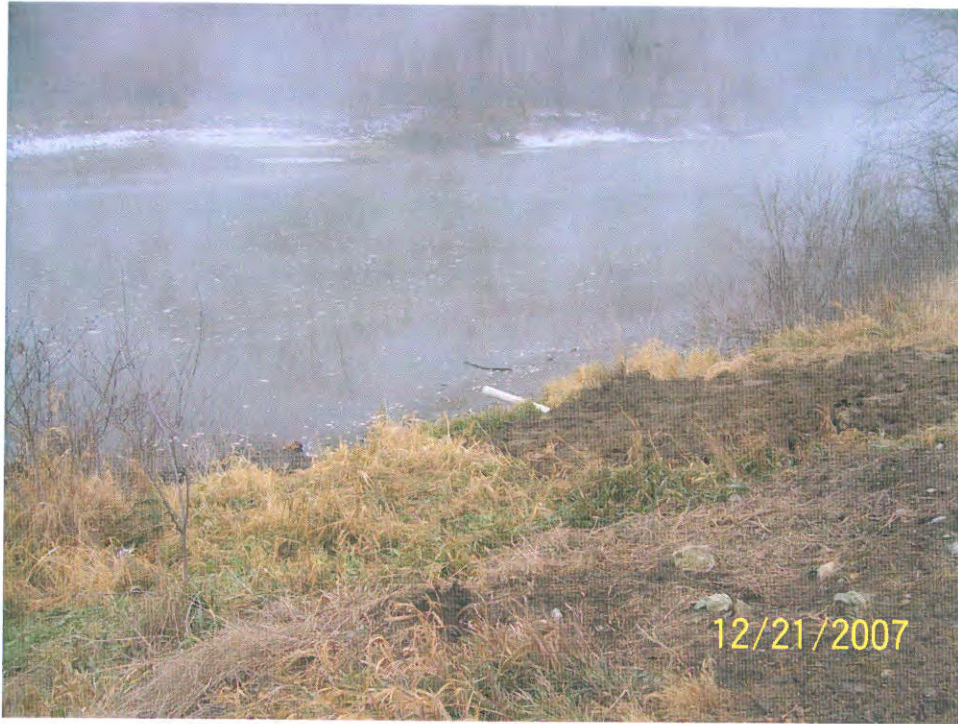
Photograph of drain tile outfall pipe. Old drain tile was determined to be the source of the seep. It was properly plumbed out to daylight so it can be observed in the future.
