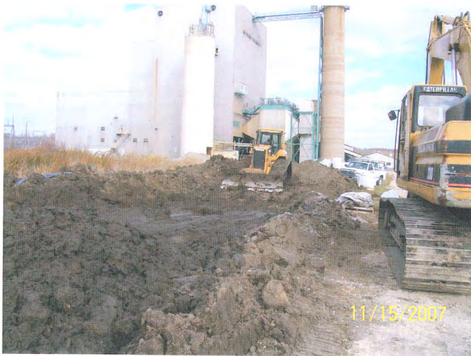
Another view of soil/bentonite mixing pit with generating station in background.
