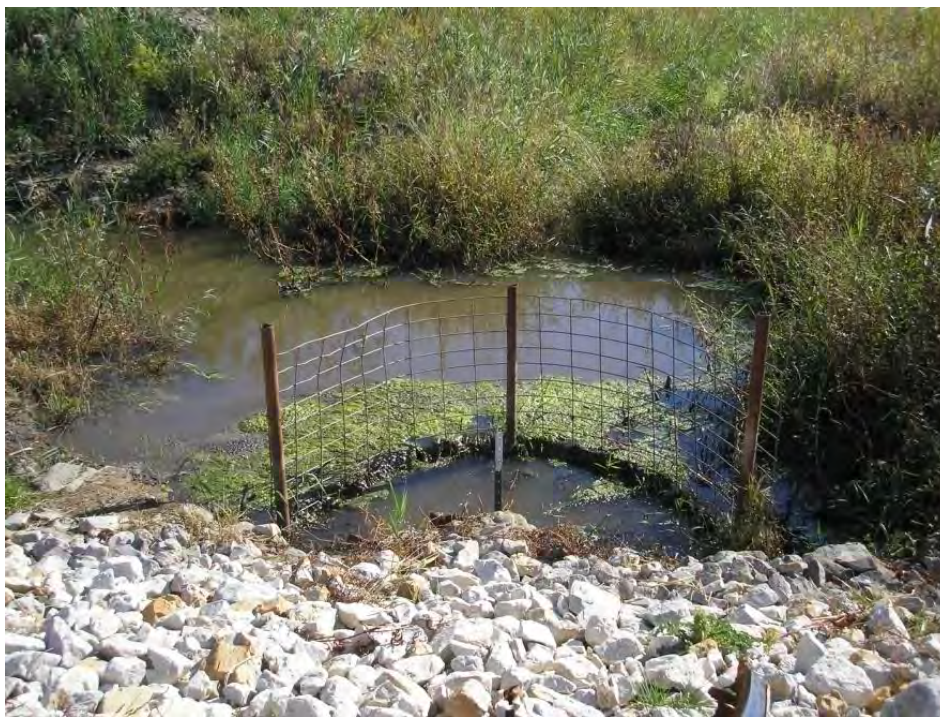
Figure 5.4.4-1: Economizer Ash Pond West Abutment and Pipe Spillway Invert
