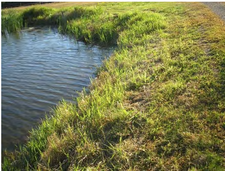
Figure 5.2.4-1: Ash Seal Pond inside Groin at Southeast Corner
