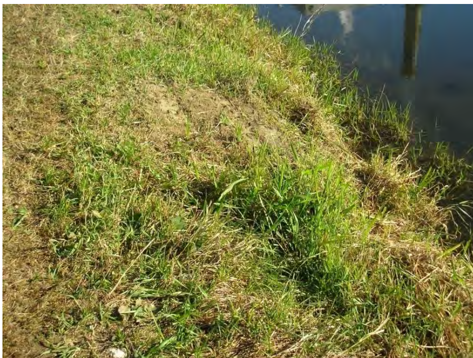
Figure 5.2.2-1: Ash Seal Pond Typical Inside Slope Vegetation Cover
