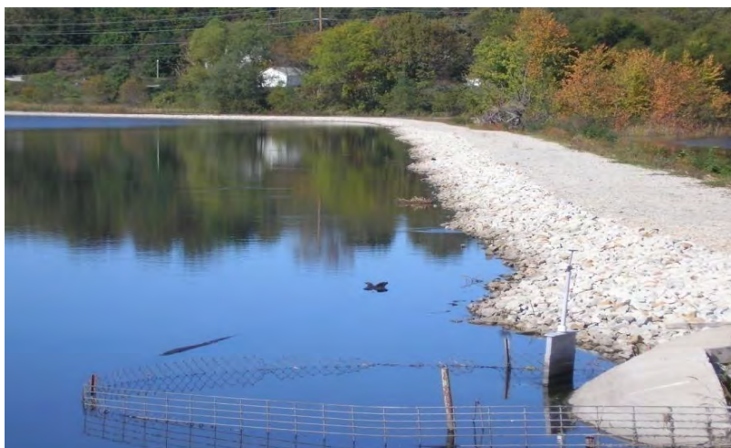
Figure 5.5.2-1: Ash Pond 1 Embankment Upstream Slope
