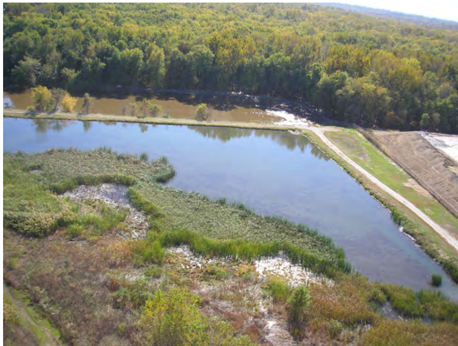
Photograph 2: Rooftop View of West Side of Ash Seal Pond
