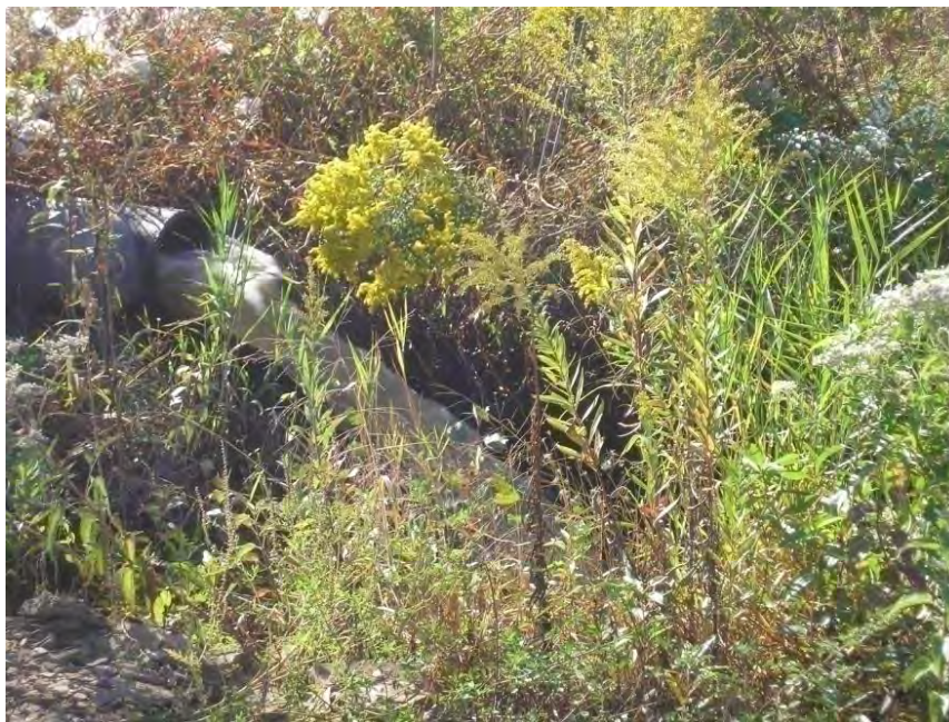
Figure 5.7.2-2: Economizer Ash Pond Spillway Outlet Conduits
