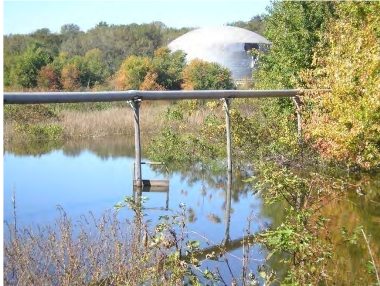
Figure 5.6.1-1: Ash Pond 2 Dike Crest Location beneath Pipe Support Columns.
