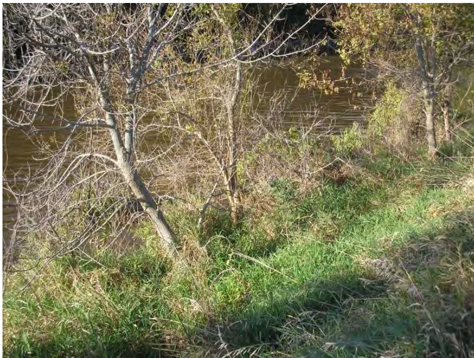
Figure 5.2.3-2: Ash Seal Pond South Dike: Canal High Water against Toe of Outside Slope
