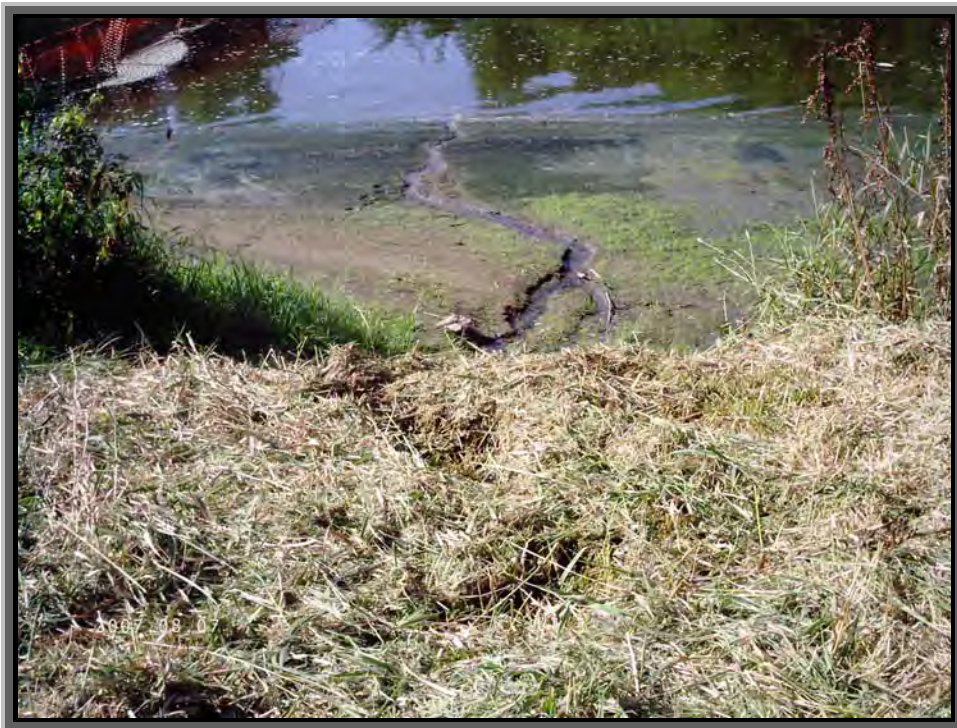
Photo 2) South – Seep Location in from Berm
