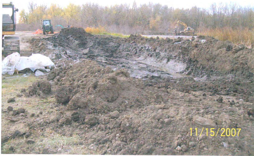
Soil/bentonite mixing pit. Slurry trench excavation is visible in background.
