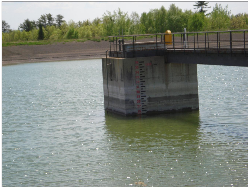
OUTLET STRUCTURE FOR BOTTOM ASH POND
