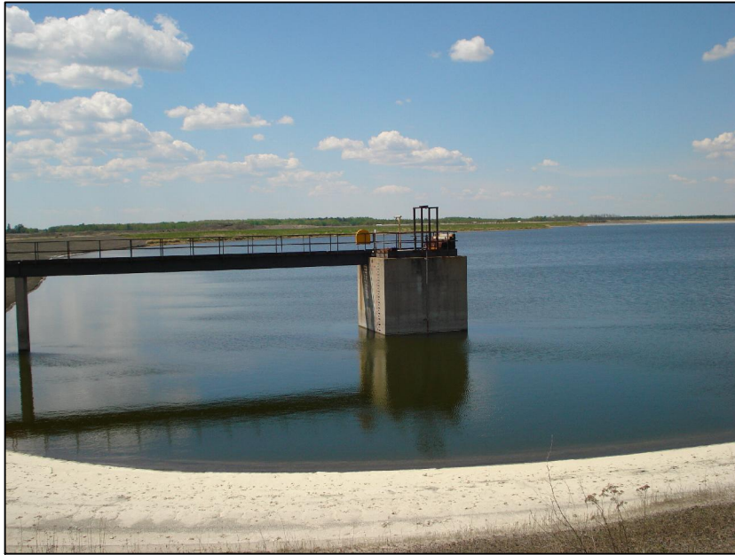
1-37 OUTLET STRUCTURE FOR POND 4
