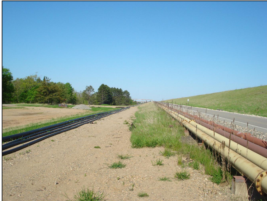
1-5 FROM TOE OF SOUTHEAST DIKE LOOKING WEST
