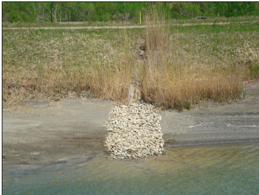
OUTLET DRAIN FOR PUMP HOUSE ALONG SOUTHEASTERN DOWNSTREAM TOE
